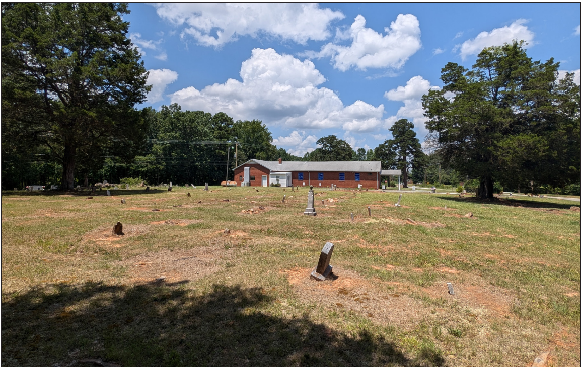
B. South Elevation Showing Cemetery Looking North
