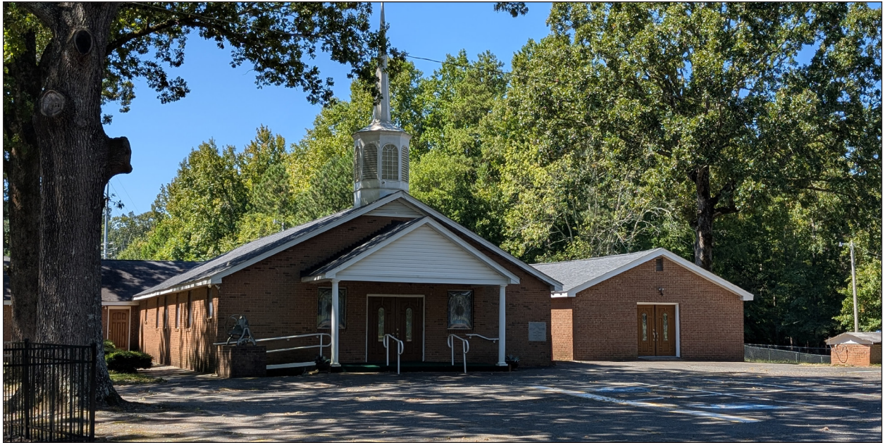
A. Façade, Looking Southwest
