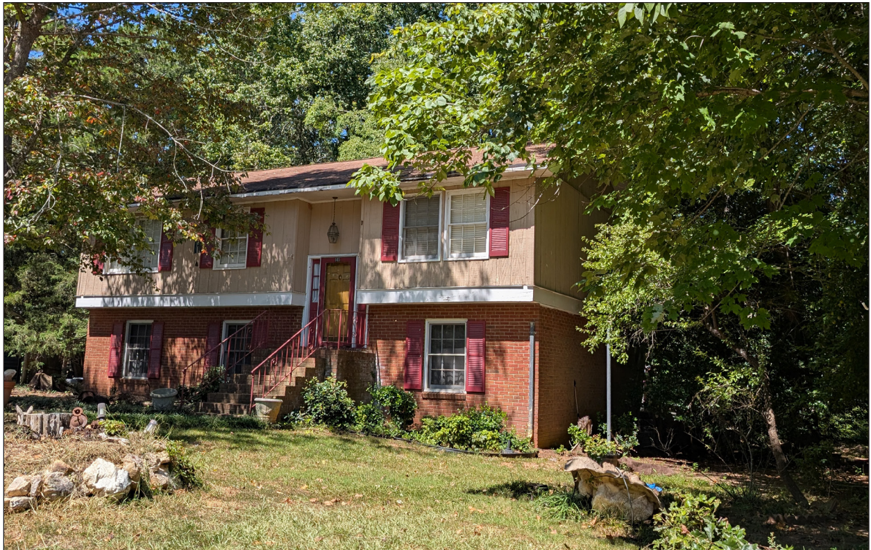
B. Façade and East Elevation, Looking Northwest
