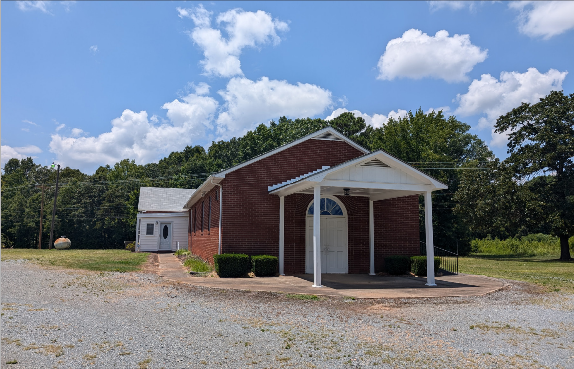
A. Façade, Looking West
