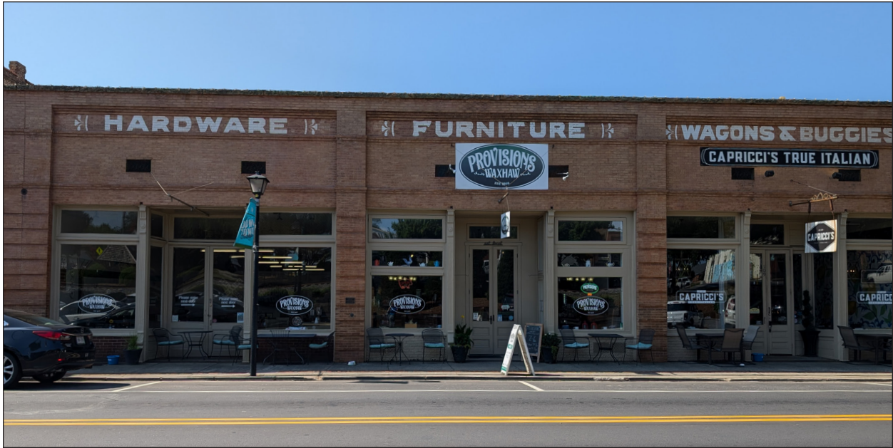
A. Façade, Looking South. (The theater was the center storefront.)
