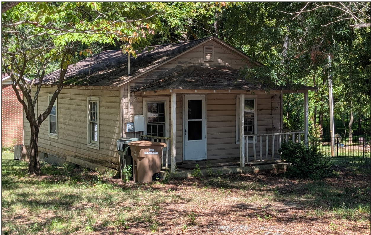
B. Additional Dwelling on Corner of Washington Street and East Price Street, Looking North
