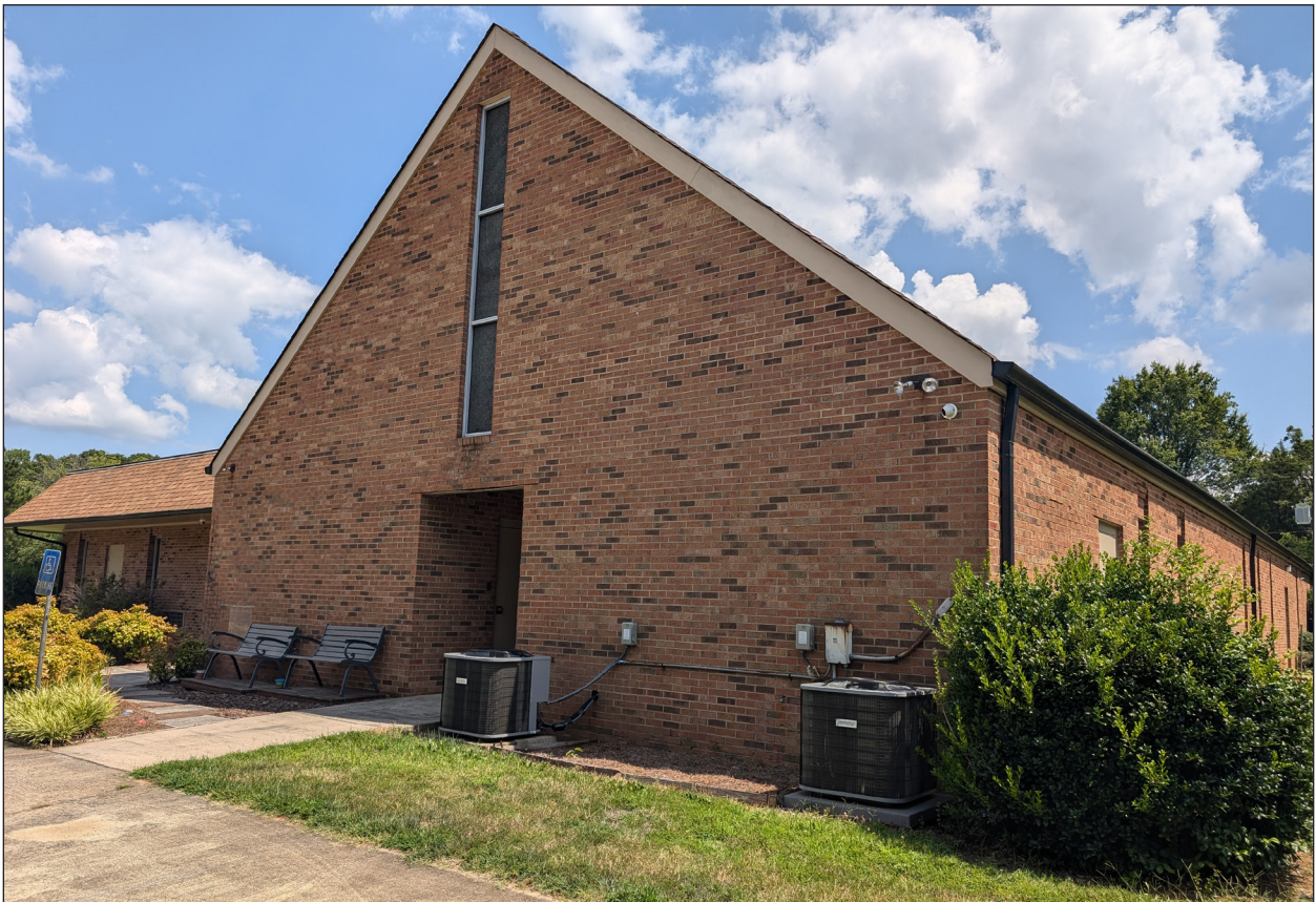
B. Rear and West Elevation, Looking Southeast
