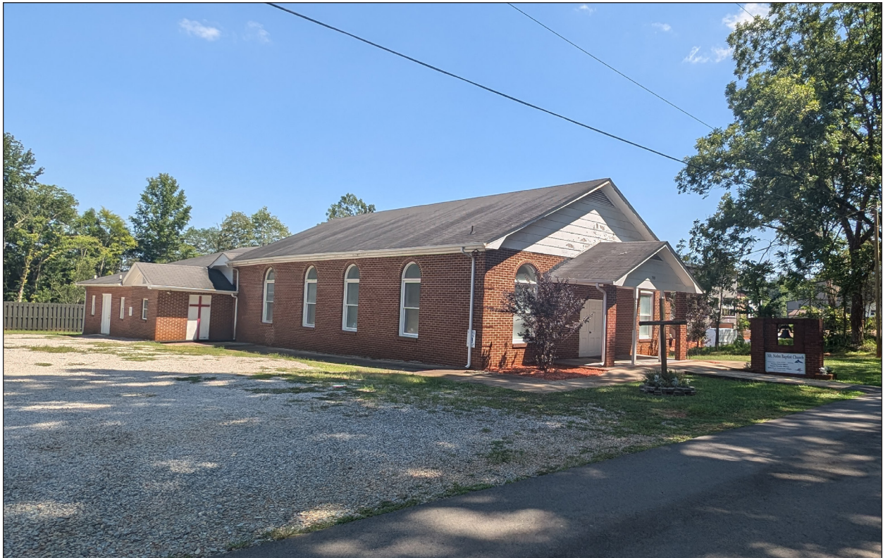
B. Façade and South Elevation, Looking Northeast
