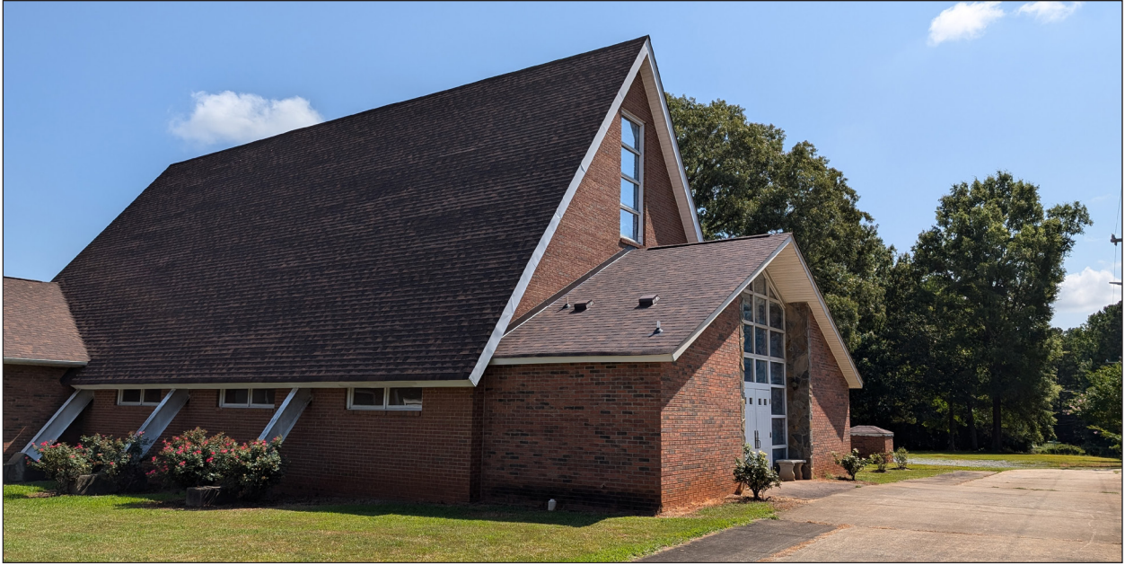
A. Façade and West Elevation, Looking Northeast
