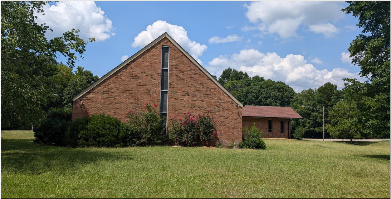
A. Façade, Looking North
