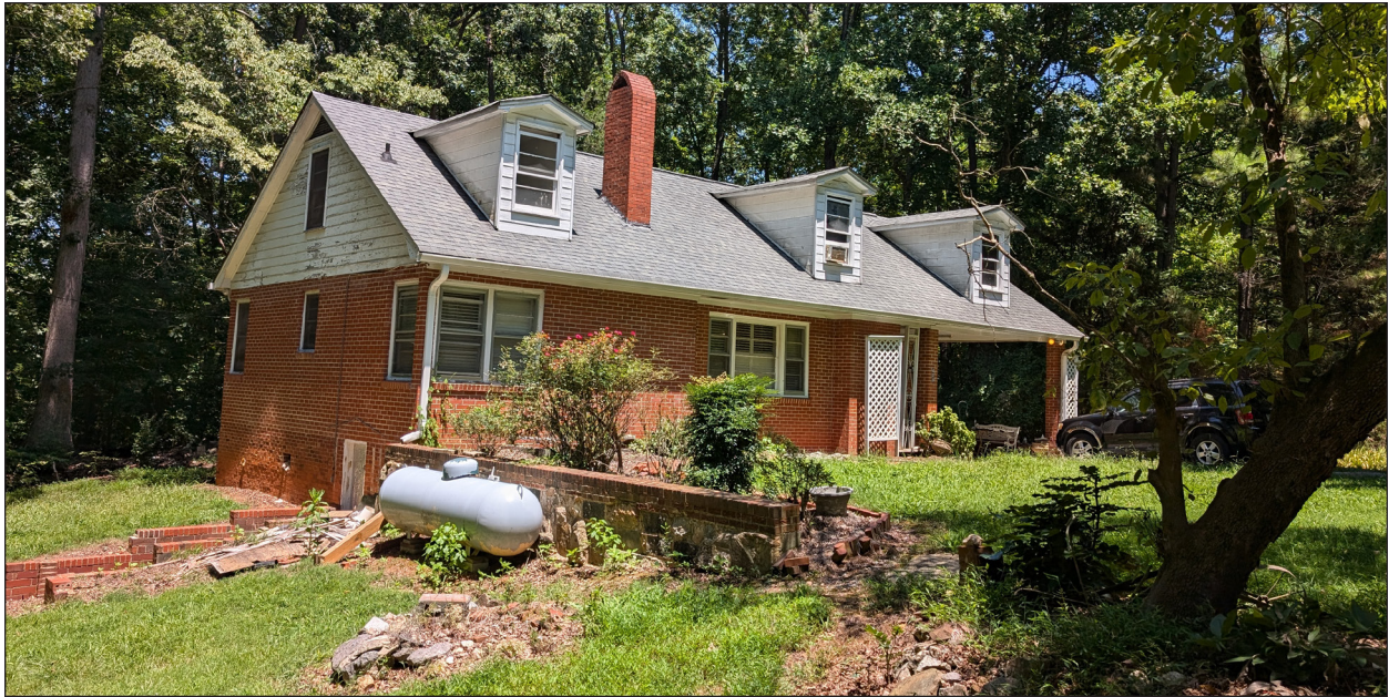
A. Façade and West Elevation, Looking Northeast
