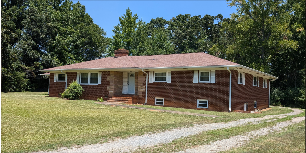
A. Façade and South Elevation, Looking Northeast
