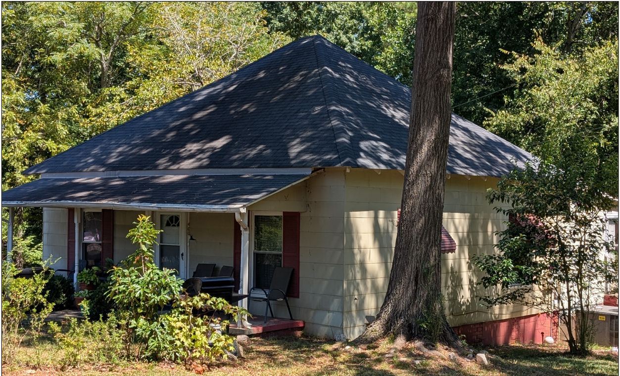
A. Façade and South Elevation, Looking Northeast
