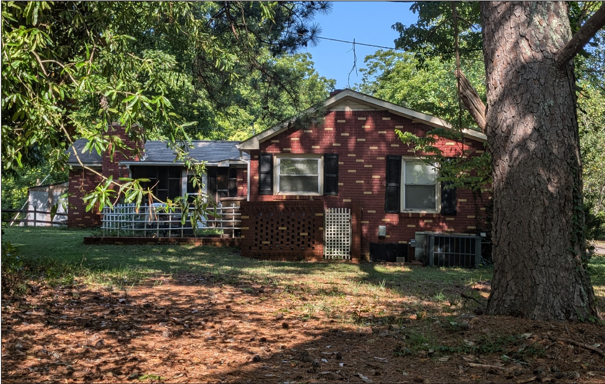
B. East Elevation, Looking West
