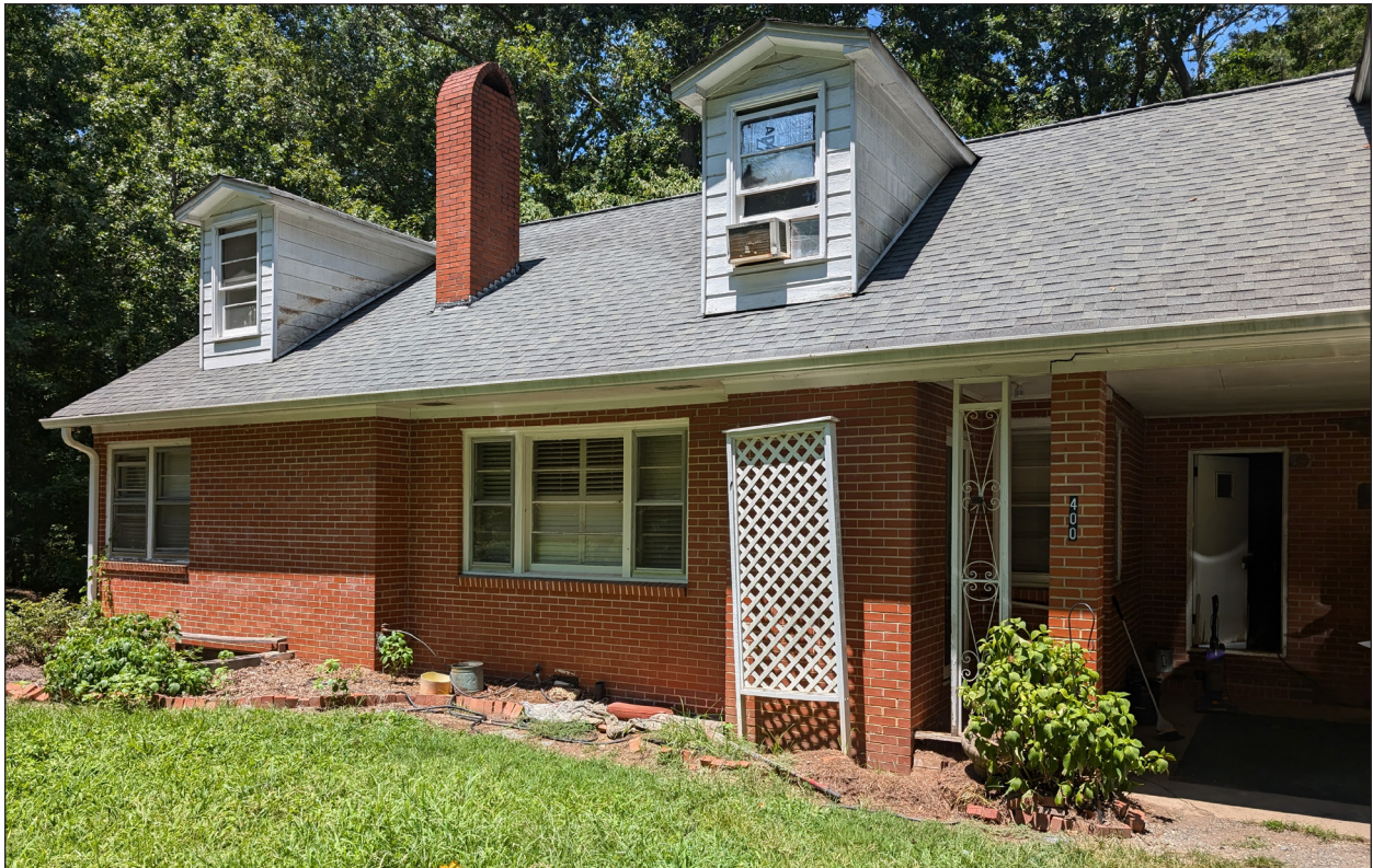
B. Façade, Looking North
