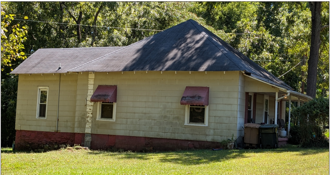
B. North Elevation, Looking South
