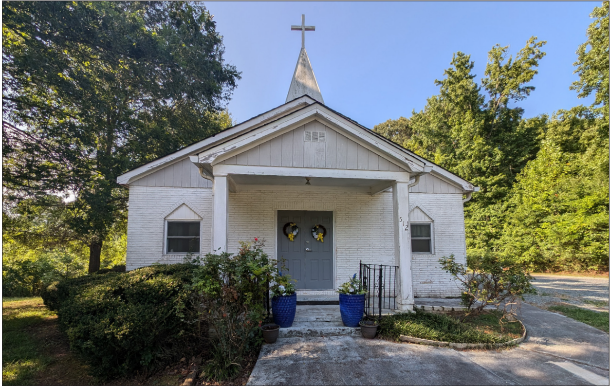
B. Façade, Looking South
