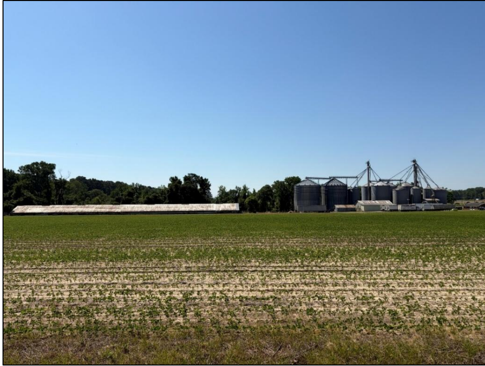
Figure 3.13: Grain elevators in southern Nash County. These structures represent a prominent mid- to late twentieth-century industrial resource type that will be documented during the Phase 2 survey.
