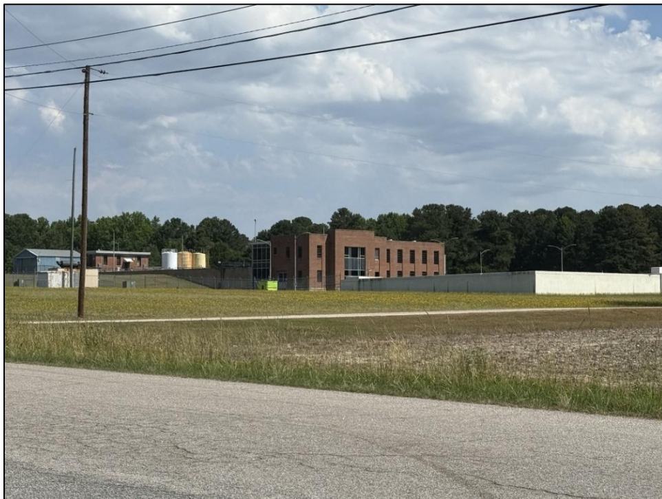
Figure 3.18: The Tar River Reservoir Water Treatment Plant. This facility represents a mid- to late twentieth-century municipal infrastructure resource type that will be documented during the Phase 2 survey.
