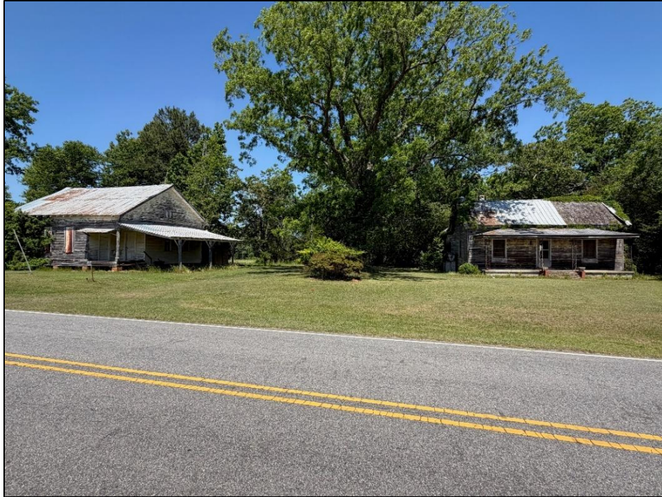
Figure 3.4: Examples of turn of the late nineteenth- or early twentieth-century front-gabled and side-gabled dwellings that will be recorded during the Phase 2 survey.
