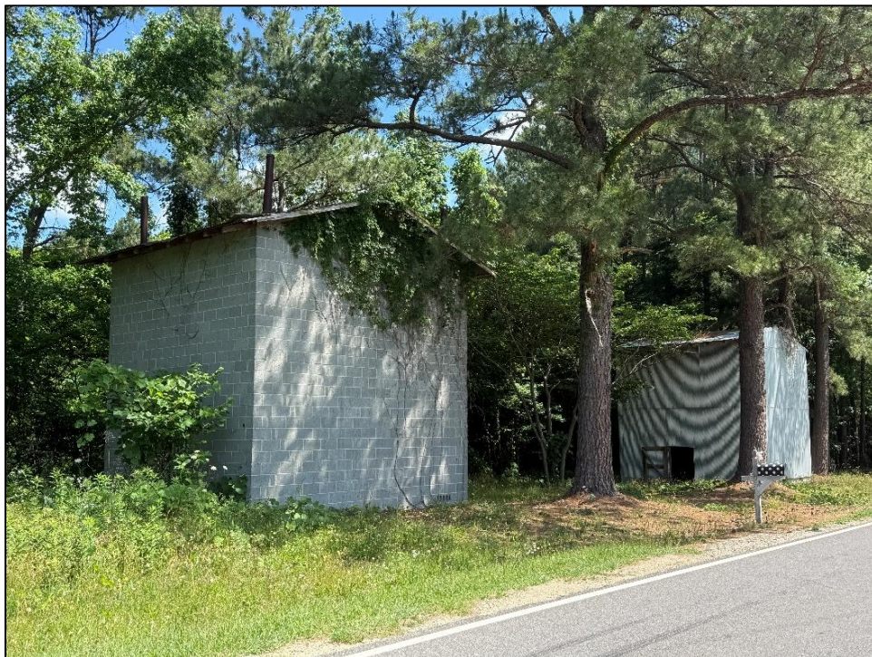
Figure 3.3: Example of isolated tobacco barns lacking an associated farm complex. These standalone agricultural structures will be recorded during the Phase 2 survey.
