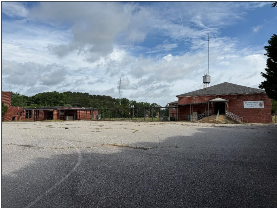
Figure 3.16: Swift Creek Elementary School. This school represents a mid-twentieth-century educational resource type that will be documented during the Phase 2 survey.
