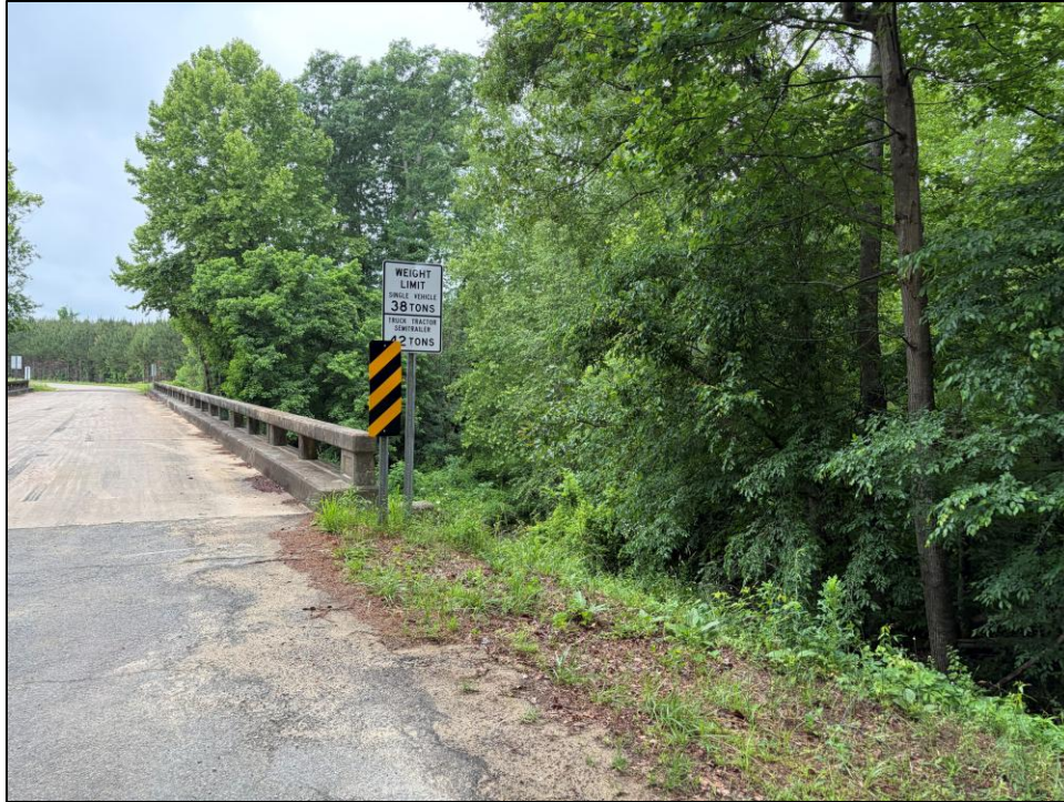
Figure 3.14: Example of an NCDOT bridge constructed in the 1960s. This structure represents a mid-twentieth-century transportation resource that will be documented during the Phase 2 survey.
