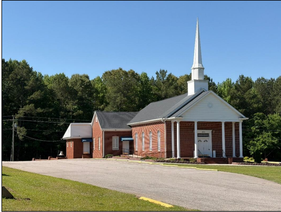
Figure 3.15: Lee's Chapel Baptist Church outside Middlesex. This property represents notable rural church architecture that will be documented during the Phase 2 survey.
