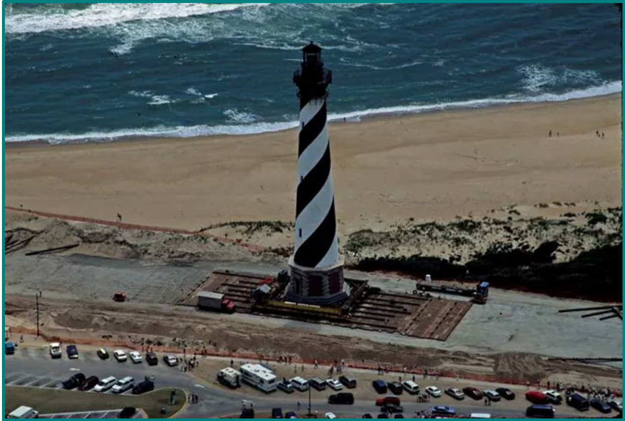
Figure 4. The Cape Hatteras Lighthouse being relocated in response to encroaching Atlantic Ocean waters. Image courtesy of the National Park Service.
