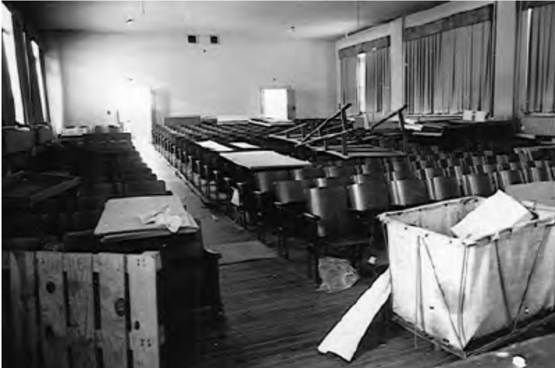
Figure 63. Ca. 1985 interior views of 1927 auditorium addition (Source: NCHPO Murphey School survey file).
