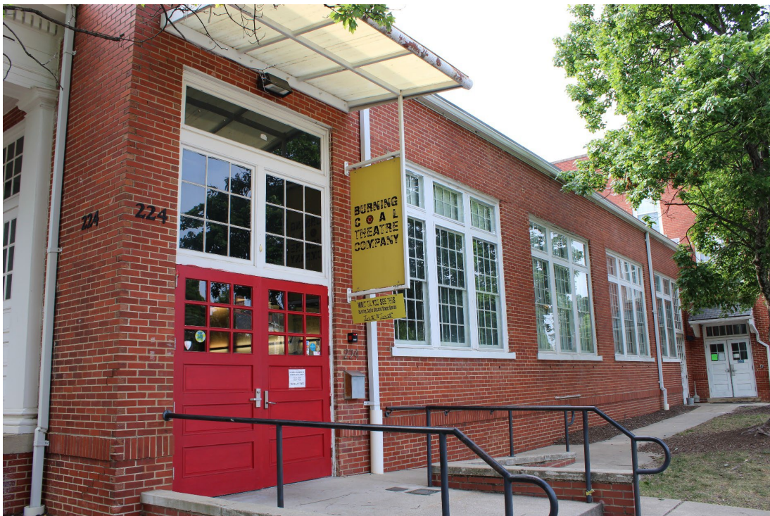
Figure 41. View of 1927 auditorium addition, northern corner of west elevation, looking southeast.
