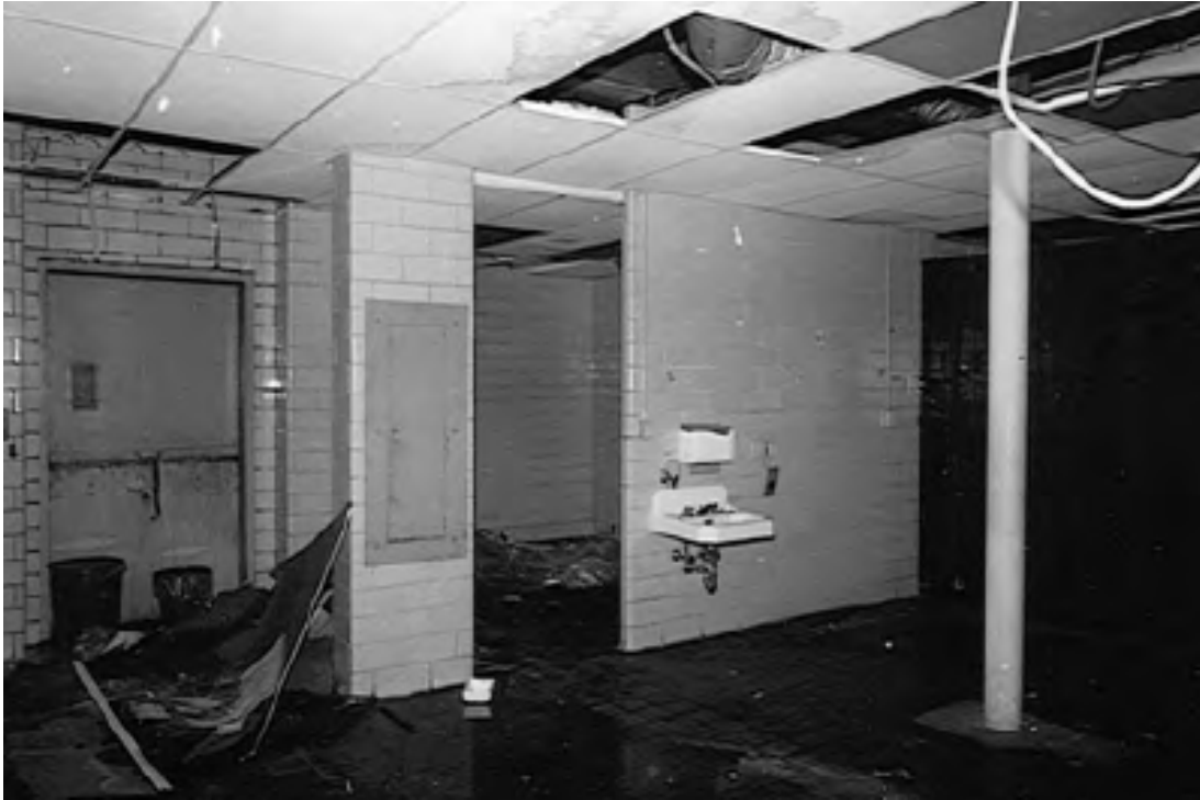
Figure 59. Ca. 1985 interior view of Murphey School basement, location unknown (Source: NCHPO Murphey School survey file).
