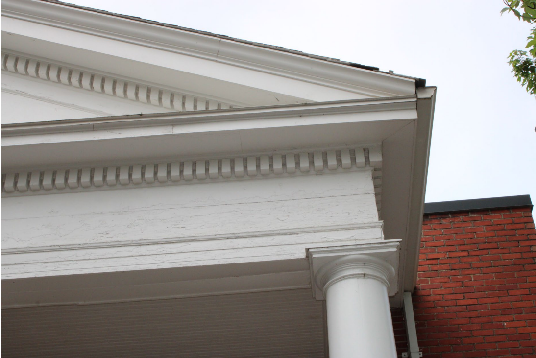
Figure 36. Detail view of 1927 auditorium addition cornice, looking south.
