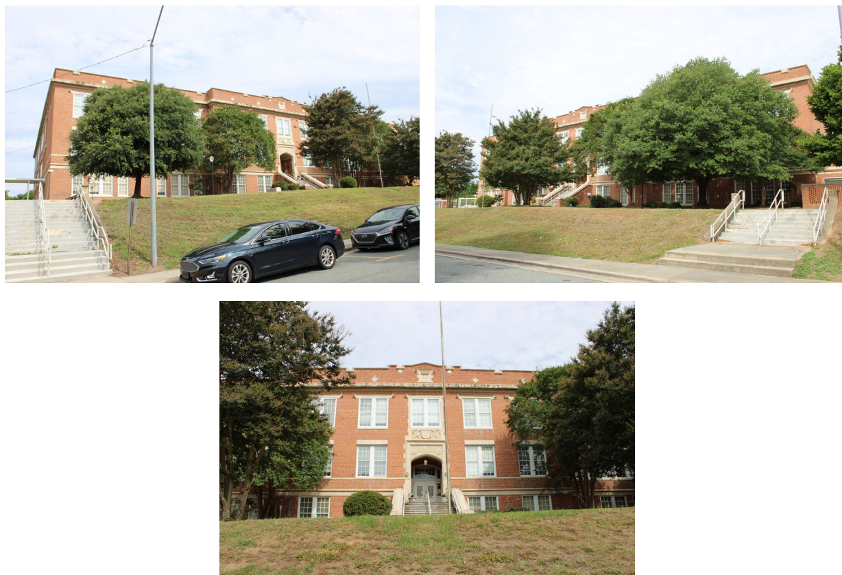
Figure 77. Washington Graded and High School (WA3360) at 1000 Fayetteville Street in Raleigh. Built ca. 1924 and NRHP listed in 2004.
