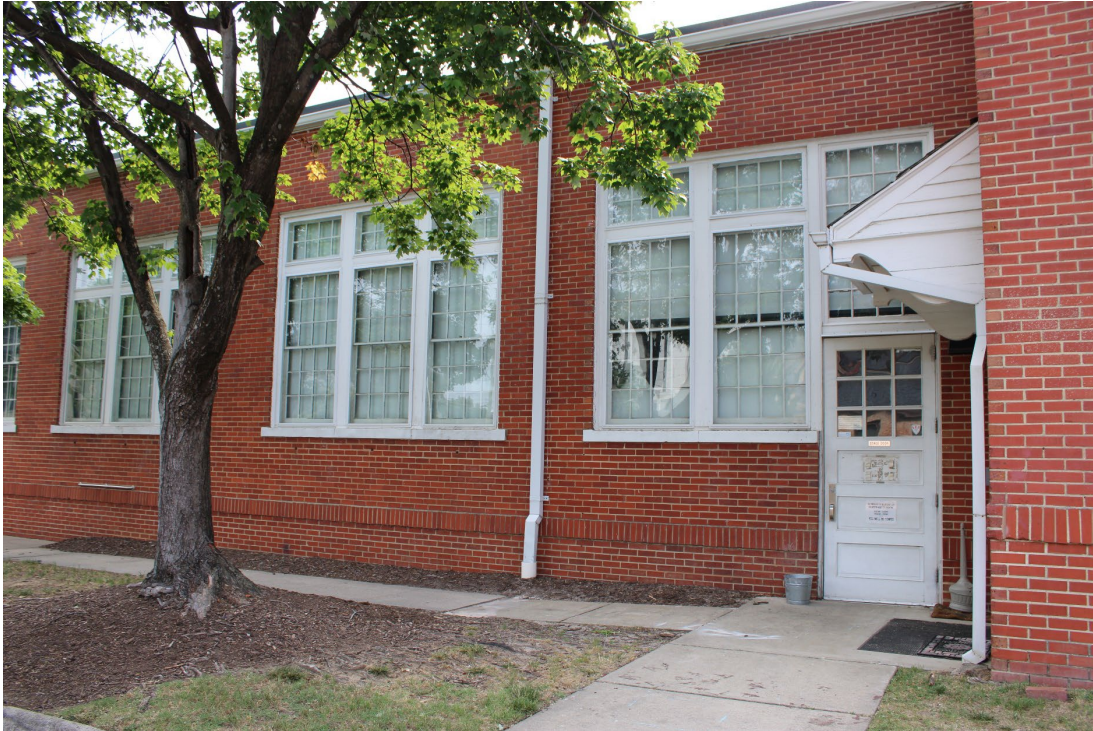
Figure 42. View of 1927 auditorium addition, southern corner of west elevation, looking east.
