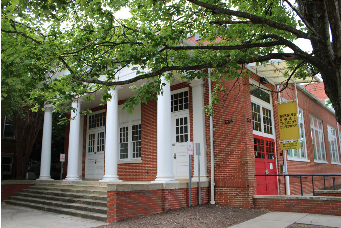
Figure 38. Oblique view of 1927 auditorium addition, north and west elevations, looking southeast.
