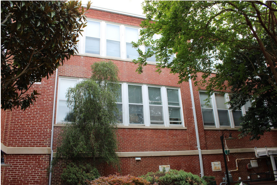
Figure 18. View of 1916-1917 Murphey School building west elevation, looking east.
