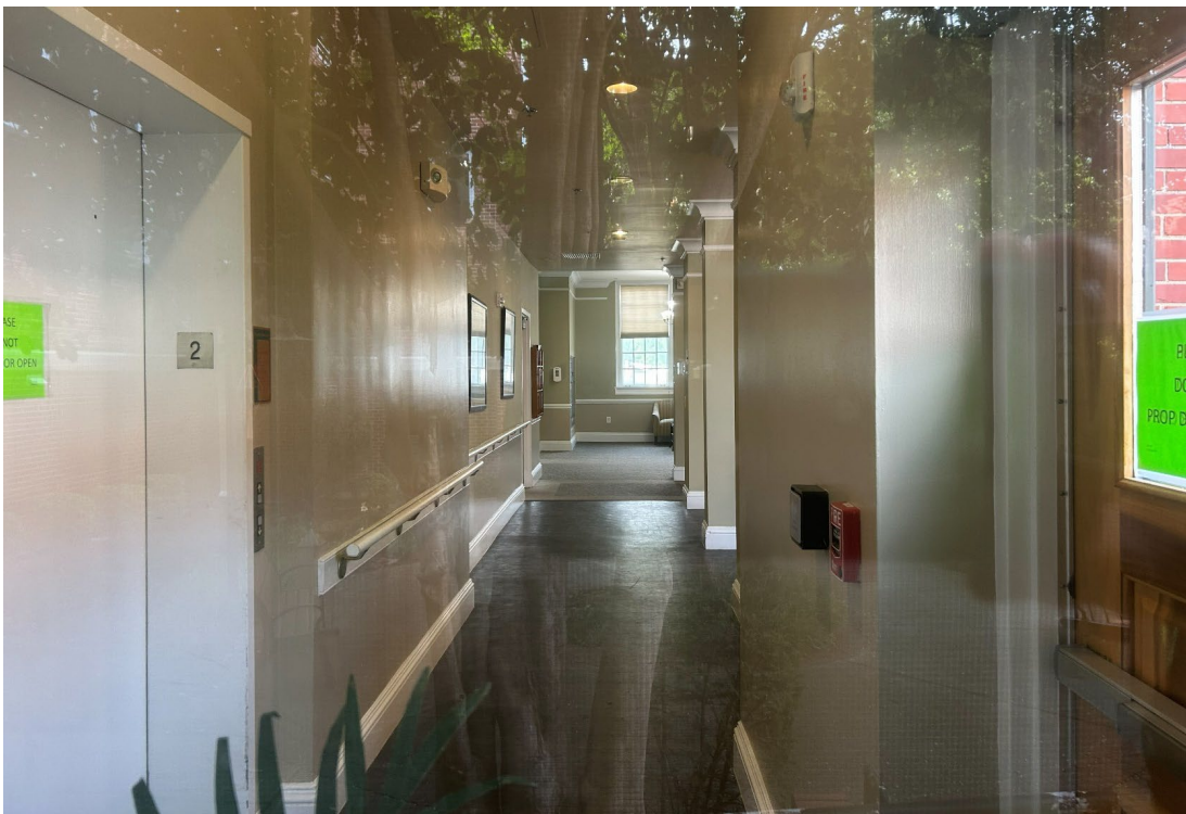
Figure 48. Ca. 2026 view through window north juncture of original building and the 1927 classroom addition. View is looking south into 1927 addition.
