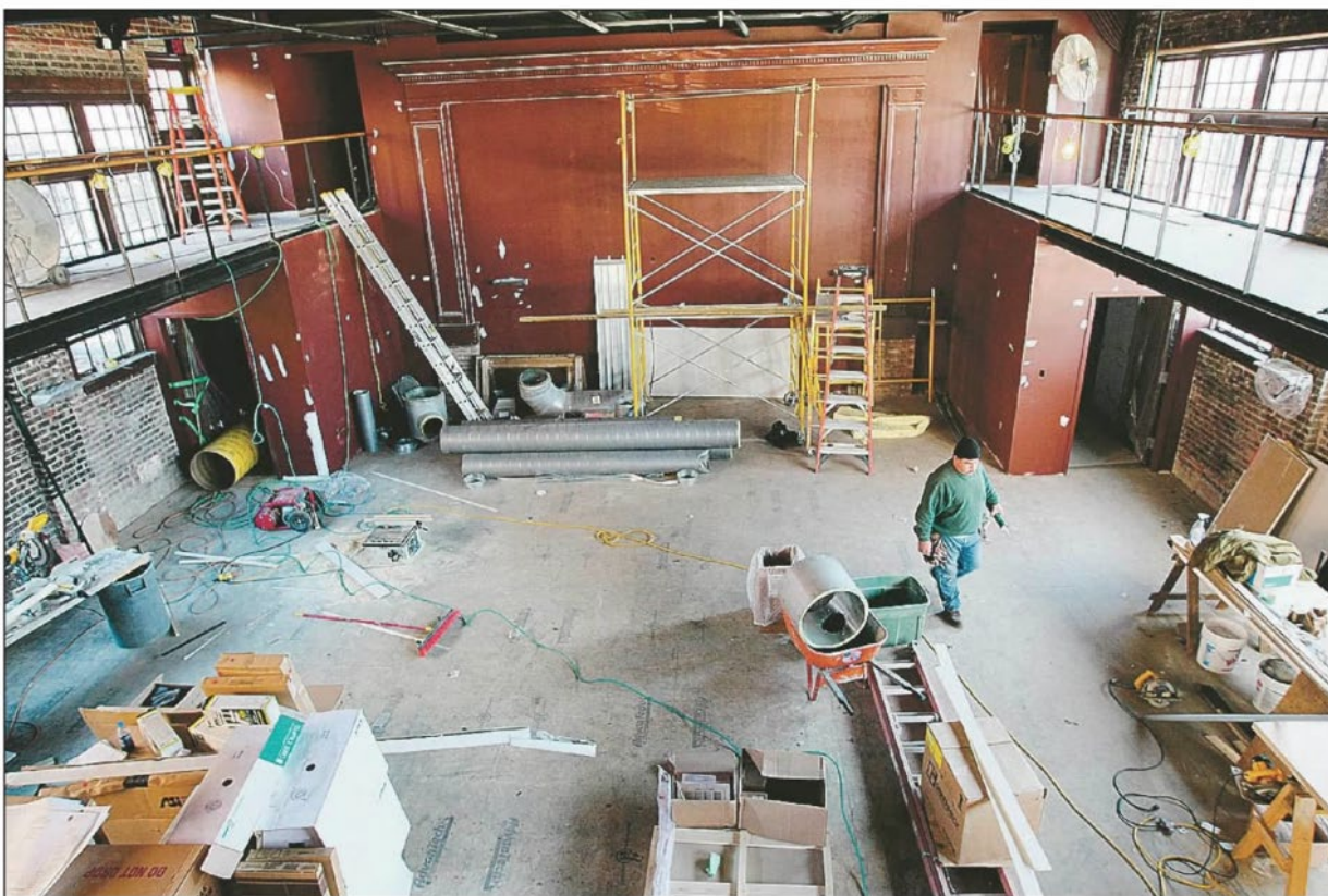
Figure 74. Photograph of the Murphey School Auditorium under construction published in the News and Observer on January 13, 2008.
