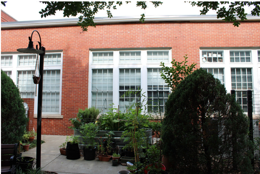
Figure 45. View of 1927 auditorium addition, east elevation, looking west from courtyard.
