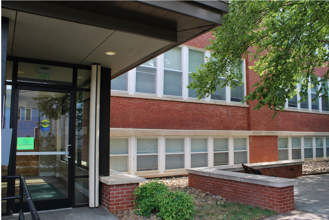
Figure 30. View of 1916-1917 Murphey School building, south elevation, looking northeast. Twentieth century door at juncture of building and 1927 classroom addition visible at left.
