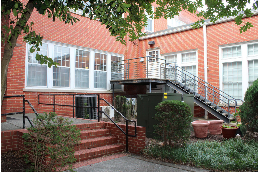
Figure 44. View of juncture of 1927 auditorium addition with 1927 classroom addition, looking southwest at east elevation of auditorium addition and north elevation of classroom addition.
