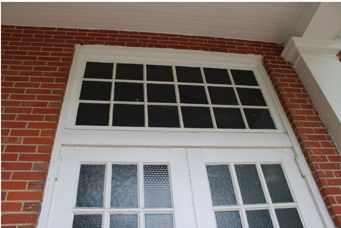
Figure 37. Detail view of 1927 auditorium addition front doors and transom, looking south.
