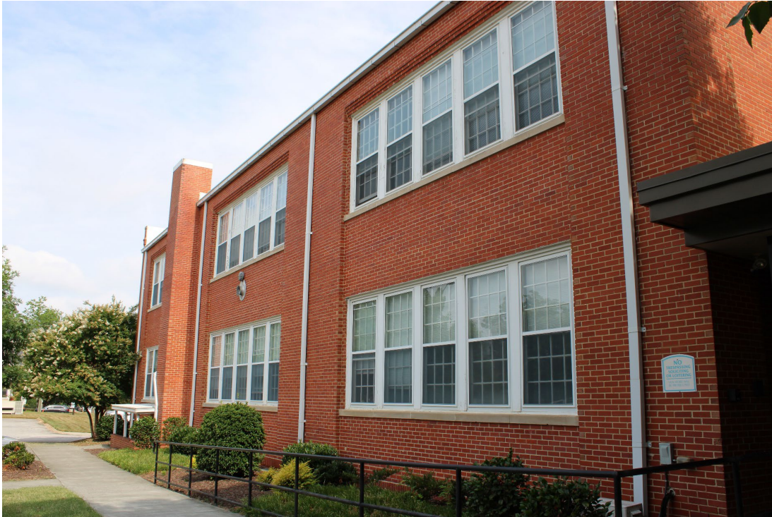
Figure 28. View of 1927 classroom addition, south elevation, looking northwest.
