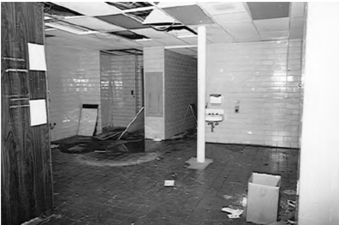
Figure 58. Ca. 1985 interior view of Murphey School basement, location unknown (Source: NCHPO Murphey School survey file).
