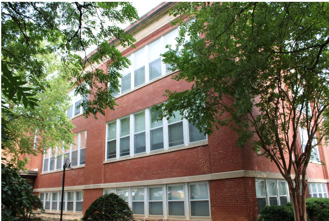
Figure 31. Oblique view of 1916-1917 Murphey School building, south elevation and east facade, looking northwest.
