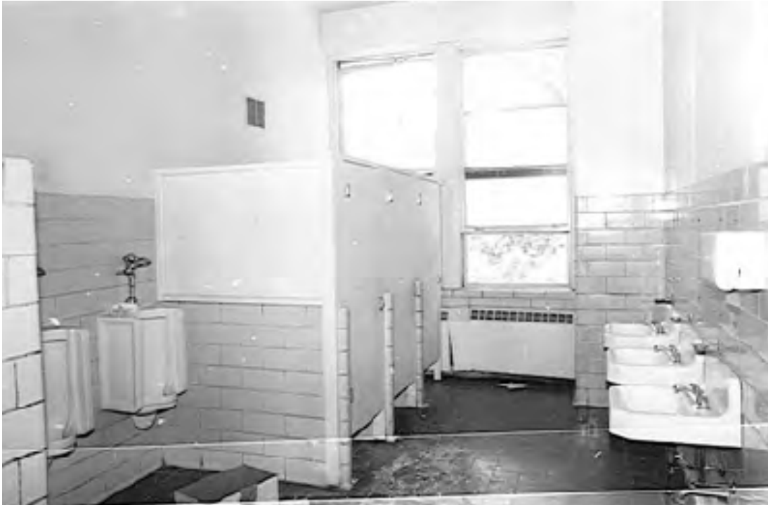
Figure 53. Ca. 1985 interior view of Murphey School bathroom, location unknown (Source: NCHPO Murphey School survey file).
