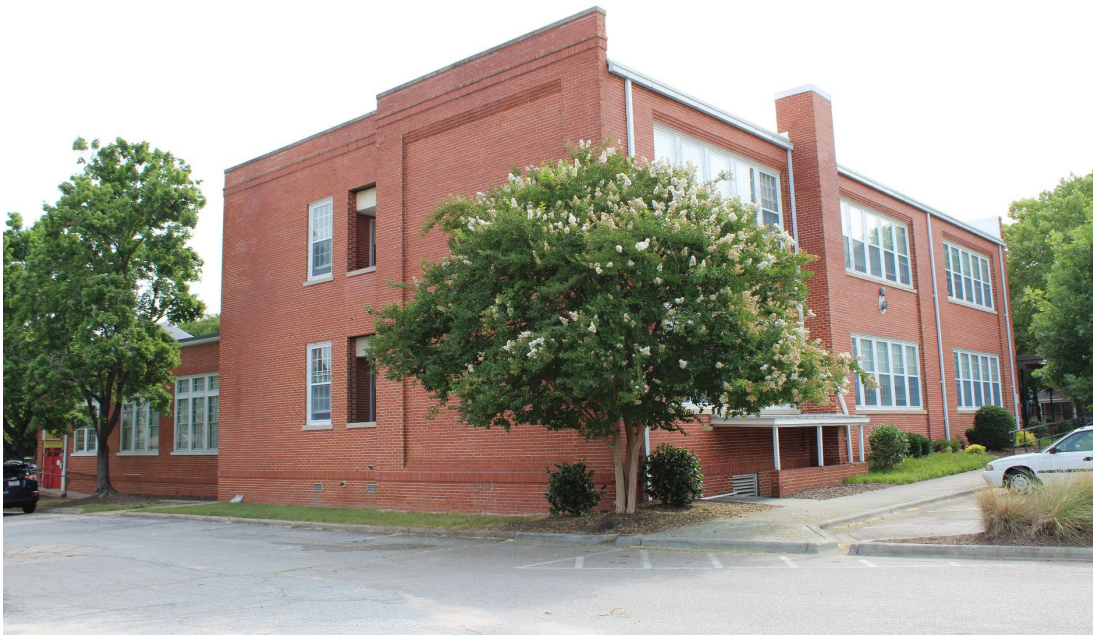
Figure 25. Oblique view of 1927 classroom addition, south and east elevations, looking northwest. Southern elevation of 1927 auditorium is seen at left.
