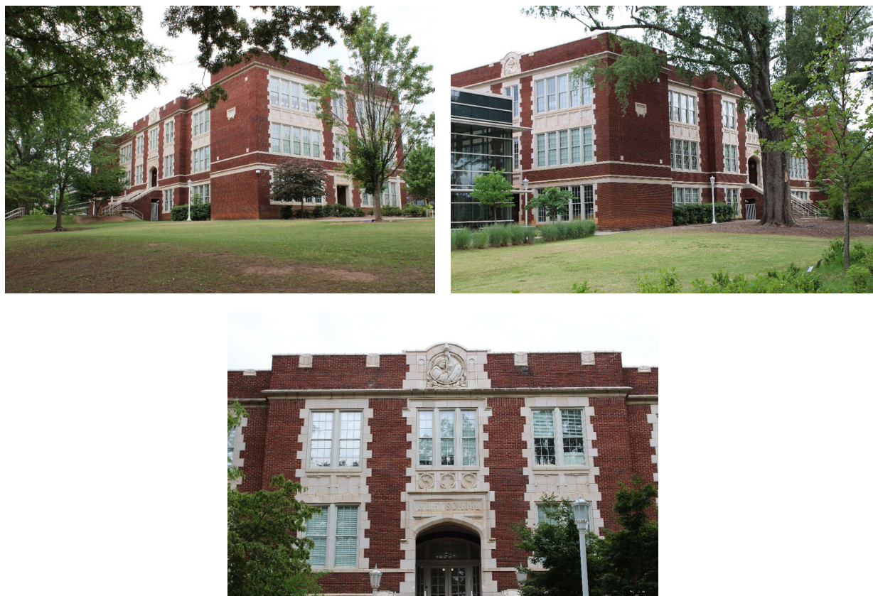
Figure 78. The Wiley School (WA3945) at 301 Saint Mary's Street in Raleigh. Built ca. 1926.
