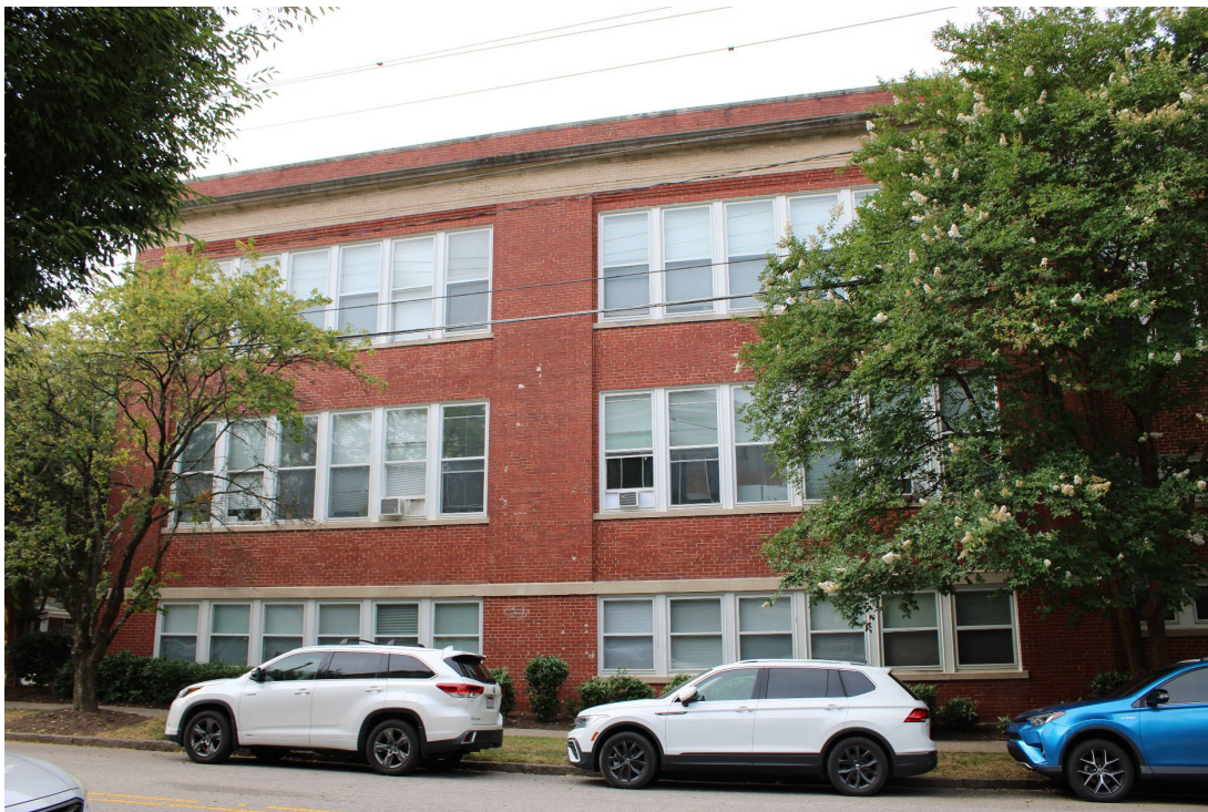
Figure 15. View of 1916-1917 Murphey School building north elevation, looking south.
