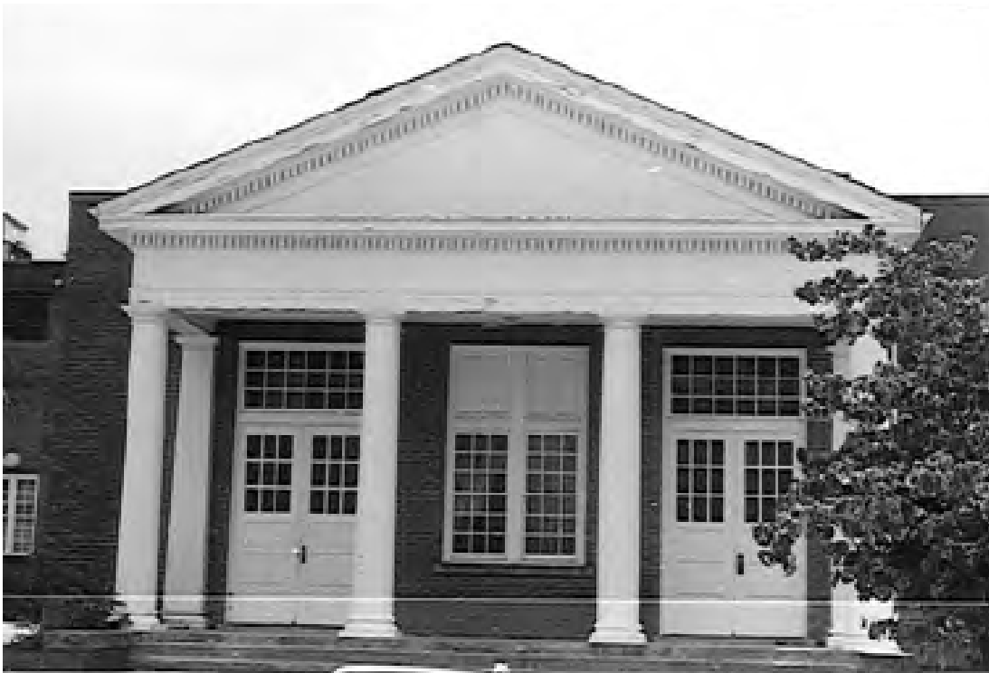
Figure 33. Ca. 1985 view of 1927 auditorium addition north facade, looking south (Source: NCHPO Murphey School survey file).
