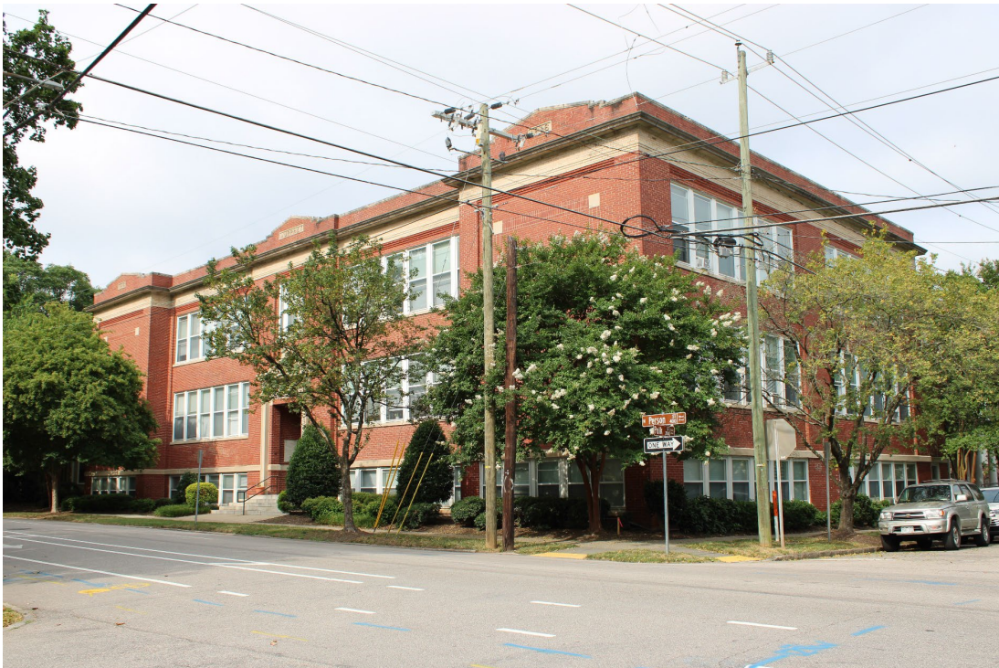
Figure 5. Contextual view of Murphey School from intersection of N Person Street and Polk Street, looking southwest.
