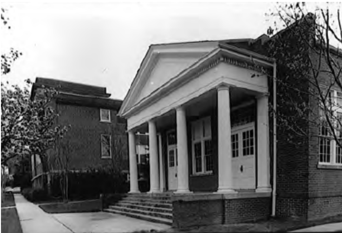
Figure 39. Oblique view of 1927 auditorium addition, north and west elevations, looking southeast with 1916-1917 school building in background at left (Source: NCHPO Murphey School survey file).
