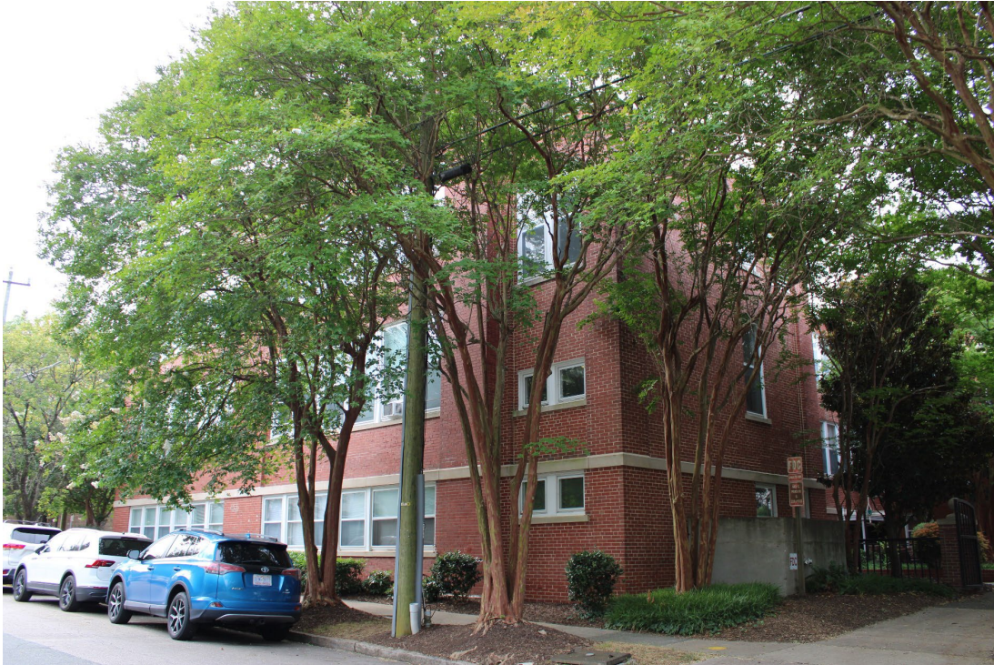
Figure 16. Oblique view of north and west elevations of 1916-1917 Murphey School building, looking southeast.
