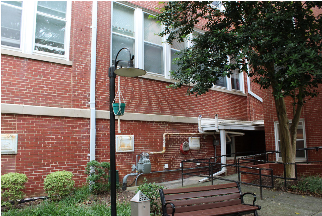
Figure 20. View of 1916-1917 Murphey School building west elevation at junction with classroom addition, looking southeast from interior courtyard.
