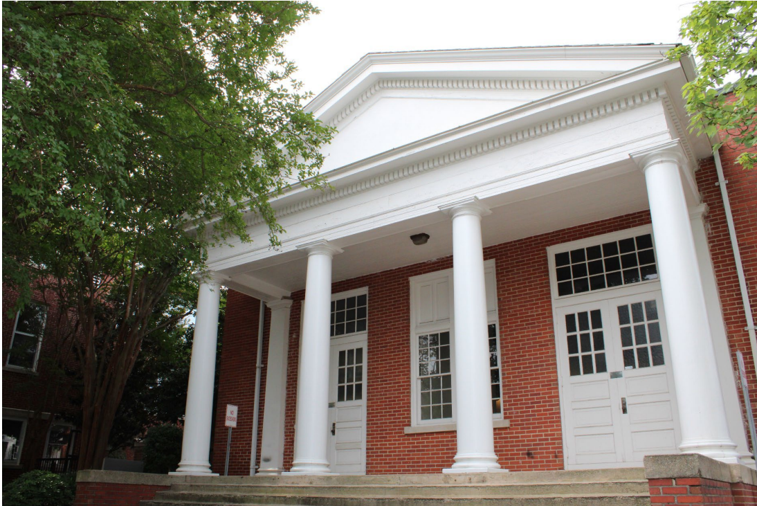
Figure 34. View of 1927 auditorium addition, north facade, looking southeast.
