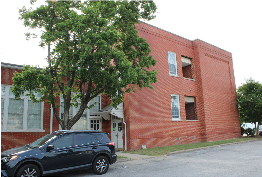
Figure 24. Oblique view of 1927 classroom addition, south and west elevations, looking northeast. Southern elevation of 1927 auditorium is seen at left.
