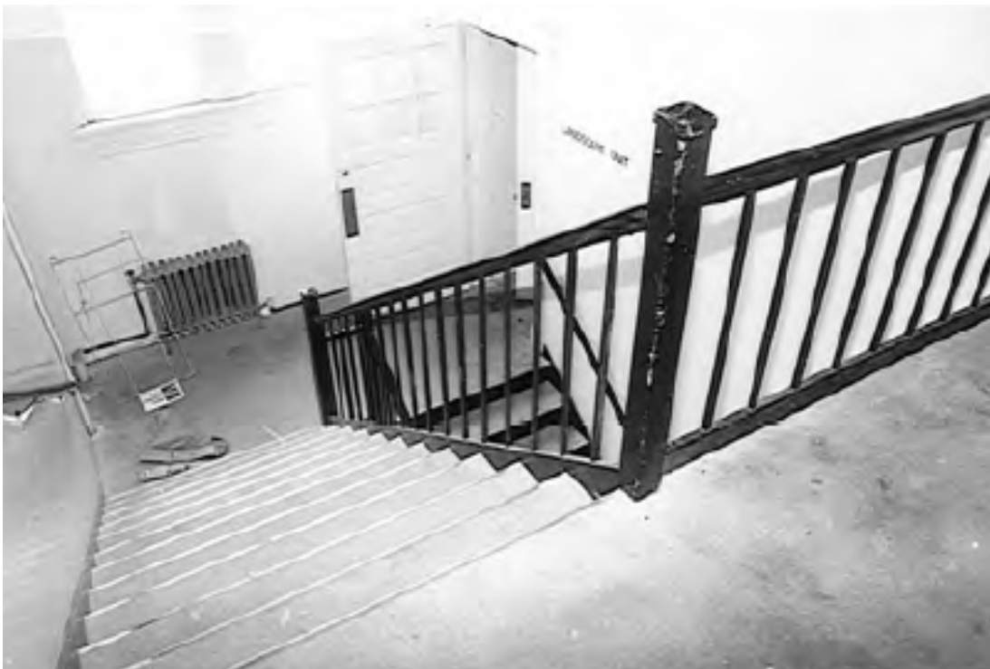
Figure 52. Ca. 1985 interior view of Murphey School stairwell, location unknown (Source: NCHPO Murphey School survey file).
