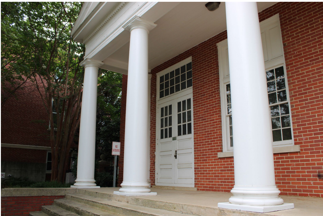
Figure 35. View of 1927 auditorium addition, north facade, looking southeast.
