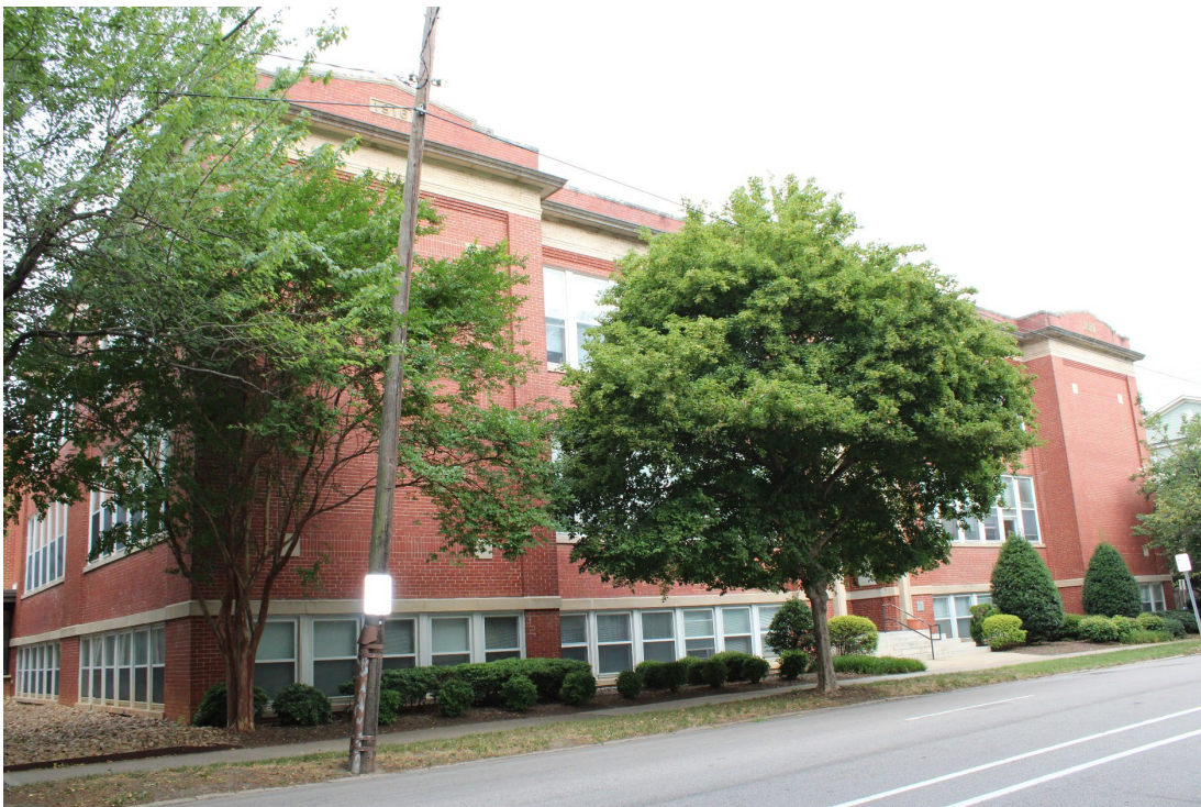
Figure 7. Oblique view of 1916-1917 Murphey School building, east facade and south elevation, looking northwest.
