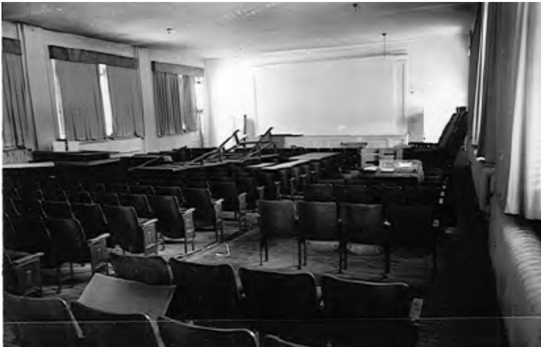
Figure 64. Ca. 1985 interior views of 1927 auditorium addition (Source: NCHPO Murphey School survey file).
