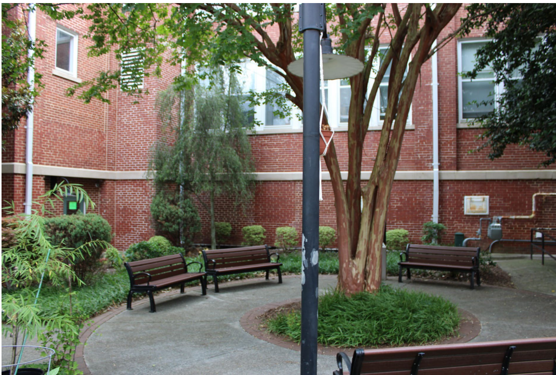
Figure 19. View of 1916-1917 Murphey School building west elevation, looking east from interior courtyard.
