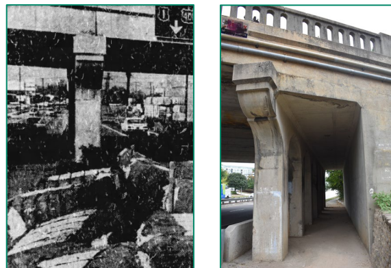
Figure 62. Left, detail of one of the bridge's piers from 1961 News and Observer article; right, detail view of the bridge's easternmost pier and walkway on south elevation, looking north.
