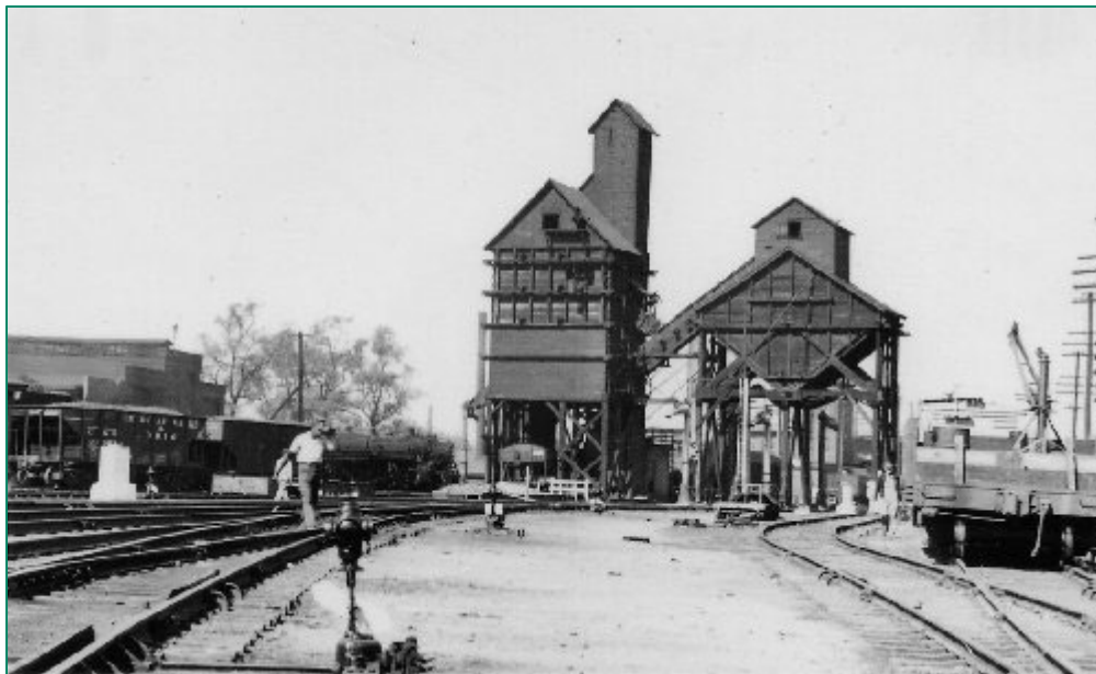
Figure 39. Undated view looking north at no-longer-extant SAL coal chutes located south of Peace Street and east of SAL roundhouse, north end of which is visible at left (PWRC n.d.D).
