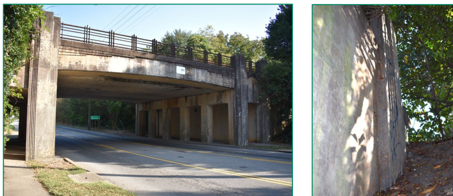
Figure 80. Left, view of bridge's west elevation from the sidewalk, looking southeast; right, detail view of bridge's abutment with Art Deco-style stepped ornamentation.
