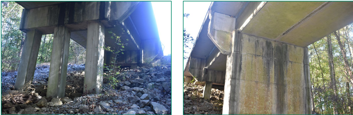
Figure 95. Left, view of bridge's substructure and underside of superstructure, looking southwest; right, view of bridge's substructure and underside of superstructure, looking northwest.
