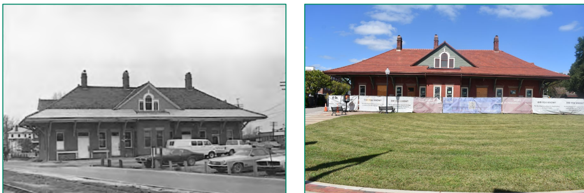
Figure 103. Left, 1980s survey photograph of north-facing façade (NCHPO 2025); right, view of façade, looking south.
