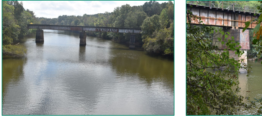
Figure 87. Left, view of bridge's north elevation from roadway bridge, looking south; right, detail view of bridge's deck and plate deck girder, and metal-capped stone pier.
