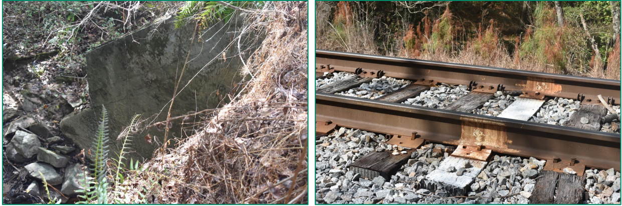
Figure 97. Little Buffalo Creek Culvert 1, west elevation, facing north, at left; white-painted tie over creek and culvert, at right.
