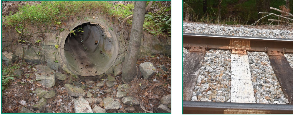
Figure 84. Shaddox Creek Culvert, northwest elevation, looking southeast, at left; looking down at white-painted tie over culvert location indicating its presence, at right.
