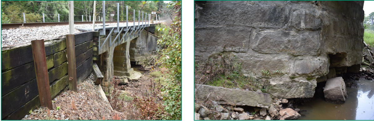
Figure 85. Left, SAL Bridge over Shaddox Creek, northwest elevation, looking southwest; right, SAL Bridge over Shaddox Creek, ca.1890 stone pier, looking northwest.
