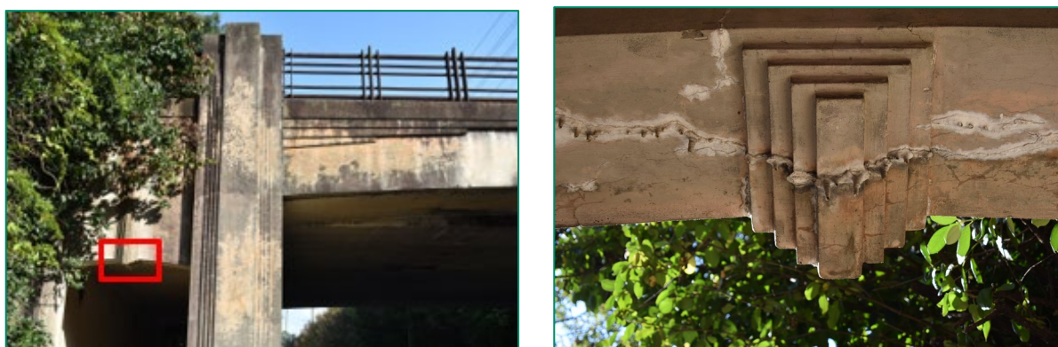
Figure 81. Left, detail view of stepped details on walkway entrance, end of column, and railing, looking southeast; right, detail view of underside of stepped ornamentation on walkway entrance (outlined in red on photo at left).
