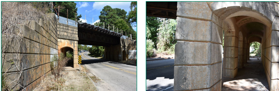
Figure 67. Left, view of bridge's south elevation, looking northwest; right, detail view of bridge's bent and eastern colonnade-like walkway.
