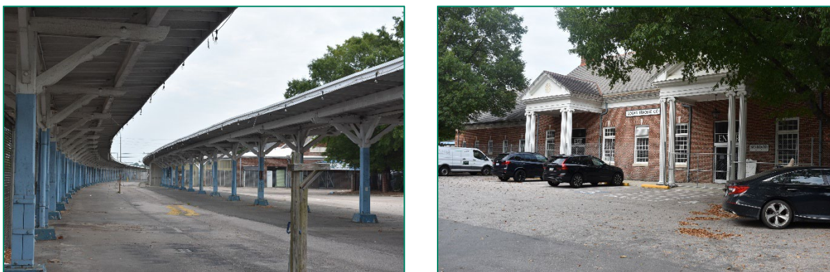
Figure 55. Left, view of Seaboard Railway Station sheds and south elevation of station, looking north; right, view of east façade of station, looking southwest.
