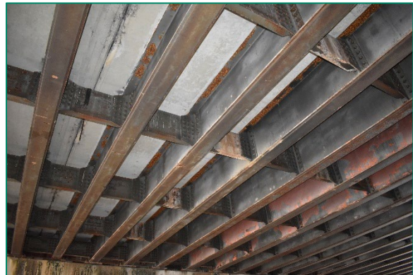
Figure 57. Left, view of west elevation of bridge, looking southeast; right, detail view of steel I-beams and diaphragms supporting the bridge's deck.
