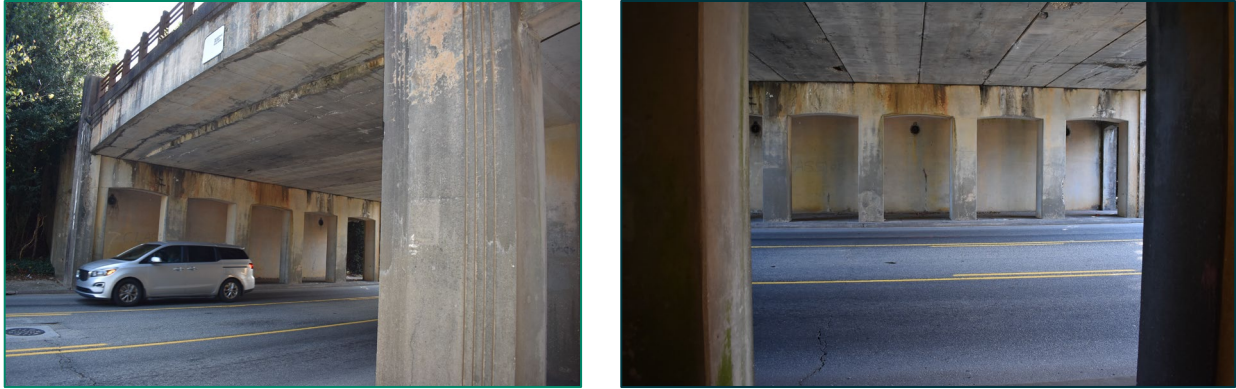
Figure 82. Left, view of walkway, bent with portal piers, and underside of deck, looking southwest; right, view of portal piers, walkway, and lights lining walkway.
