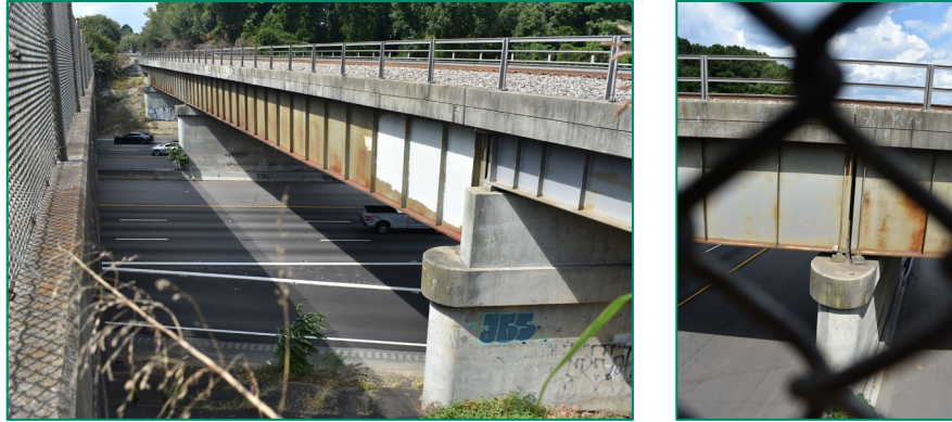
Figure 70. Left, view of bridge's south elevation, looking northwest; right, detail view of bridge deck, steel stringers, and concrete piers from pedestrian walkway, looking west.
