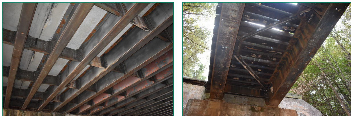
Figure 27. At left, multiple deck beams and bolted diaphragms at Peace Street bridge; at right, pair of steel girders supporting ties of Olives (or Wombles) Creek bridge.
