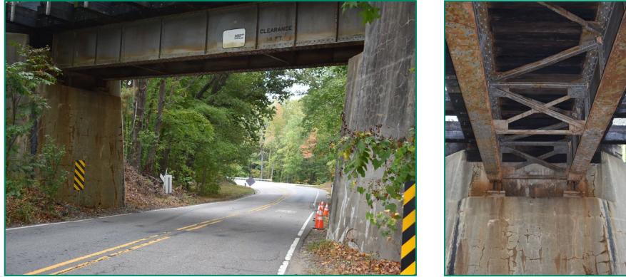
Figure 74. Left, SAL Bridge over W. Chatham Street, west elevation, looking east; right, SAL Bridge over W. Chatham Street, detail of underside with steel girders, riveted cross-bracing, wooden deck, and abutment.
