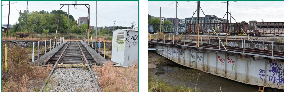
Figure 58. Left, view of turntable and motor house, looking southwest; right, view of turntable pit and track, looking northeast.
