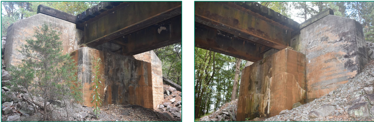
Figure 93. Left, view of bridge's concrete abutments, wooden deck, and steel I-beams on east elevation, looking southwest; right, view of bridge's concrete abutments, wooden deck, and steel I-beams on east elevation, looking northwest.
