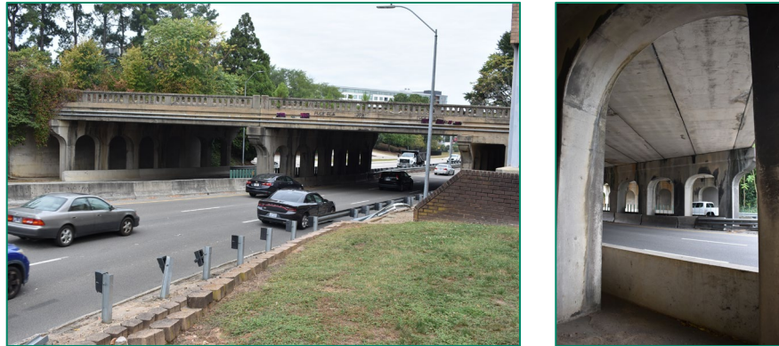
Figure 60. Left, view of bridge's south elevation, looking northwest; right, detail view of bridge's bent and underside of superstructure from eastern walkway, looking west.
