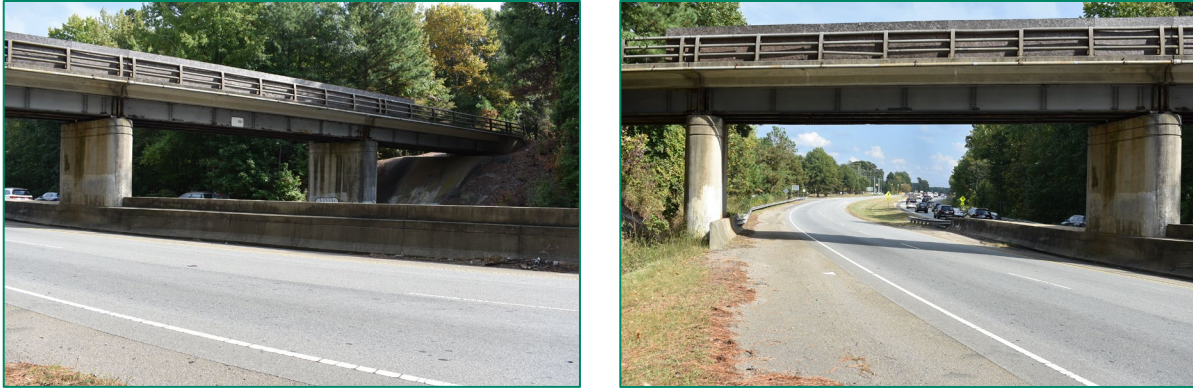
Figure 75. Left, SAL Bridge over US 64, west elevation and abutment, looking east; right, SAL Bridge over US 64, west elevation, looking east toward westbound lanes.
