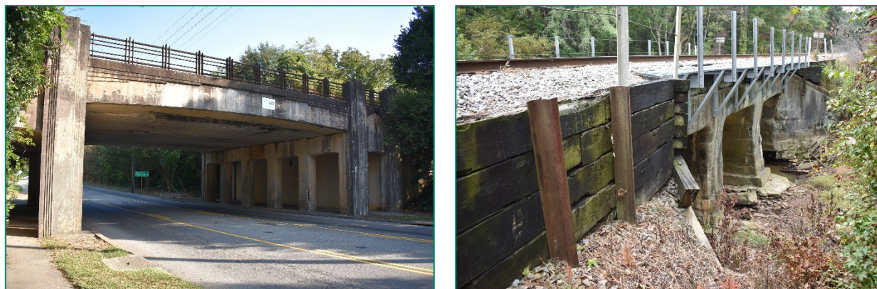
Figure 28. At left, 1939 concrete bridge over Williams Street/NC 55 in Apex, looking south; at right, concrete-encased deck girder bridge over Shaddox Creek in Chatham County.
