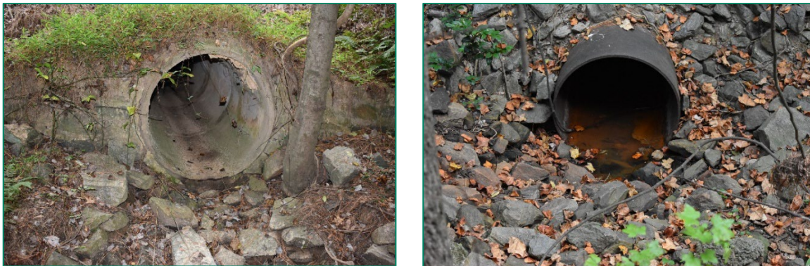
Figure 32. Shaddox Creek Culvert (CH0925) with concrete pipe and stone enframement, at left; steel bore-and-jack culvert located north of Apex and southeast of North Salem Street, at right.
