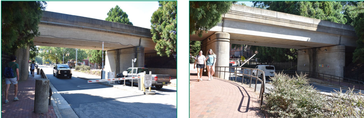
Figure 64. Left, view of bridge's north elevation, looking southwest; right, view of bridge's south elevation, looking northeast.
