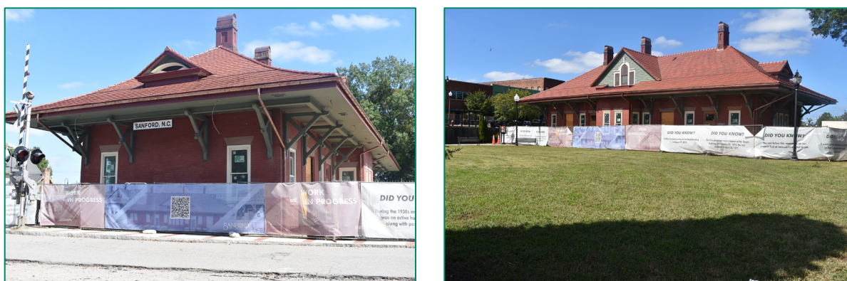
Figure 104. Left, view of west (side) and south (rear) elevations, looking northeast; right, view of south (rear) and east (side) elevations, looking northwest.
