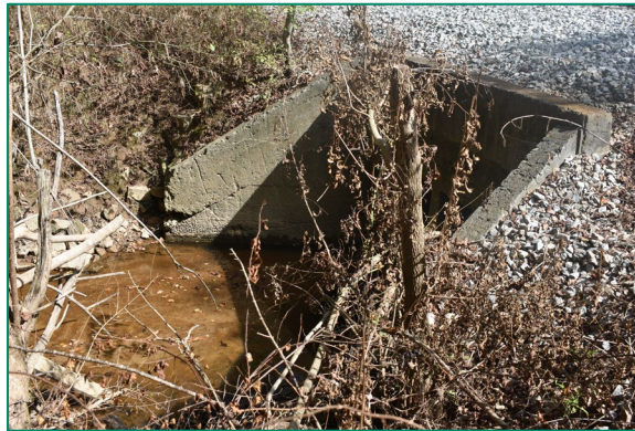
Figure 99. Little Buffalo Creek Culvert 2, looking northeast at west elevation.
