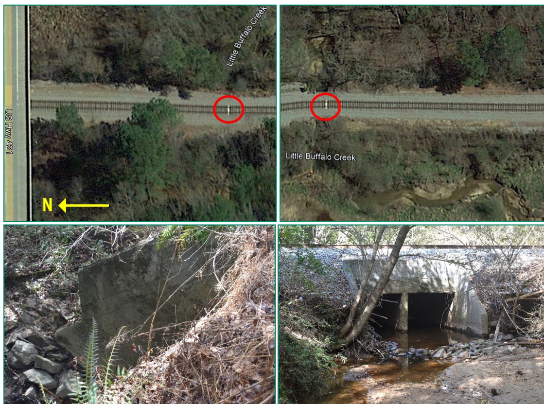
Figure 31. Screen captures of 2018 Google Earth views of white-painted ties at Little Buffalo Creek Culvert I, at top left, and Culvert II approximately 1,800' to the south, at top right; Culvert I, at bottom left, looking north, and Culvert II, at bottom right, looking northwest.
