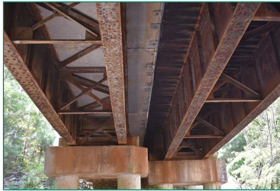
Figure 73. Detail view of bridge's girders and decks (left is concrete, right is wood).
