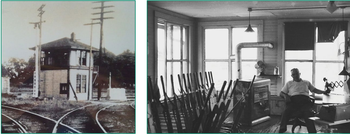
Figure 38. At left, undated photograph of lost Apex switch tower shared by the SAL and Durham & Southern Railway (PWRC n.d.A); at right, interior of no-longer-extant SAL switch tower at wye near Boylan Avenue in Raleigh, 1960s (NCRR n.d.).
