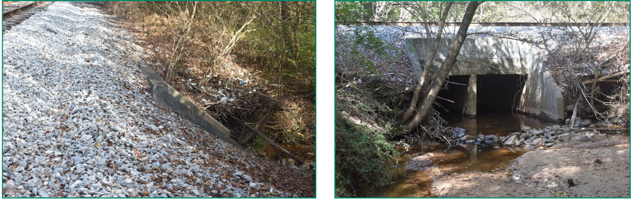
Figure 98. Left, Little Buffalo Creek Culvert 2 and CSX rail line, facing north with east elevation of culvert at right; right, east elevation of culvert, facing west.
