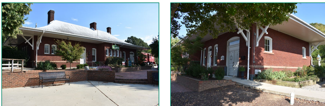
Figure 78. Left, Apex Union Depot, west façade, looking south; right, Apex Union Depot, west façade and south elevation, looking northeast.
