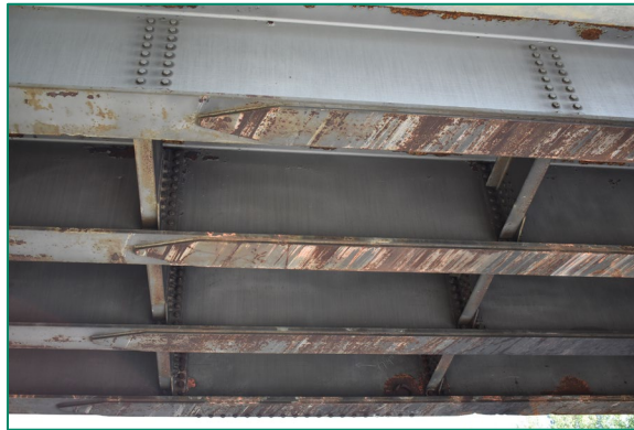
Figure 76. SAL Bridge over US 64, detail of underside with tapered cover plates and bolted steel stringers.
