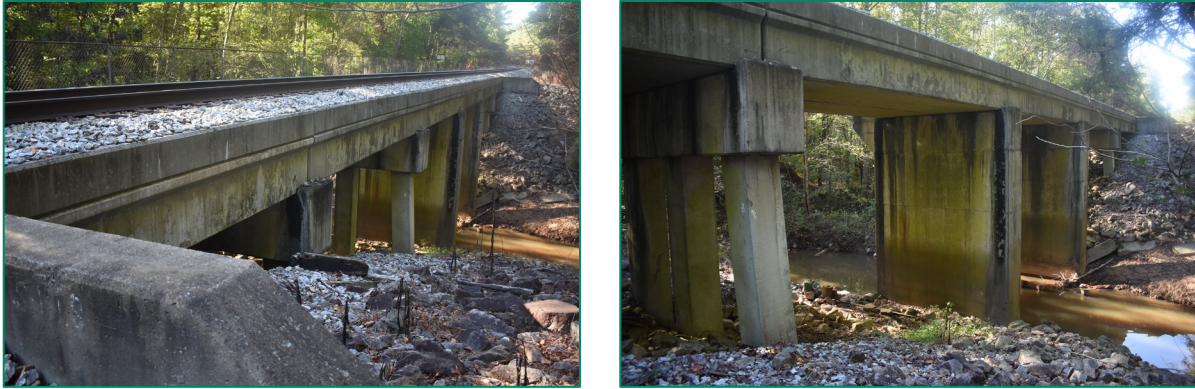
Figure 94. Left, view of bridge's track and concrete deck, looking northwest; right, view of bridge's bents, looking northwest.
