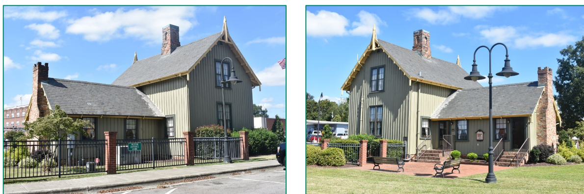
Figure 102. Left, view of south (rear) and east (side) elevations, looking northwest; right, view of west (side) and south (rear) elevations, looking northeast.
