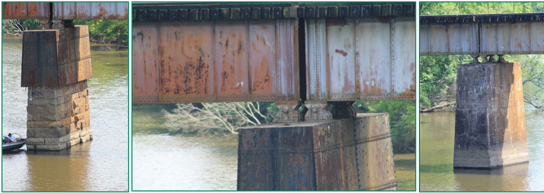
Figure 88. Left, 2015 photograph of bridge's center stone pier with riveted metal jacket; center, 2015 photograph of girder and pier connection; right, 2015 photograph of bridge's western pier (Haley and Haley 2015).
