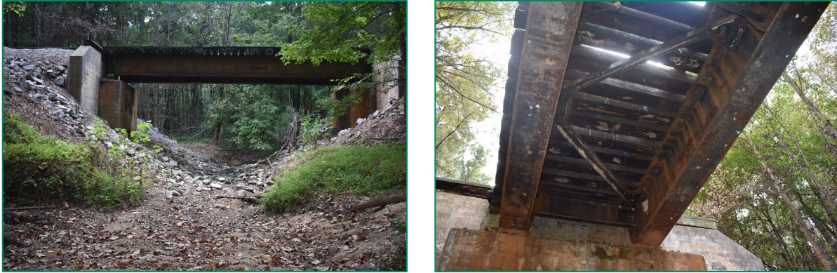
Figure 92. Left, view of bridge's east elevation, looking west; right, detail view of bridge's deck and I-beams.
