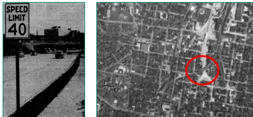
Figure 61. Left, photograph of Capital Boulevard with bridge in background from 1955 News and Observer article; right, detail of 1955 NCDOT aerial image with the bridge outlined in red and new "Downtown" Boulevard under construction.
