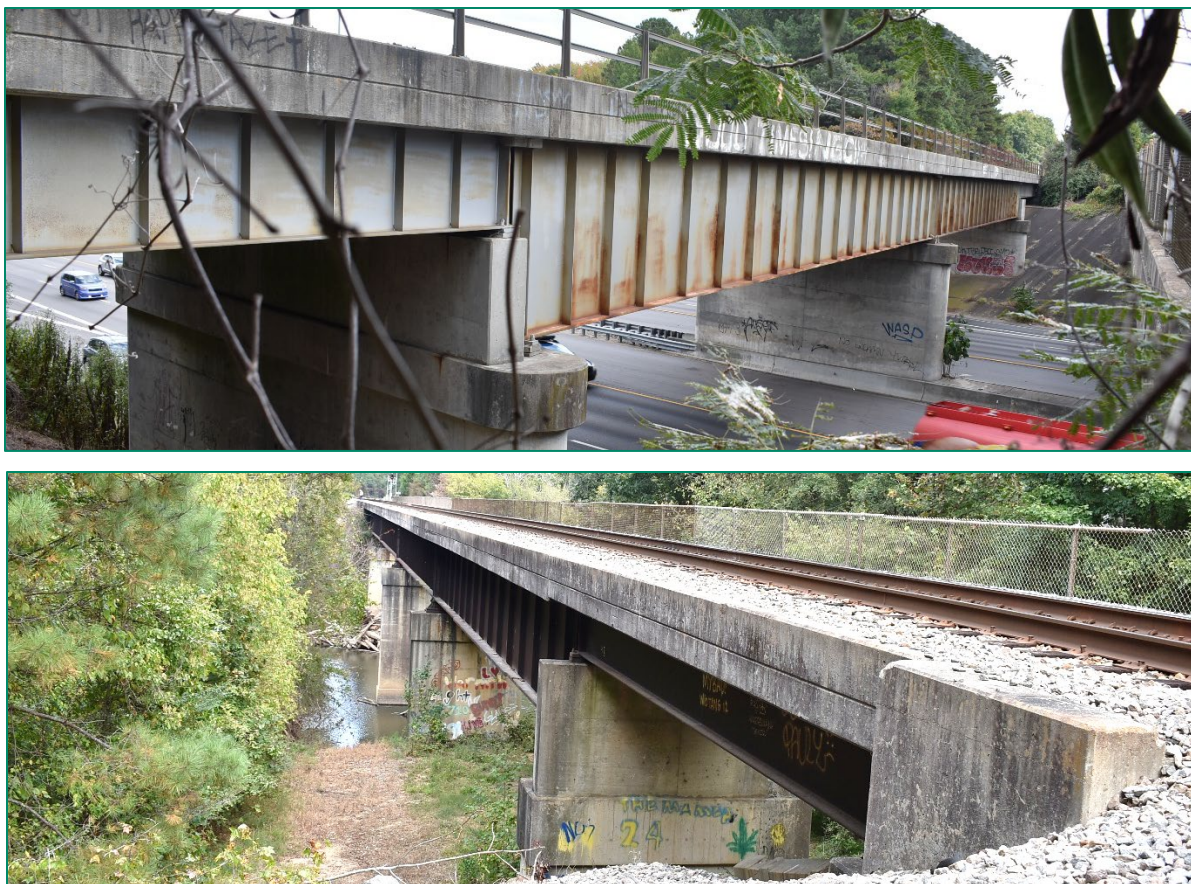
Figure 26. 1983 welded plate girder bridge over I-40, at top; 1972 Deep River bridge with welded plate girder spans and shallower deck beam approaches, at bottom.
