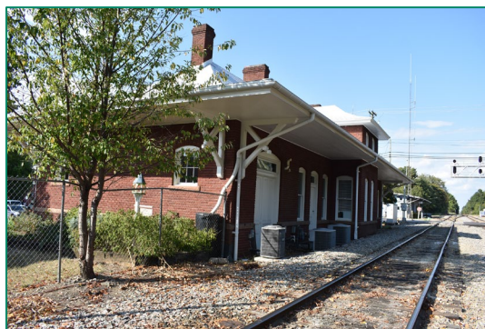
Figure 79. Apex Union Depot, south and east elevations and railroad tracks, looking north.
