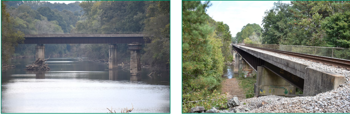
Figure 89. Left, view of bridge's north elevation (stone pier from earlier crossing in right foreground), looking east; right, view of bridge's tracks and deck, looking south.
