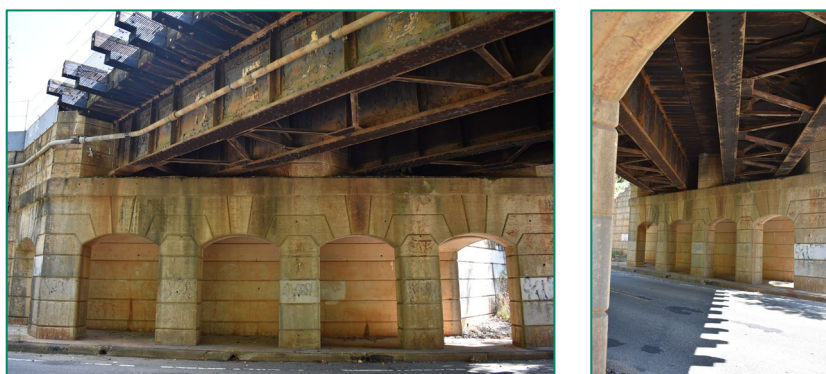
Figure 68. Left, view of bridge's substructure and underside of superstructure from eastern walkway, looking southwest; right, detail view of bridge's girders and ties from eastern walkway.
