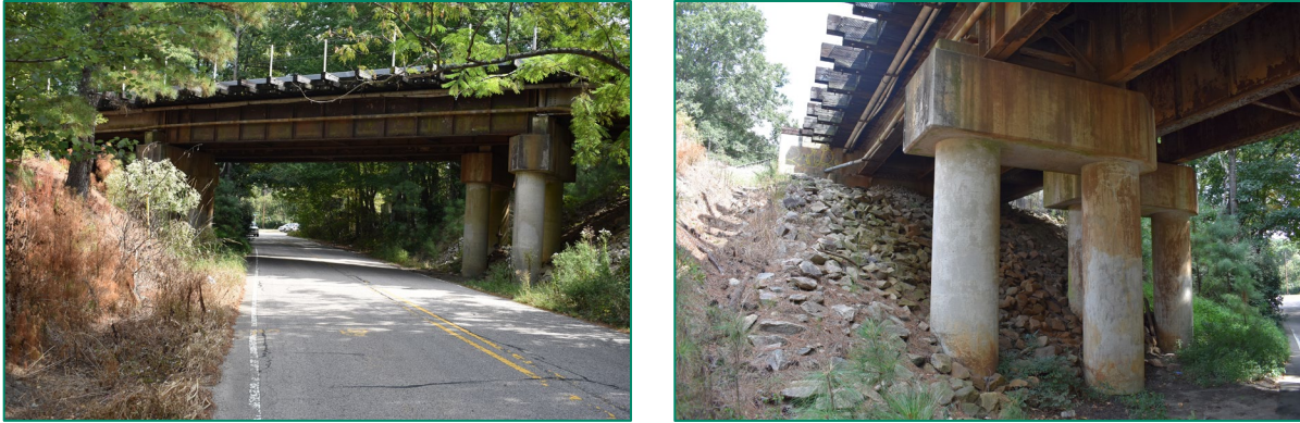
Figure 72. Left, view of bridge's east elevation, looking west; right, detail view of bridge's bent and underside of superstructure.
