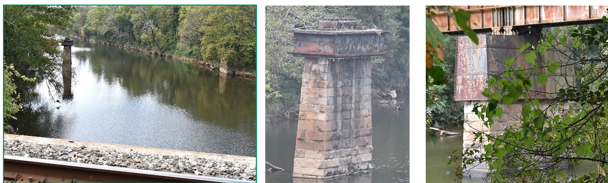
Figure 23. Looking northwest at two surviving Deep River Bridge stone piers, at left, and central pier, at center; looking northeast at central stone pier of Haw River Bridge, at right.
