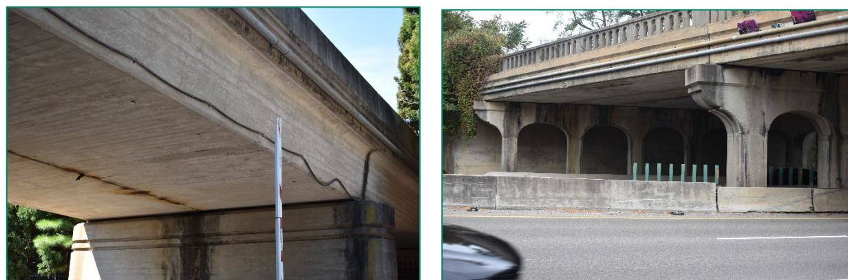
Figure 29. At left, concrete-covered steel-stringer superstructure of early 1950s Dan Allen bridge in Raleigh, looking southwest; at right, 1955 concrete slab bridge over Capital Boulevard, Raleigh, looking west.
