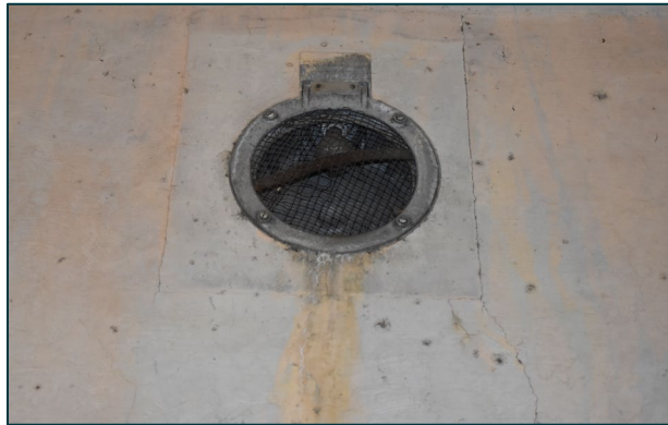
Figure 83. Detail view of porthole-like lights that line wall of walkway.
