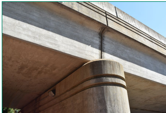
Figure 65. Detail view of bridge's bent and underside of superstructure from western walkway.
