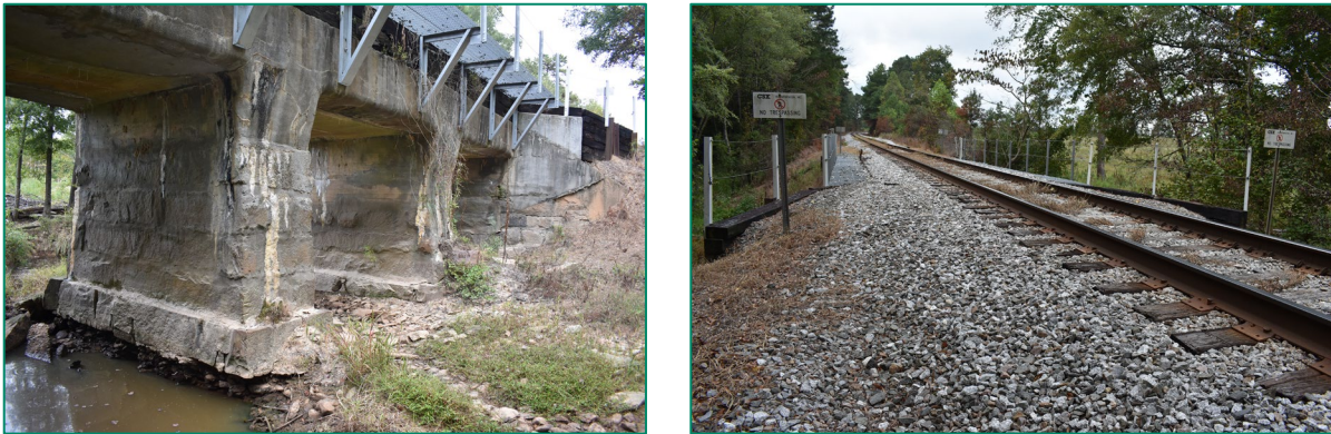
Figure 86. Left, SAL Bridge over Shaddox Creek, east approach including stone piers covered in concrete and abutment, looking northeast; right, SAL Bridge over Shaddox Creek, deck and tracks, looking northwest.
