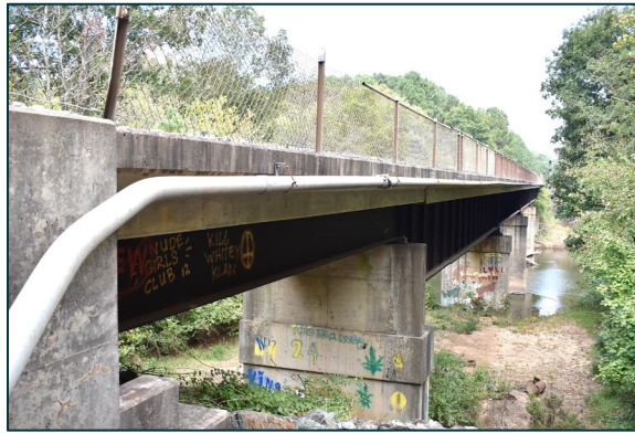
Figure 90. View of bridge's girders, beams, and bents, looking north.
