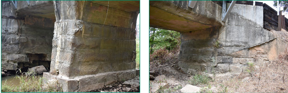
Figure 24. Shaddox Creek Bridge stone and later-extended concrete substructure looking west, at left, and north, at right.
