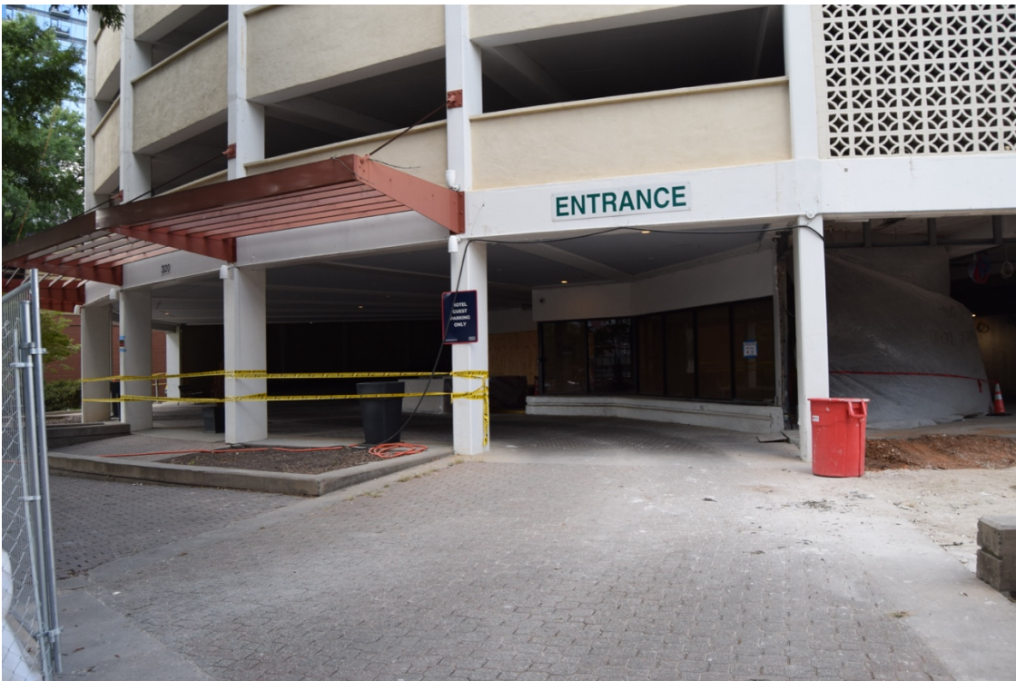
State Capitol Holiday Inn (WA8030), 320 Hillsborough Street, Raleigh, Wake County, showing vehicular entry to building at Hillsborough Street side, view northwest. The awnings seen here have since been removed.
