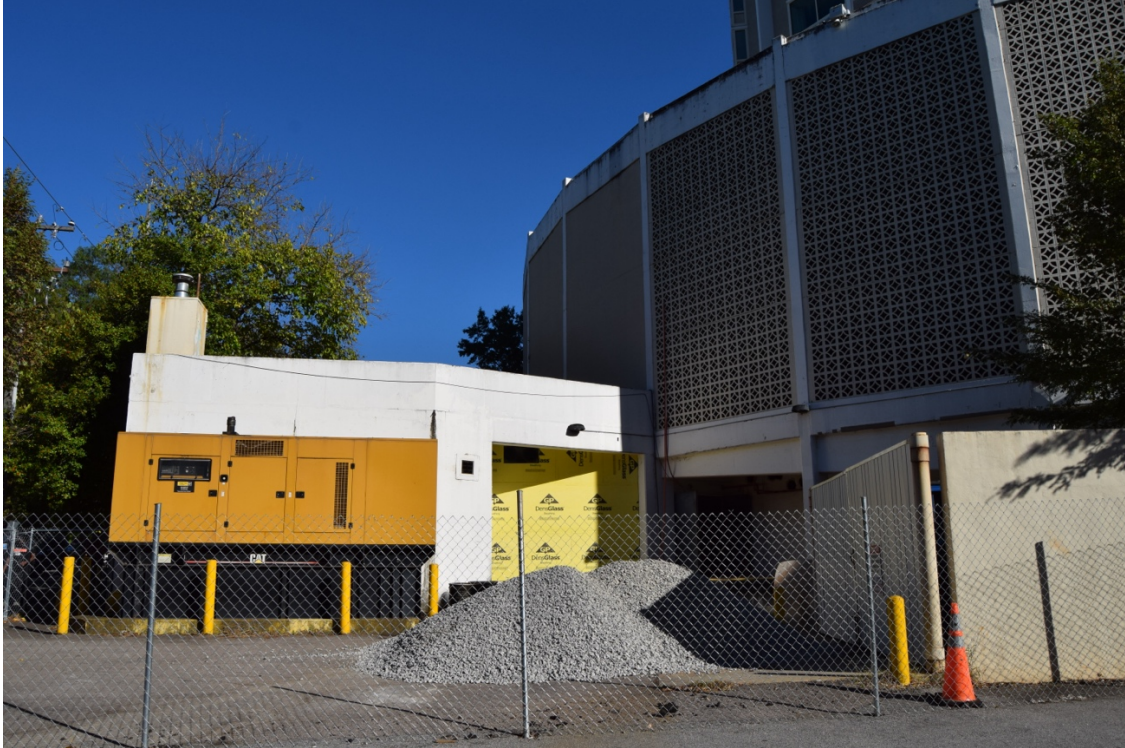
State Capitol Holiday Inn (WA8030), 320 Hillsborough Street, Raleigh, Wake County. Base at the north side of the building, showing loading dock wing.
