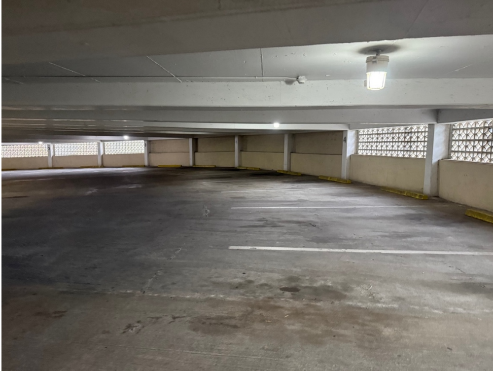
State Capitol Holiday Inn (WA8030), 320 Hillsborough Street, Raleigh, Wake County. Parking garage interior in 2024, photo by Caitlin Herrnsstadt, Heritage Consulting Group.
