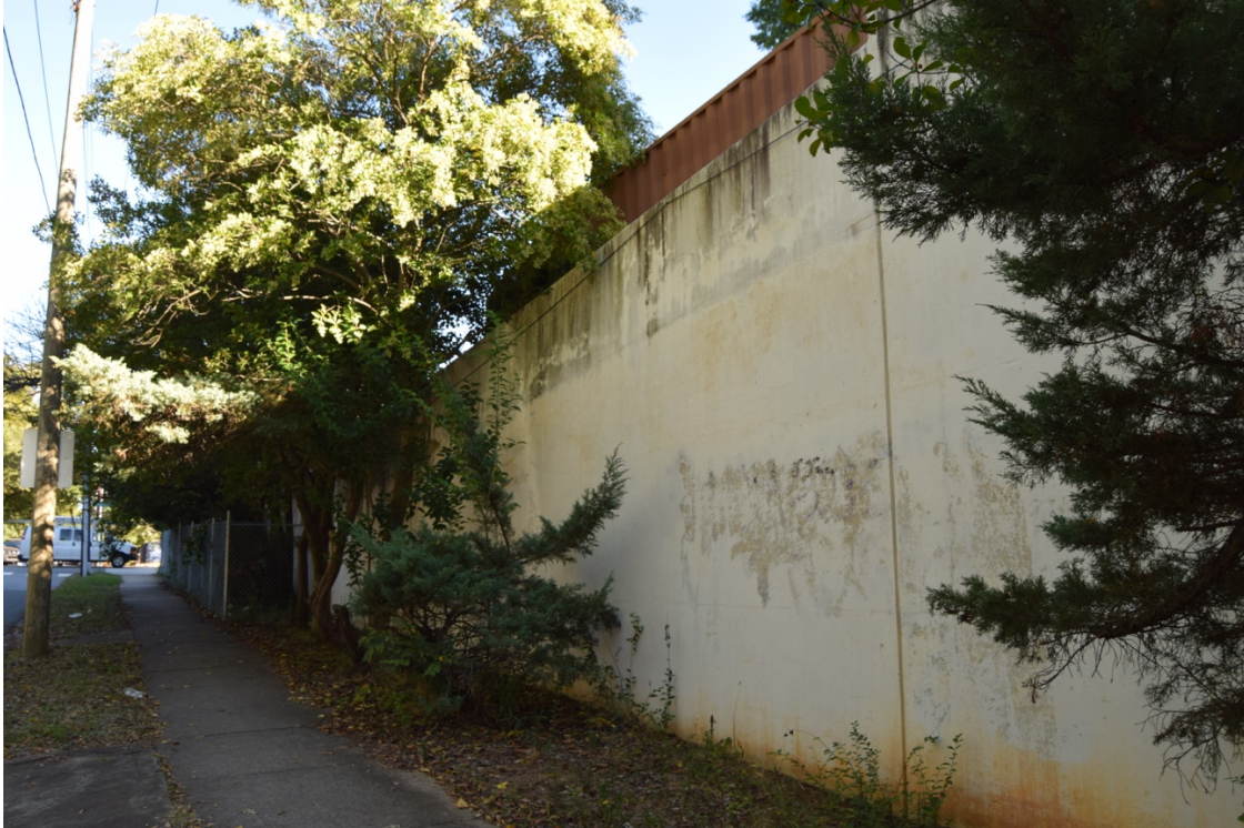
State Capitol Holiday Inn (WA8030), 320 Hillsborough Street, Raleigh, Wake County. View east-southeast along wall at the north property line.
