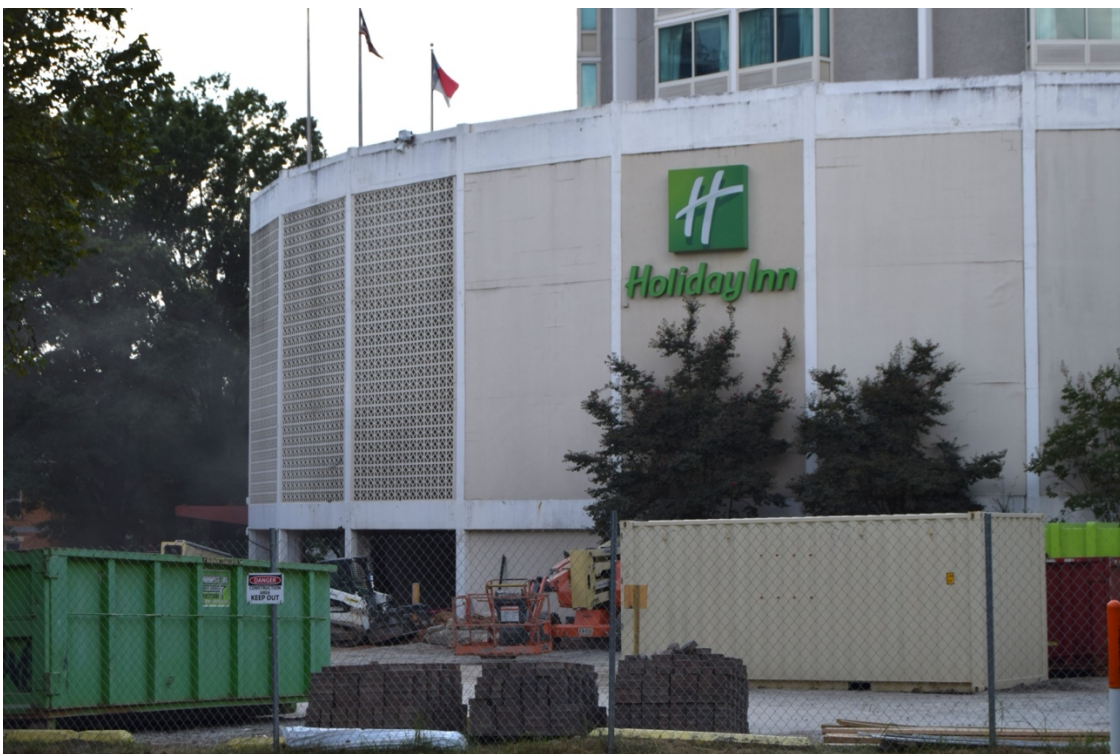
State Capitol Holiday Inn (WA8030), 320 Hillsborough Street, Raleigh, Wake County. Base at southeast curve of the building, showing breezeblock and solid panels.
