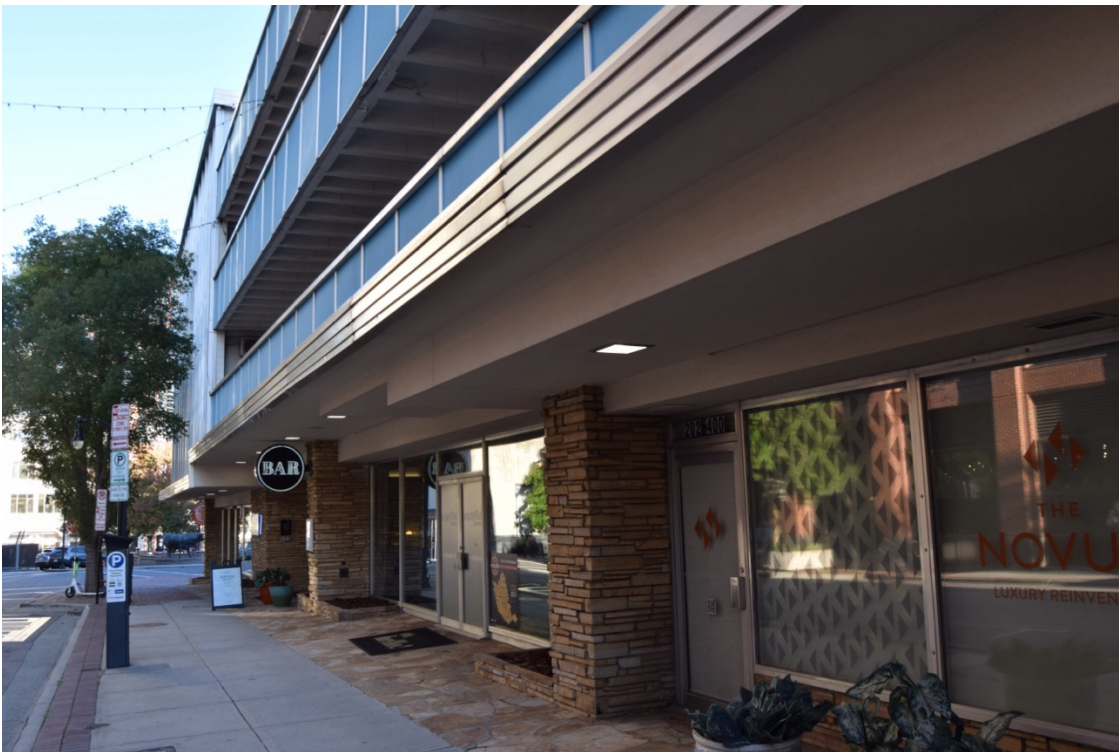
Jack Tar Motel (DH3342) on Corcoran Street in the Downtown Durham Historic District (DH1692), view to west showing storefronts at Parrish Street elevation with parking deck levels above.
