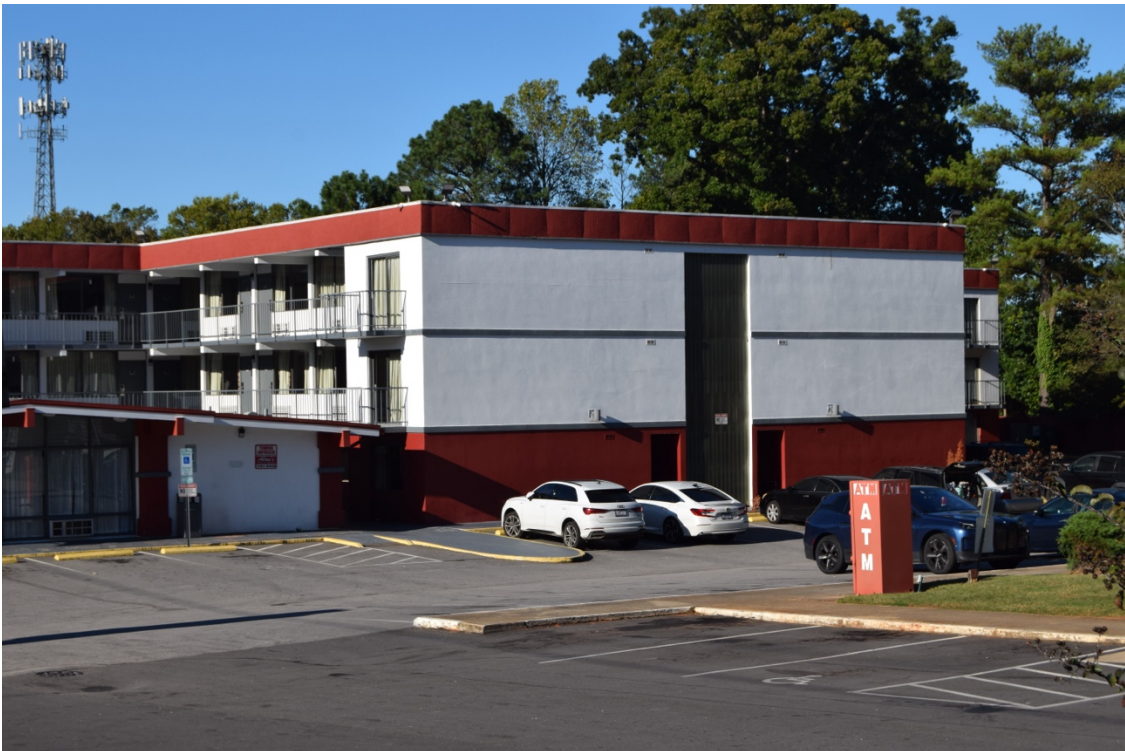
Happy Inn Motel (WA8119) at 3901 S. Wilmington Street, Raleigh, view to north.
