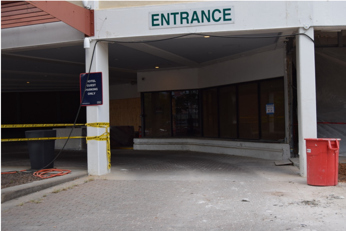
State Capitol Holiday Inn (WA8030), 320 Hillsborough Street, Raleigh, Wake County, showing exterior wall of lobby at vehicular entrance to the building. View northwest.
