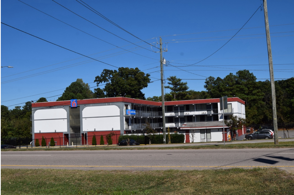
Happy Inn Motel (WA8119) at 3901 S. Wilmington Street, Raleigh, view to north east, showing courtyard between three-story building and single-story office.
