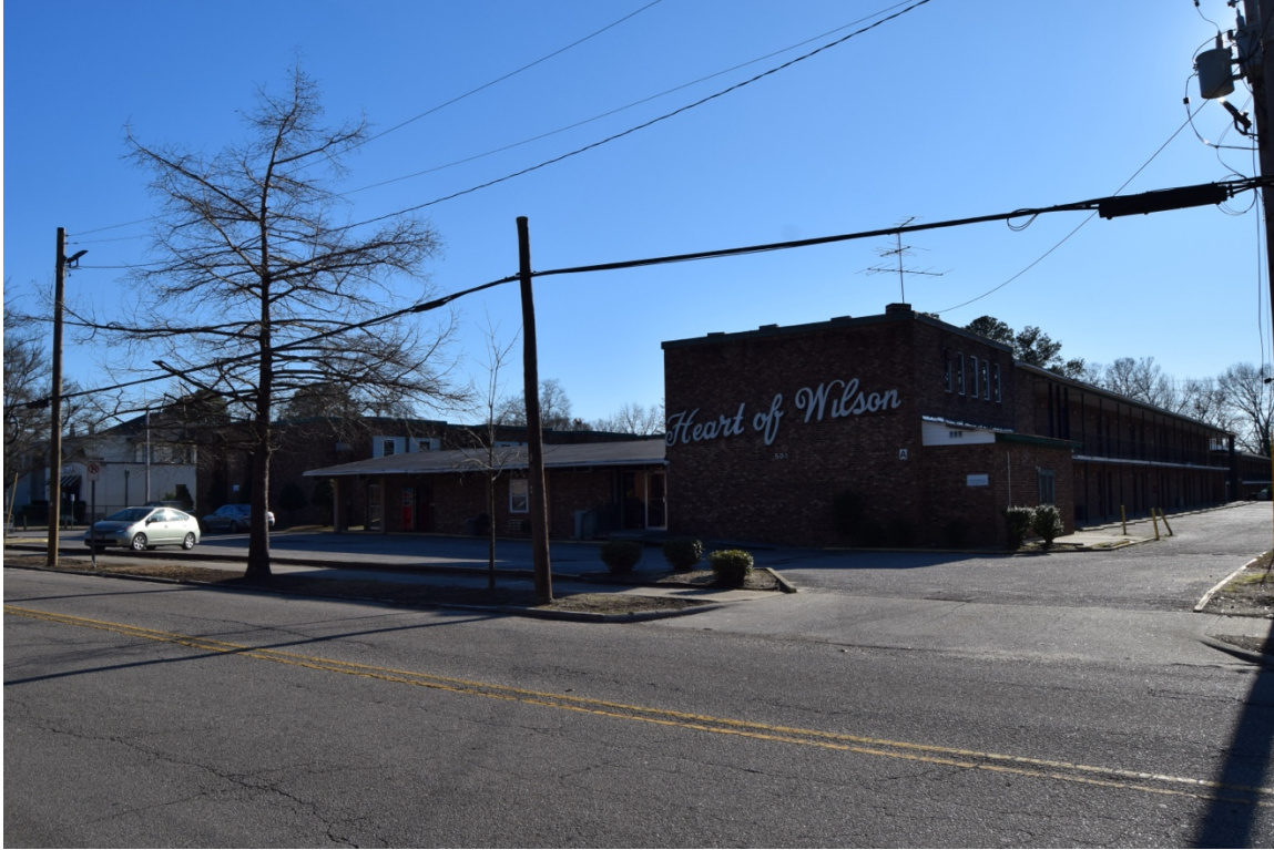
Urbanna Inn/Heart of Wilson Motor Inn (WL2381), 501 Nash Street West, Wilson, Wilson County, view south.
