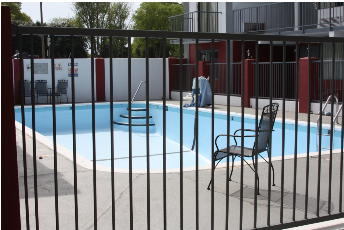
Happy Inn Motel (WA8119) at 3901 S. Wilmington Street, Raleigh, view of swimming pool. Photograph by Jenny Harper from 2018 survey.
