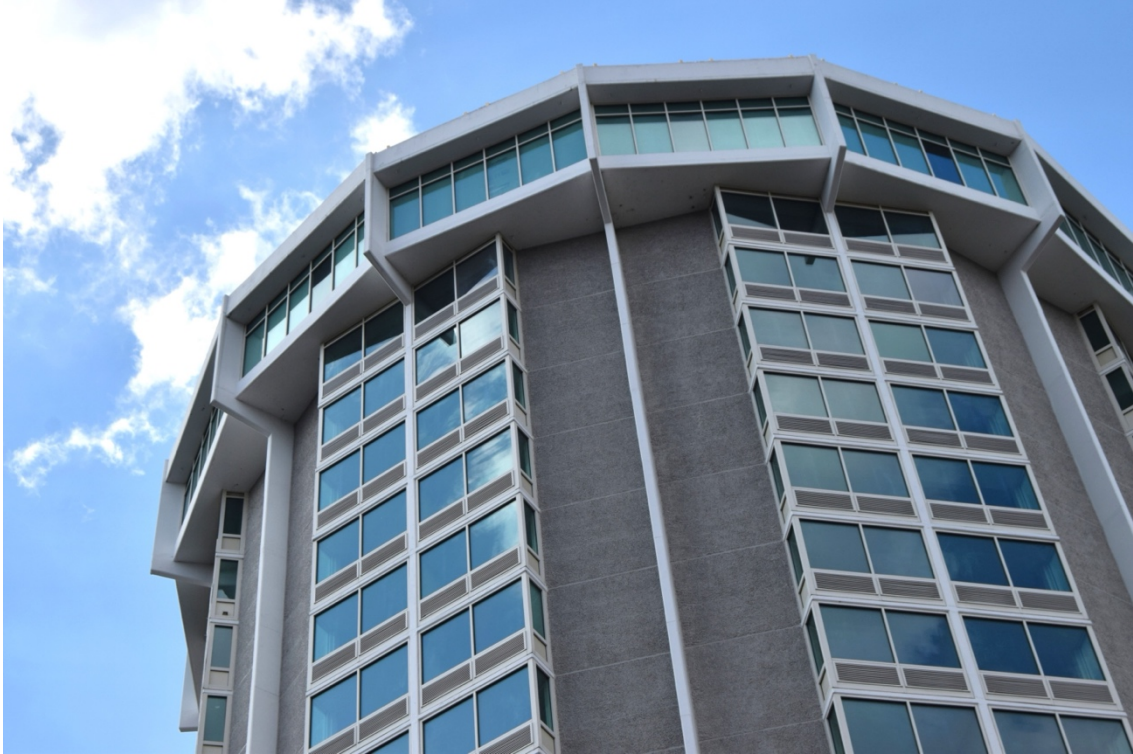
State Capitol Holiday Inn (WA8030), 320 Hillsborough Street, Raleigh, Wake County. View of upper stories including projecting top floor, looking northwest.
