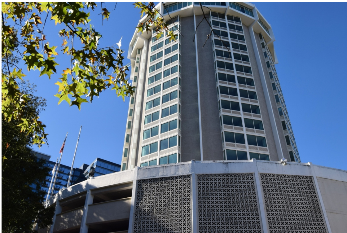
State Capitol Holiday Inn (WA8030), 320 Hillsborough Street, Raleigh, Wake County. View of guest room floors at the shaft section of the building, looking northwest.
