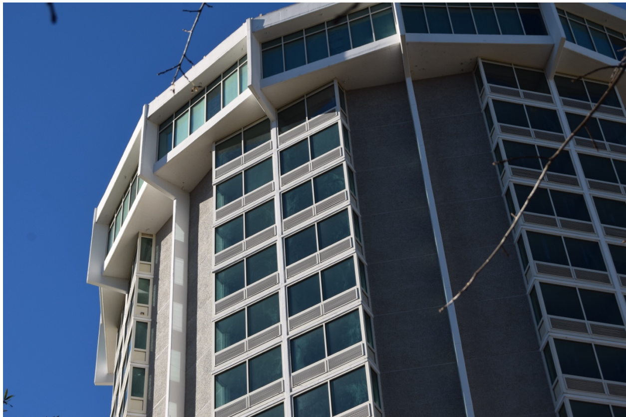
State Capitol Holiday Inn (WA8030), 320 Hillsborough Street, Raleigh, Wake County. View of uppermost stories from east side.
