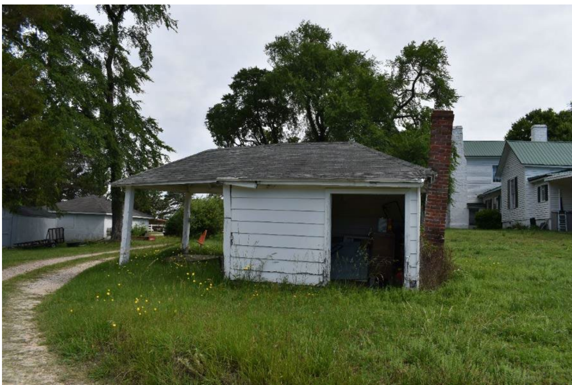
Photograph 17: 5104 Riley Hill Road, Washhouse facing north
