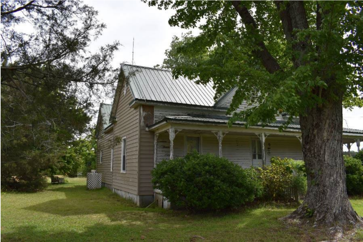
Photograph 3: Jones Tenant House, 2617 Rolesville Road, Facade (south elevation) and west elevation
