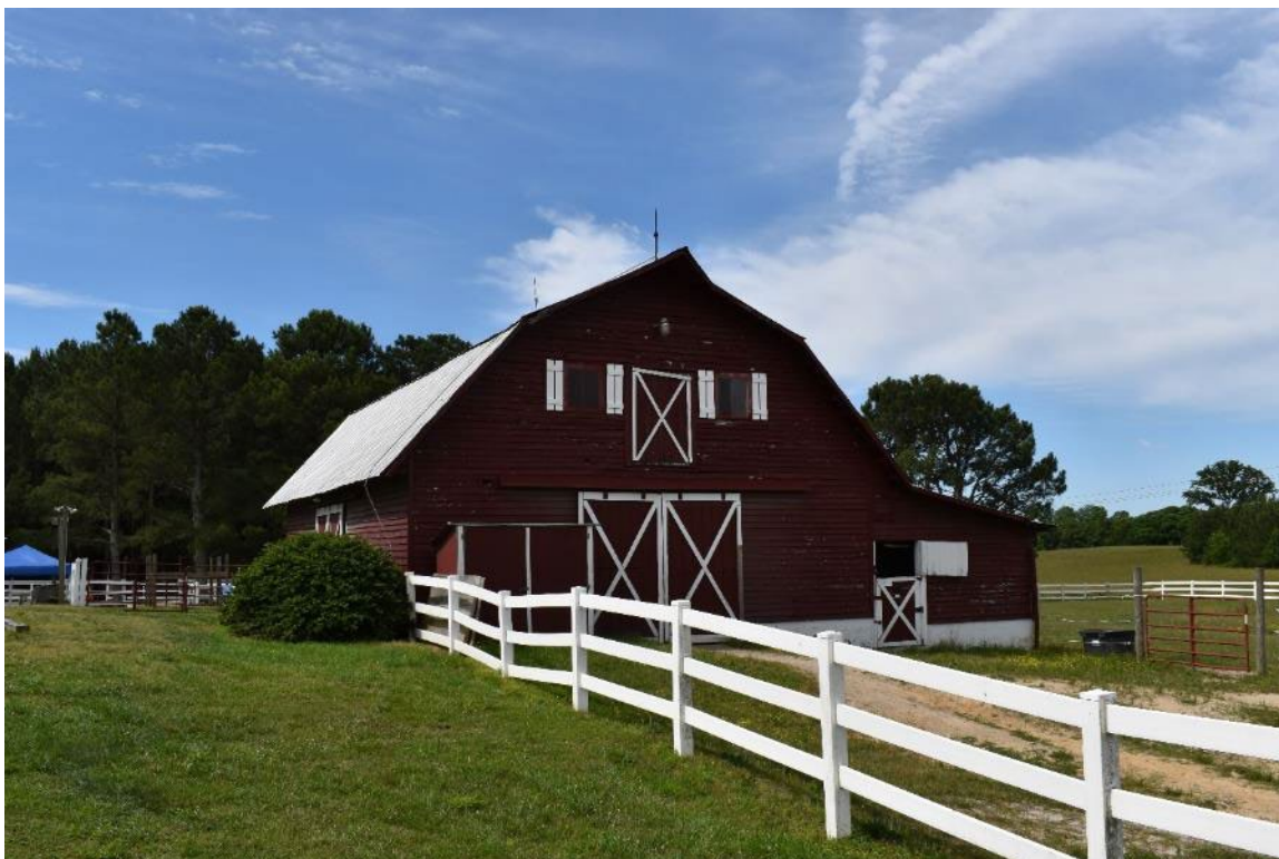
Photograph 24: 5104 Riley Hill Road, Barn, north elevation
