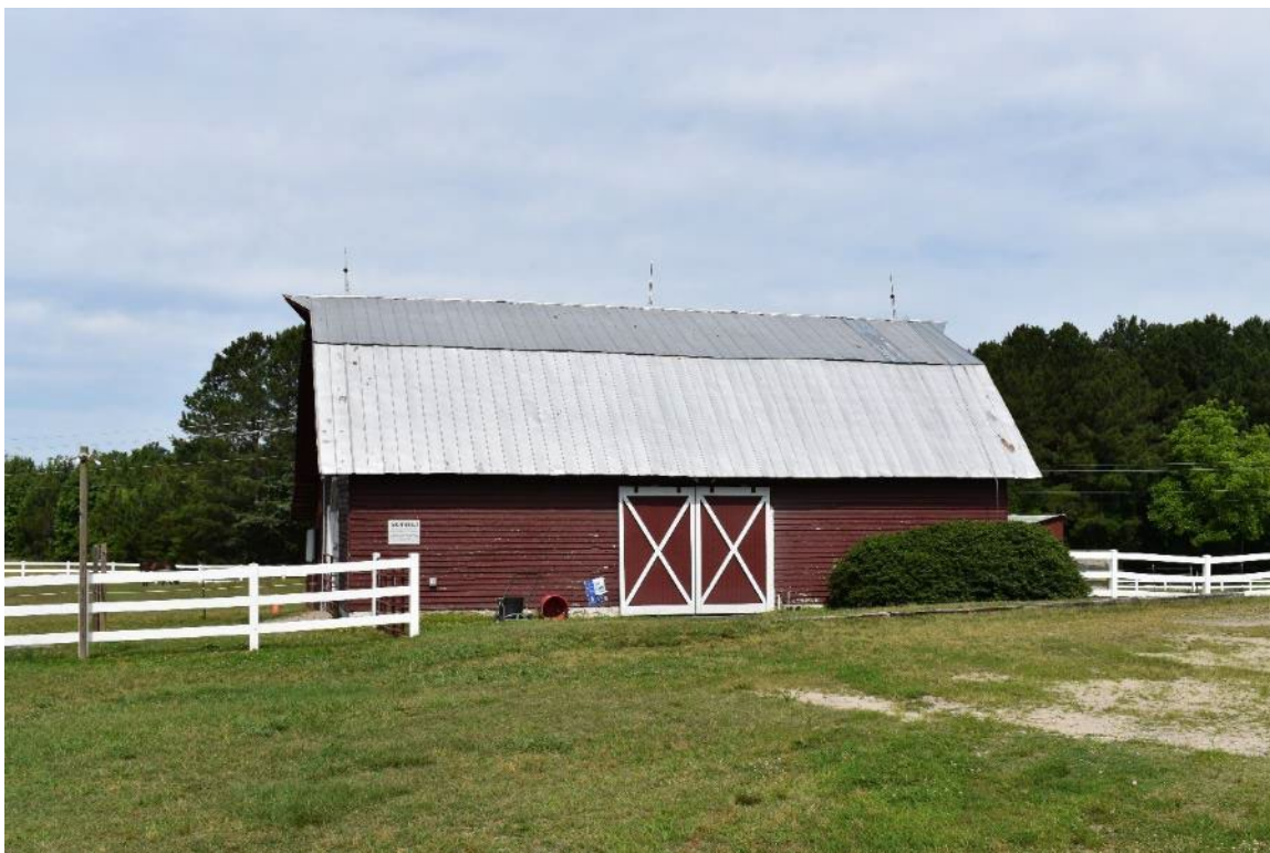
Photograph 22: 5104 Riley Hill Road, Barn, west elevation
