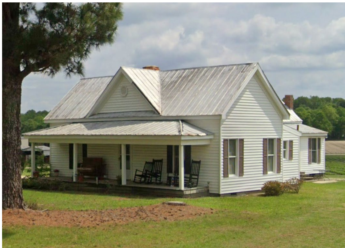
Figure 11: Ogburn-Honeycutt House (WA1142)
