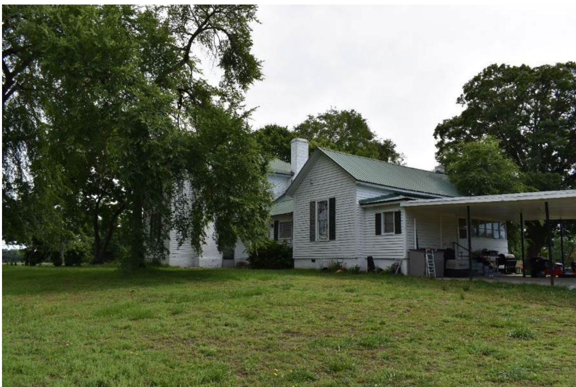
Photograph 15: 5104 Riley Hill Road, West elevation and rear (south elevation)
