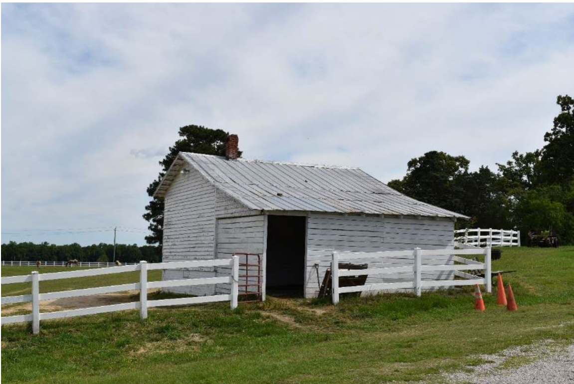
Photograph 27: 5104 Riley Hill Road, Rear of packhouse
