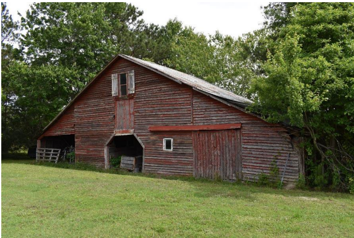
Photograph 6: Jones Tenant House, 2617 Rolesville Road, Barn facing southwest
