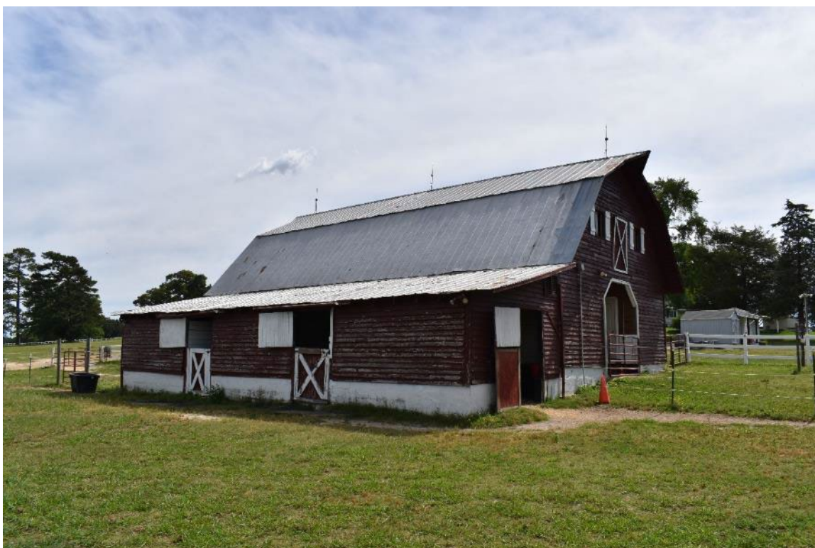
Photograph 25: 5104 Riley Hill Road, Barn, east elevation
