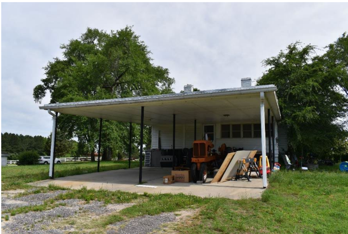
Photograph 16: 5104 Riley Hill Road, Rear (south elevation)
