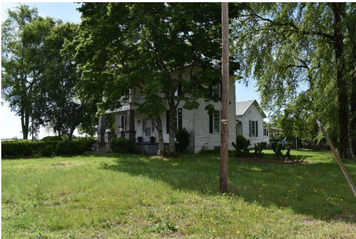
Photograph 14: 5104 Riley Hill Road, Facade (north elevation) and west elevation
