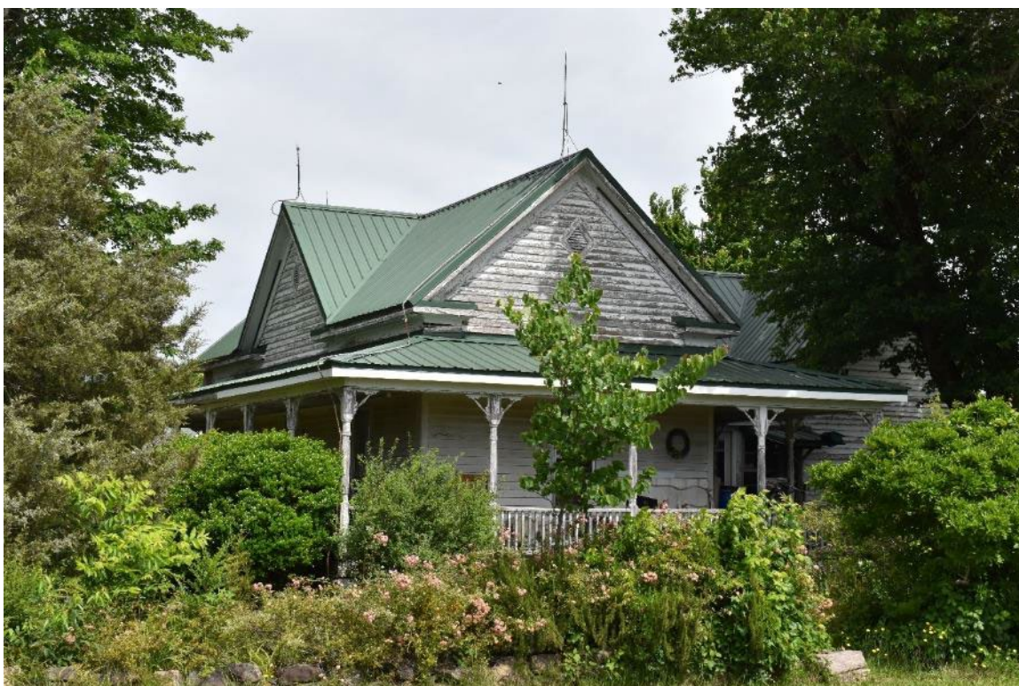
Photograph 2: Jones Tenant House, 2617 Rolesville Road, Facade (south elevation) and east elevation
