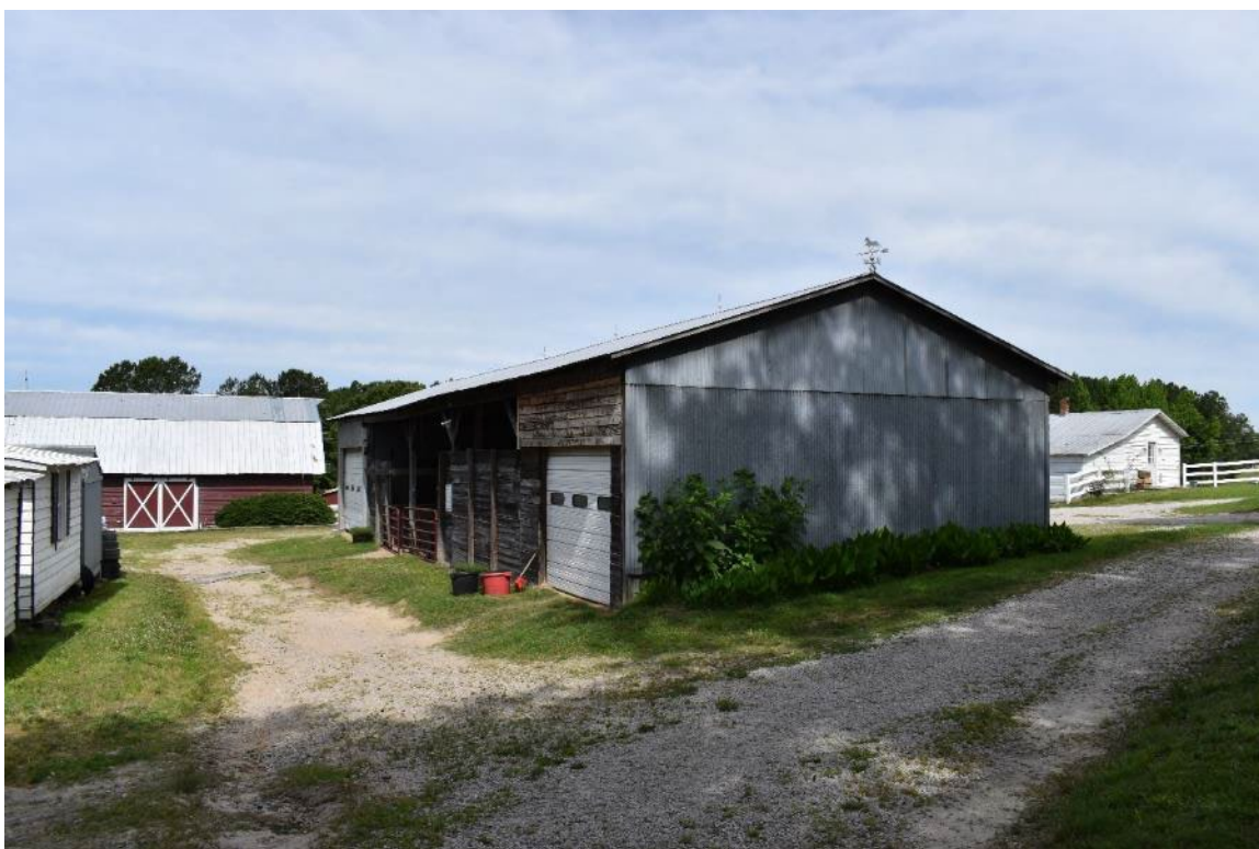
Photograph 21: 5104 Riley Hill Road, Metal shed southeast corner
