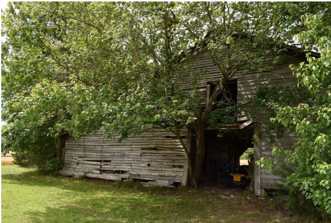
Photograph 7: Jones Tenant House, 2617 Rolesville Road, Backside of barn
