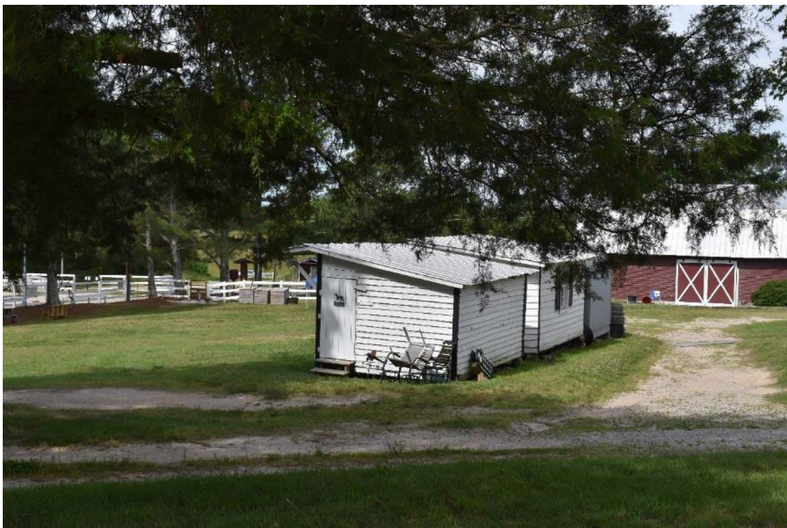
Photograph 18: 5104 Riley Hill Road, Outbuilding/chicken house facing northeast
