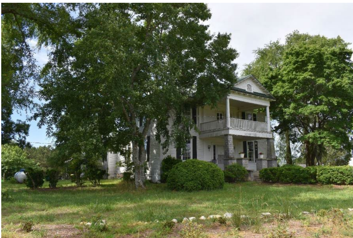
Photograph 13: 5104 Riley Hill Road, Facade (north elevation) and east elevation
