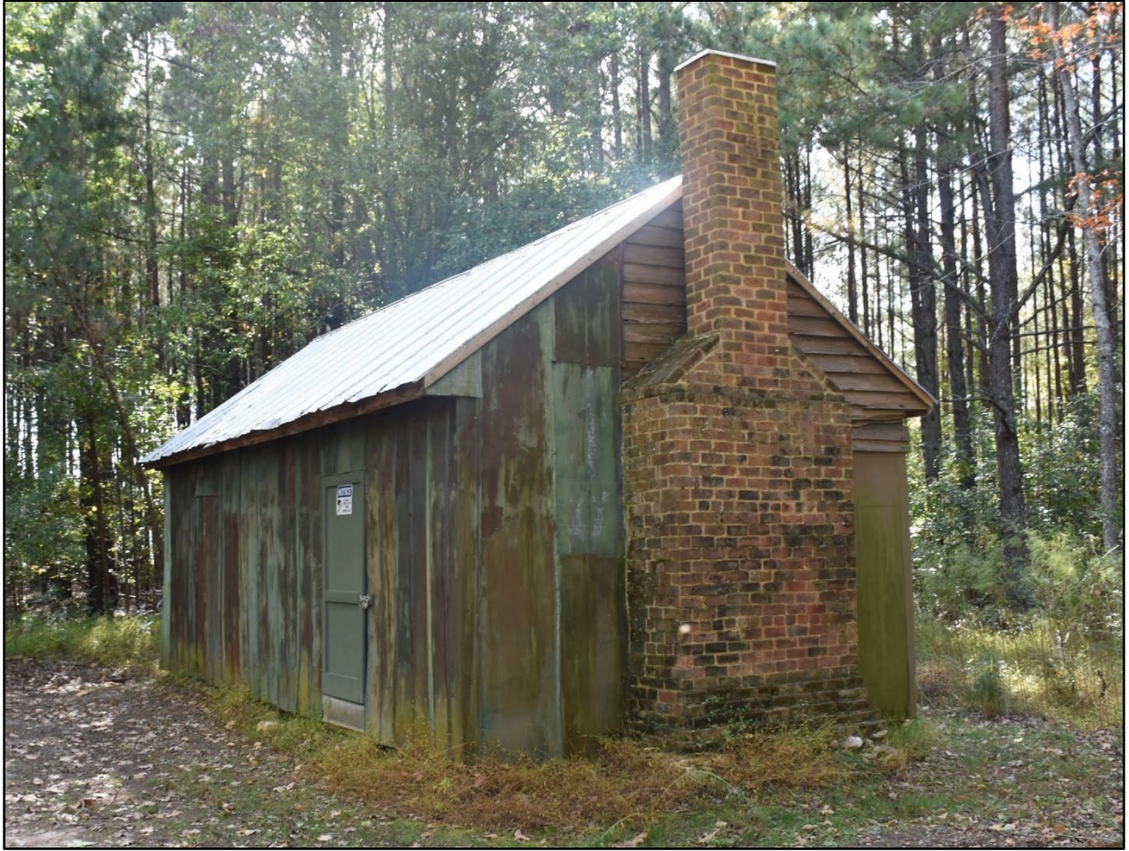
Figure 186- Oblique view of the Rueben Jones House/purported slave quarters, facing southwest.
