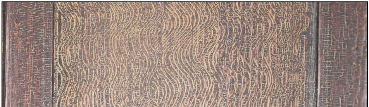
Figure 241- Detail of one of the wood-grained doors at the Barnabas Jones House for comparison.
