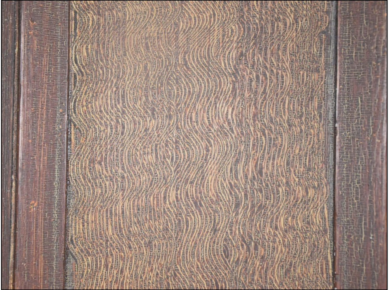
Figure 144- Detail of painted wood graining on one of the downstairs doors in the farmhouse.
