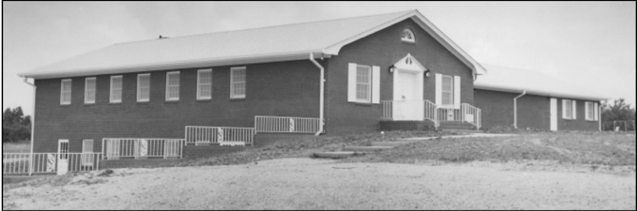
Figure 5- Circa 1965-1968 view of completed original sanctuary/educational building, facing northwest (Source: Macedonia Baptist Church archives).
