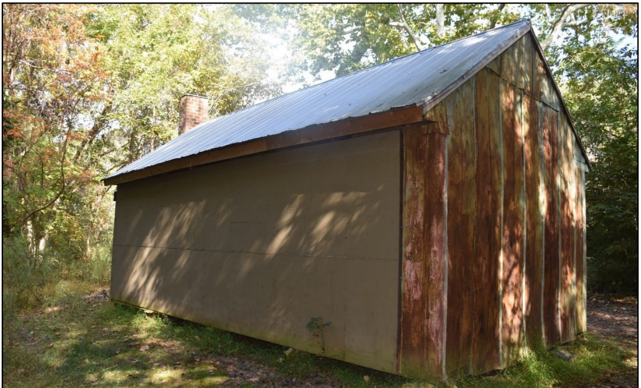
Figure 196- An oblique view of the structure from the southwest, with historic tin siding visible on the right/south elevation and non-historic modern siding visible on the left/west elevation (alongside the footprint of the shed-roofed addition visible in Figures 211 and 212 that was later removed).
