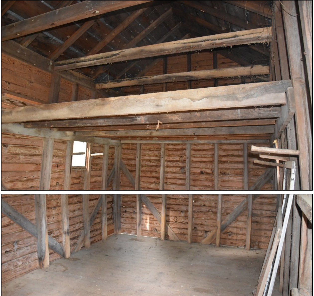
Figure 207- Composite image of the interior of the grain barn, facing north-northwest, with original wood framing visible throughout.
