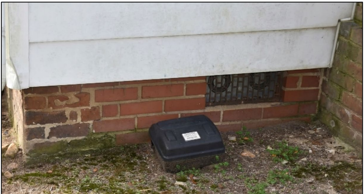
Figure 102- Original brick foundation piers (left) and brick chimney (right) on the southeast corner of the house, with a post-1961 brick foundation course between (compare with Figure 124).
