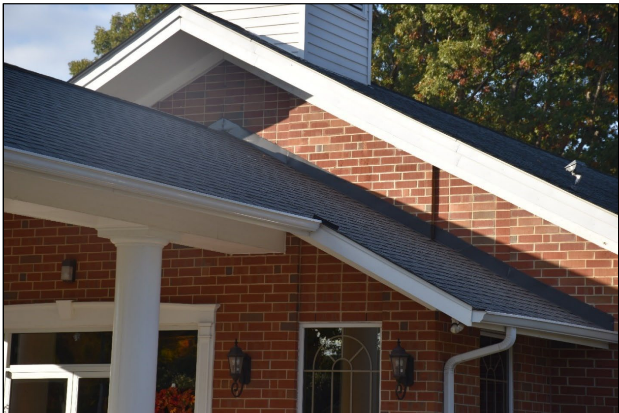
Figure 29- Detail of historic sanctuary and non-historic front addition and porte-cochère added between 2014 and 2015.
