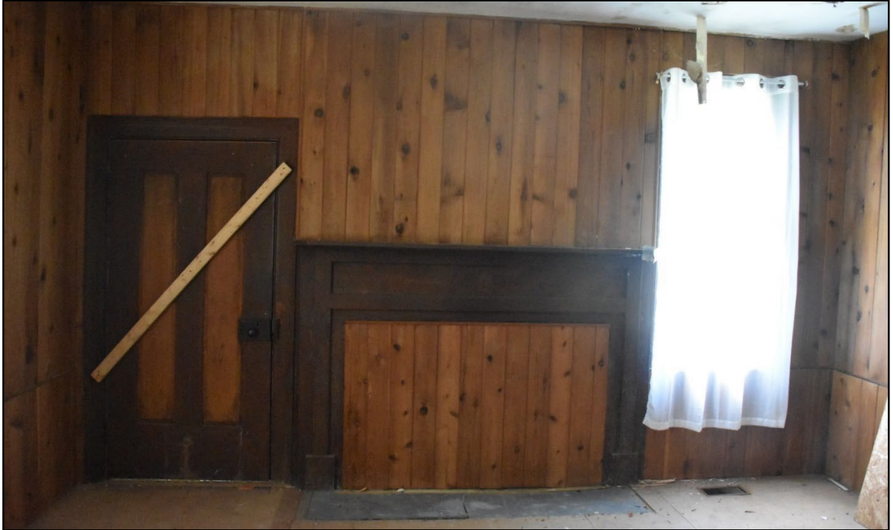
Figure 137- West wall of the west room on the first floor, featuring original door, window, and mantel as well as non-historic wood paneling.
