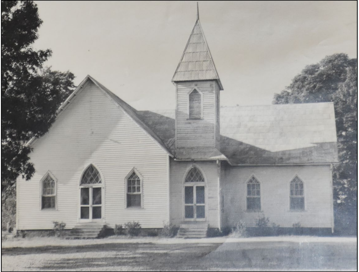
Figure 71- Image of the non-extant 1880 sanctuary, which was extended in 1910, 1919, and 1952, and demolished in September 1964 (Source: Swift Creek Baptist Church archives).
