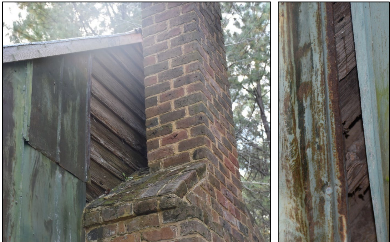
Figure 189 (left) and 190 (right)- View facing southwest of the original brick chimney on the north elevation; wood siding underneath the metal siding on the northeast corner of the house.
