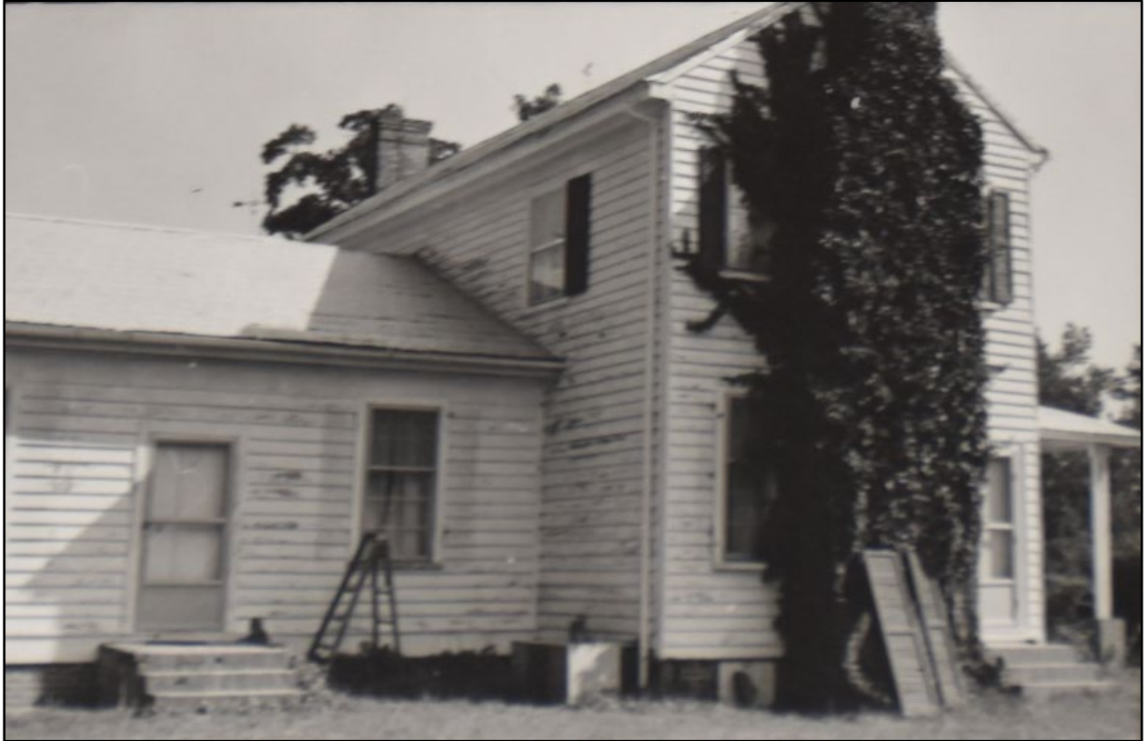
Figure 218- Undated photo of the west elevation of the main house from the WA0679 site file (Source: HPO).
