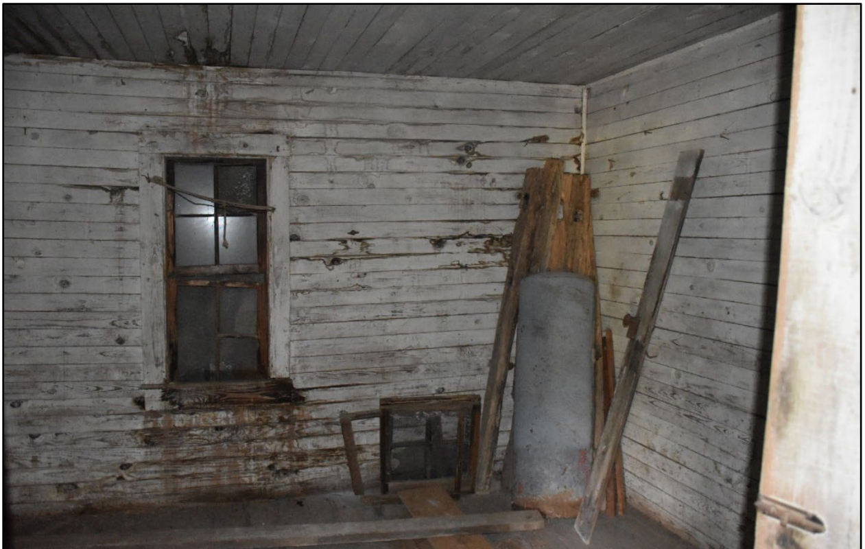
Figure 194- Looking towards the southwest corner of the south room, with historic wood walls and covered window visible.
