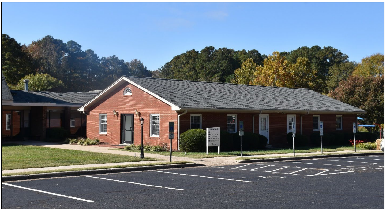
Figure 18- Oblique view of the second wing of the educational building, facing southwest.
