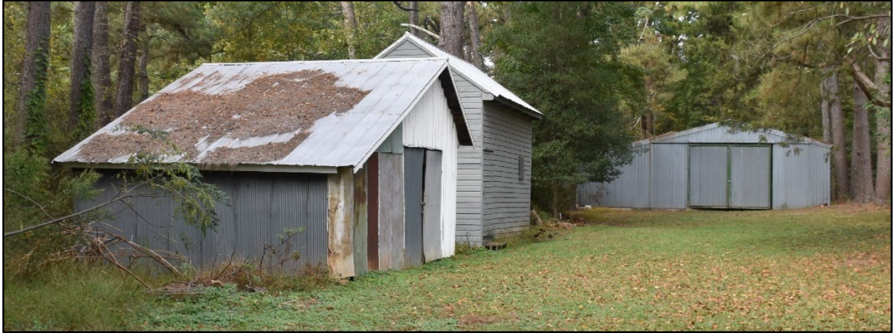
Figure 199- Overview of the farmstead's northwestern group of outbuildings, facing north: the circa 1840s/50s cider barn/shed (left), circa 1820s/30s grain barn (middle), and circa 1960s livestock barn (right).
