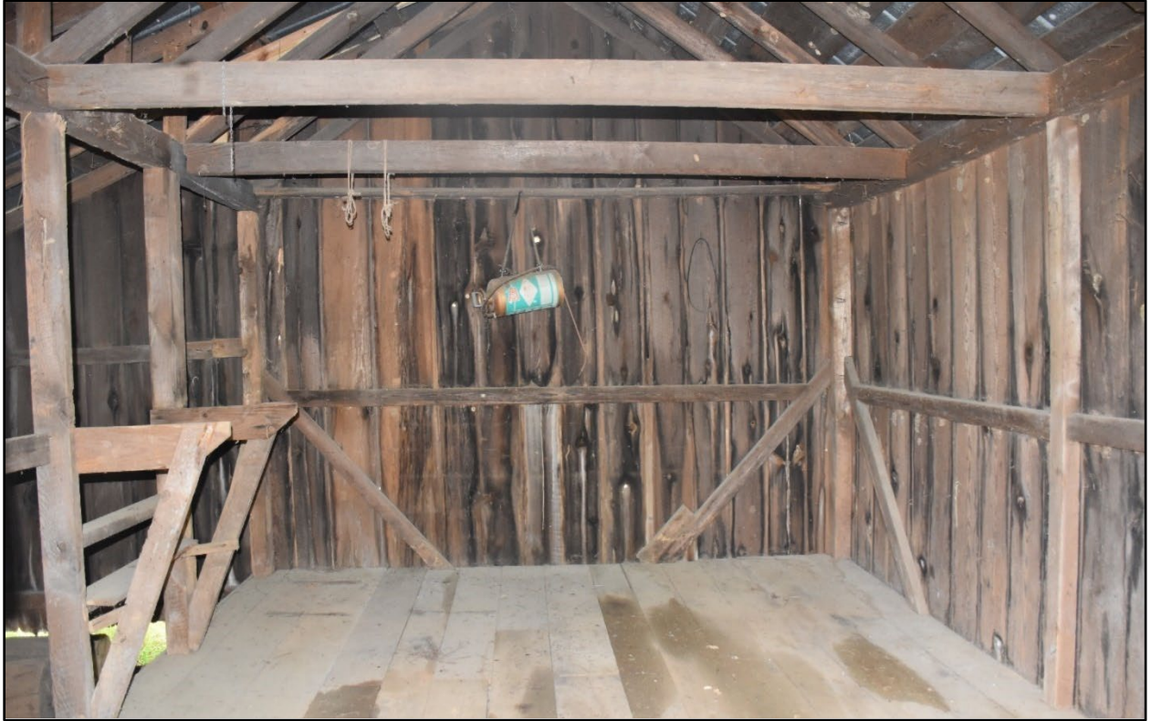
Figure 203- Interior view of the wood framing of the cider barn/shed, facing west.
