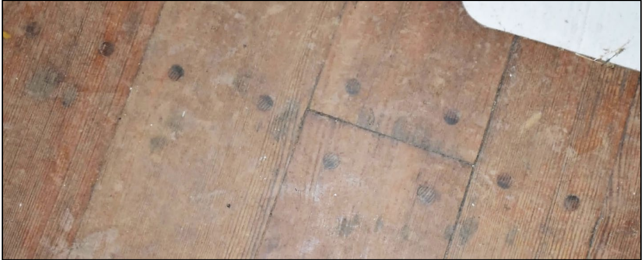
Figure 123- Historic wood floors in the rear ell, with wood plugs covering nail holes.
