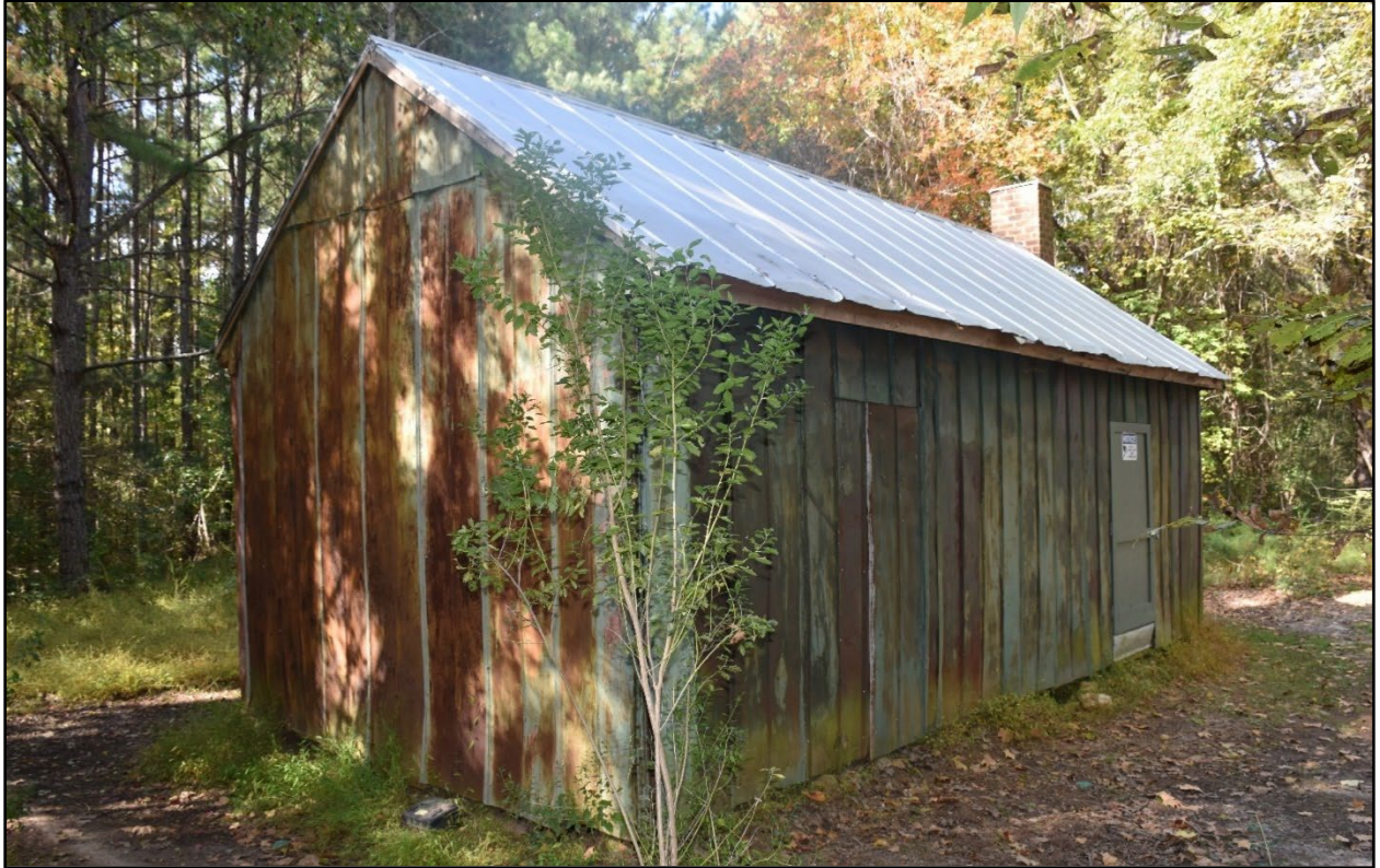
Figure 195- Oblique view of the purported slave quarters/Reuben Jones House from the southeast.
