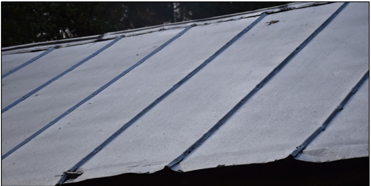
Figure 187- Detail of the standing seam metal roof, viewed from the northeast.
