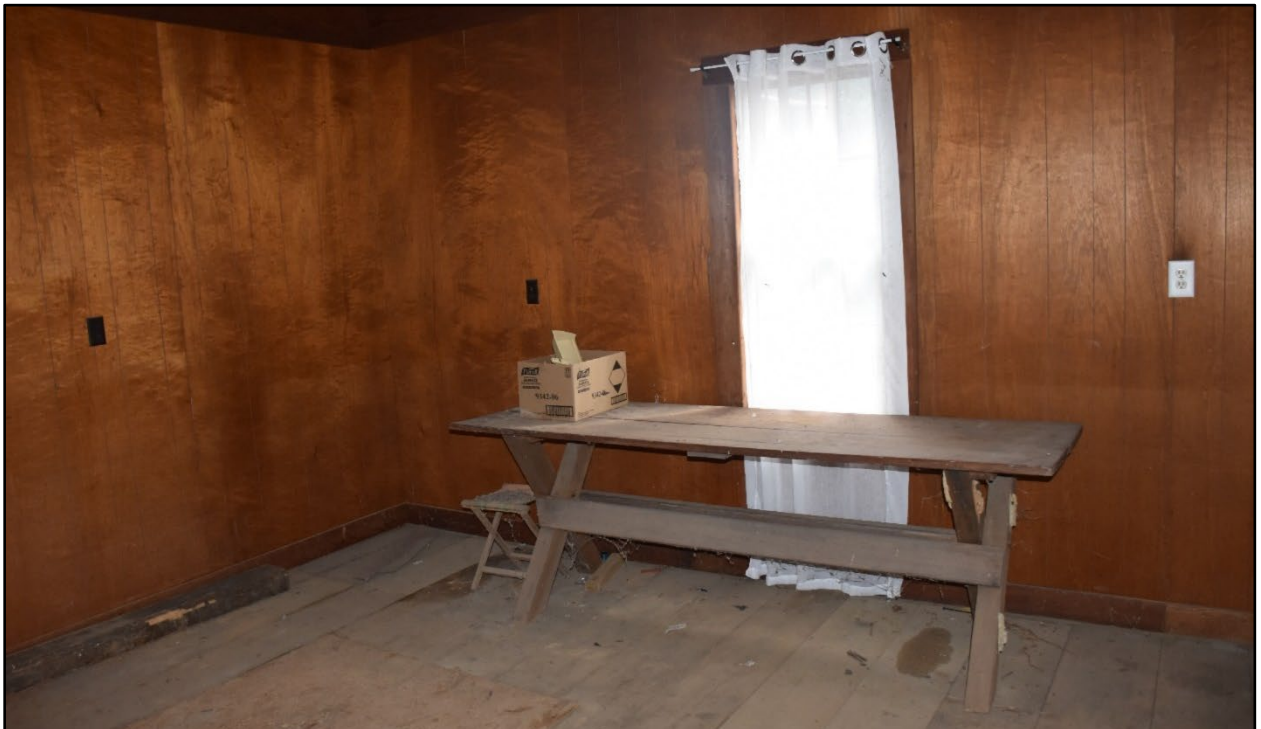
Figure 179- The south wall of the kitchen/schoolhouse, with historic wood floors and non-historic wood wall paneling.
