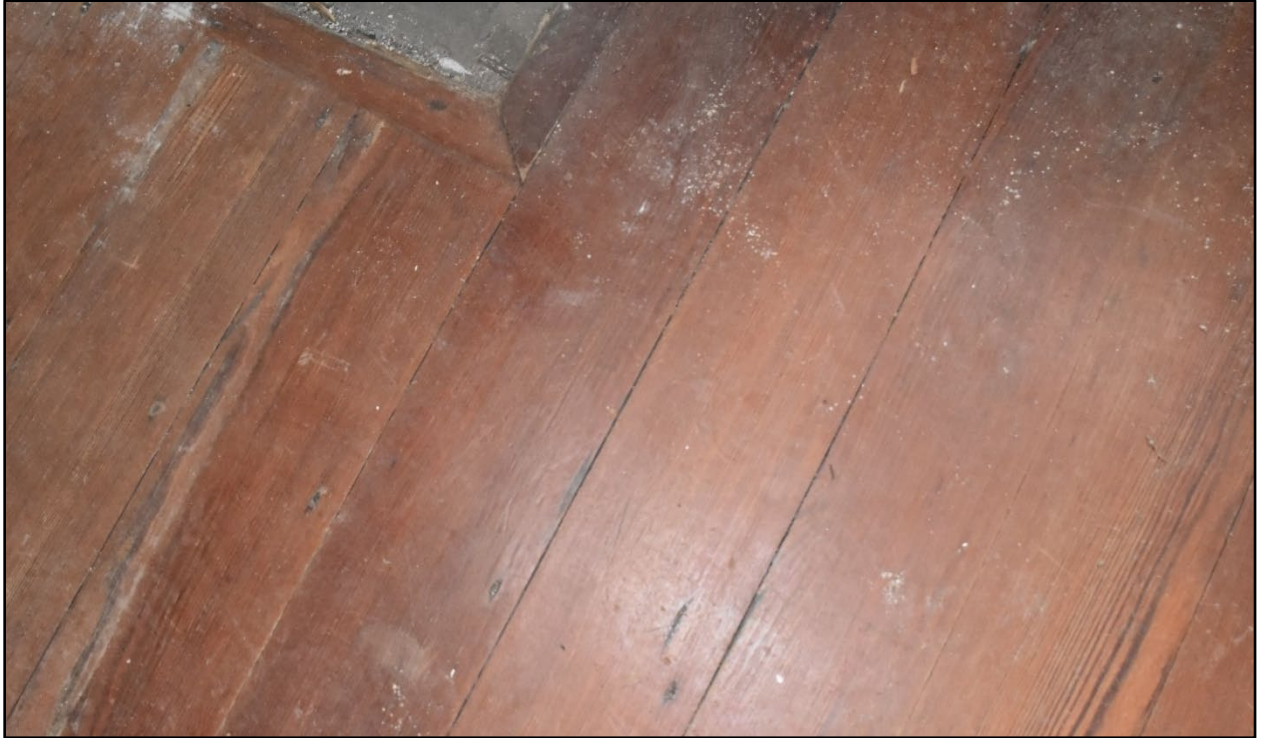
Figure 148- Intact pine flooring in the downstairs east room of the farmhouse.
