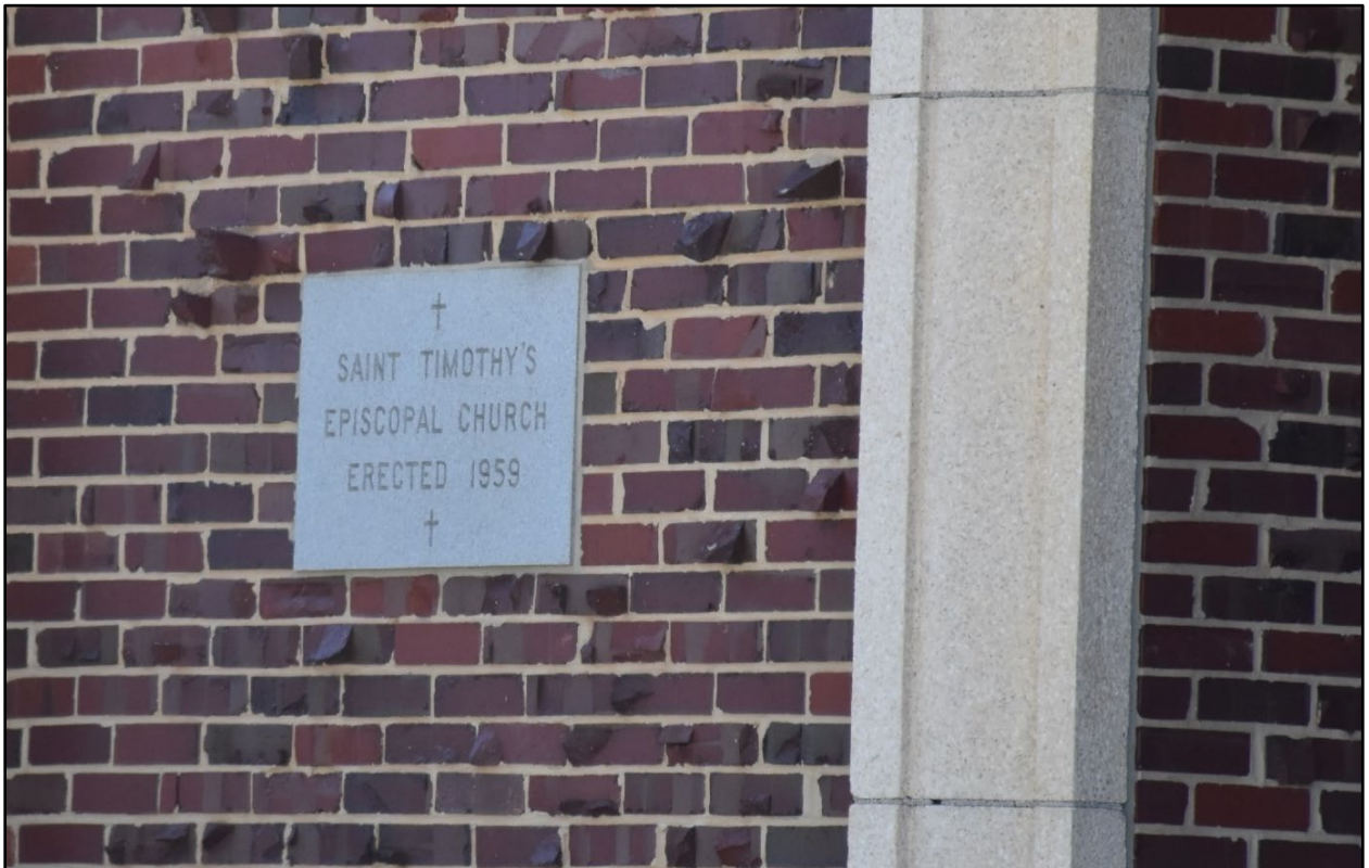
Figure 18- Detail of clinker brick and cornerstone at St. Timothy's Episcopal Church.
