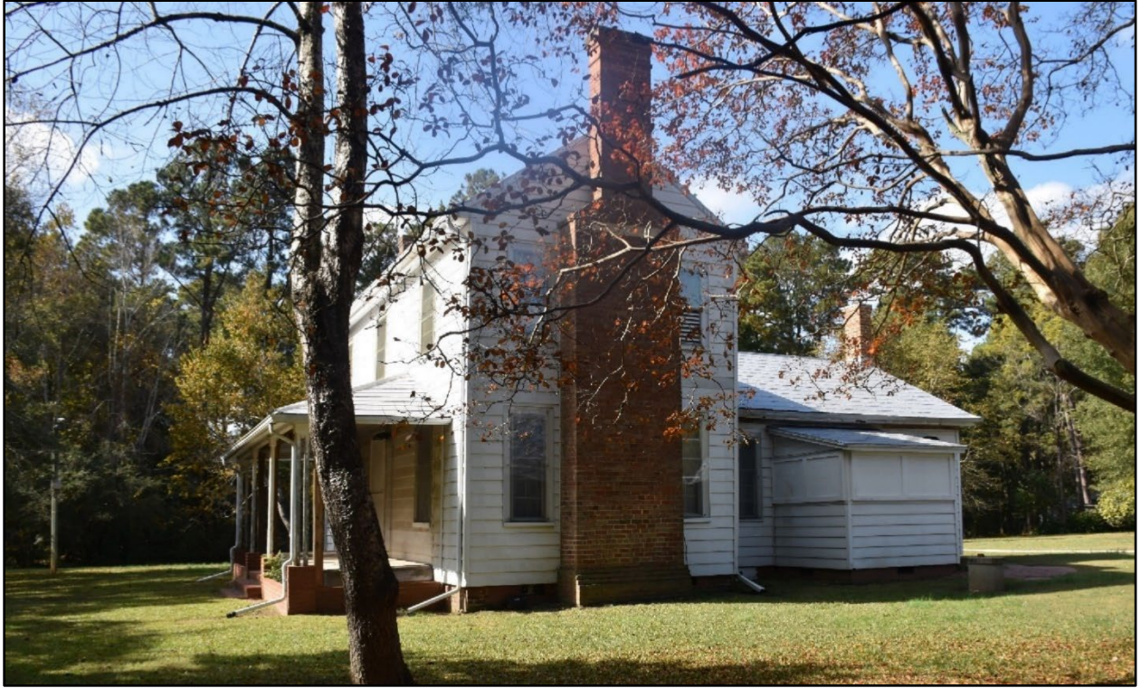
Figure 98- Oblique view of the main farmhouse, facing northwest.
