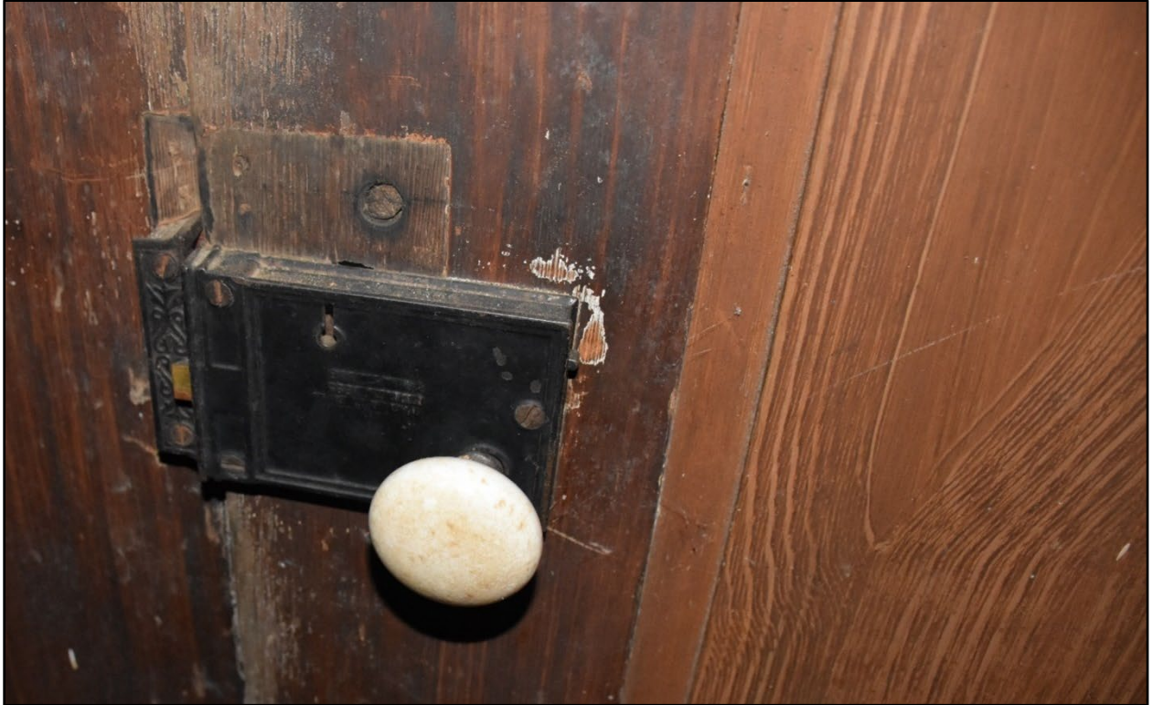
Figure 135- Detail of the hardware on the inside of the entry doors; note the two-tone painted wood graining on the doors and lack thereof in the footprint of the original entry hardware.
