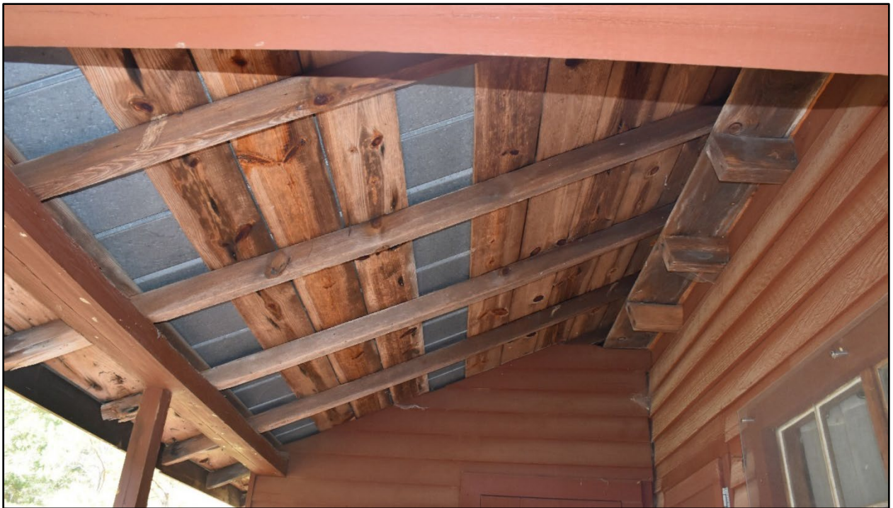
Figure 174- View looking up and to the north at the kitchen/schoolhouse porch ceiling.
