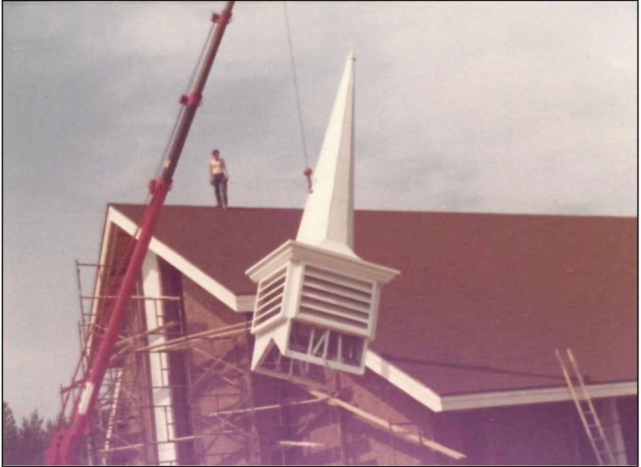
Figure 10- Hoisting the steeple onto the sanctuary roof, facing southwest (Source: Macedonia Baptist Church archives).
