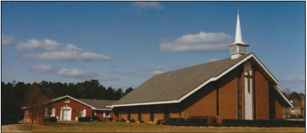
Figure 11- Circa 1970s/1980s view of the completed ensemble of church and educational wings, facing northwest (Source: Macedonia Baptist Church archives).
