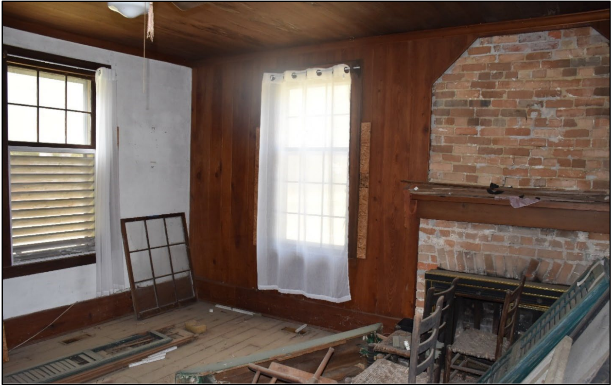
Figure 121- The rear ell of the house, facing northwest, with non-historic wood paneling on the back wall.
