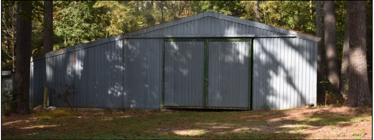
Figure 209- View of the south elevation of the livestock barn.
