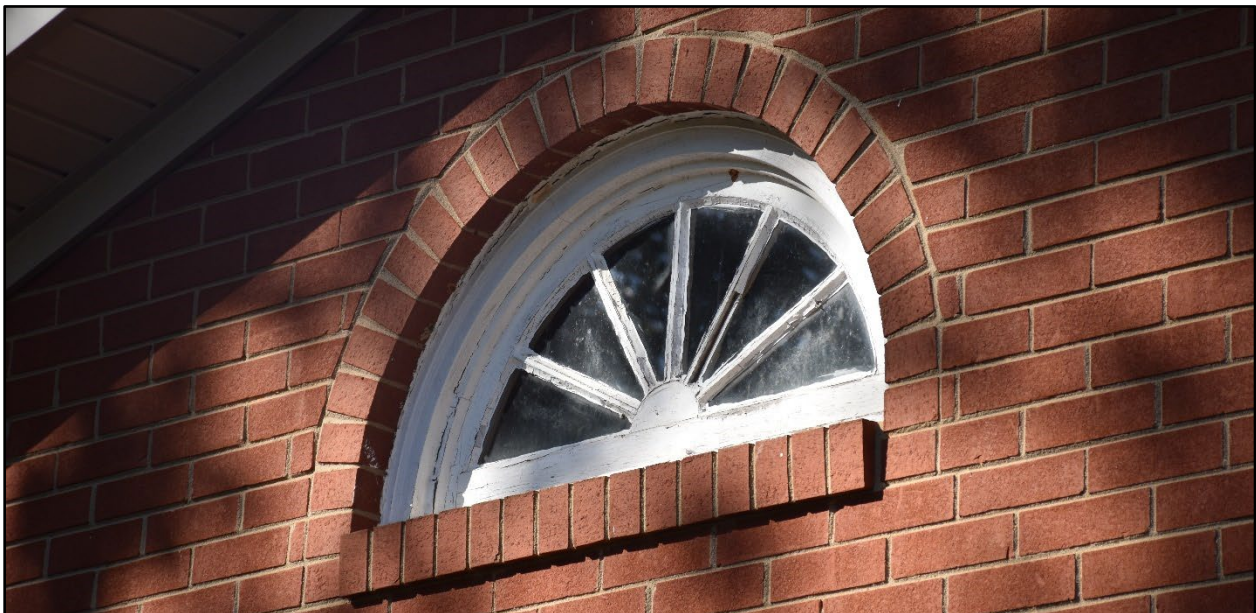
Figure 7- View of original semicircular gable-end window on the 1964 sanctuary/educational building.
