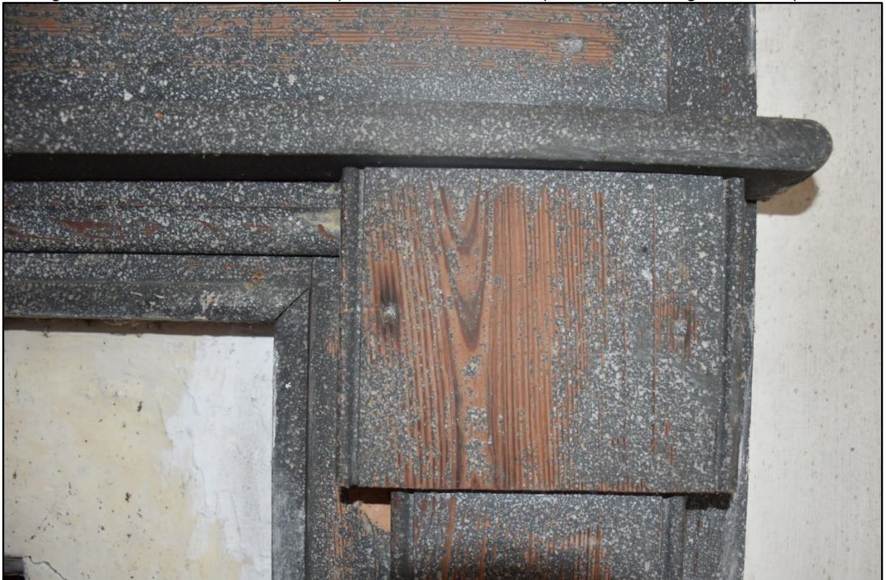
Figures 162 and 163- Details of the upstairs east room mantel profile and eroding faux-stone paint.
