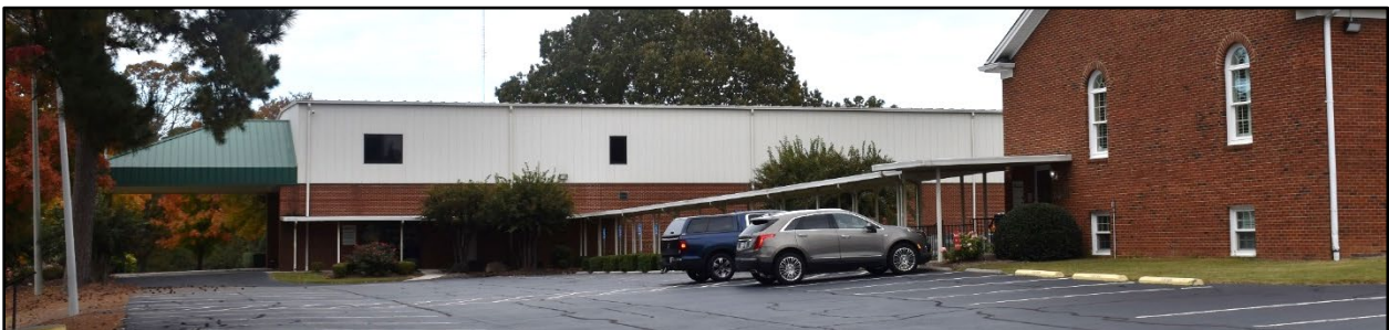
Figure 88- View of the modern gymnasium building behind the sanctuary at Catawba Springs Church.
