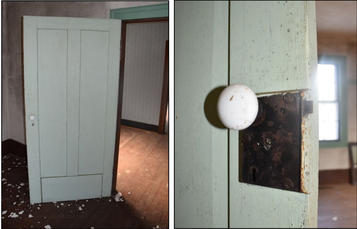
Figures 159 (left) and 160- Two-panel door into the upstairs east room, with historic doorknob.
