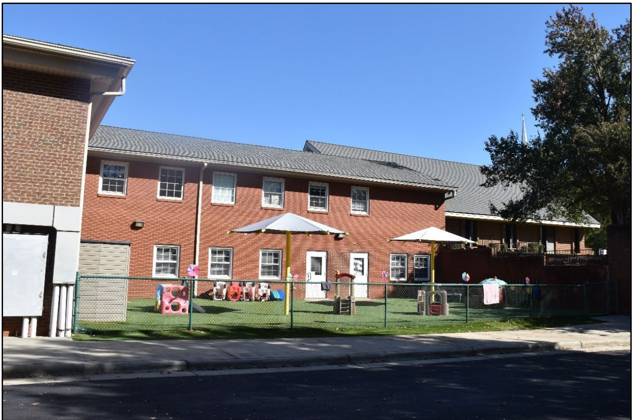
Figure 22- View of both stories on the south side of the 1964 sanctuary/education building, facing northeast.
