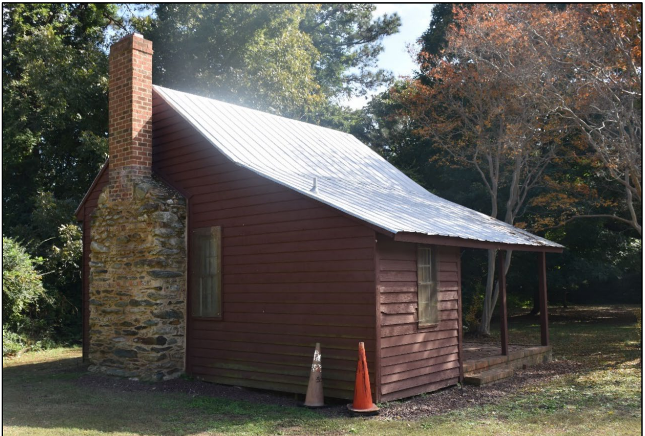
Figure 170- Oblique view facing southeast of the north and west elevations of the kitchen/schoolhouse.
