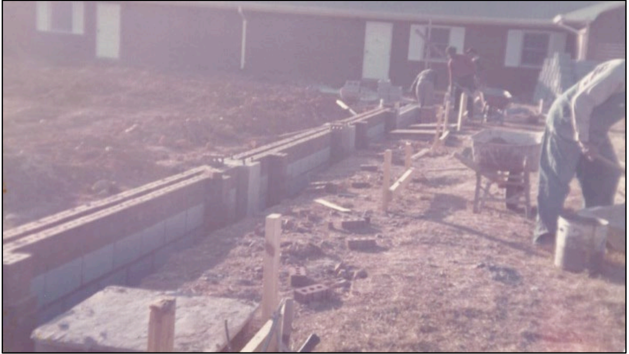
Figure 8- View of foundation construction of 1974 sanctuary, facing west (Source: Macedonia Baptist Church archives).
