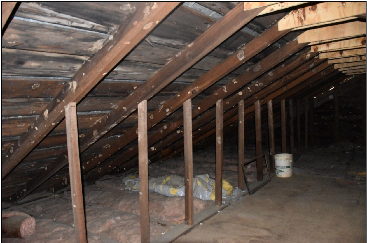
Figure 166- View inside the attic of the one-story ell, facing northwest.
