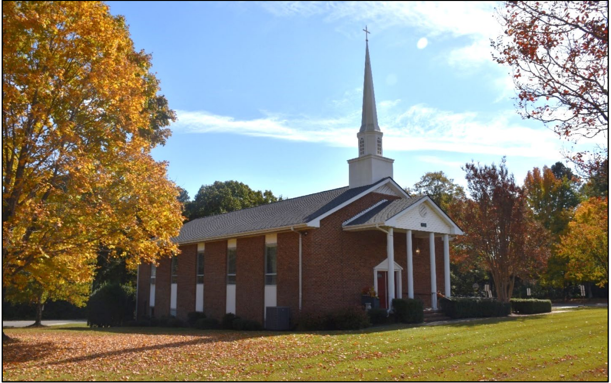
Figure 80- Oblique view of Reedy Creek Baptist Church in Cary, looking towards the southeast.
