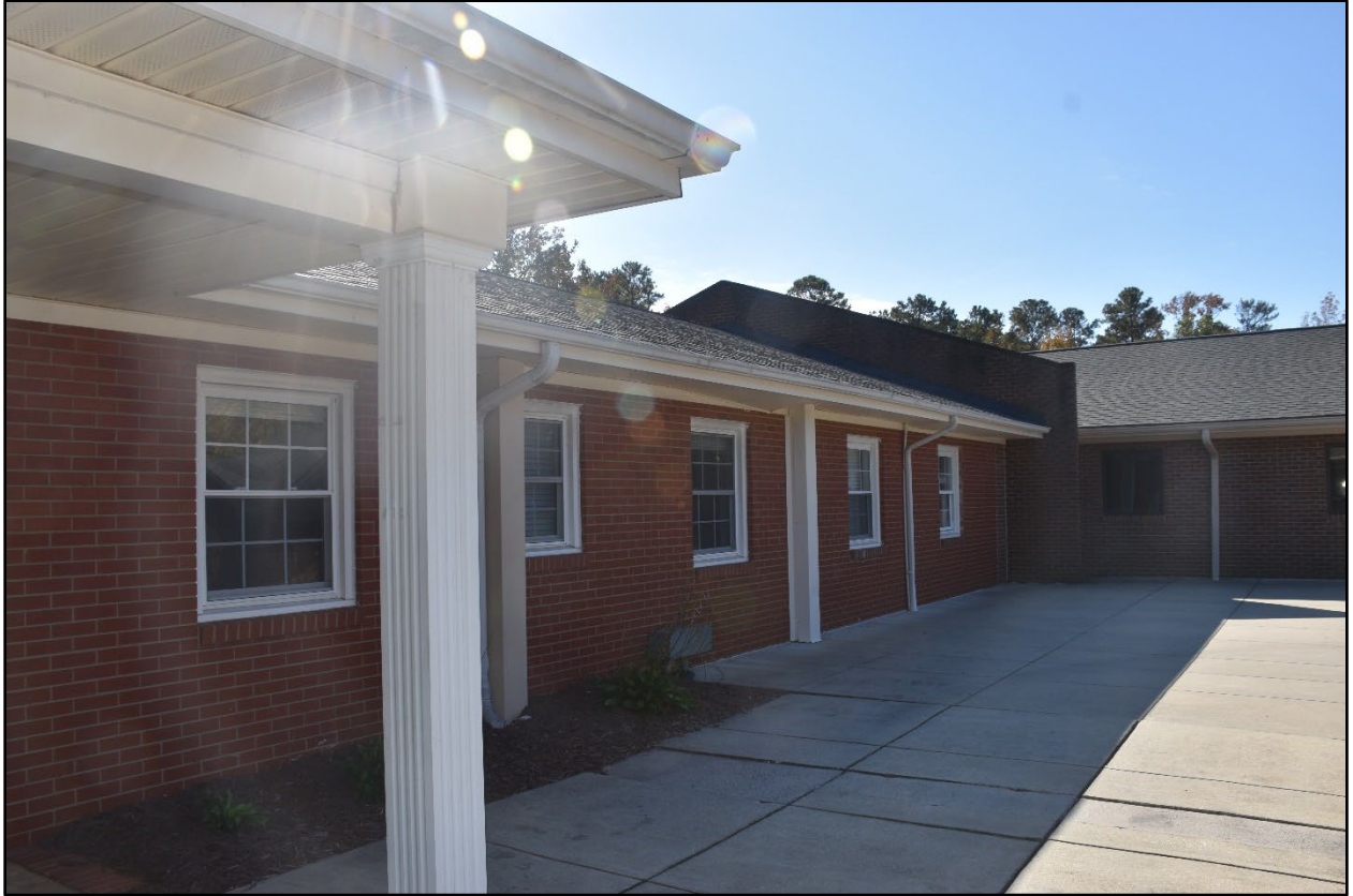
Figure 19- View of the rear elevation of the ell connecting the two educational wings, facing south.
