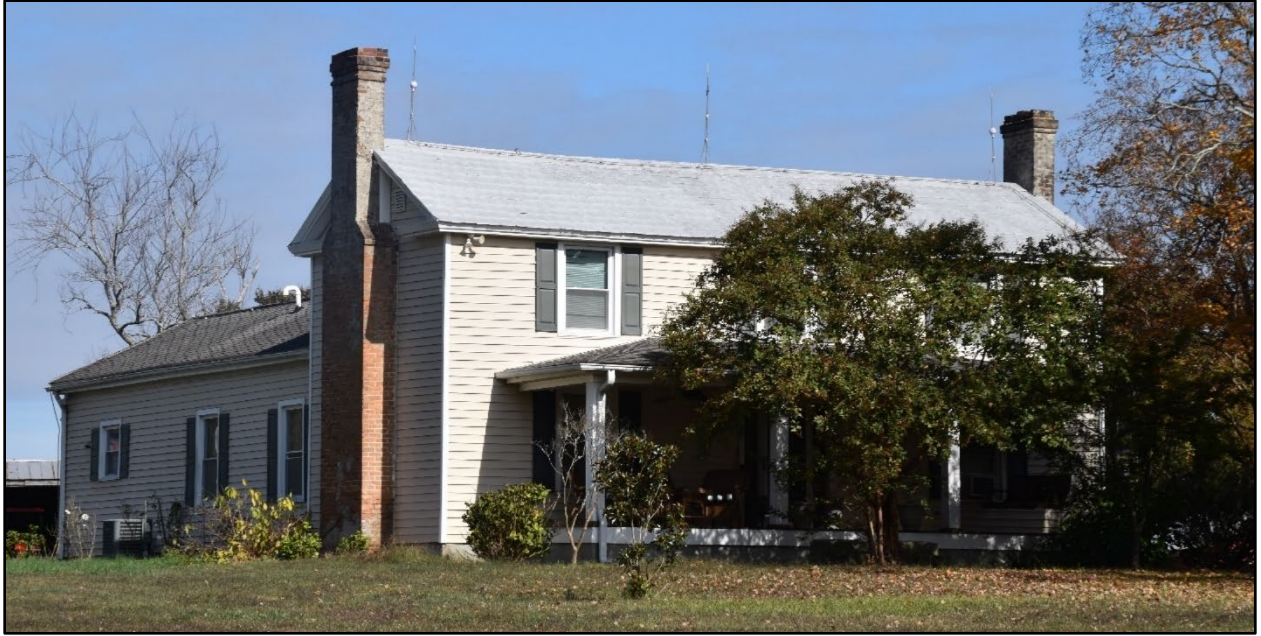
Figure 228- The farmhouse of the Horton-Upchurch Farm (WA0764) in Cary, similar in layout to the Barnabas Jones House and similarly clad in replacement siding; view looking north.
