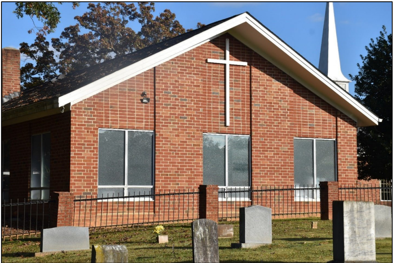
Figure 43- West elevation of the ell of the 1965 building; note stacked-bond spandrel designs above windows.
