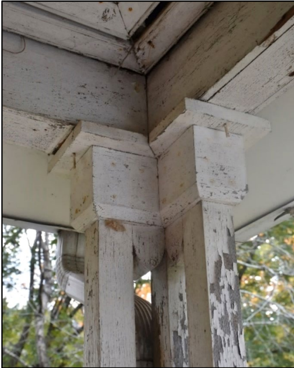
Figure 104 (left)- Design of the wood capitals on the front porch columns.
