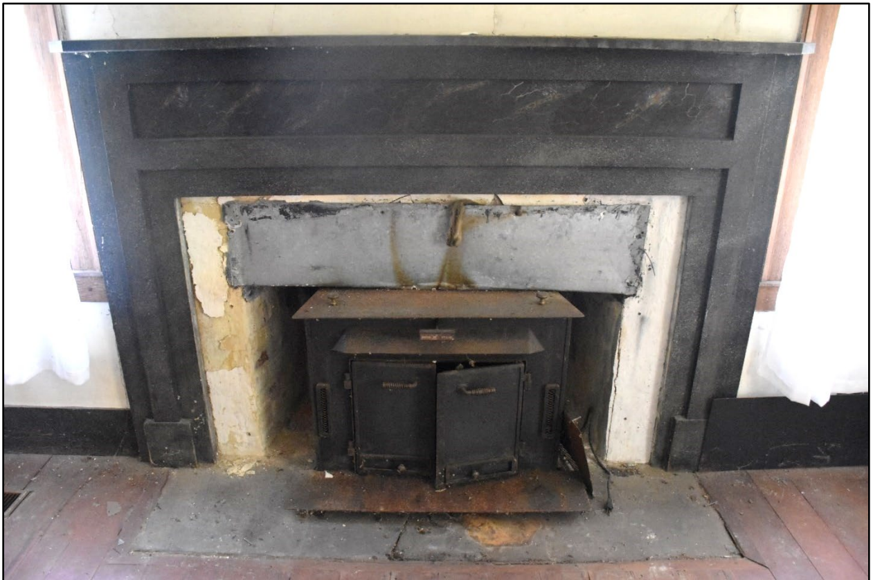
Figure 149- View of the fireplace and mantel in the downstairs east room.
