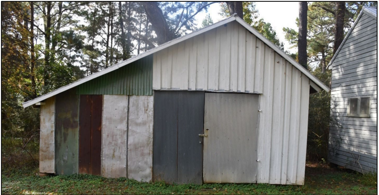
Figure 202- The east elevation of the cider barn/shed, with an amalgamation of wood, corrugated metal, standing seam metal, and fiberglass siding present.
