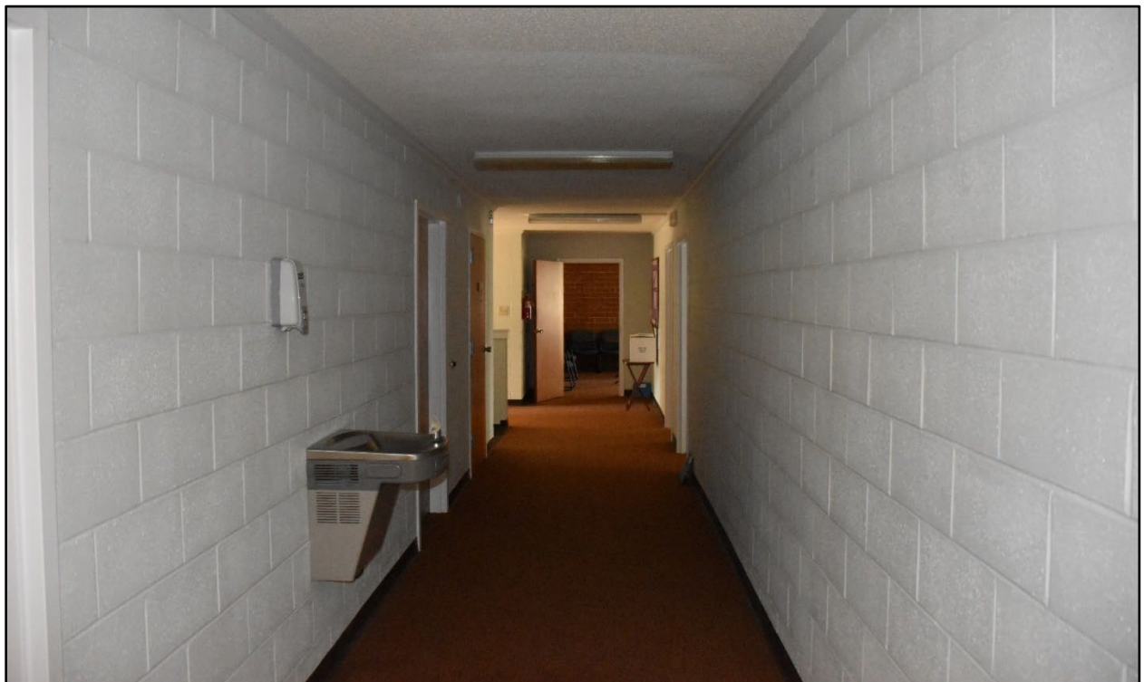
Figure 39- Rear hallway behind sanctuary, with concrete block walls and carpeted floor; view facing west.
