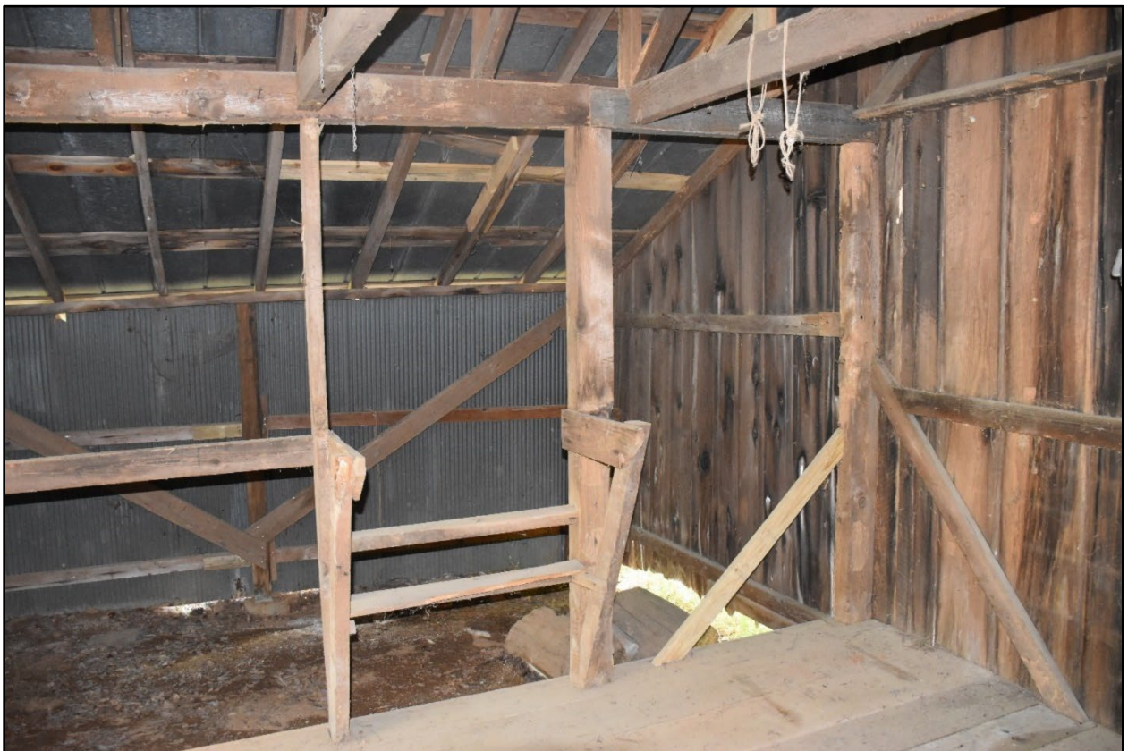
Figure 204- View towards the southwest of the cider barn/shed interior.
