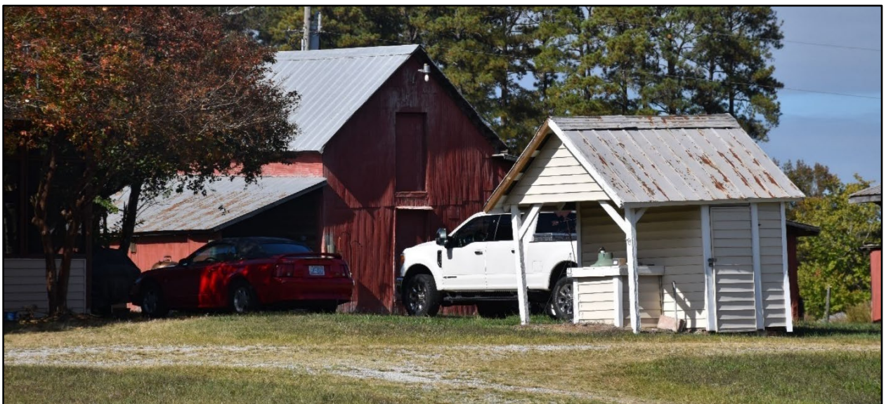
Figure 233- Vinyl-clad wellhouse (or other minor outbuilding) on the Horton-Upchurch Farm.
