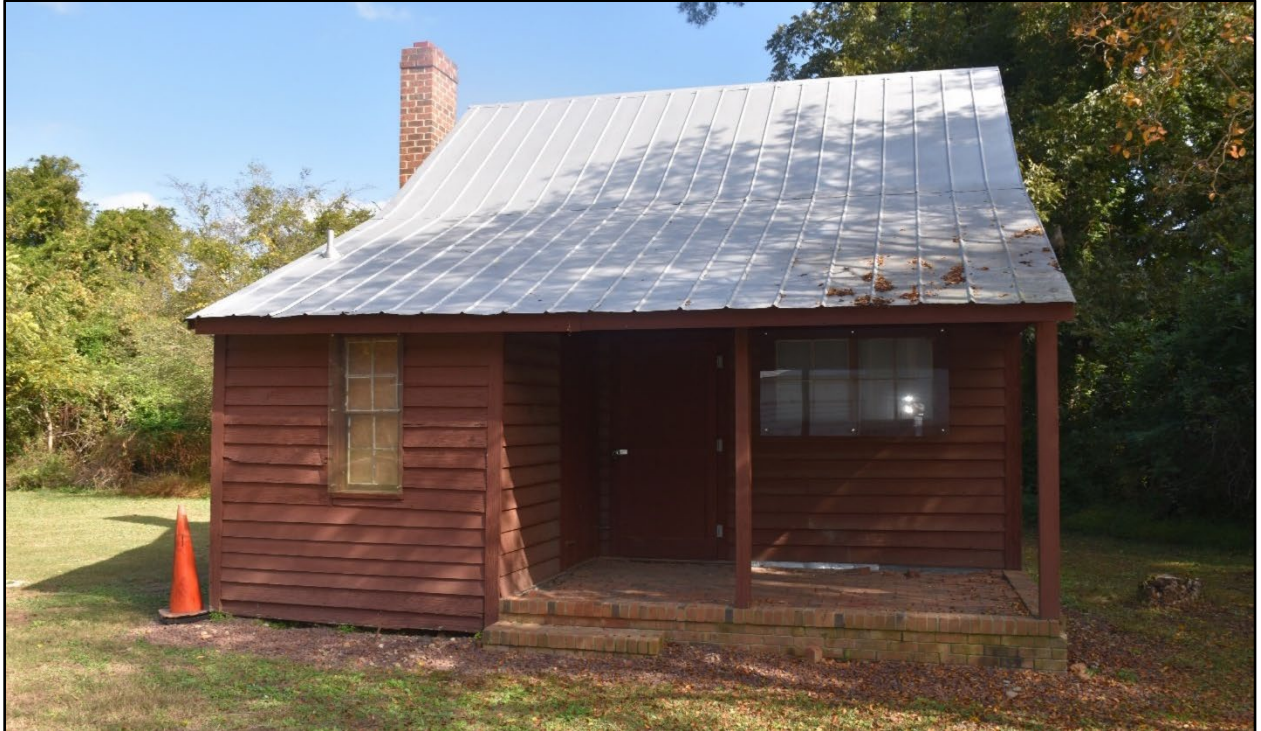
Figure 169- View of the west elevation of the kitchen/schoolhouse, facing east.
