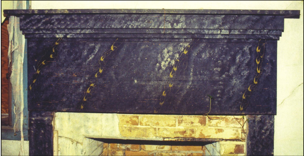
Figure 234- Mantel detail from the mid-nineteenth century James A. Johnson House in Harnett County, NC. (Source: Phillips, Grand Illusions). Note the similarity of the amoeba-like designs above and below to the Barnabas Jones House mantle inset panel on the following page.
