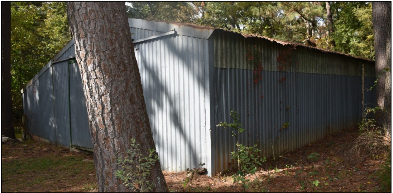
Figure 210- Oblique of the livestock barn from the southeast corner.
