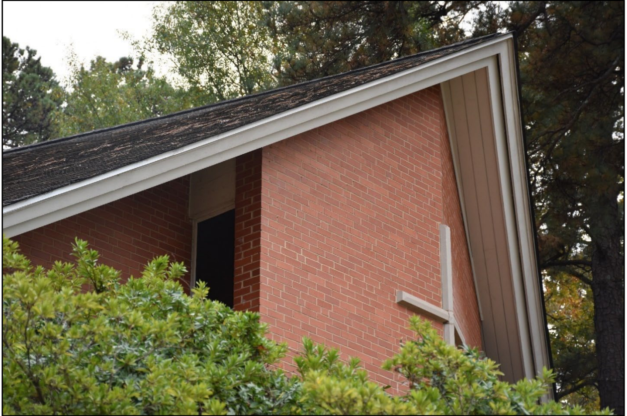
Figure 21- Beveled sanctuary walls on the Community United Church of Christ (WA7996) in Raleigh.
