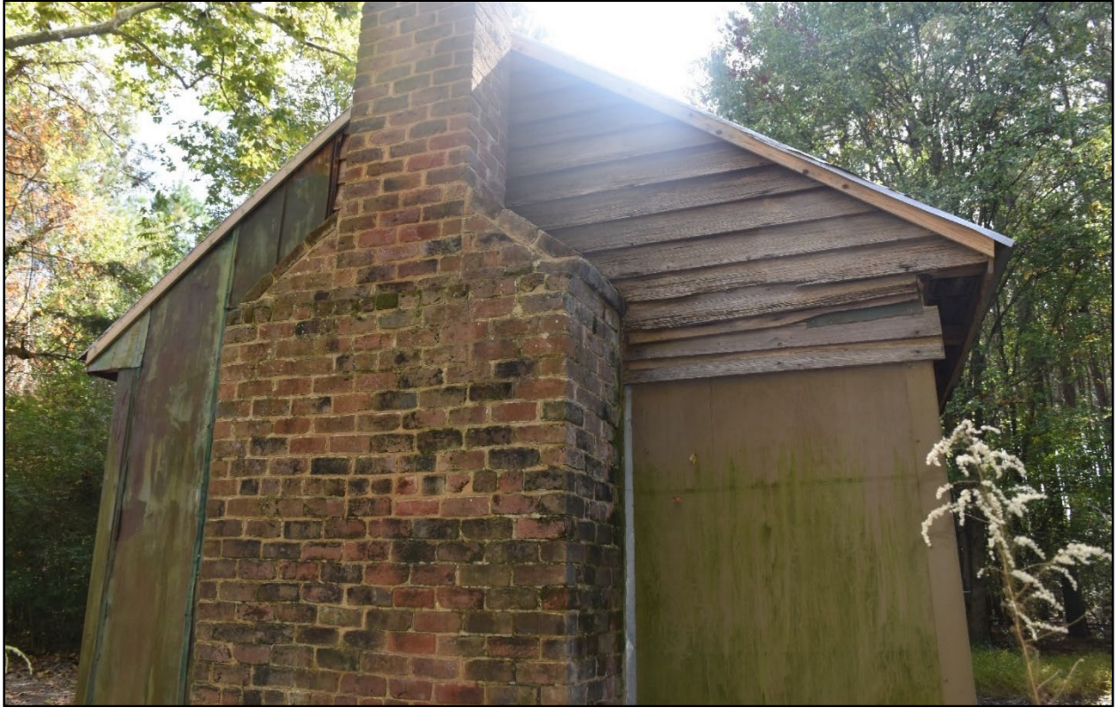
Figure 188- View of the chimney and siding on the north elevation of the slave quarters.
