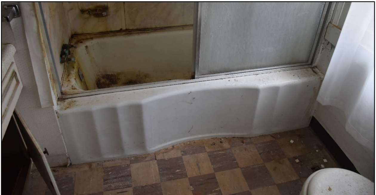
Figure 131- Facing north, the bathroom floor and bathtub.
