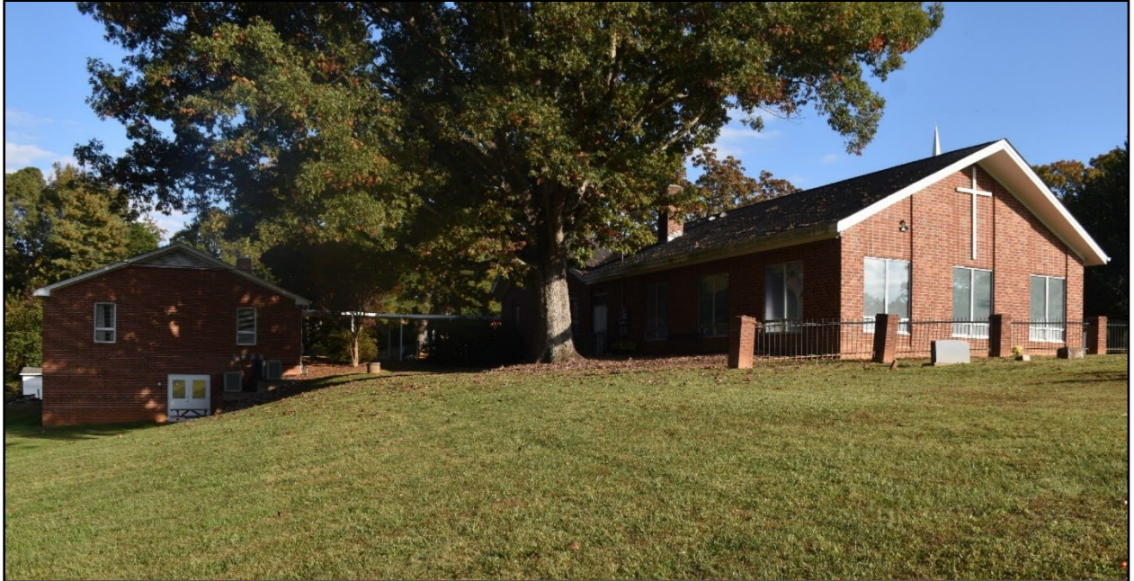
Figure 44- The 1979 educational building and fellowship hall (left) and the ell of the 1965 building (right).
