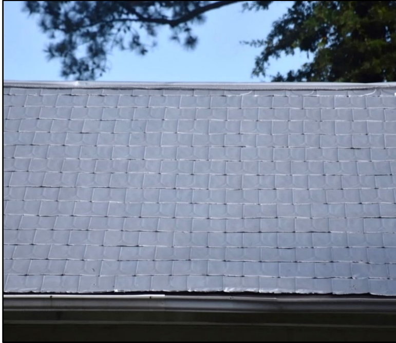
Figure 113 (left)- Detail of the historic metal shingles on the two-story section of the farmhouse.
