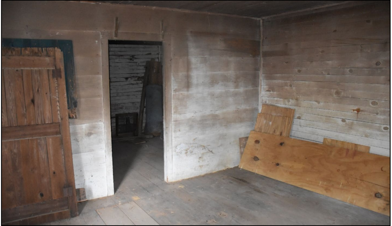
Figure 193- View looking southwest from the north room of the purported slave quarters/Reuben Jones House, with intact wood floors and walls visible.
