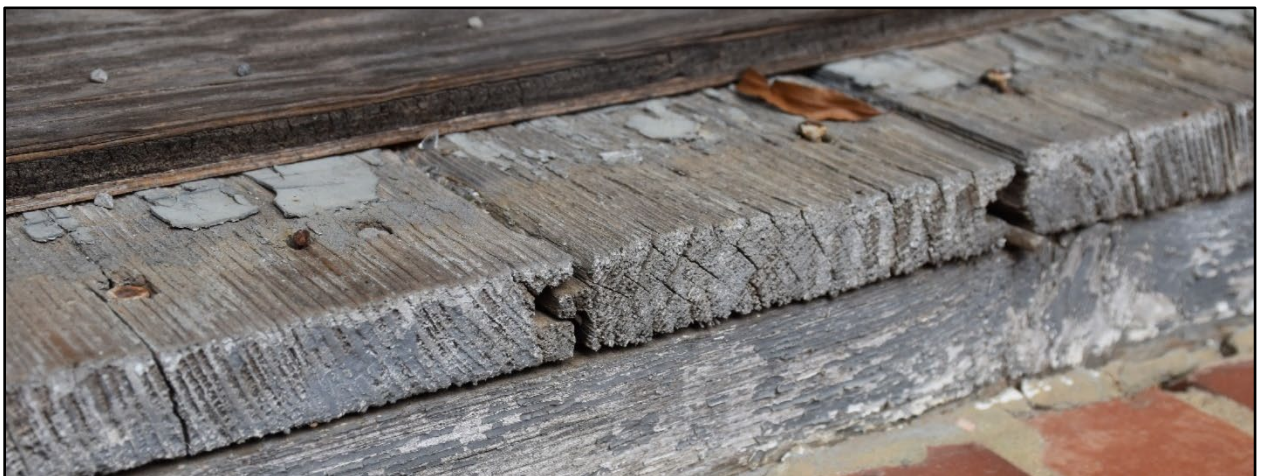
Figure 106- Historic tongue-and-groove decking on the front porch, with modern plywood above.
