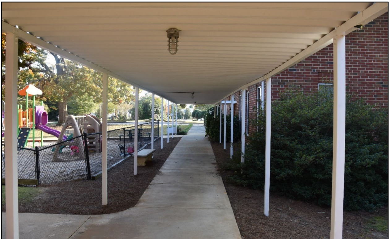
Figure 53- Corrugated metal covered walkway connecting the educational building to the sanctuary, facing south.
