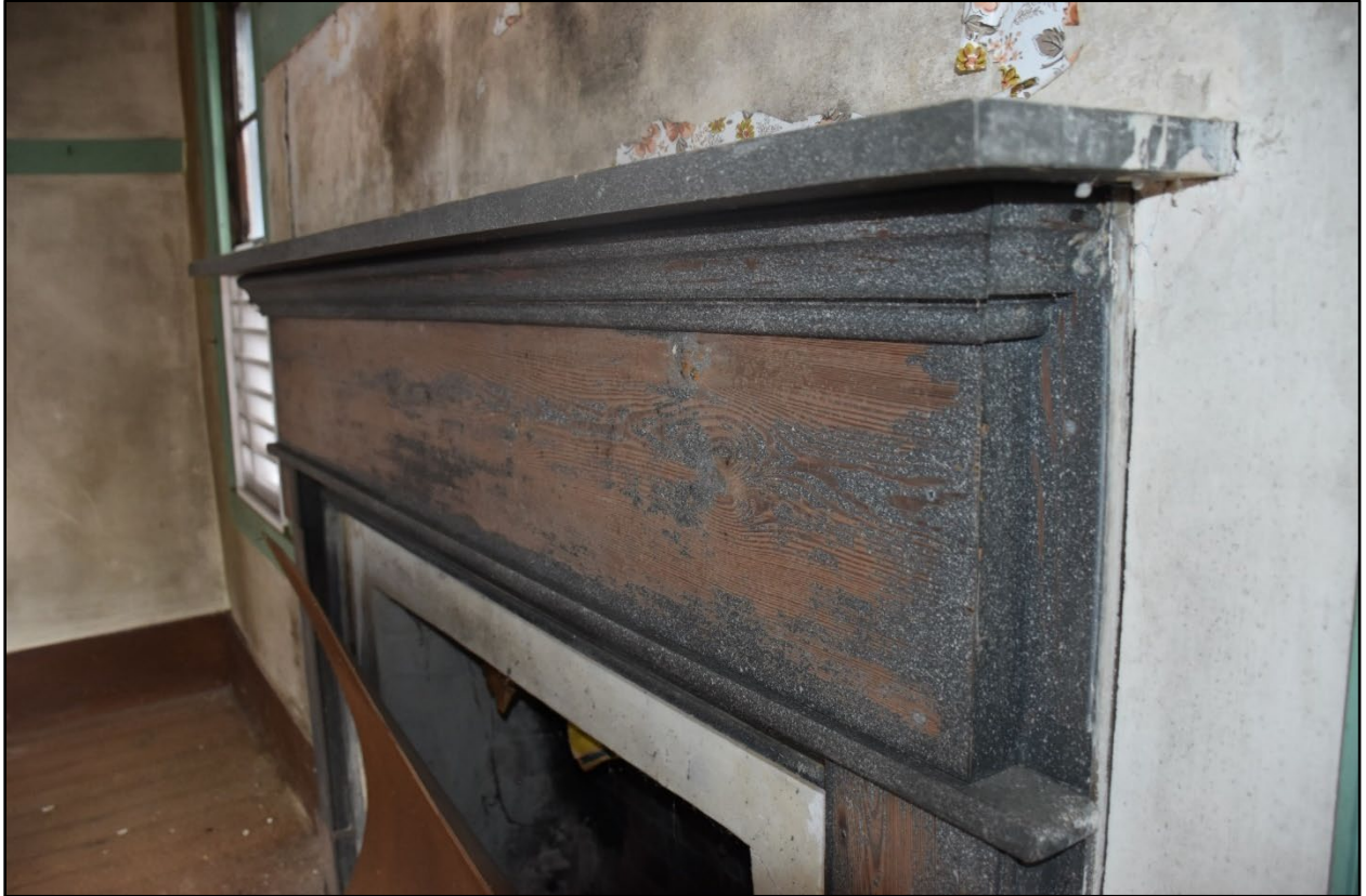
Figures 162 and 163- Details of the upstairs east room mantel profile and eroding faux-stone paint.
