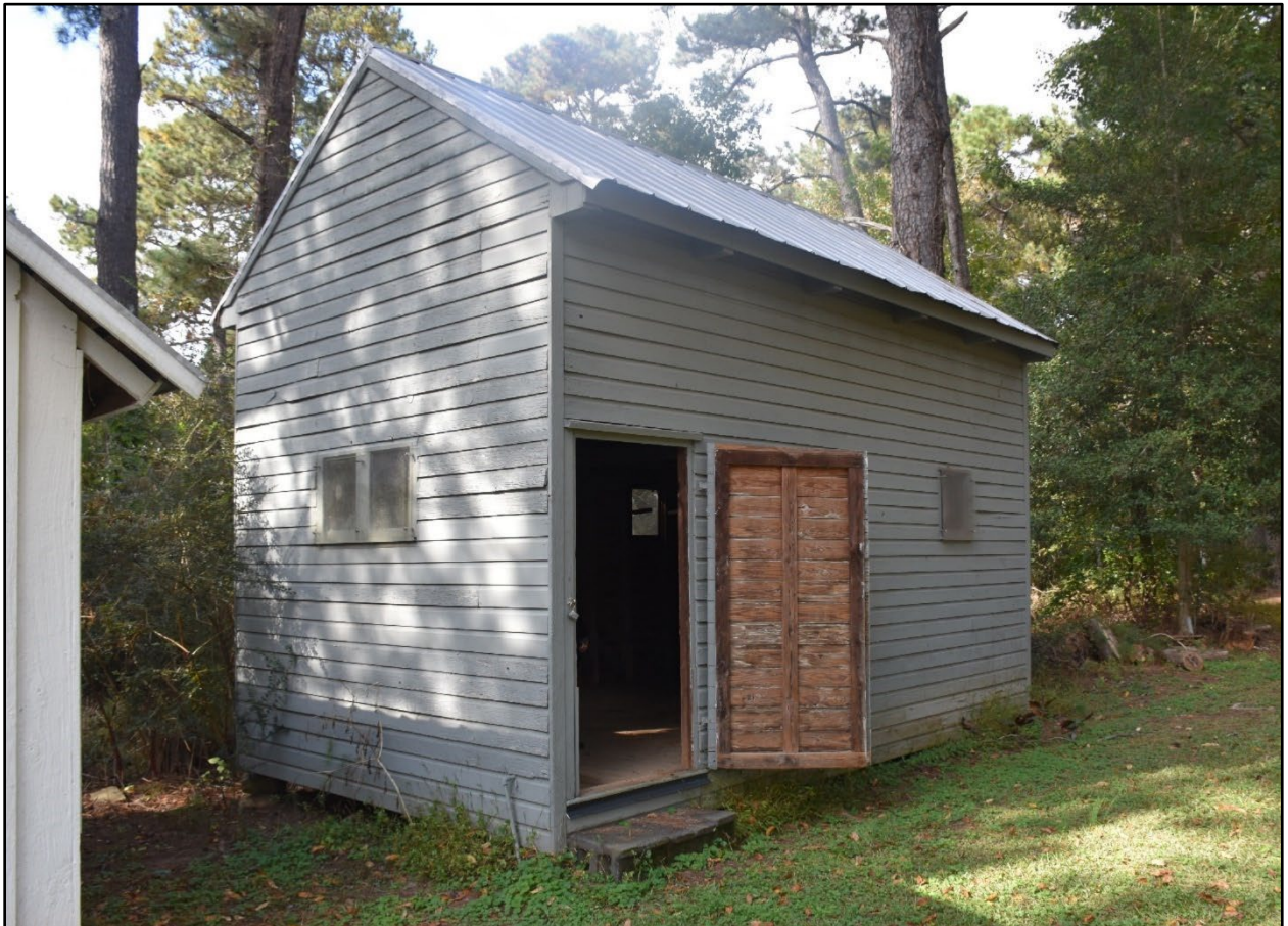
Figure 206- Oblique view of the grain barn from the southeast, showing wood siding and minimal windows.
