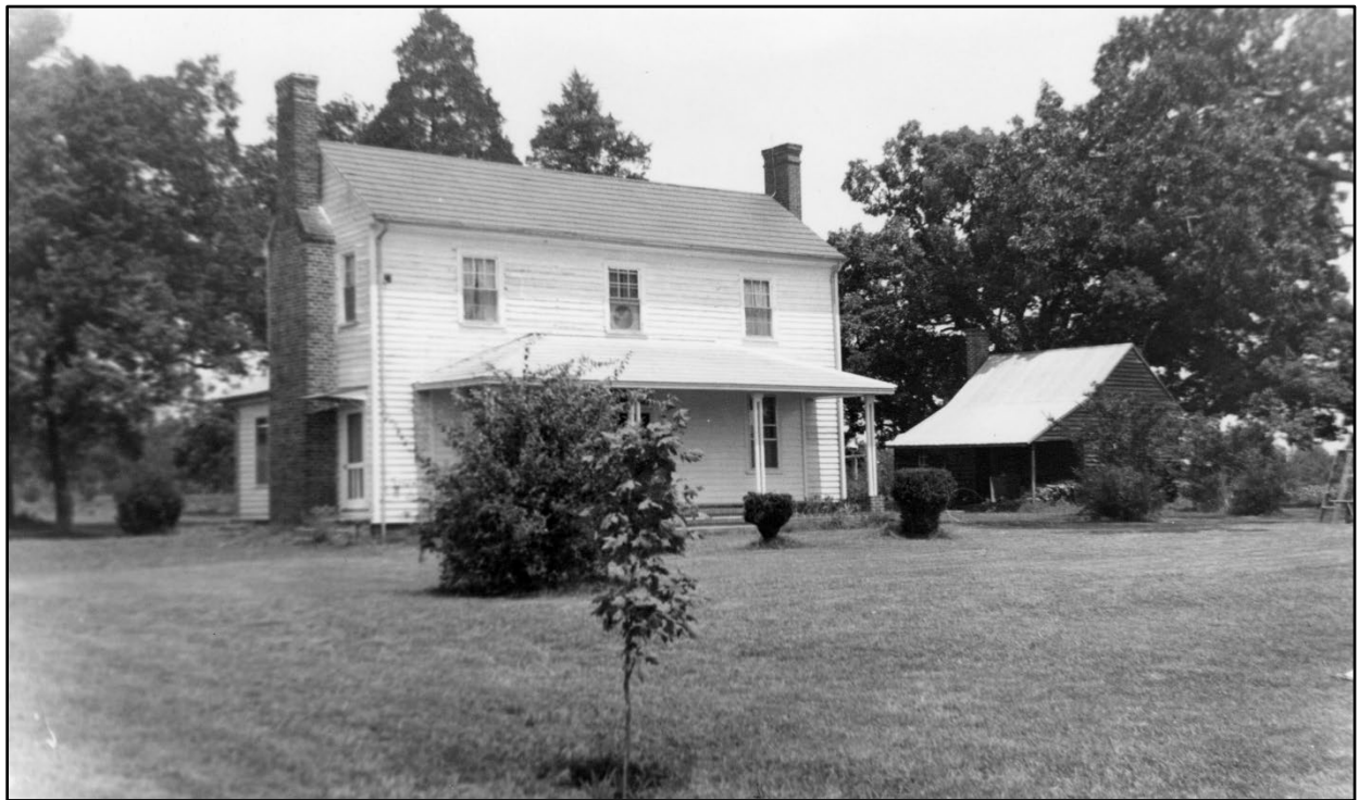
Figure 219- Circa 1961 photograph of the main house (left) and kitchen/schoolhouse, viewed from the southwest (Source: Knott, HABS, NCSU).
