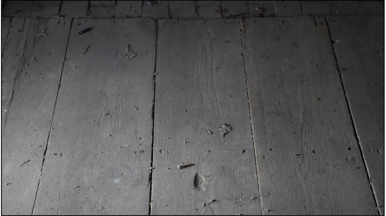
Figure 182- Detail of the historic wood floors in the kitchen/schoolhouse.
