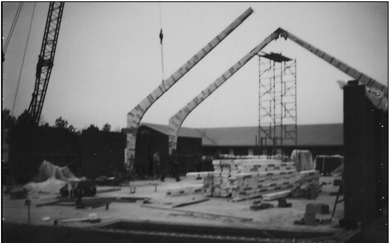
Figure 9- Assembly of the trusses for the 1974 sanctuary, facing west (Source: Macedonia Baptist Church archives).
