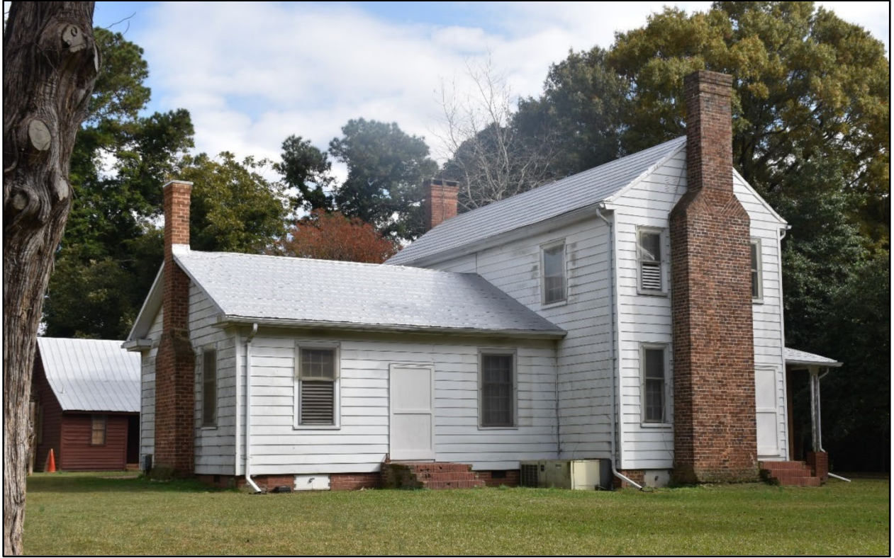
Figure 111- Looking southeast at the convergence of the two-story and one-story sections of the house.
