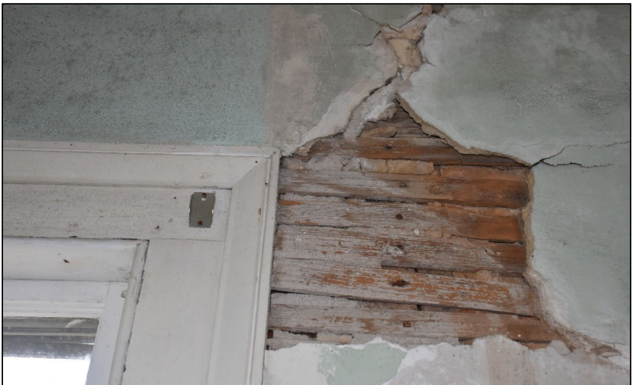
Figure 158- Detail of lath and plaster construction in the upstairs west room.
