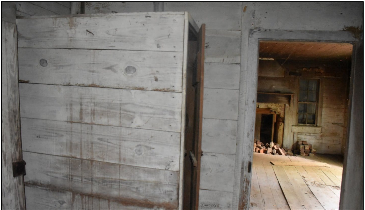
Figure 192- View looking north in the south room, featuring a historic wood closet; note the historic wood-panel walls and the historic wood floors visible at right in the north room.
