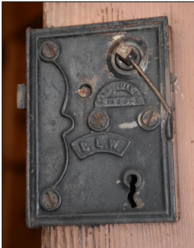
Figure 142 (left)- Distinctive hardware on the storage room door, marked "B.L.W. [Branford Lock Works of Branford, Connecticut], Pat'd [Patented] July 21, 1863." Figure 143 (right)- View of the door between the west room and the hallway.
