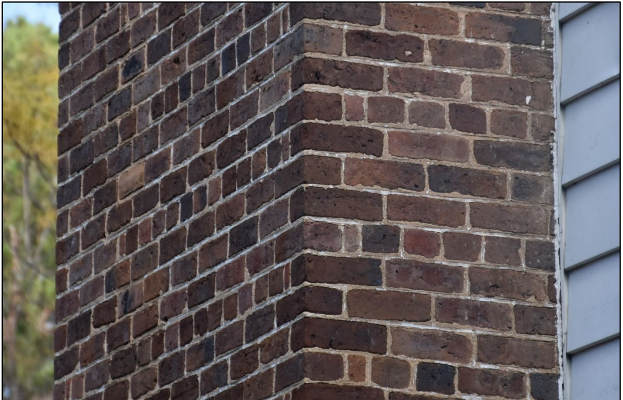
Figure 112- Detail view of the nineteenth-century bricks on the west side chimney.
