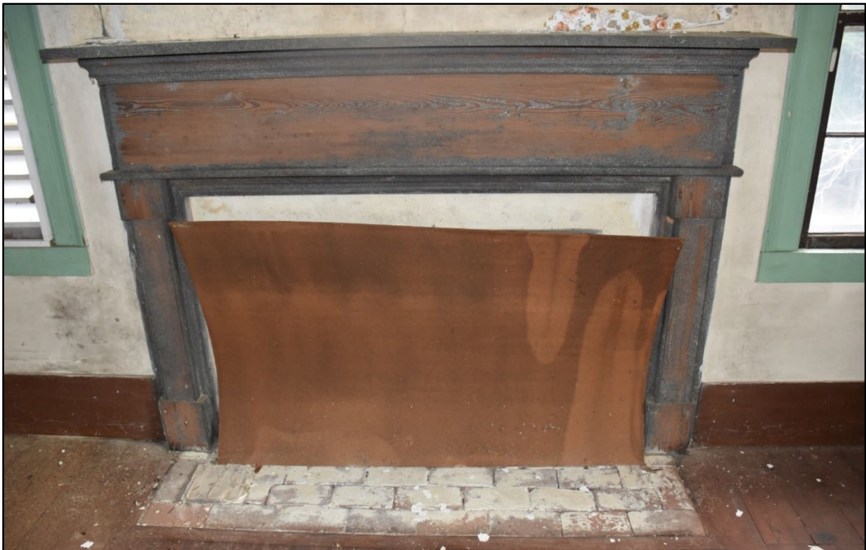
Figure 161- View of the painted wood mantel in the upstairs east room, located on the east wall.
