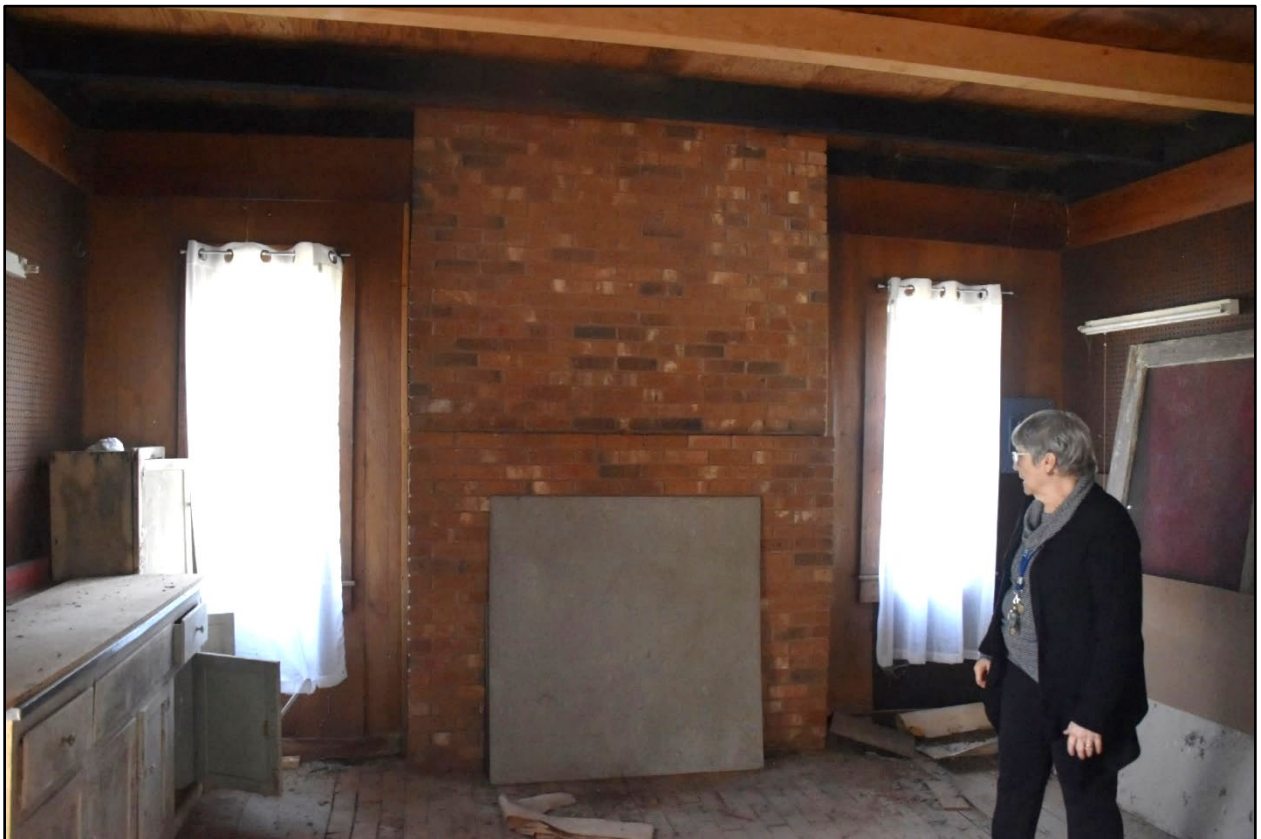
Figure 181- The north wall of the kitchen/schoolhouse, with non-historic brick veneer over the historic brick chimney.
