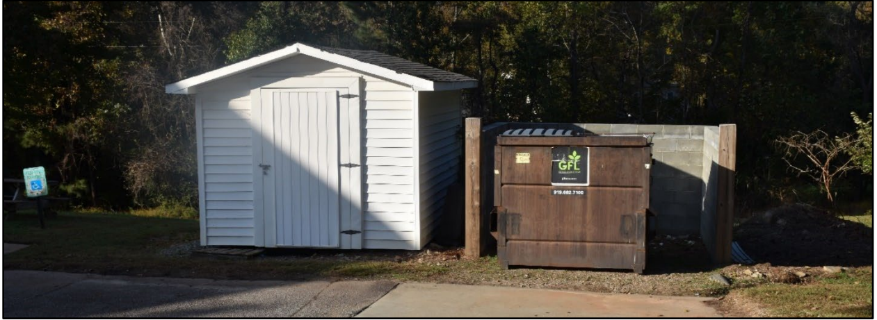
Figure 49- Non-historic portable storage building and dumpster enclosure northeast of the educational building.
