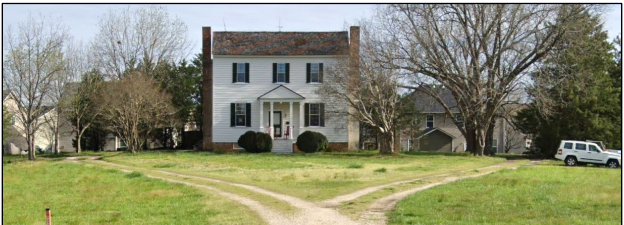
Figure 225- View of the Beaver Dam Farm house in April 2024; note the subdivision houses in the background (Source: Google Street View).
