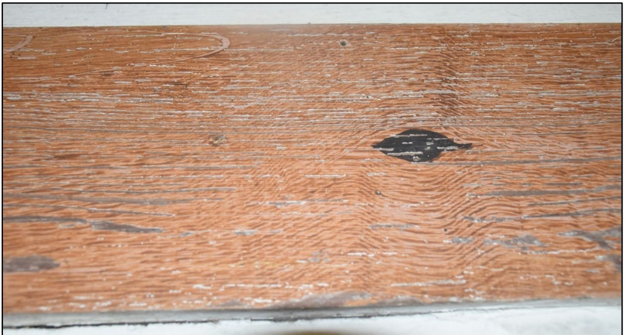
Figure 145- View of painted wood graining on the trim above the fireplace in the east room on the first floor.
