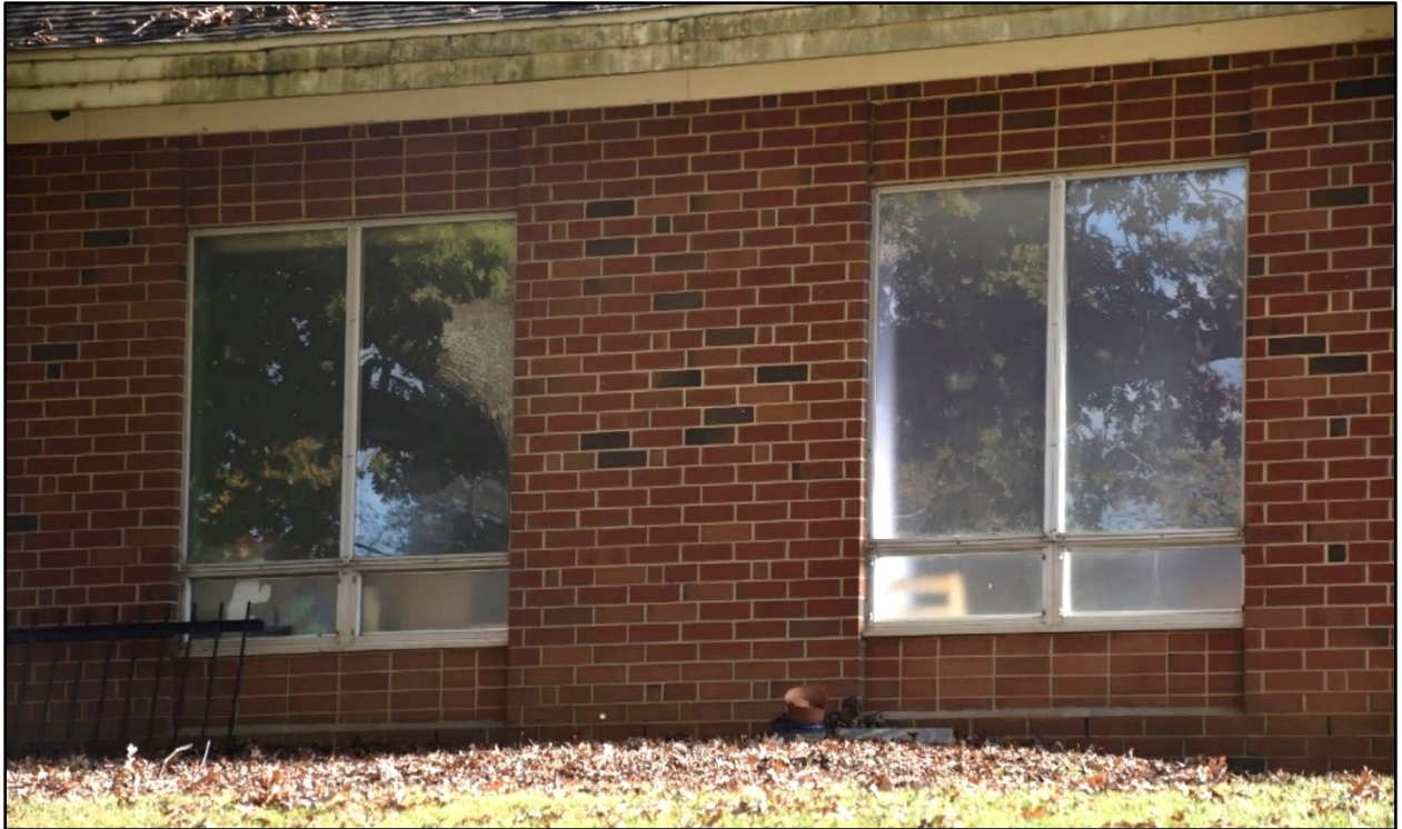
Figure 46- Detail of the windows on the north elevation of the 1965 building.
