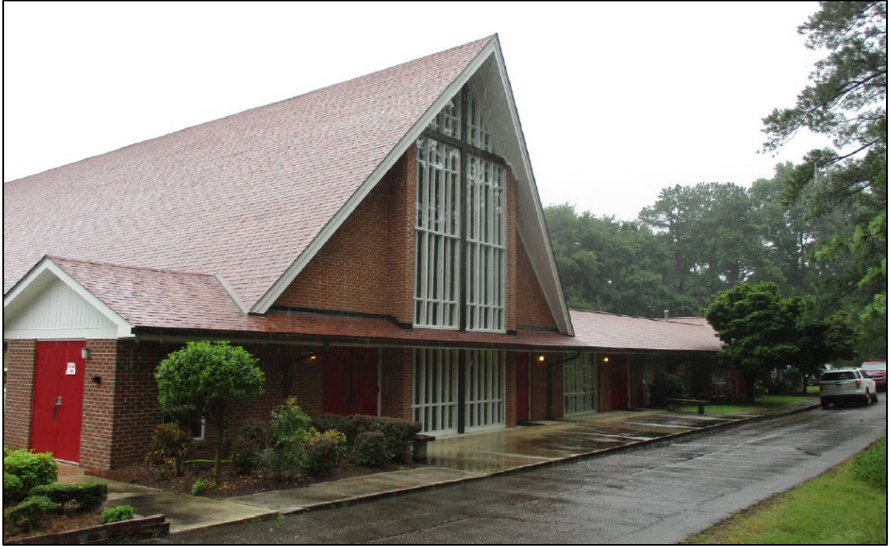
Figure 23- Front elevation of the NRHP-listed St. Ambrose Episcopal Church, WA8136, facing northeast, 2018 (Source: NRHP registration form).
