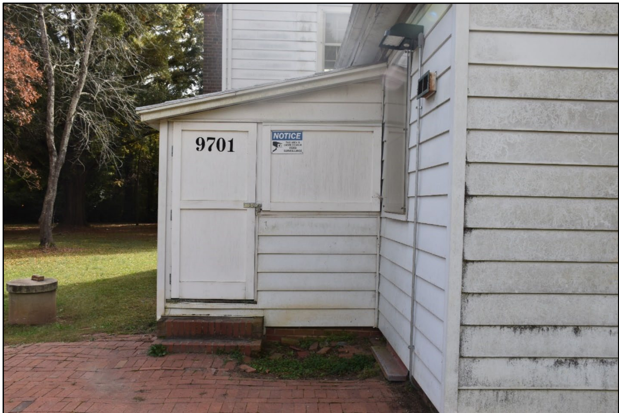
Figure 115- Looking south at the post-1961 shed-roofed addition on the rear of the house (see Figure 126 for view from the other direction).
