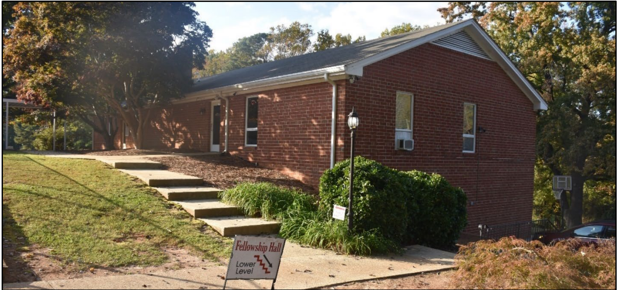
Figure 50- Southeast corner of the educational building.
