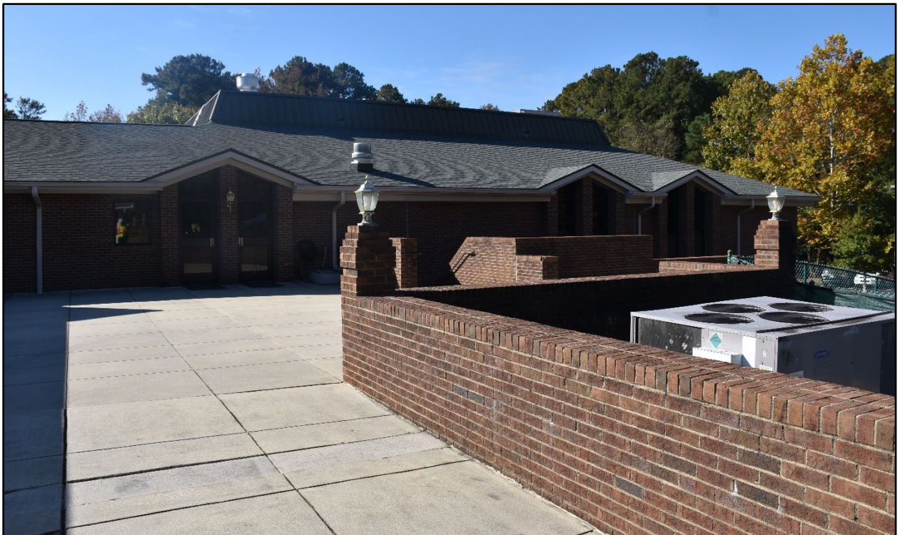
Figure 20- The circa 2000 daycare building, facing southwest.
