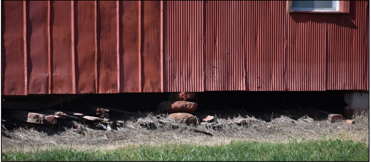
Figure 231- Detail of intact rock foundation stones on one of the Horton-Upchurch Farm barns.
