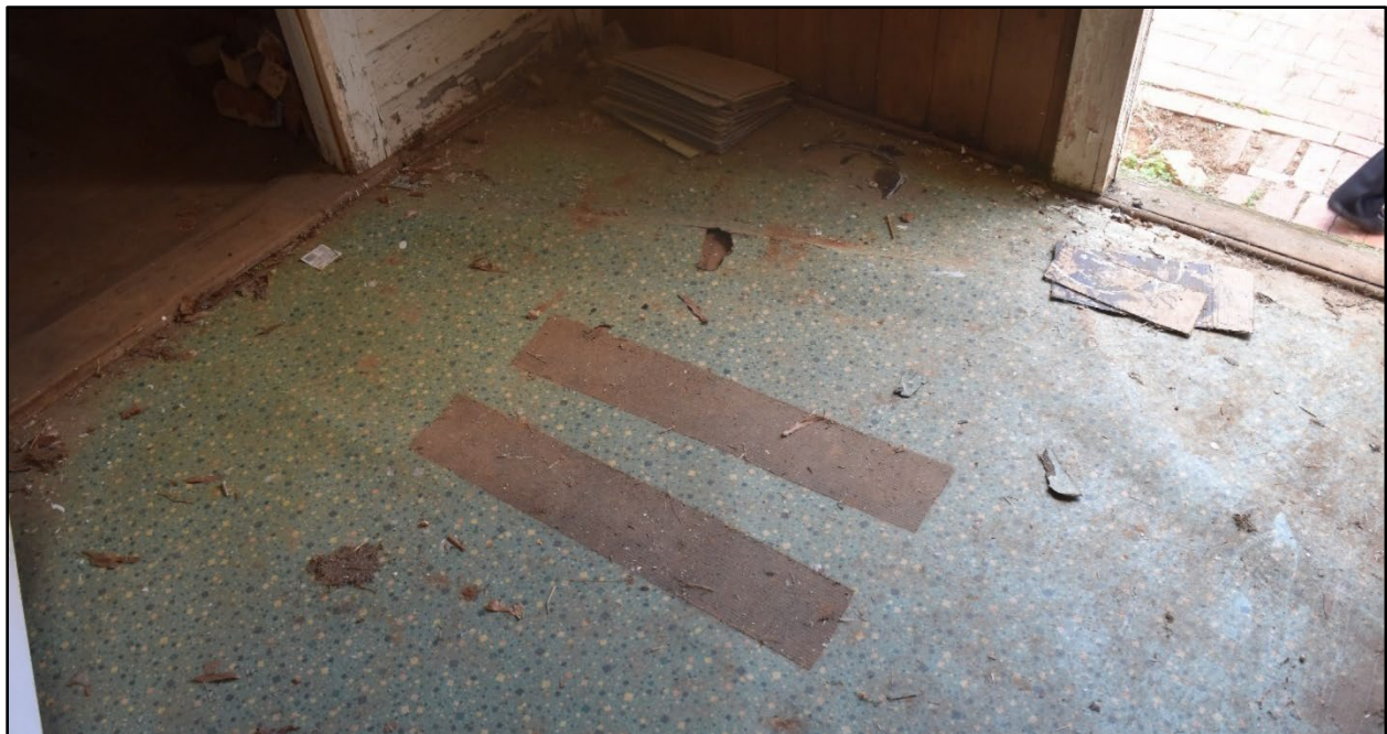
Figure 118- Flooring inside the shed-roofed entry addition.
