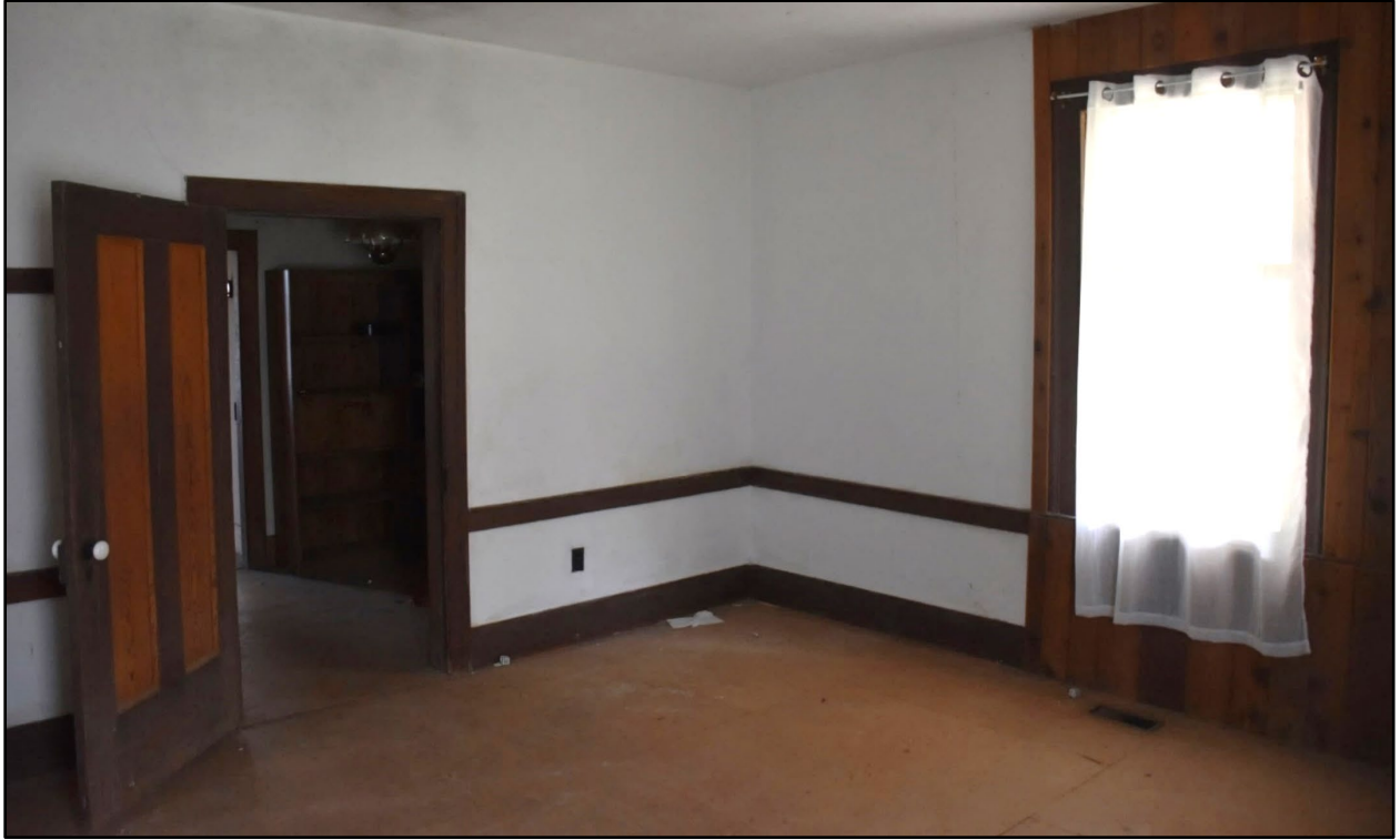
Figure 139- The west room on the first floor, facing southeast towards the hallway and entrance door.
