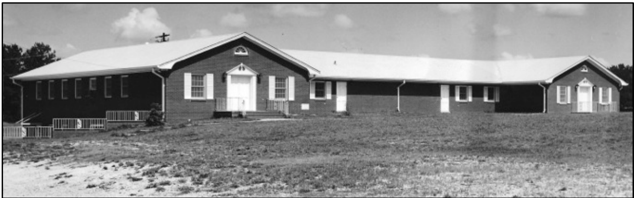
Figure 6- Circa 1969-1973 view, facing northwest, of the completed symmetrical complex before construction of the 1974 sanctuary (Source: Macedonia Baptist Church archives).
