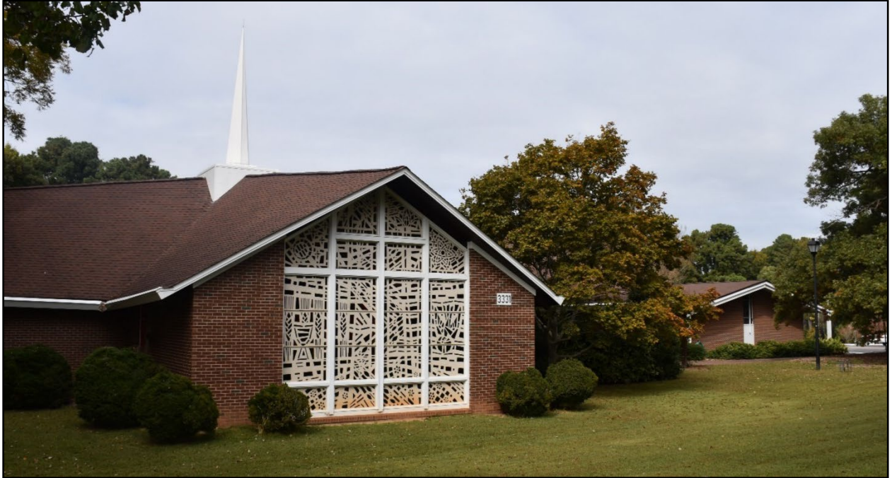
Figure 12- St. Paul's Christian Church (WA7971) sanctuary elevation facing Blue Ridge Road in Raleigh.
