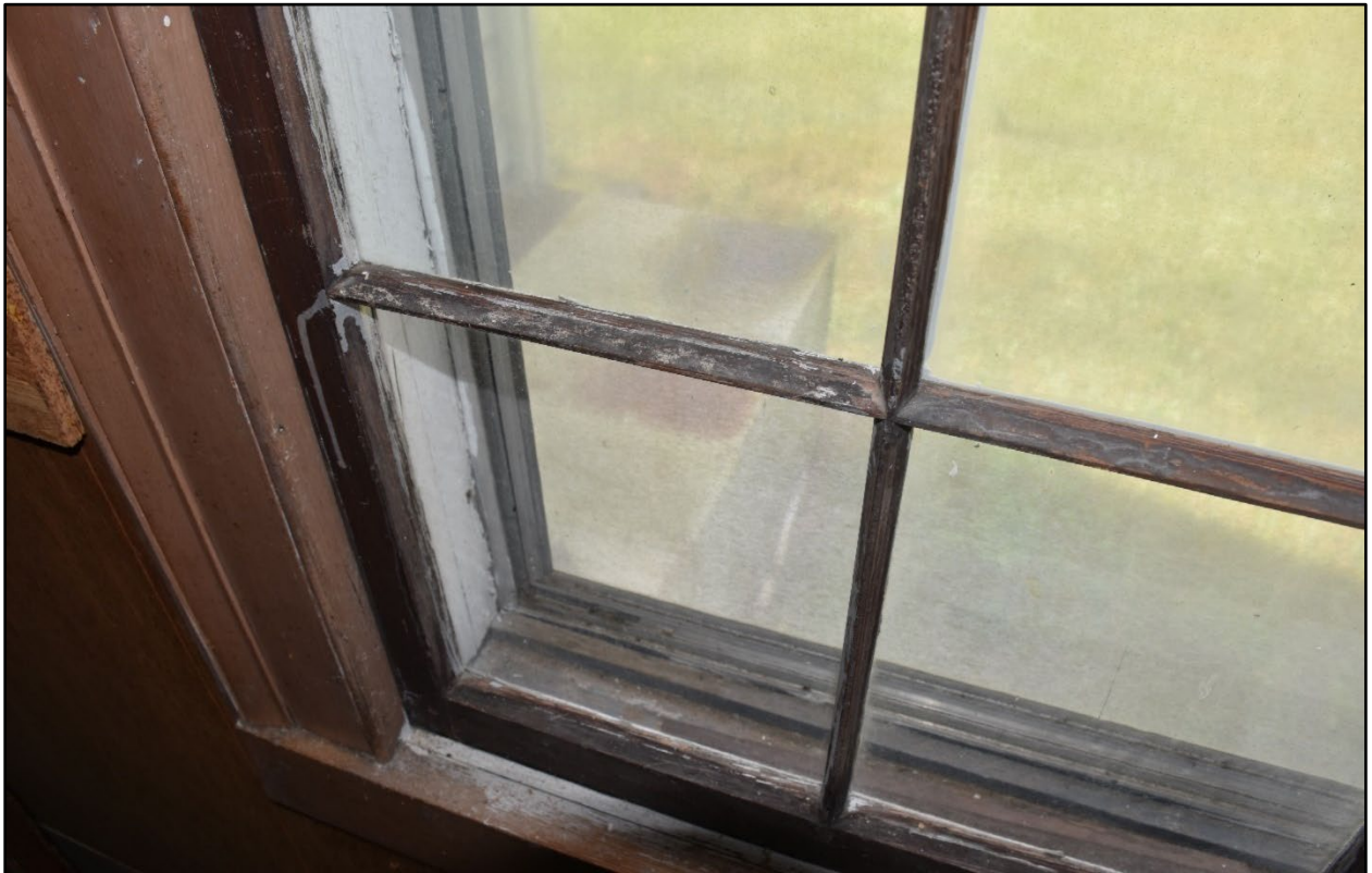
Figure 140- View of original wood-sash windows and modern storm windows in the west room.
