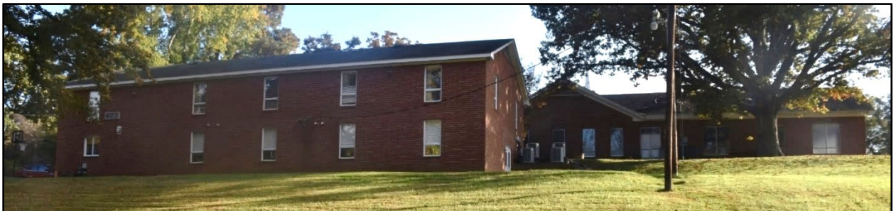
Figure 47- View of the north elevation of the educational building (left) and sanctuary/ell (right).
