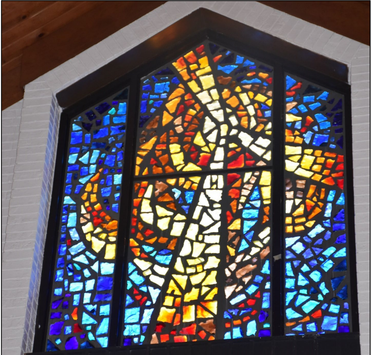
Figure 5- The stained glass window on the upper rear (west) elevation of the sanctuary, created using the dalle de verre technique.
