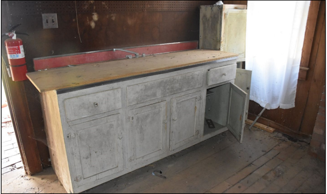
Figure 180- The lower west wall of the kitchen/schoolhouse, with non-historic cabinetry.
