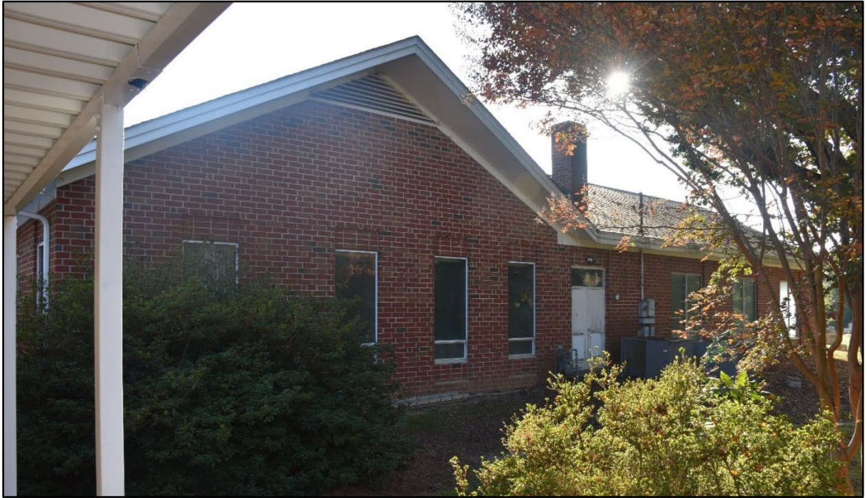
Figure 52- View of the north elevation of the 1965 building, facing southwest.
