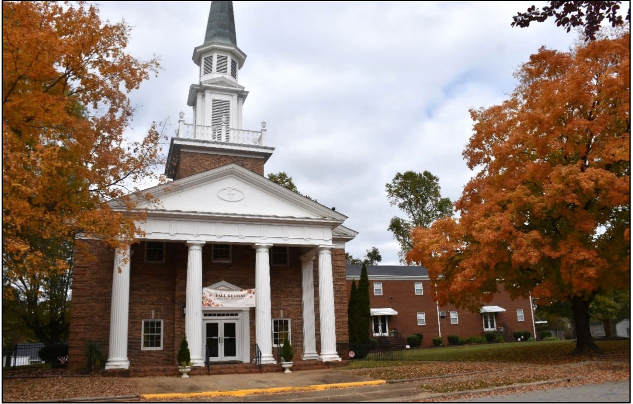
Figure 89- Front (south) elevation of Christian Faith Baptist Church, Raleigh, with side wing behind.
