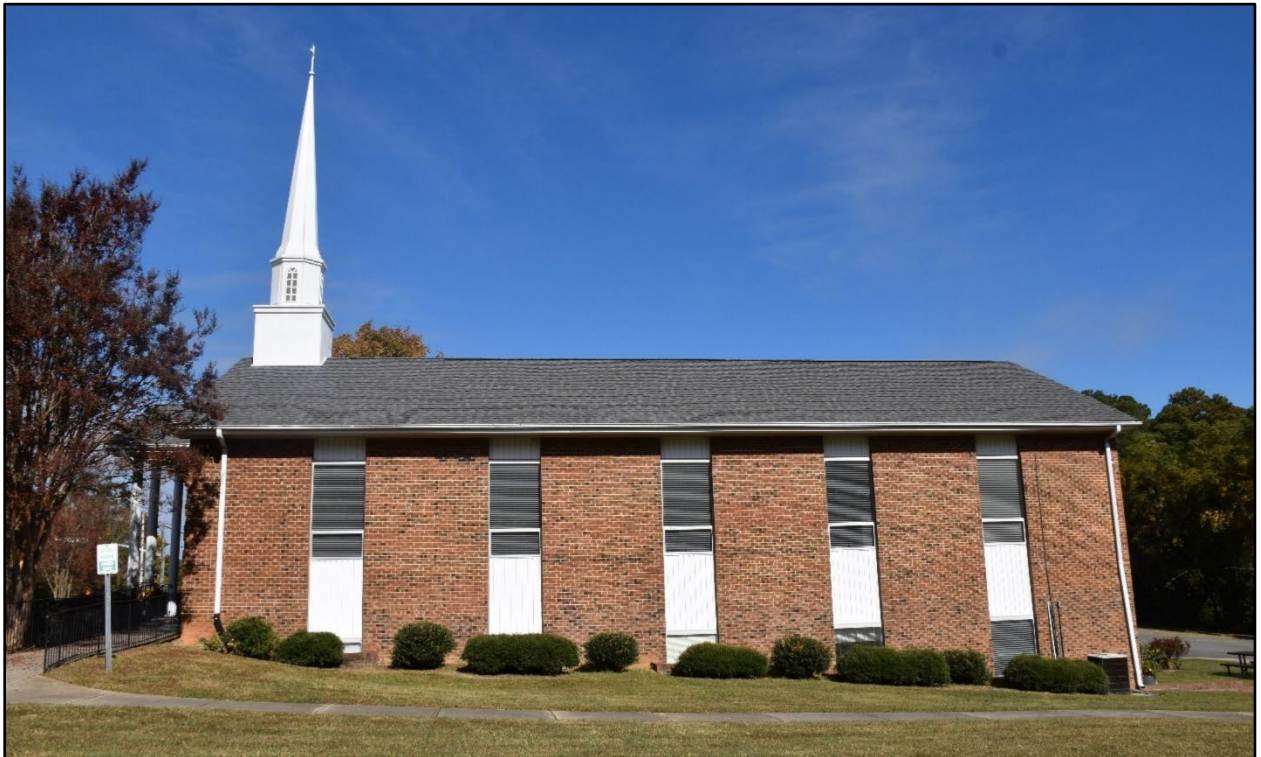
Figure 81- Side/south elevation of Reedy Creek Baptist Church, illustrating the 1960s combo of colonial revival steeple and International-style emphasized spandrel panels that Swift Creek Baptist Church shares.
