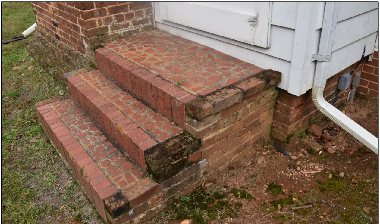
Figure 108- Mid-to-late twentieth century addition of a tile-shard treading surface on brick side entry steps.
