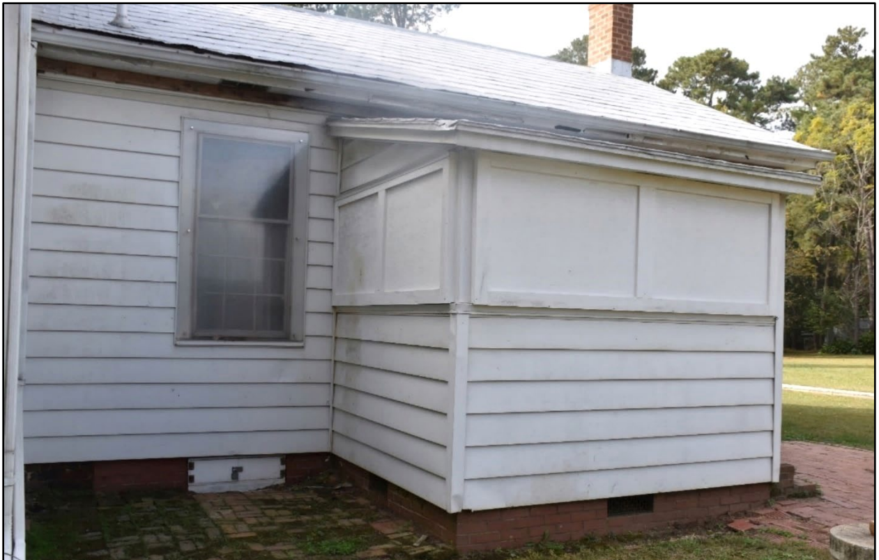
Figure 99- Detail of the post-1961 rear addition on the east elevation.
