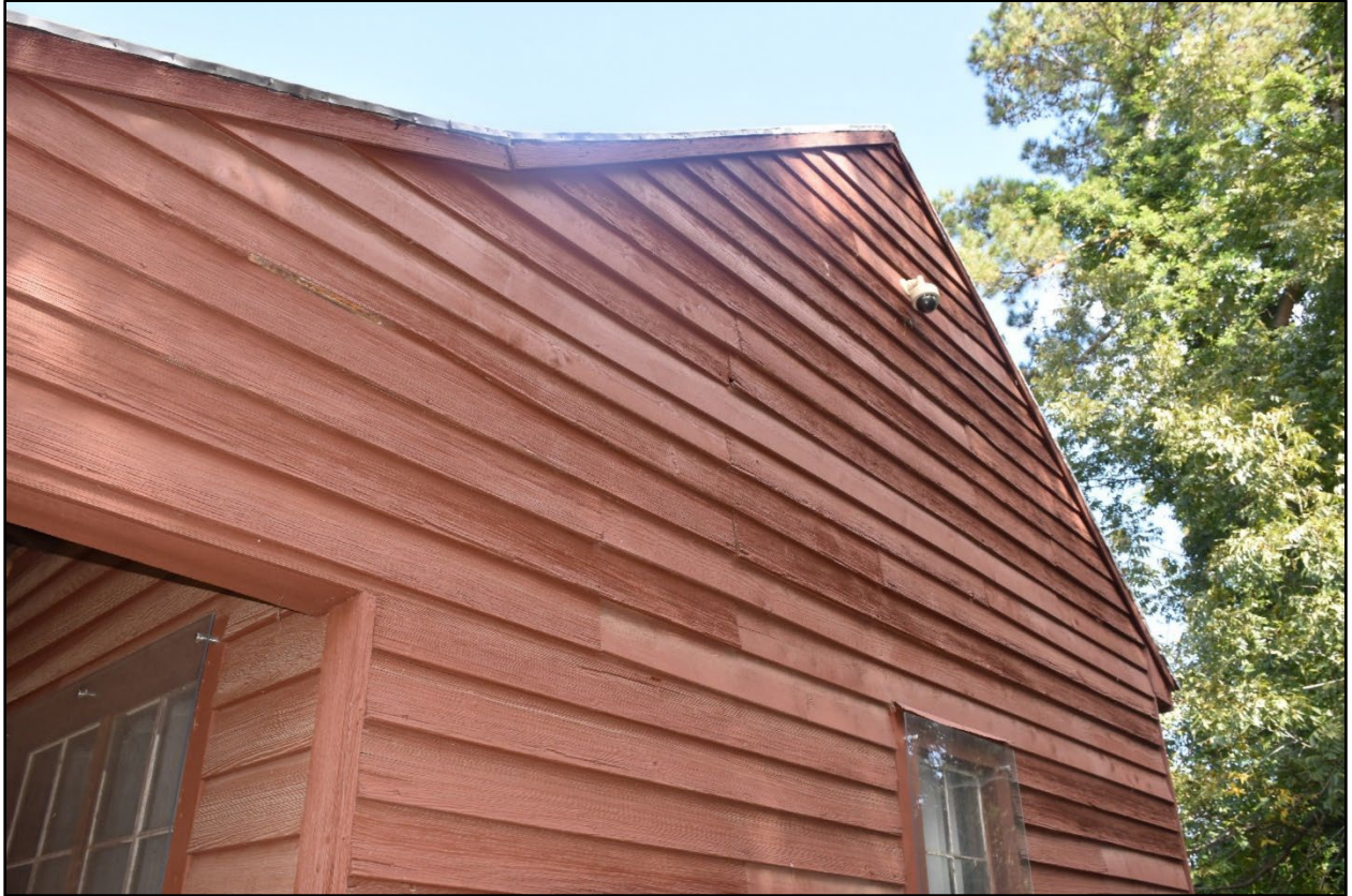
Figure 173- The wood siding of the kitchen/schoolhouse along the south elevation.
