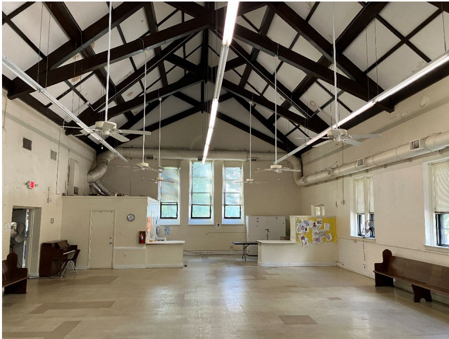
Photo 26: Church, interior, sanctuary view to south
