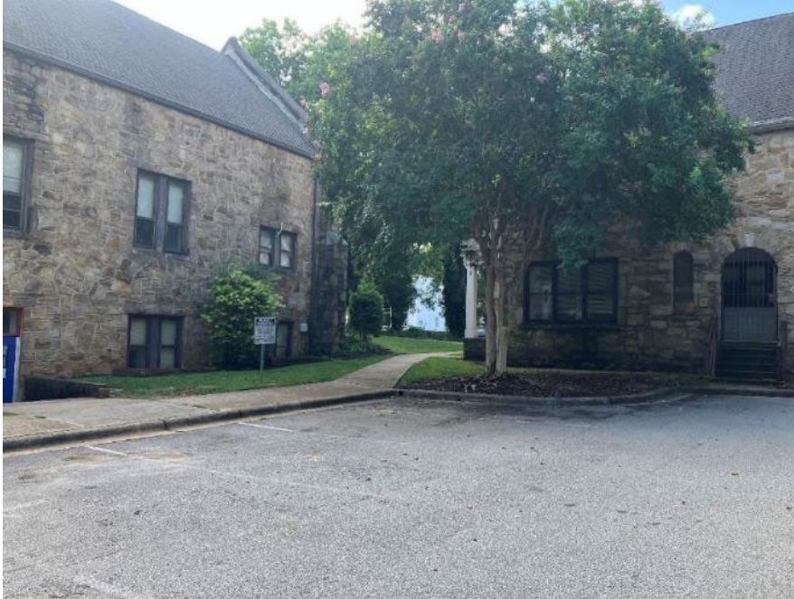
Photo 1: Northwest parking area, view to southeast
