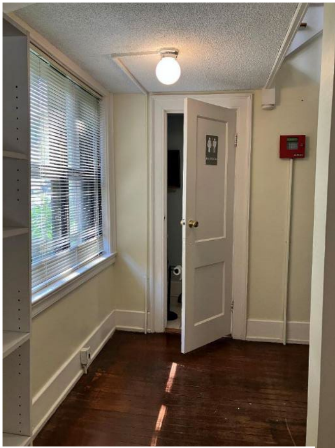
Photo 8: Rectory, first floor, hall, view to south
