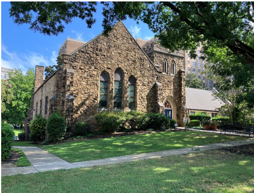
Photo 17: Church, façade, view to northeast
