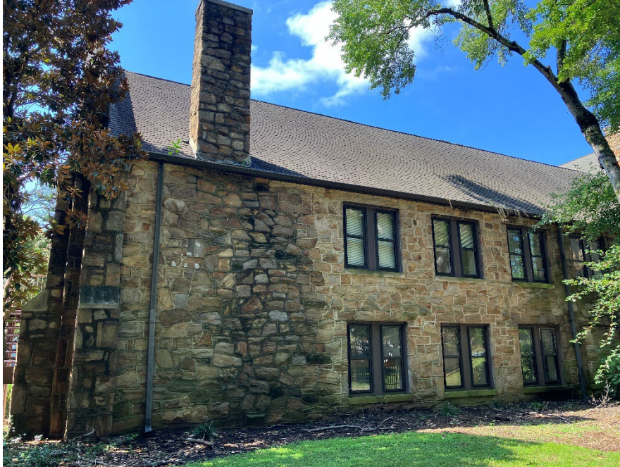
Photo 22: Church, parish hall wing, view to southwest
