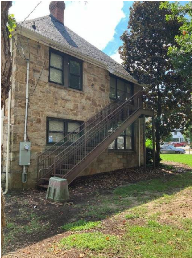
Photo 5: Rectory, west elevation, view to southeast
