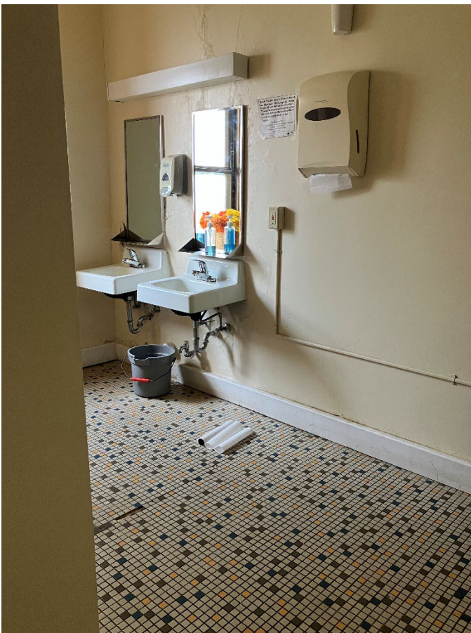
Photo 32: Church, interior, parish hall, upper level, view to southwest
