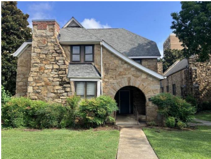
Photo 2: Rectory, facade, view to north
