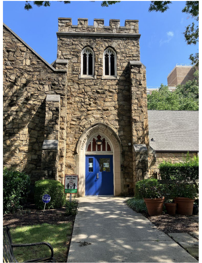
Photo 18: Church, entrance tower, view to north
