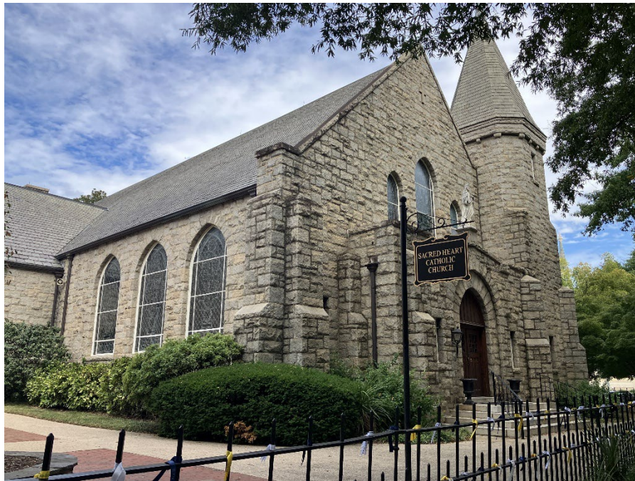
Photo 40: Sacred Heart Cathedral, view to northeast
