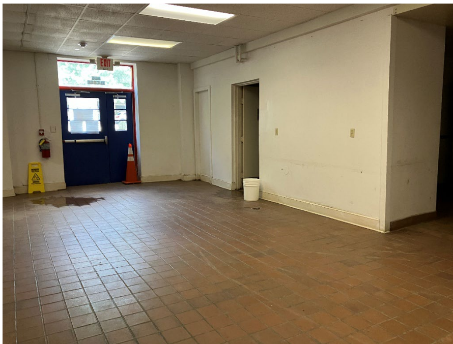
Photo 36: Church, interior, lower level, view to northwest
