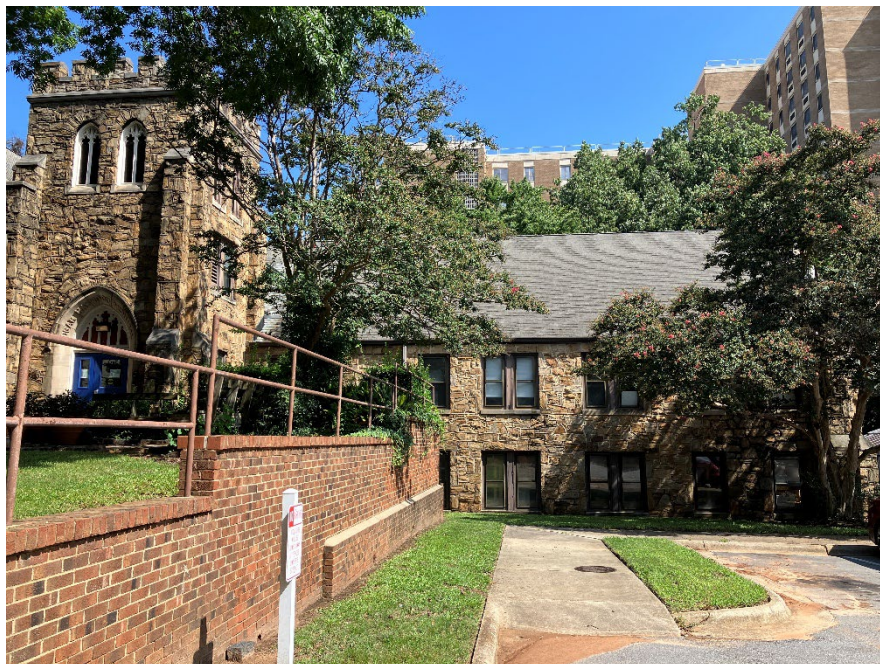
Photo 19: Church, parish hall wing, view to north
