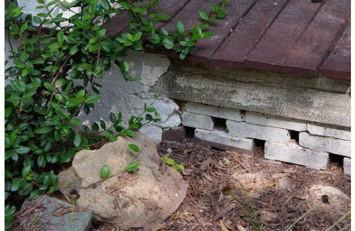
Image 9. Foundation detail at south elevation
