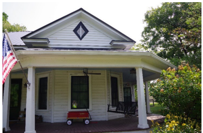
Image 4. Façade porch detail
