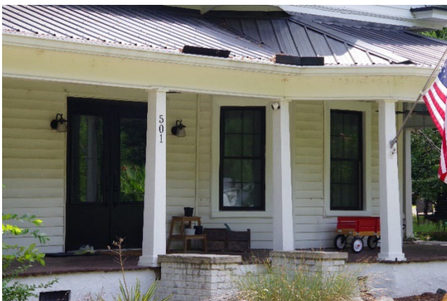
Image 3. Façade replacement doors and windows
