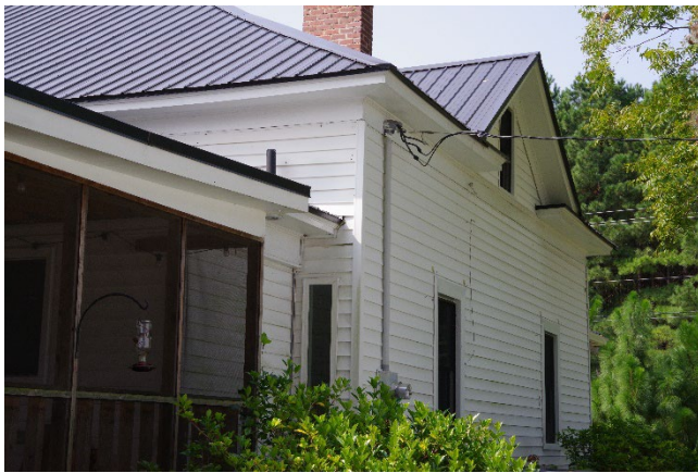
Image 5. Rear oblique, facing southwest
