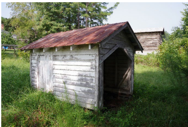
Image 18. Historic storage outbuilding, facing northwest
