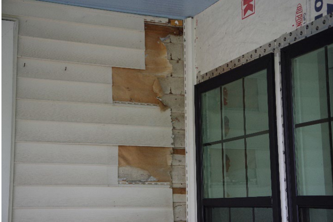
Image 8. Exposed original wood weatherboard siding
