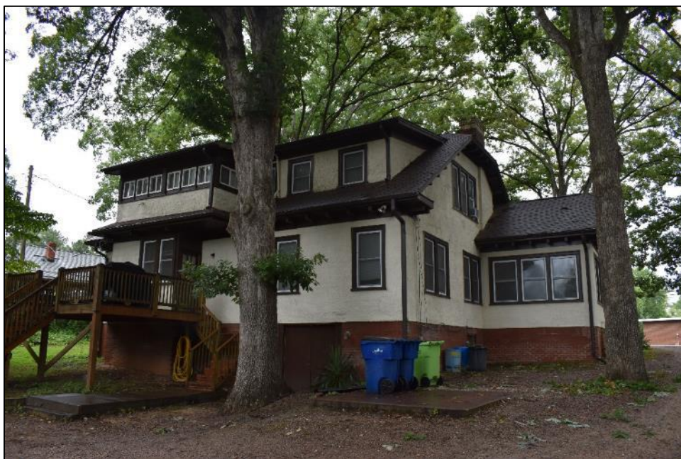
Photograph 4: 136 Jones Franklin Road, rear (west elevation).
