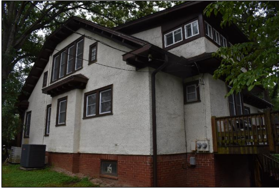
Photograph 5: 136 Jones Franklin Road, north elevation.
