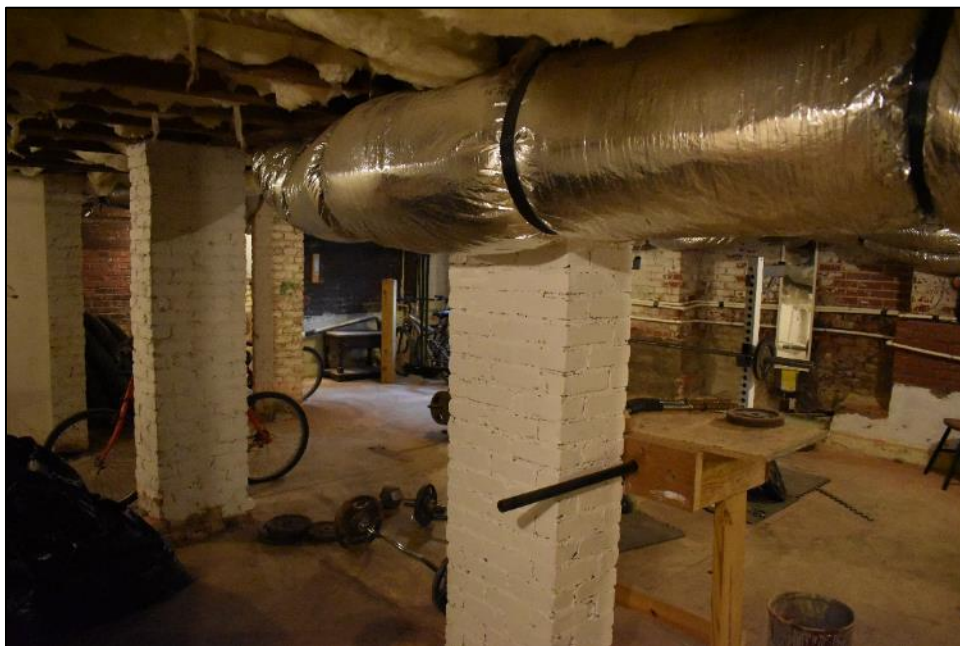
Photograph 15: 136 Jones Franklin Road, Basement level
