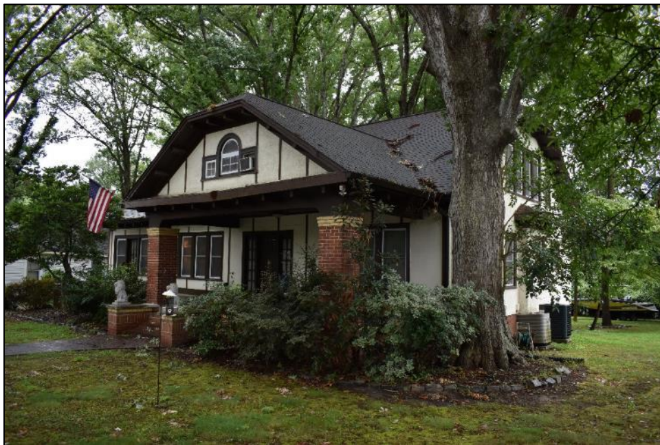
Photograph 3: 136 Jones Franklin Road, façade (east elevation) and north side elevation.
