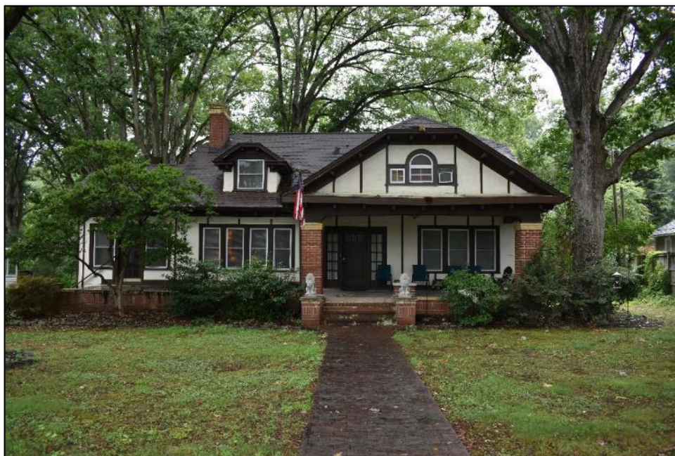
Photograph 1: 136 Jones Franklin Road, facade (east elevation).
