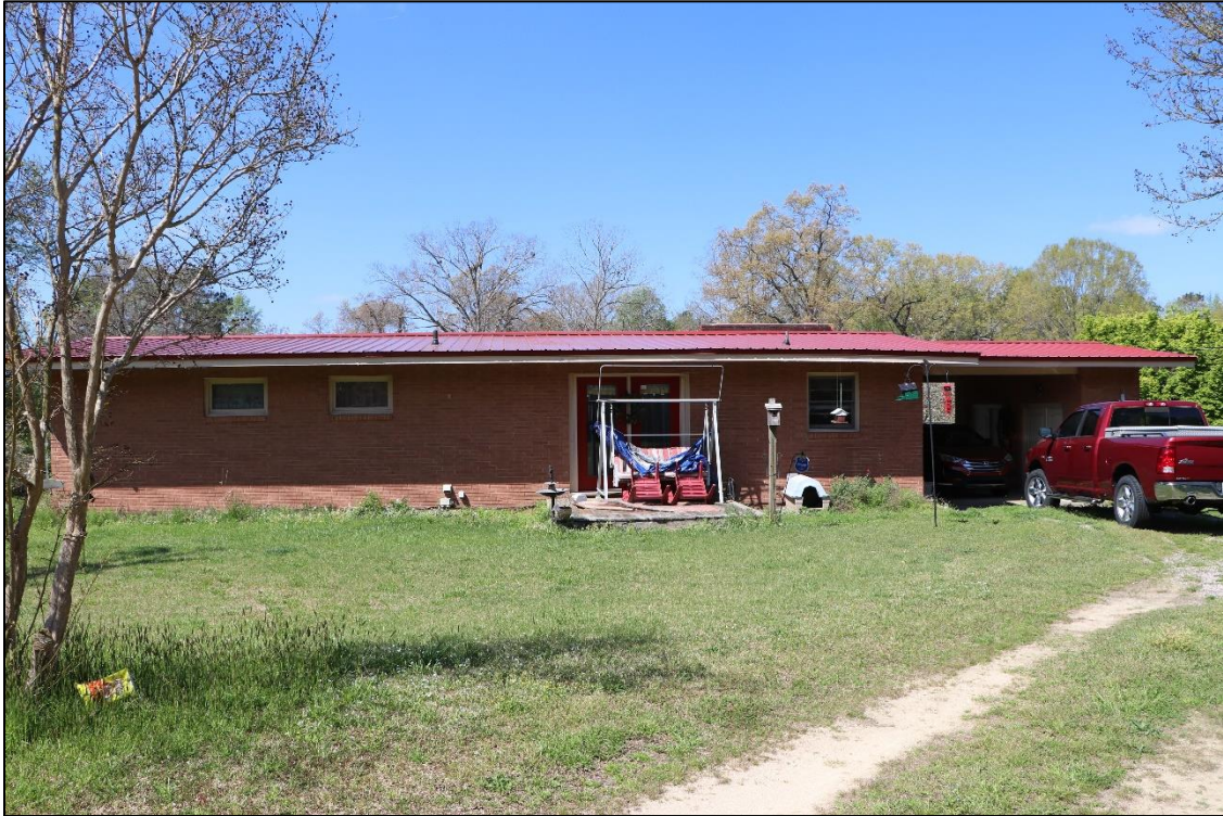
Figure 7: Alva and Dan Benton House, east elevation, 2023.
