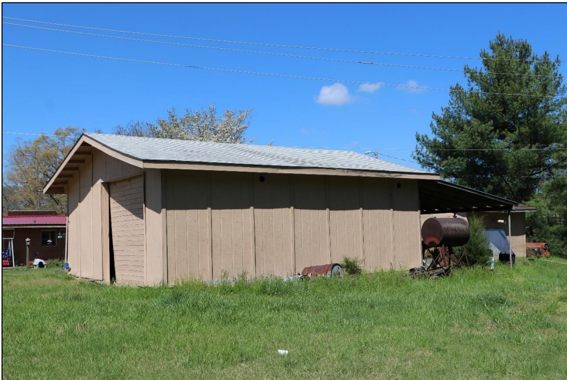
Figure 10: Circa 1967 storage shed, south and east elevations, 2023.
