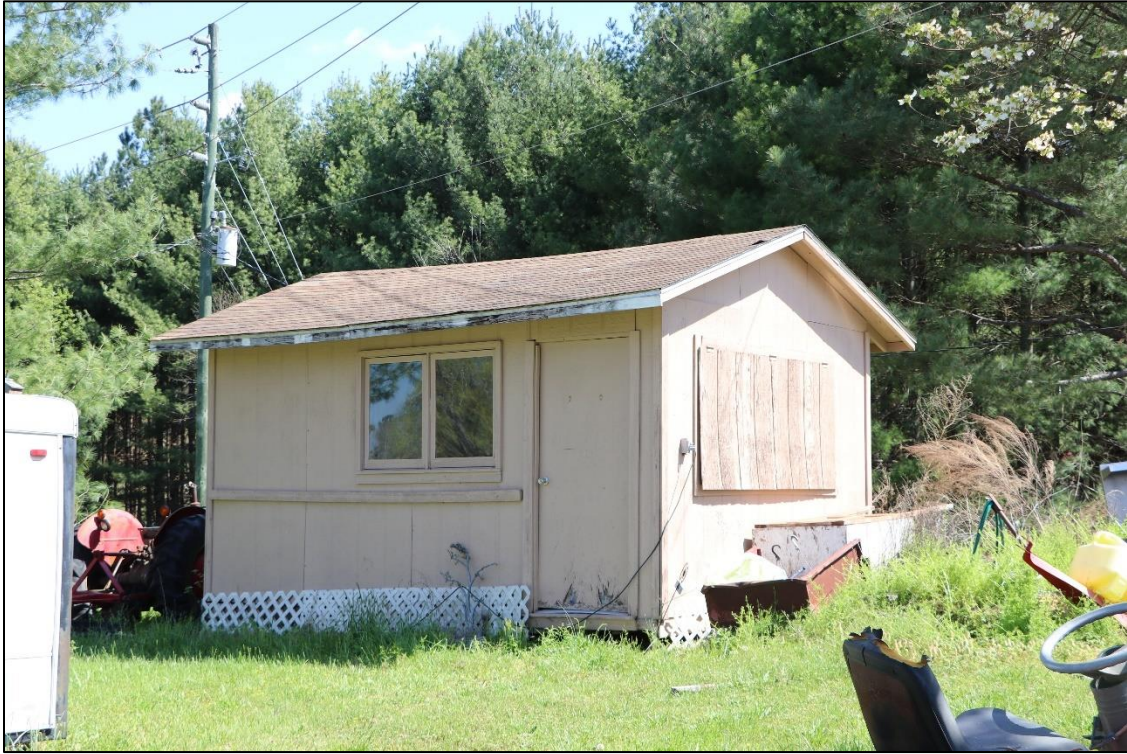
Figure 11: 1990s storage shed, west and south elevations, 2023.
