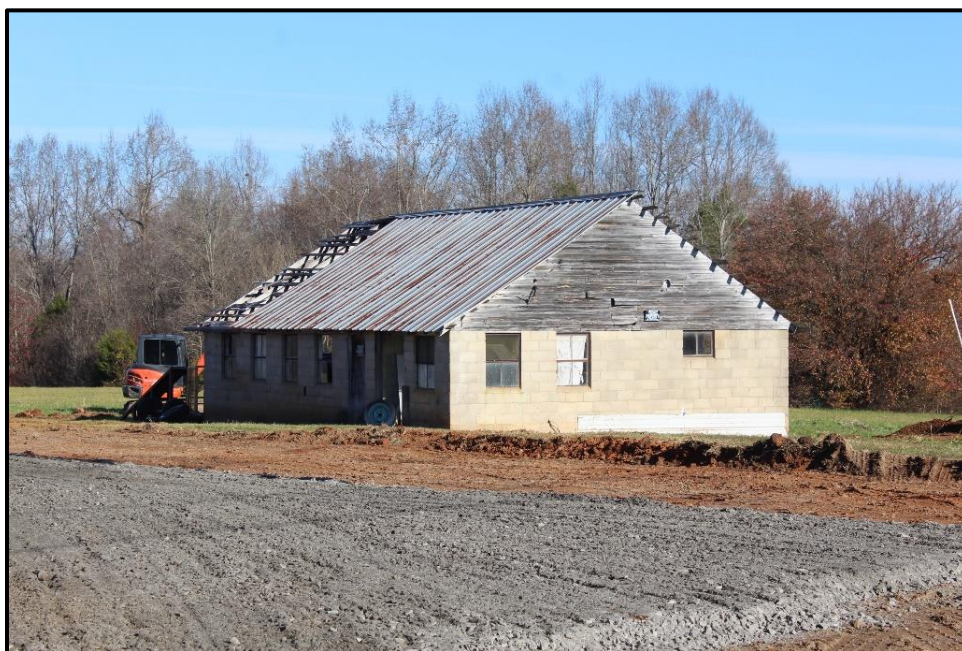
Figure 10 Machine/Maintenance Shop (CT1811), 1710 NC Highway 16, View Looking Southwest.
