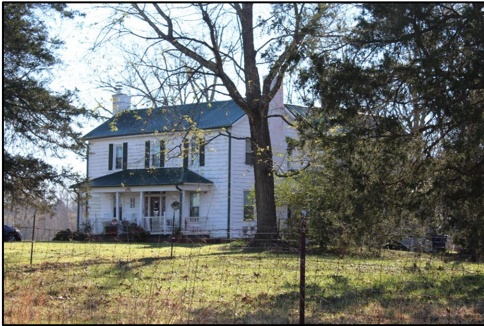
Figure 7 Frederick William Smith House (CT0794), 1710 NC Highway 16, View Looking Southeast.
