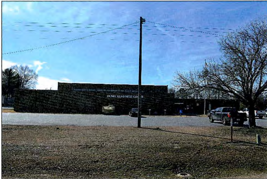
Figure 8.4. North elevations of the Dunn Armory.
