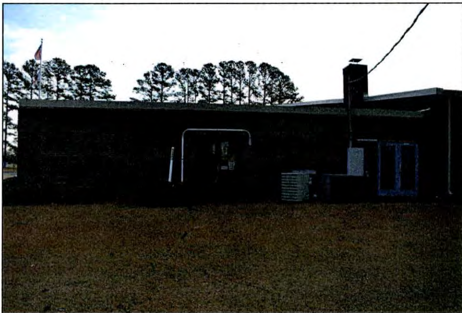
Figure 13.11. Side entrance on west elevation of the Whiteville Armory.
