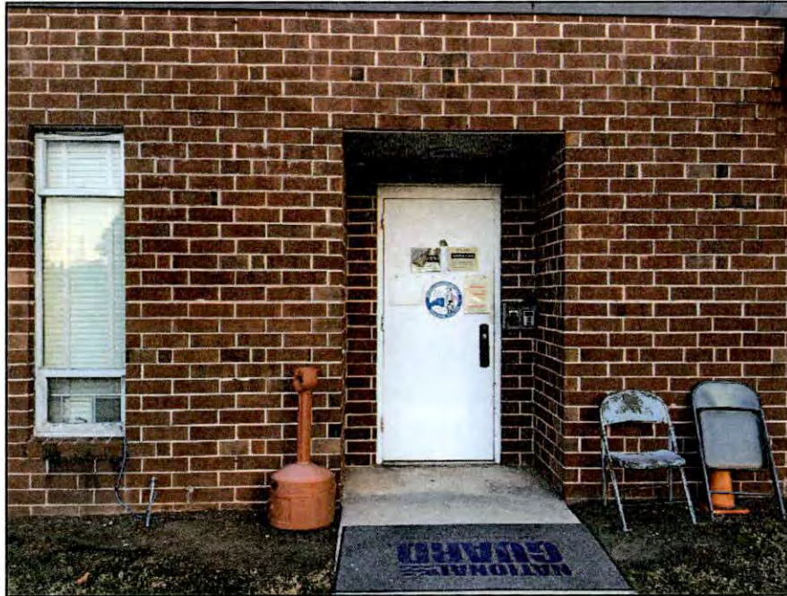
Figure 7.10. Second entrance along the south elevation of the Butner Armory.
