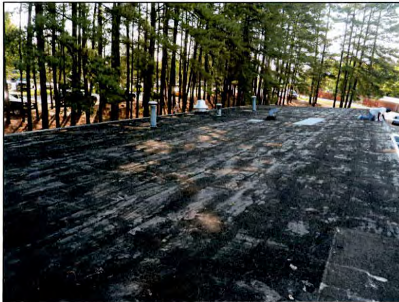
Figure 12.11. Roof of the Raleigh TMP at Raleigh Armory before renovation.
