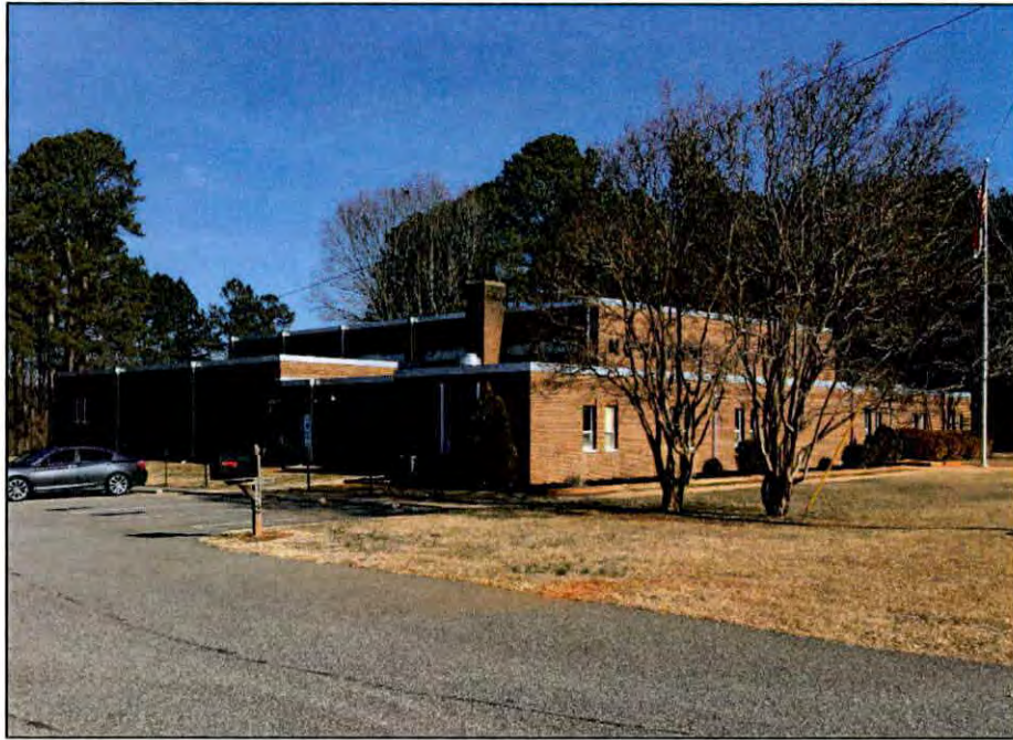
Figure 14.5. West and south elevations of the Youngsville Armory.
