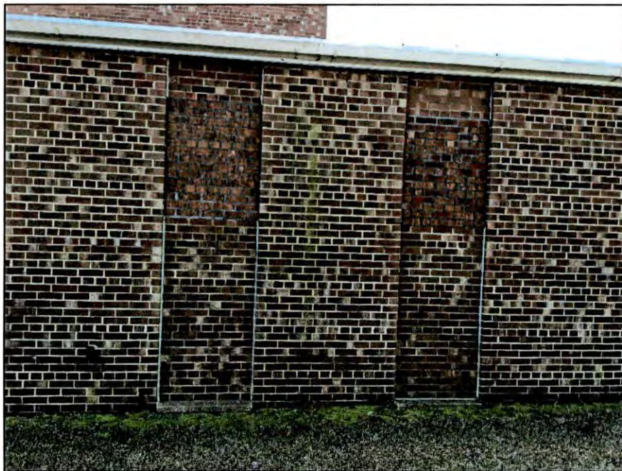
Photo 5.8. View of wall openings infilled with brick along the north elevation of the Beulaville Armory.
