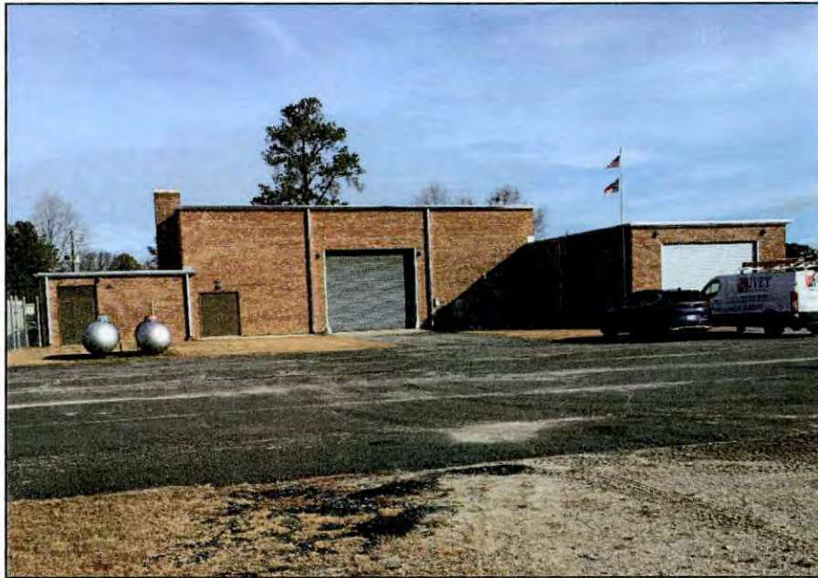
Photo 5.5. South and west elevations of the Beulaville Armory, facing northeast.
