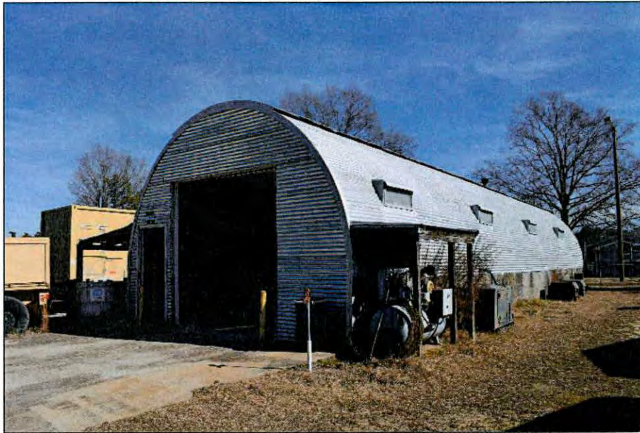
Figure 8.14. West and south elevations of the Quonset Storage Building.
