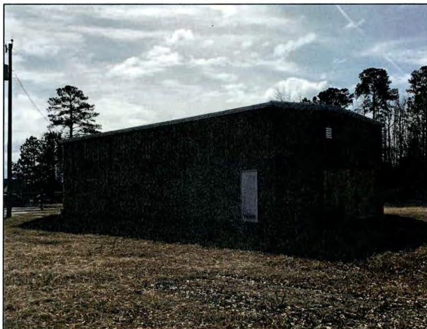
Photo 5.30. North and west elevations of the large storage building at the Beulaville Armory.
