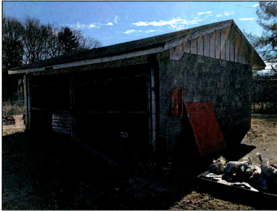
Figure 11.21. North and west elevations of the first Organizational Storage Building.
