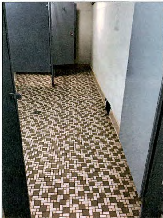
Figure 14.19. Representative bathroom at the Youngsville Armory.
