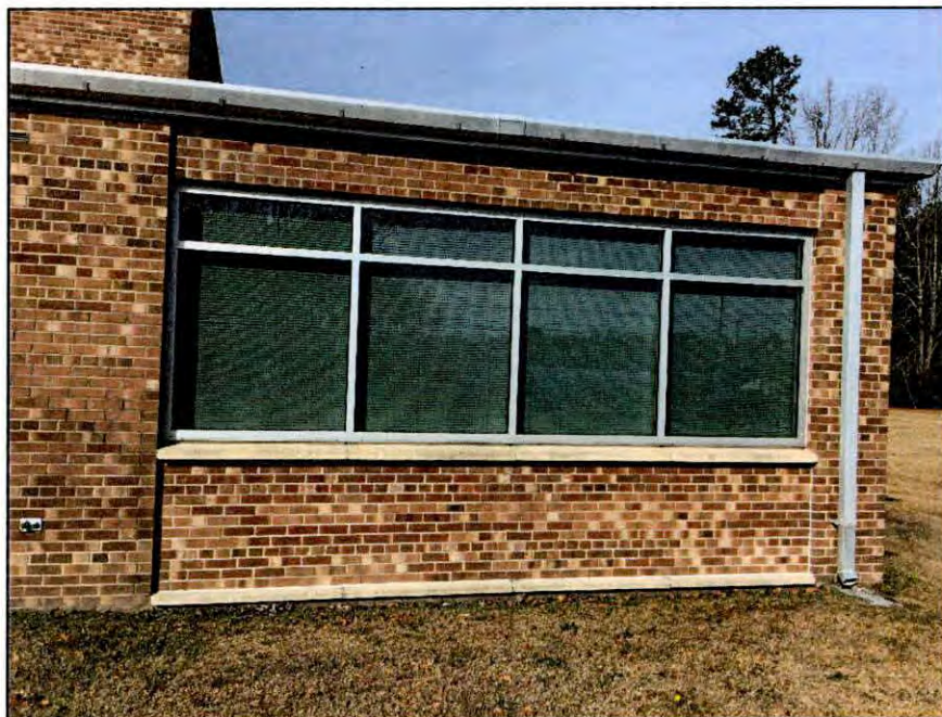
Photo 5.2. View of group of four fixed windows with transoms along the east or front elevation of the Beulaville Armory.
