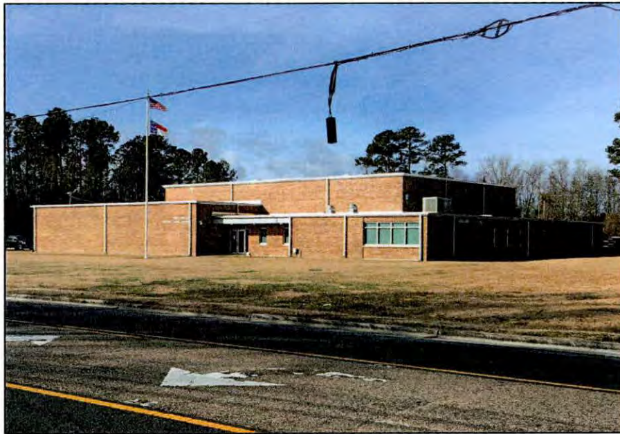
Photo 5.1. East and north elevations of the Beulaville Armory, facing southwest.
