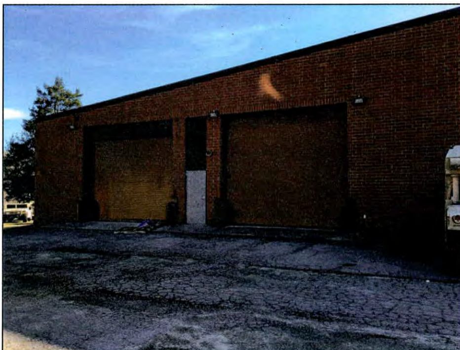
Figure 10.9. North elevation of the Louisburg Armory.
