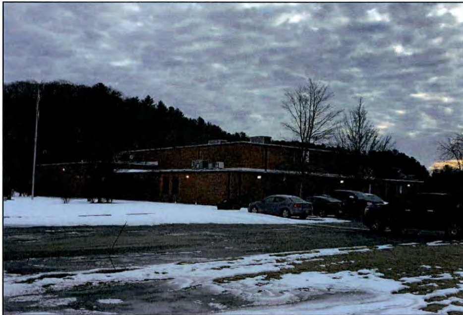
Photo 6.1. North and west elevations of the Boone Armory.
