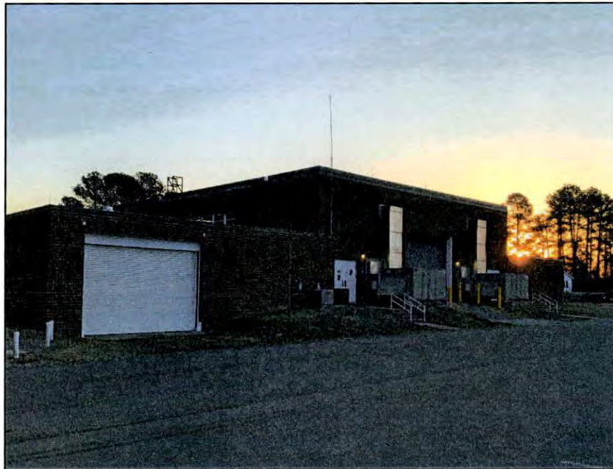
Figure 7.11. West elevation of the Butner Armory.
