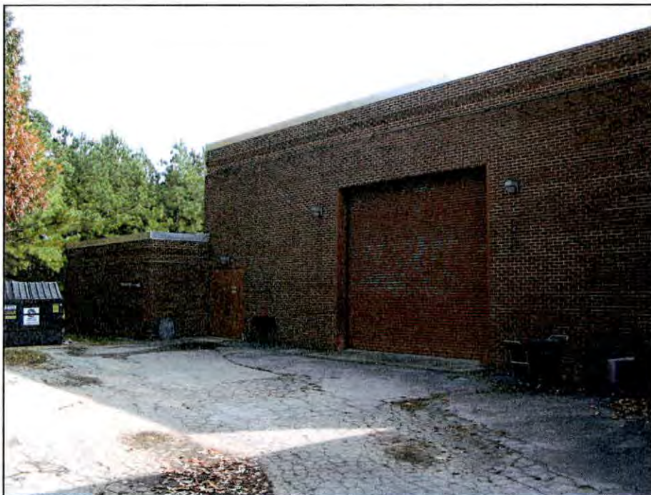
Figure 14.30. Original overhead garage door at the Youngsville Armory.
