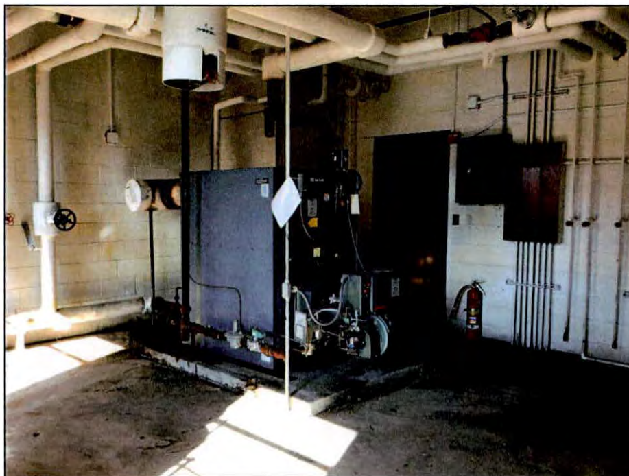
Figure 6.29. Boiler Room at Boone Armory.
