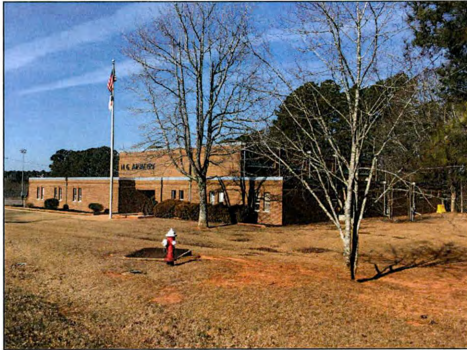
Figure 14.11. South and east elevations of the Youngsville Armory.
