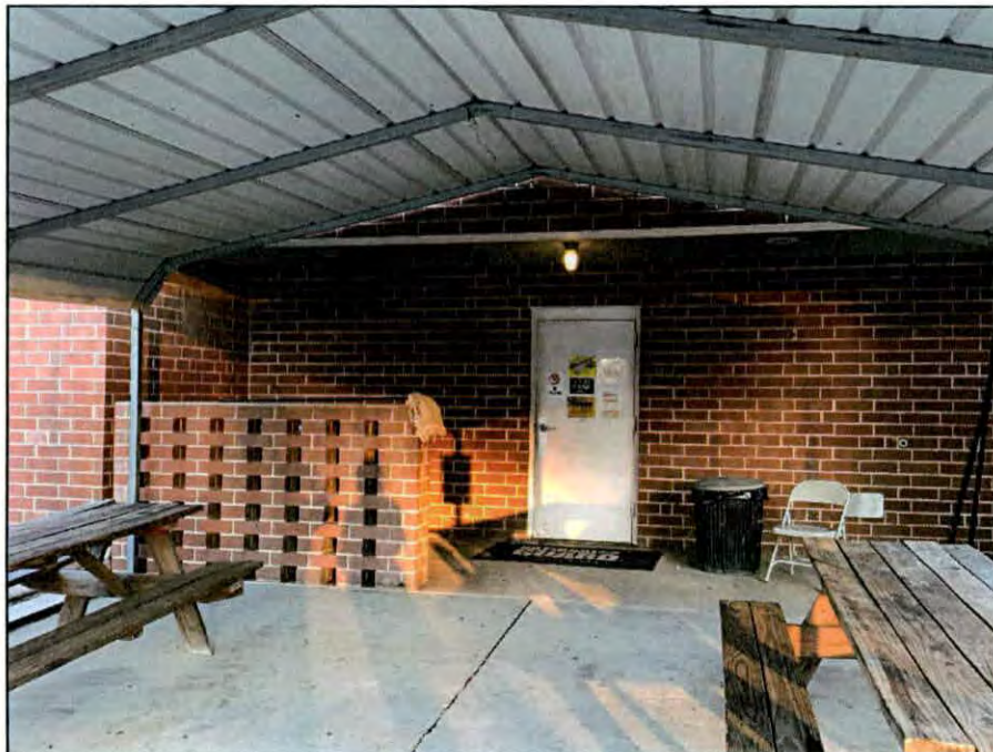
Figure 7.9. First entrance along the south elevation of the Butner Armory.
