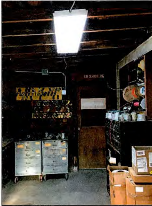
Figure 7.51. The interior of the fire repair building tool room associated with the Butner Armory.
