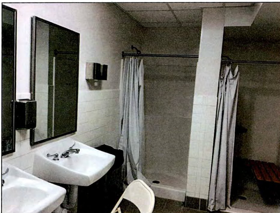
Photo 5.16. Representative restroom at the Beulaville Armory.
