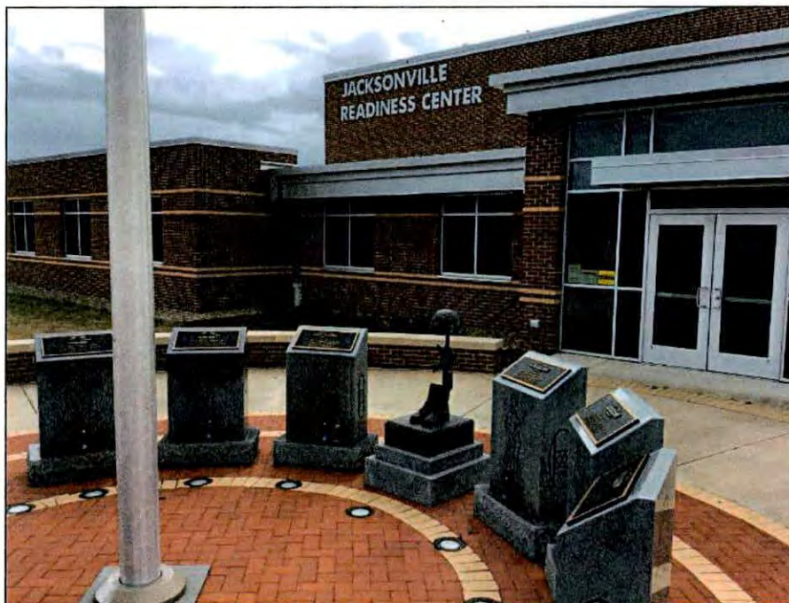
Figure 9.7. Lettering along the northeast elevation of the Jacksonville Armory and partial view of memorial to fallen soldiers near front entrance.
