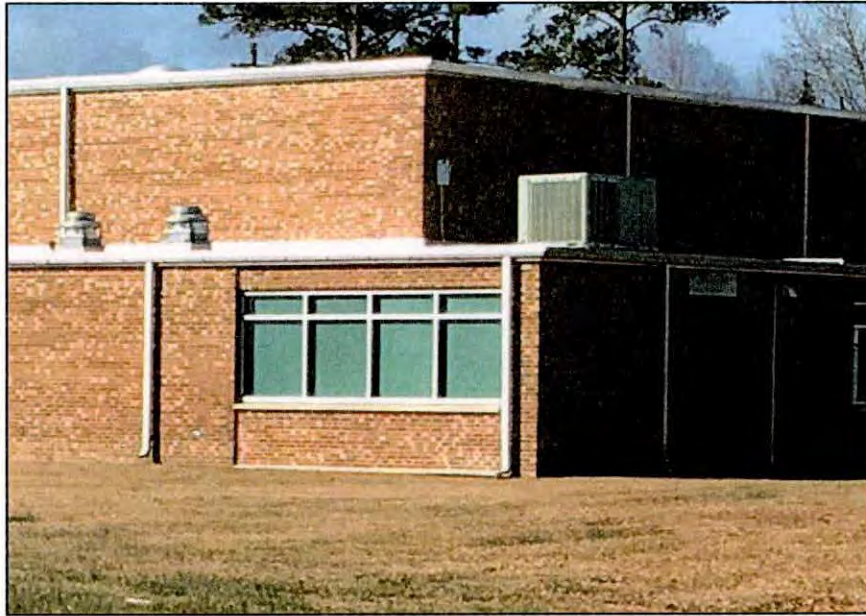
Photo 5.28. Replacement windows along the south elevation of the Beulaville Armory.
