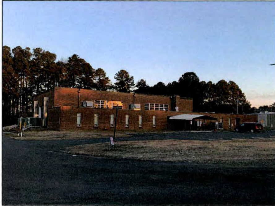
Figure 7.8. West and south elevations of the Butner Armory.
