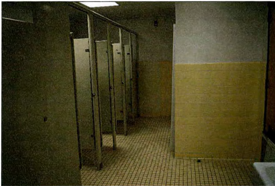
Figure 8.11. Representative restroom at the Dunn Armory.
