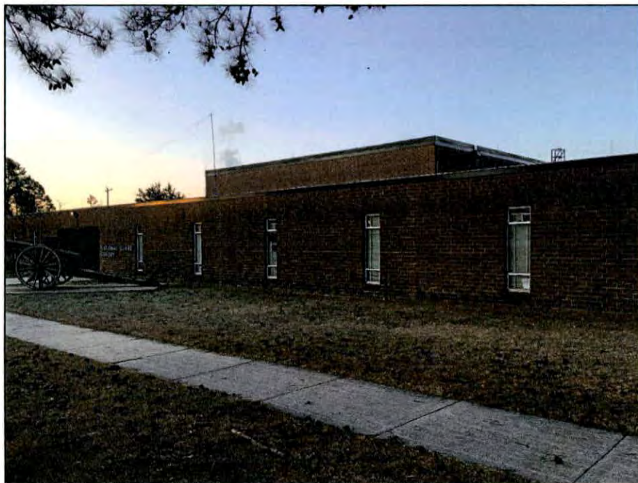
Figure 7.5. Row of windows along the east elevation of the Butner Armory.
