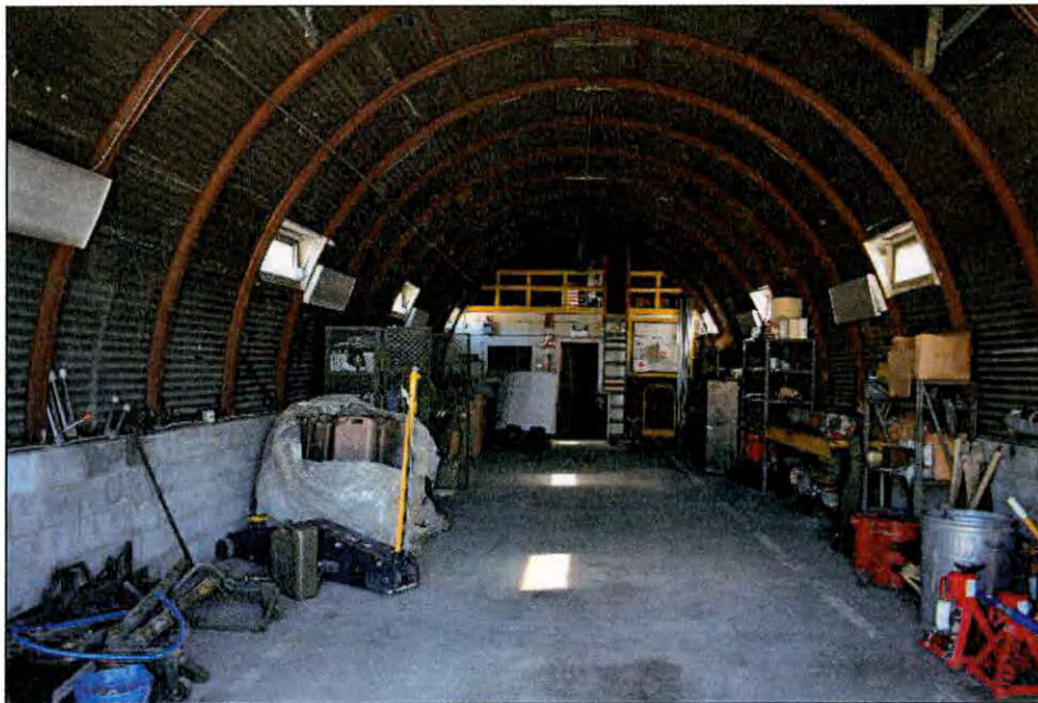
Figure 8.15. Interior of the Quonset Storage Building.
