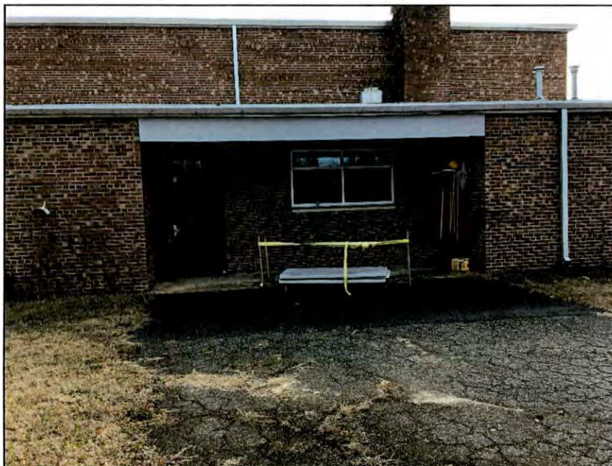
Photo 5.12. Recessed entrance along the west elevation of the Beulaville Armory, facing east-southeast.
