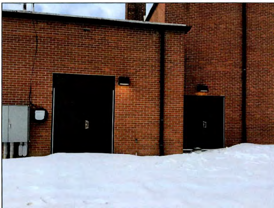
Figure 6.12. East elevation of the Boone Armory.
