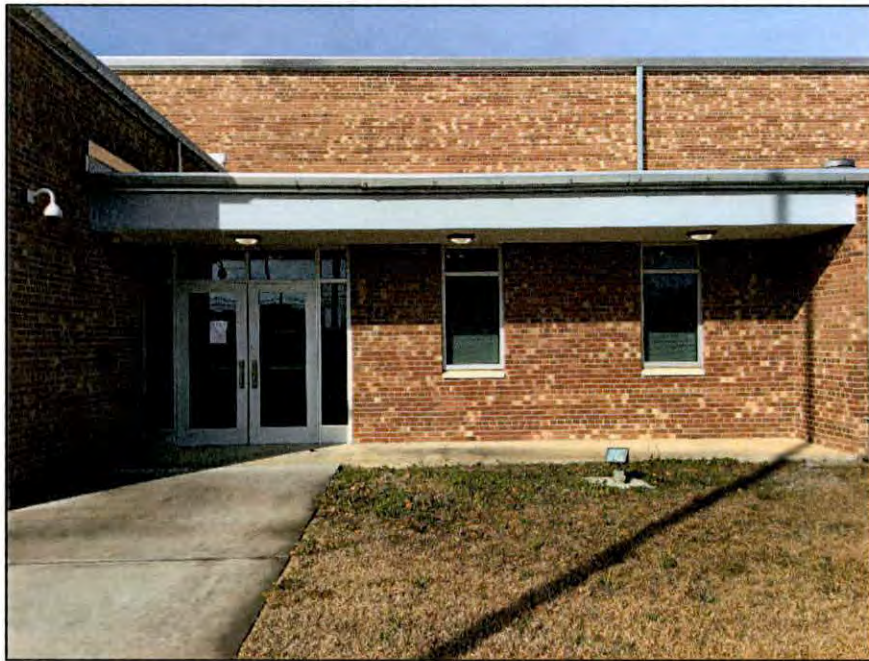
Photo 5.3. View of main entrance and windows along the east or front elevation of the Beulaville Armory.
