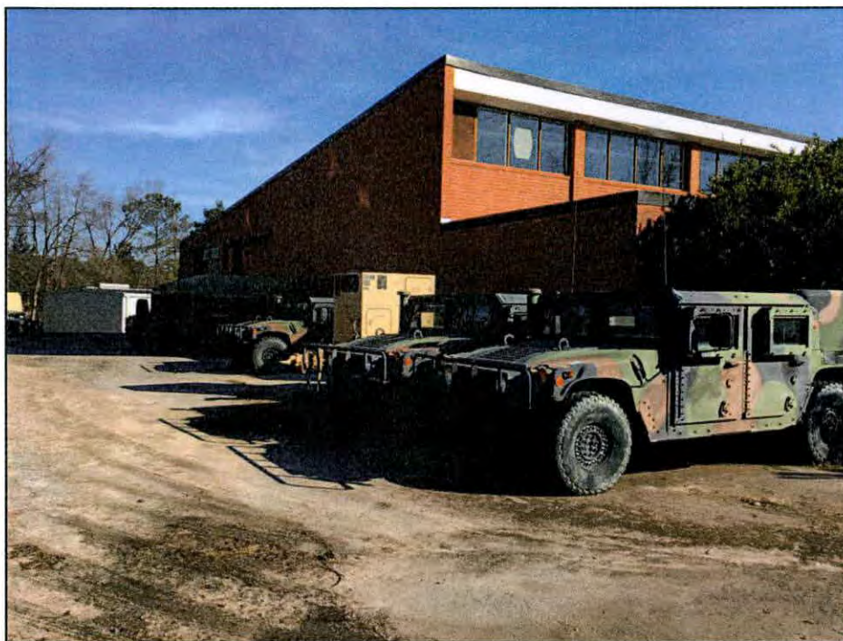
Figure 10.8. North and west elevations of the Louisburg Armory and motor pool.
