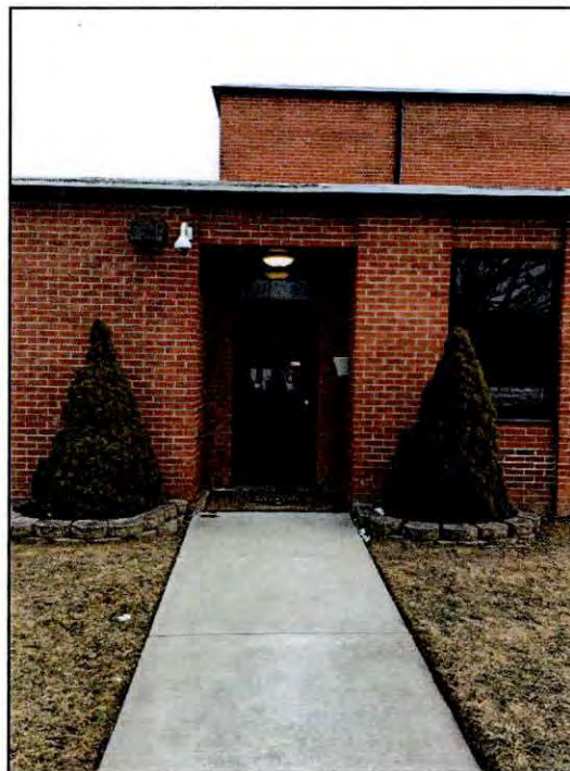
Figure 6.10. West elevation of the Boone Armory.
