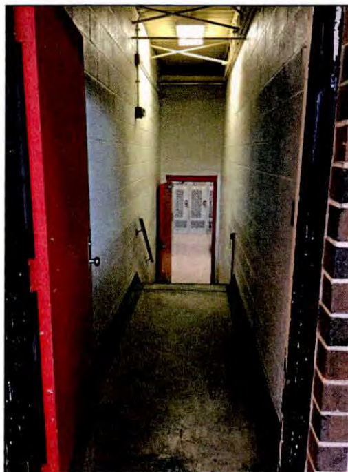
Figure 7.17. Representative corridor or hall at the Butner Armory.
