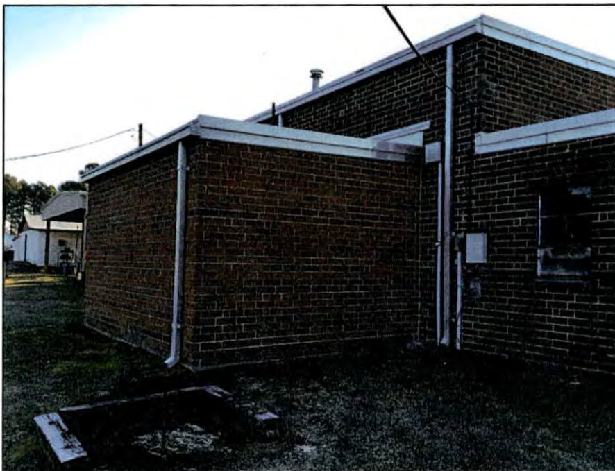
Figure 7.31. Small one-story addition along the north elevation of the original section of the Facility Maintenance Shop (FMS).
