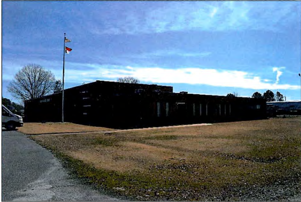
Figure 8.6. North and west elevations of the Dunn Armory.
