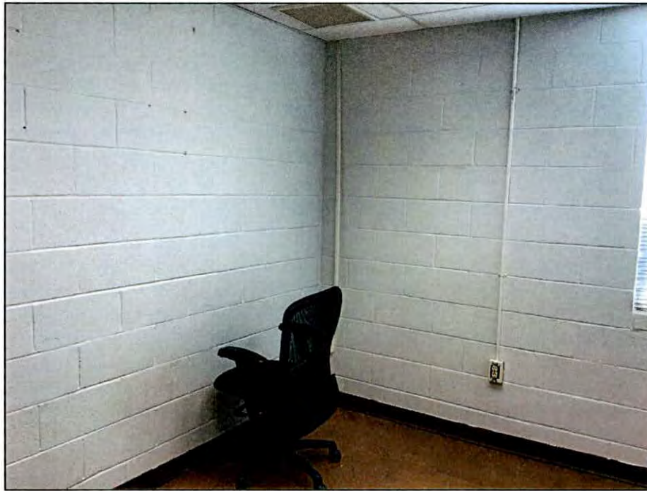
Figure 14.28. Representative empty office space at the Youngsville Armory.
