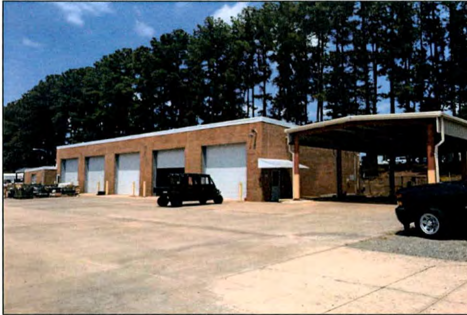
Figure 12.2. South and east elevations of the Raleigh TMP at Raleigh Amory; note the non-historic carport.
