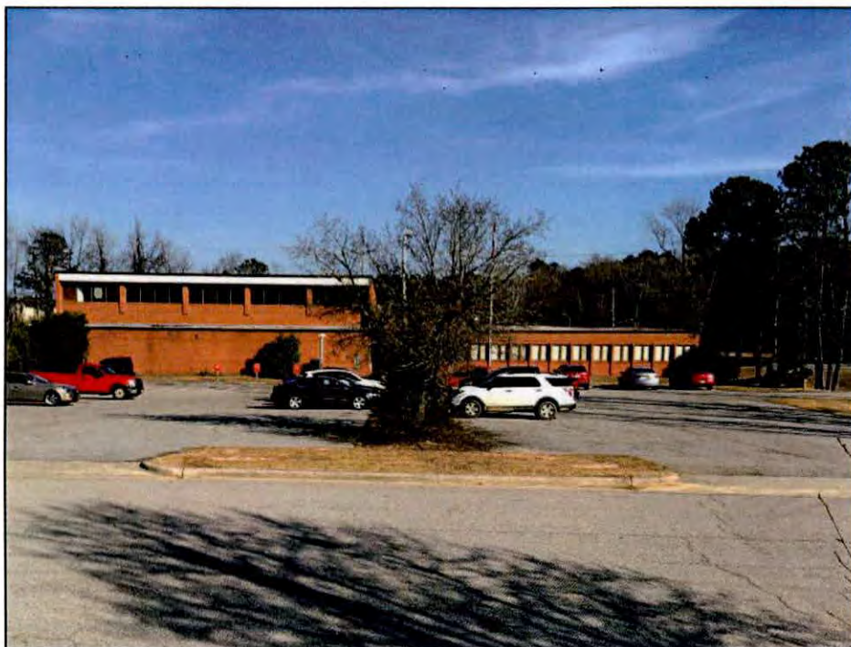
Figure 10.7. West elevation of the Louisburg Armory.
