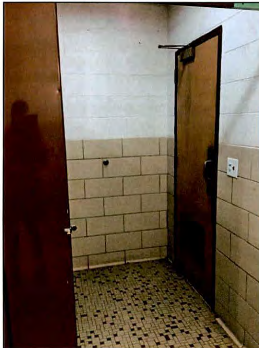
Figure 11.18. Representative restroom at the Mocksville Armory.
