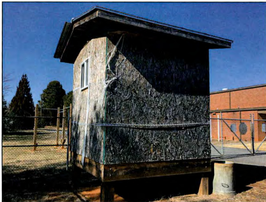
Figure 11.24. South and east elevations of the Training Building.
