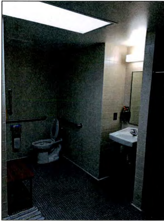
Figure 12.18. Bathroom of the Raleigh TMP at Raleigh Armory after renovation.
