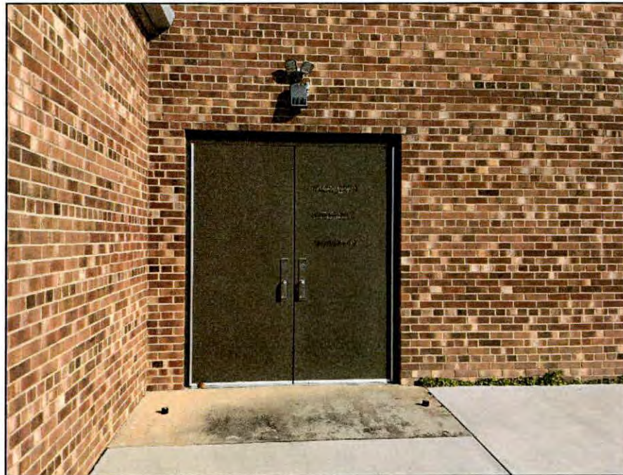
Photo 5.6. Set of metal replacement double doors along the south elevation of the Beulaville Armory.
