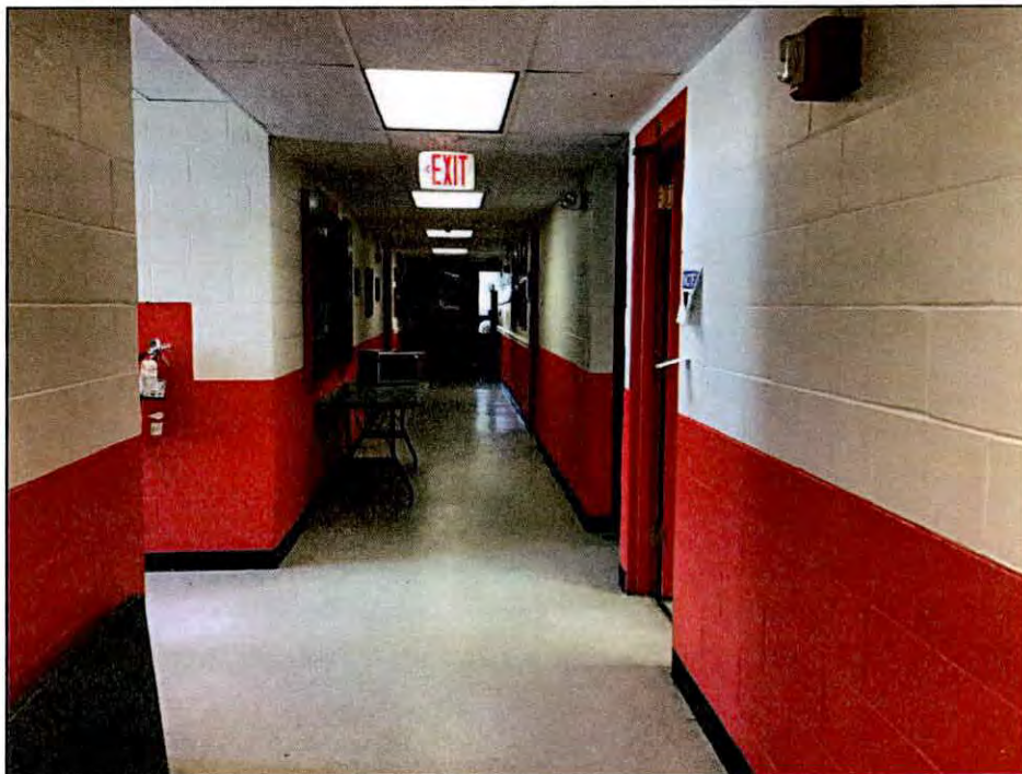
Figure 10.16. Representative corridor in the Louisburg Armory.
