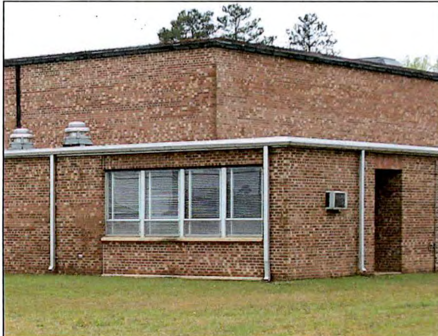
Photo 5.27. Original windows before replacement along the south elevation of the Beulaville Armory.
