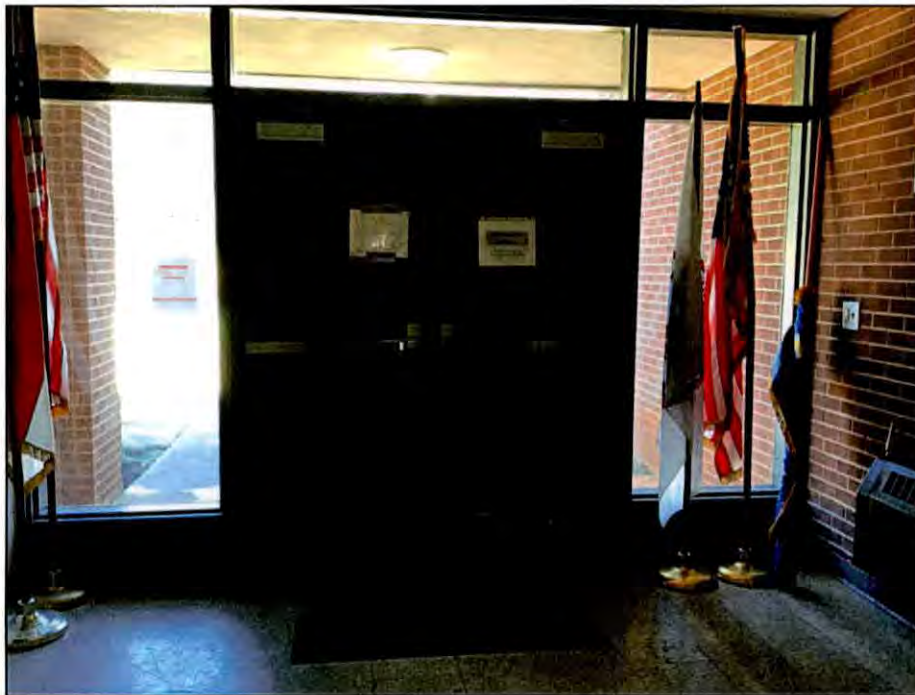
Figure 11.10. The interior of the main front entry of the Mocksville Armory.
