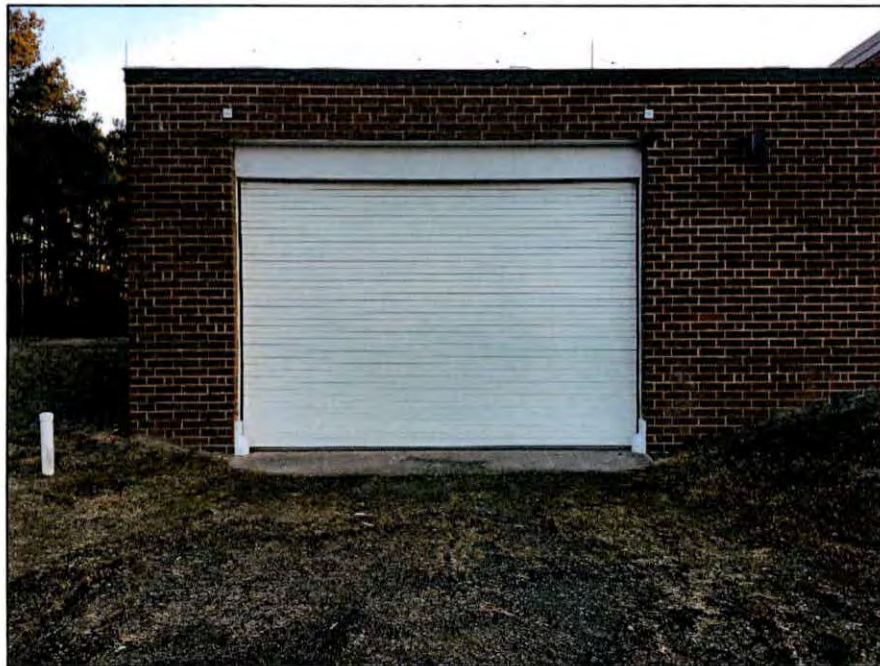
Figure 7.13. First garage door along the west elevation of the Butner Armory.
