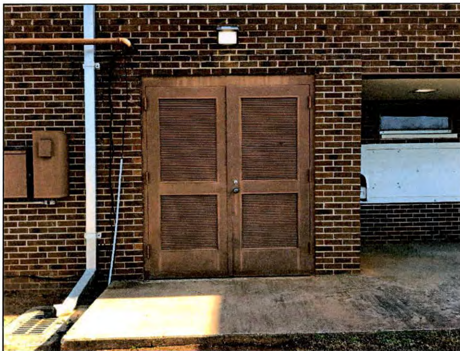
Figure 14.8. Louvered double doors along the west elevation of the Youngsville Armory.
