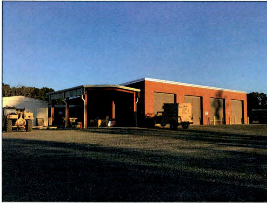
Figure 7.28. West and south elevations of the Facility Maintenance Shop (FMS).
