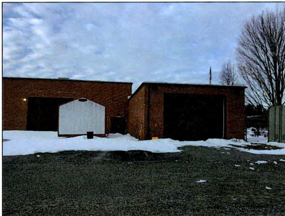
Figure 6.13. East elevation of the Boone Armory.
