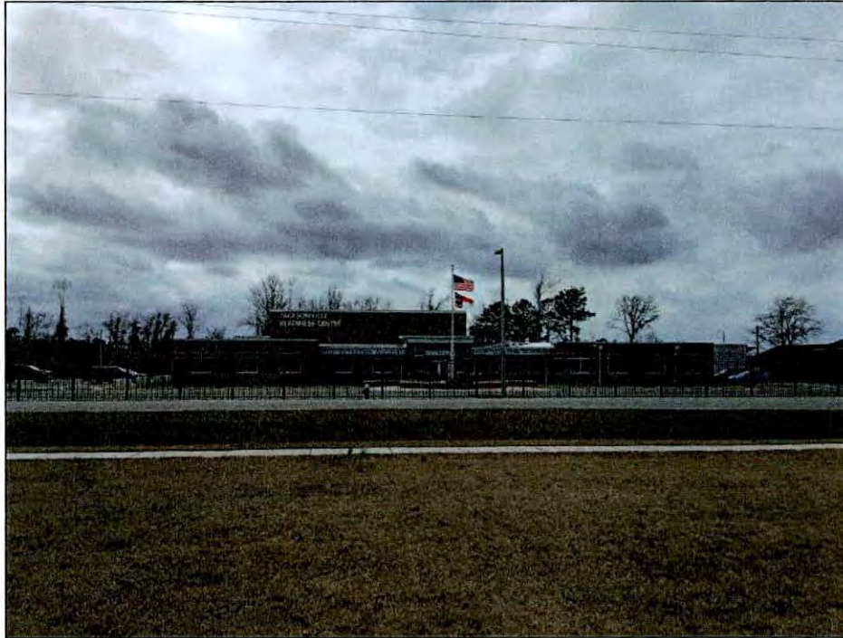
Figure 9.6. Northeast or main elevation of Jacksonville Armory.
