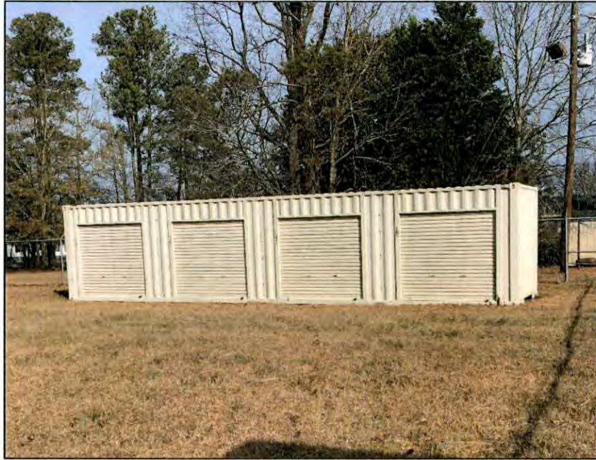
Photo 5.32. South elevation of the small storage building at the Beulaville Armory.
