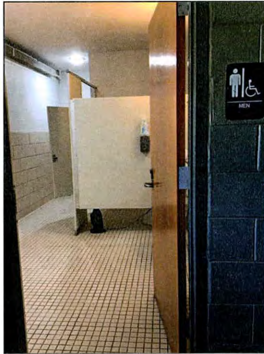
Figure 11.19. Men's restroom at Mocksville Armory.
