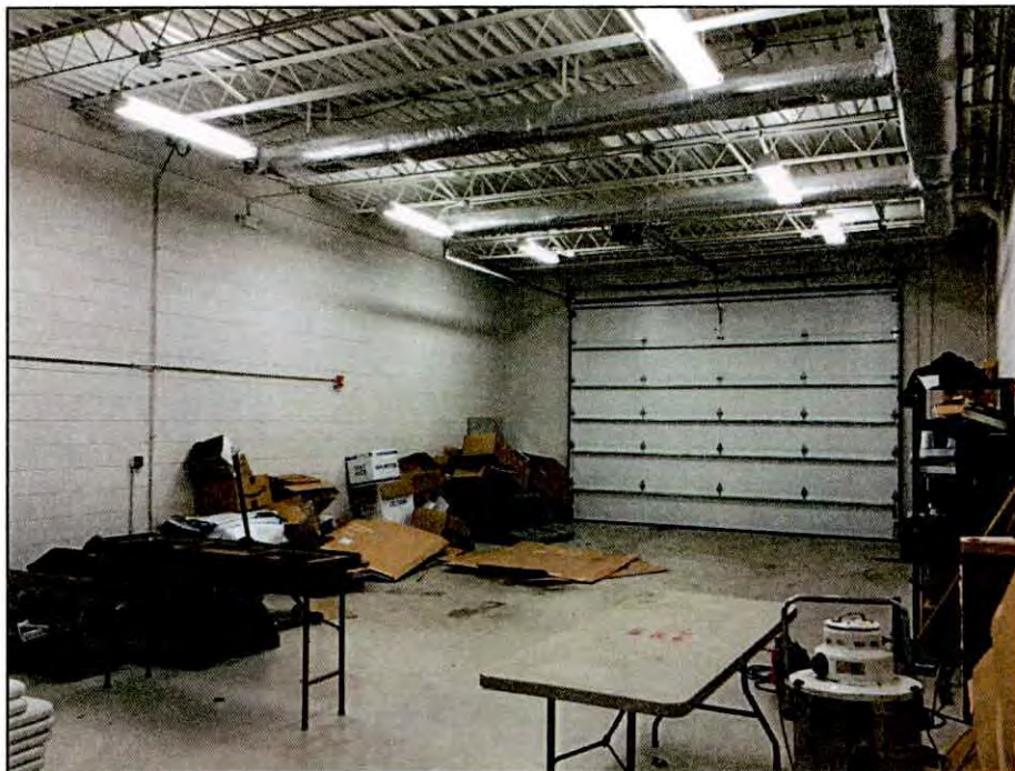
Figure 6.31. Vehicle maintenance room (former rifle range) at Boone Armory.
