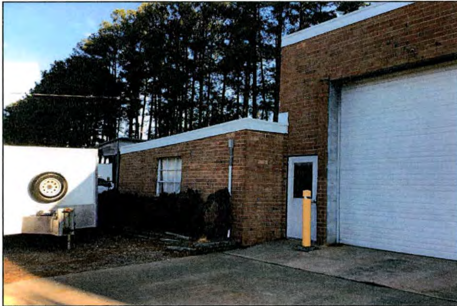
Figure 12.4. South elevation of the Raleigh TWP at Raleigh Armory.
