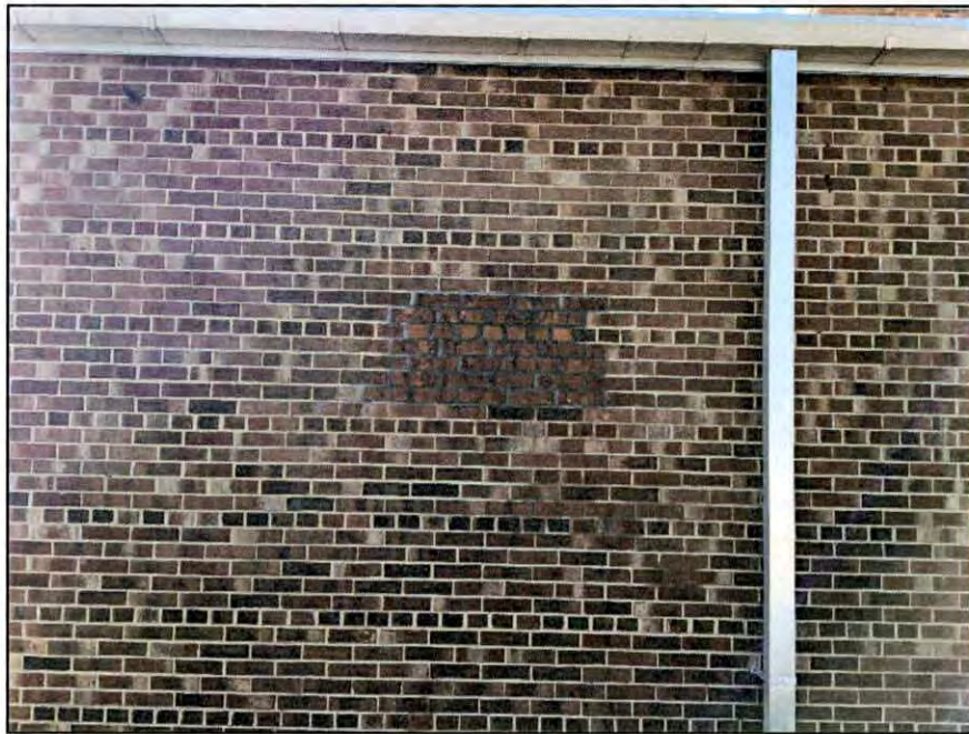
Photo 5.7. View of former vent wall opening infilled with brick along the north elevation of the Beulaville Armory.
