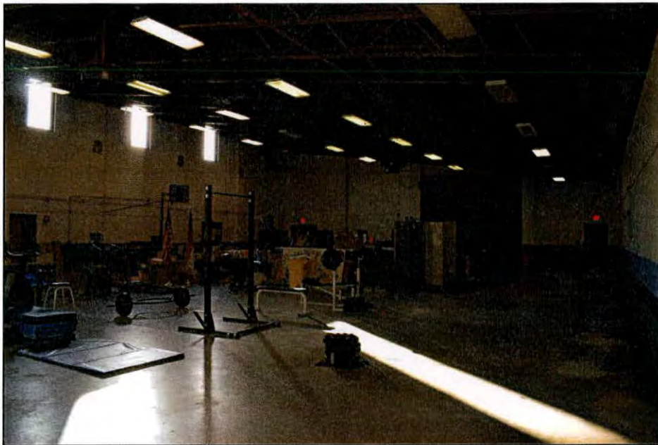
Figure 13.18. The centralized assembly hall at Whiteville Armory.
