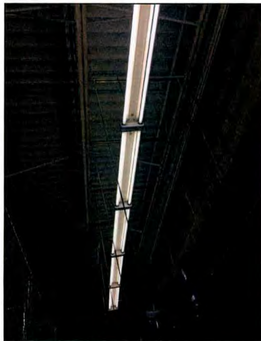
Figure 12.15. Interior overhead lighting of the Raleigh TMP at Raleigh Armory before replacement.
