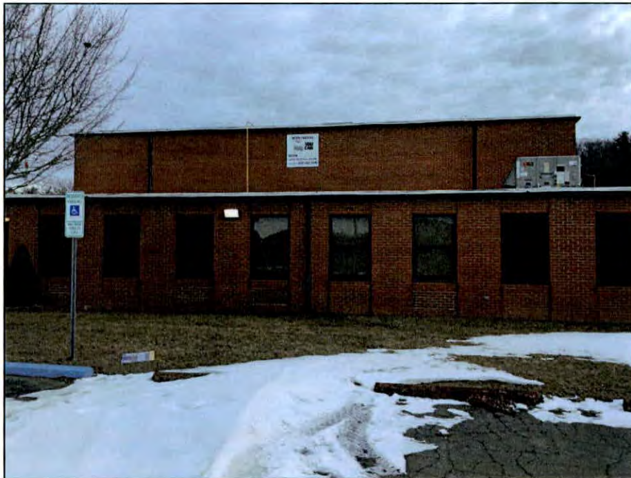
Figure 6.11. West elevation of the Boone Armory.
