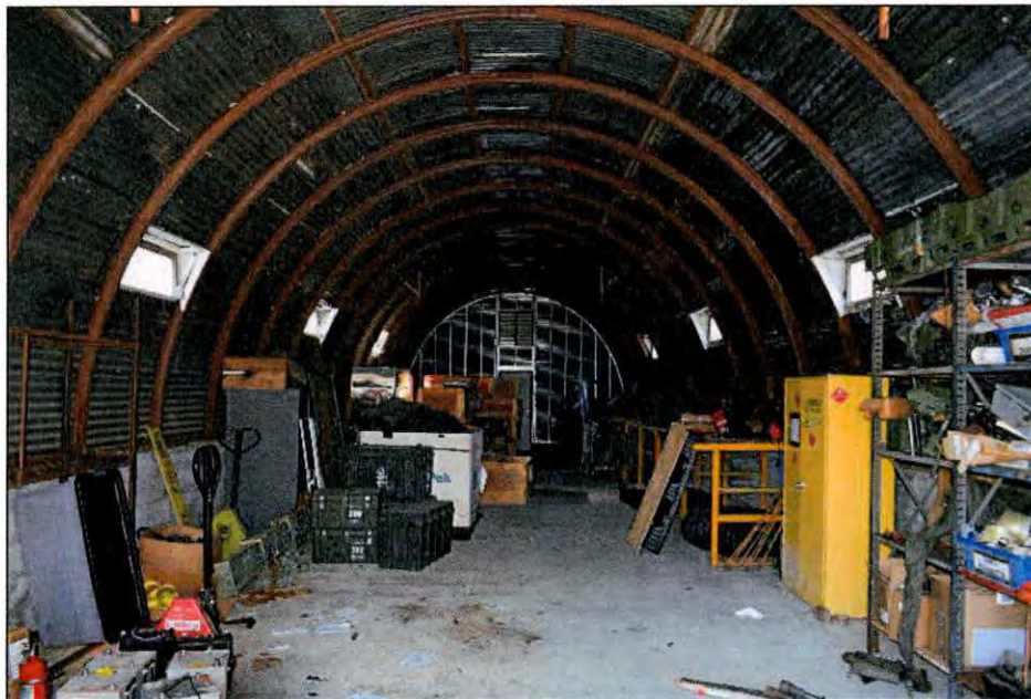
Figure 8.17. Interior of the Quonset Storage Building.
