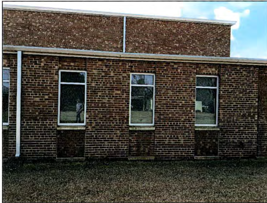
PHoto 5.9. View of wall openings infilled with brick beneath the fixed windows along the north elevation of the Beulaville Armory.
