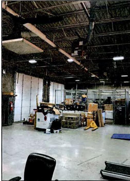
Figure 12.16. Interior overhead lighting of the Raleigh TMP at Raleigh Armory after replacement.
