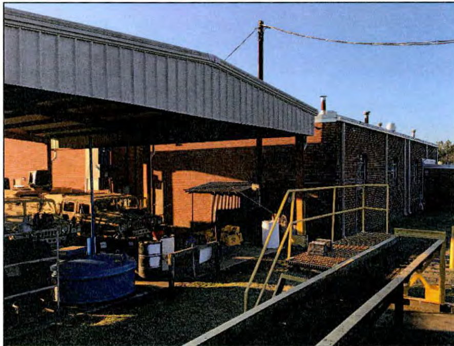
Figure 7.30. East and north elevations of the Facility Maintenance Shop (FMS).
