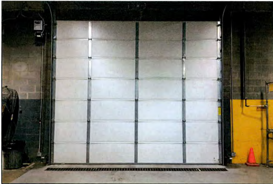
Figure 12.8. Vehicle maintenance bay or motor pool in the Raleigh TMP at Raleigh Armory.
