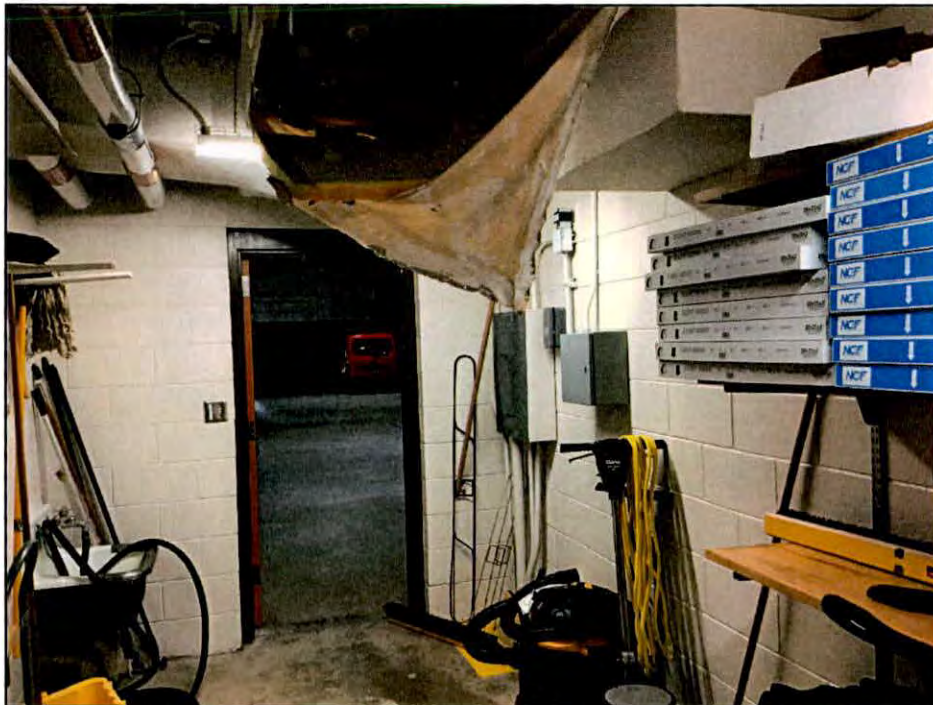
Photo 5.21. Representative storage room at the Beulaville Armory.
