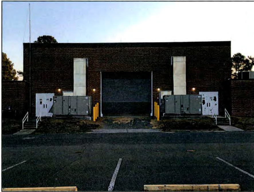
Figure 7.12. Set of double doors and a large garage door along the west elevation of the Butner Armory.
