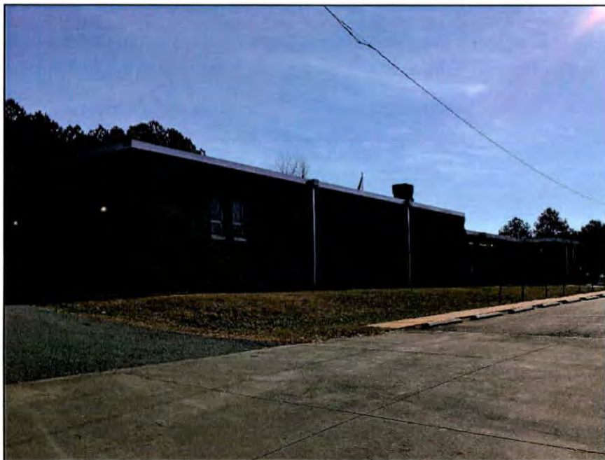
Figure 14.10. North elevation of the Youngsville Armory.
