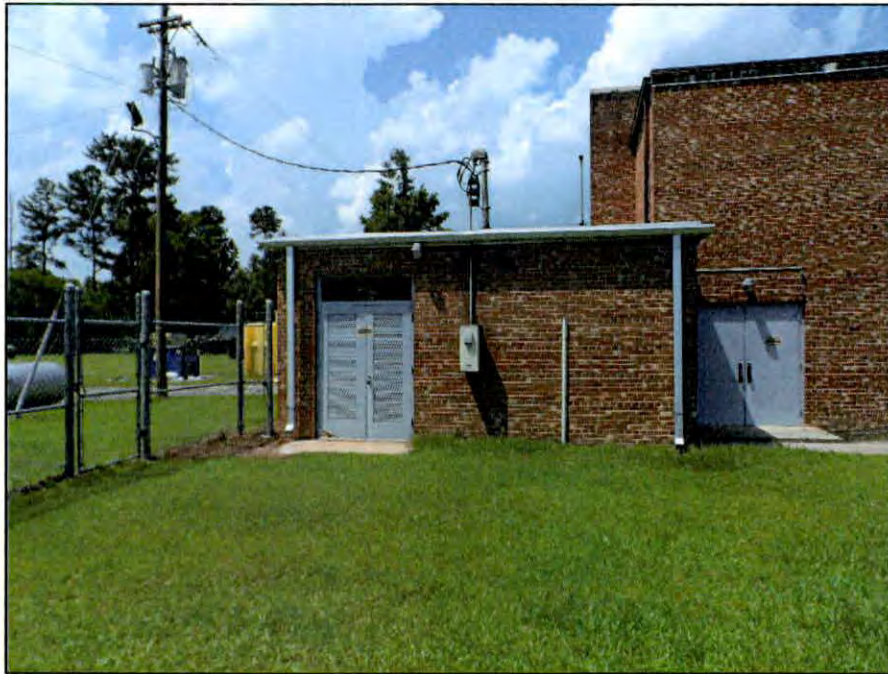
Photo 5.26. Original doors before replacement along the south elevation of the Beulaville Armory.
