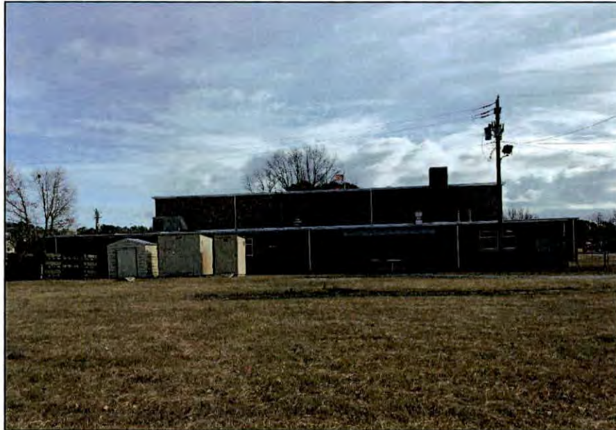
Photo 5.11. West elevation of the Beulaville Armory, facing east-southeast.
