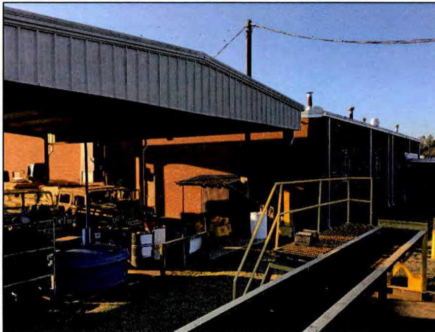
Figure 7.43. North and west elevations of the first shelter associated with the Butner Armory.
