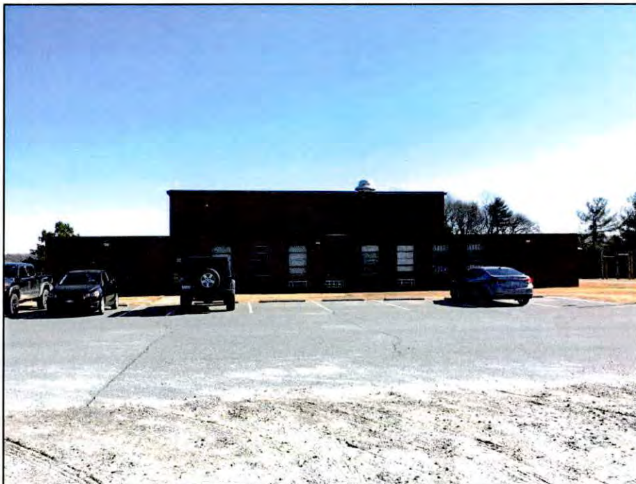
Figure 11.9. West elevation and parking lot of the Mocksville Armory.
