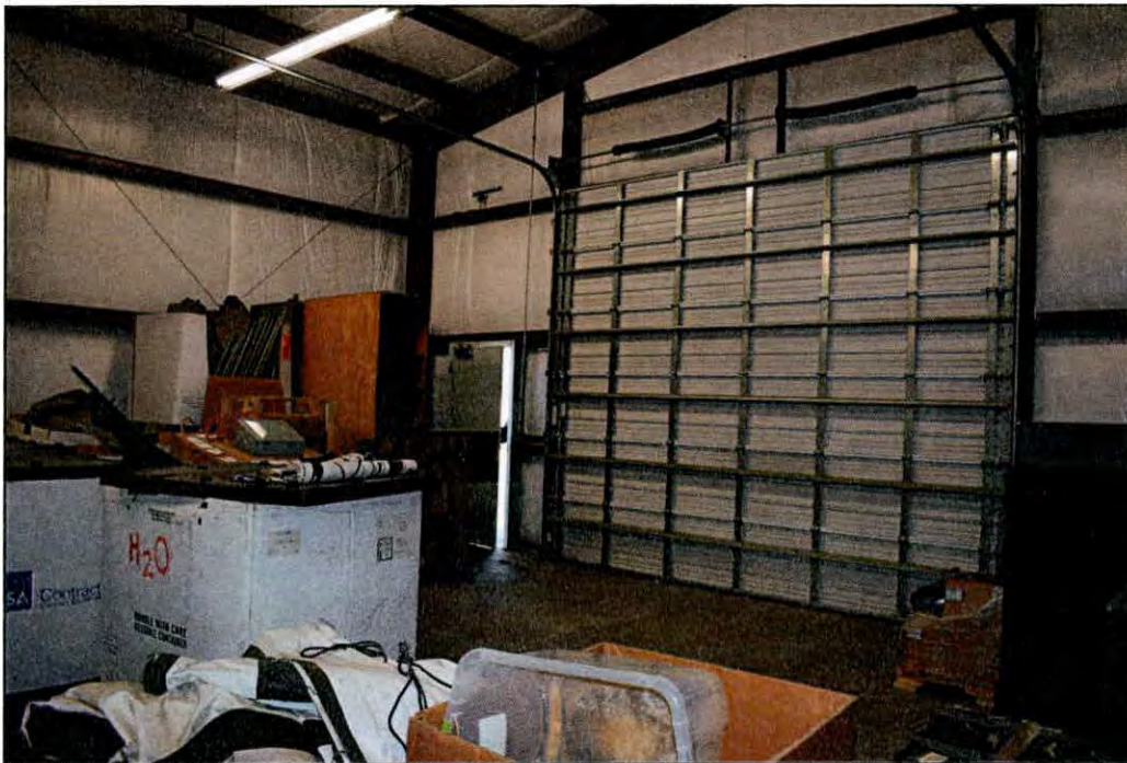
Figure 13.25. Interior of the Maintenance/Storage Building.
