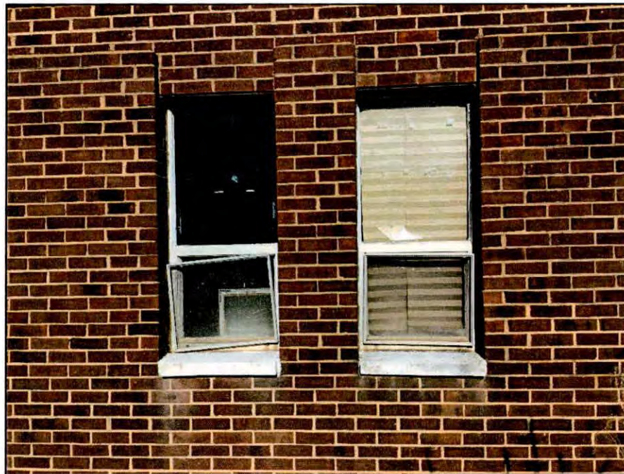
Figure 14.4. Example of windows along the one-story section of the south elevation of the Youngsville Armory.
