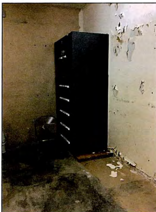
Figure 6.32. Vault Room at Boone Armory.
