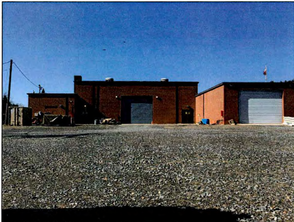
Figure 11.5. East elevation of the Mocksville Armory and motor pool.
