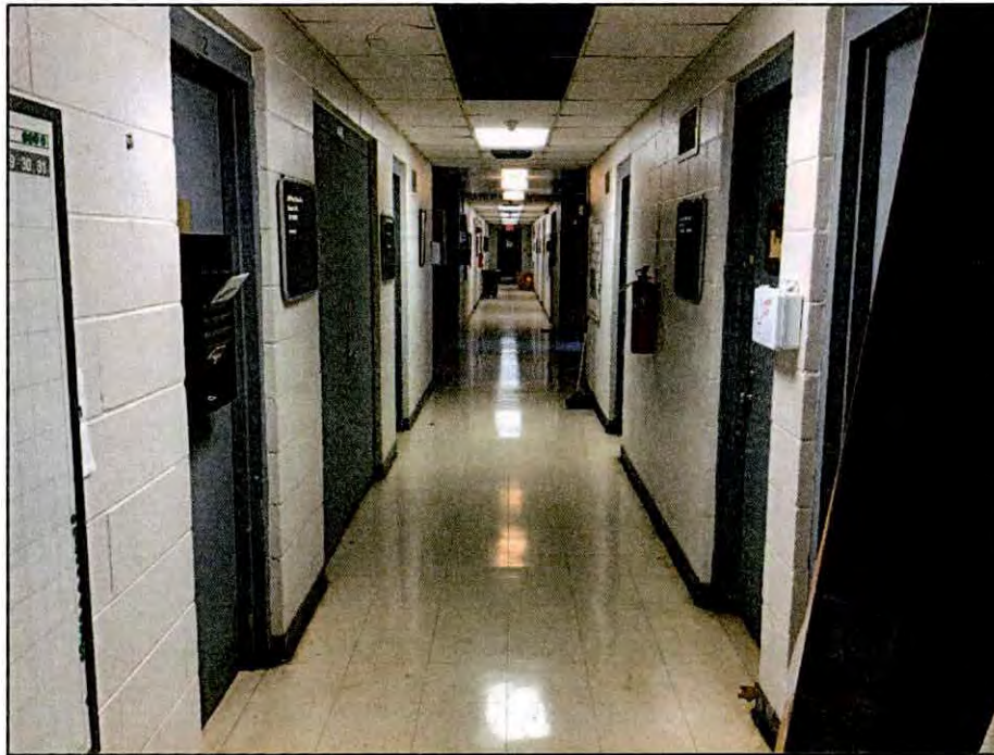
Figure 7.16. Representative corridor or hall at the Butner Armory.
