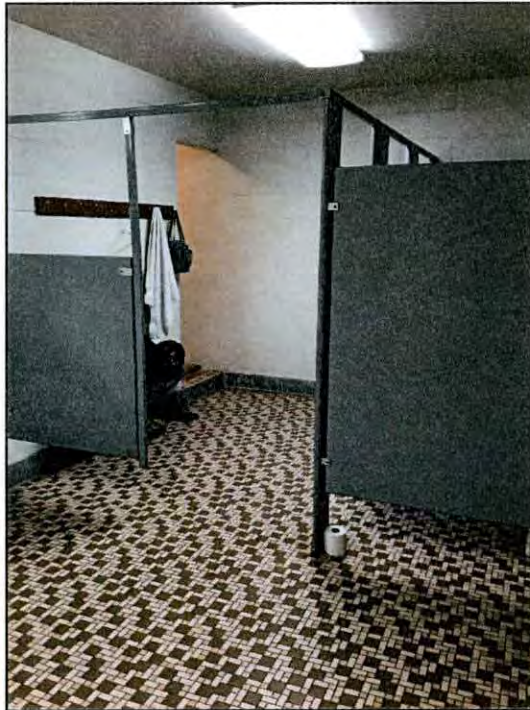
Figure 14.18. Representative bathroom/shower at the Youngsville Armory.
