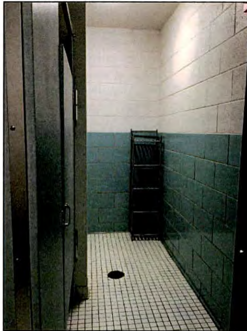
Figure 6.21. Representative restroom at the Boone Armory.
