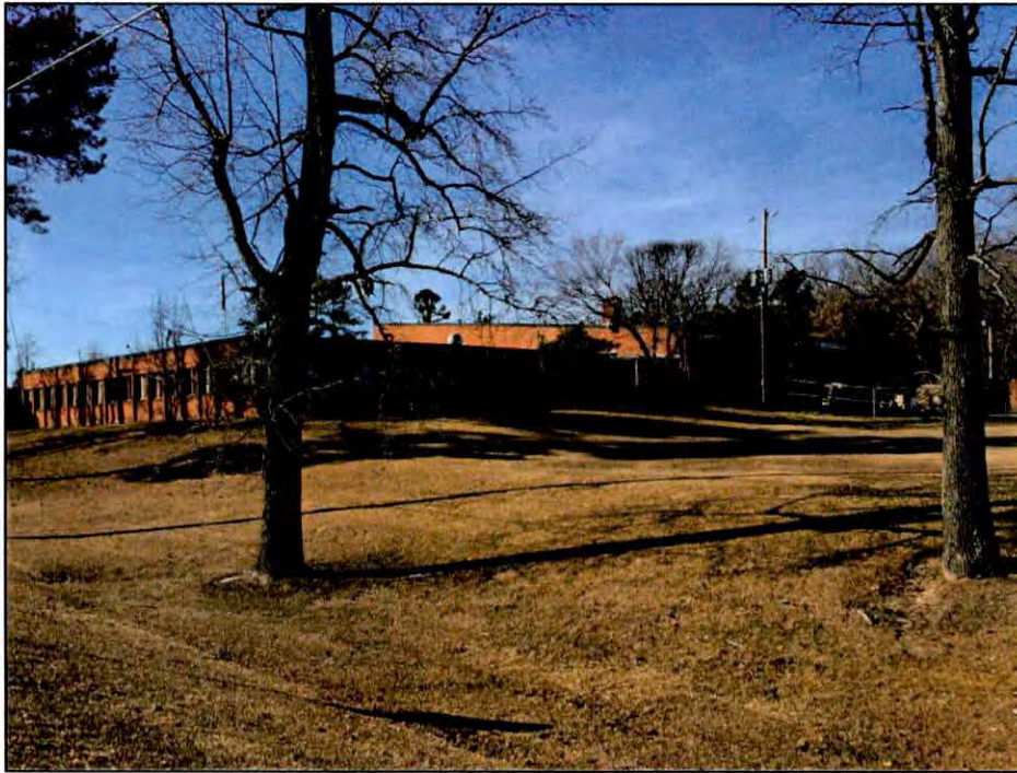
Figure 10.10. South and east elevations of the Louisburg Armory.
