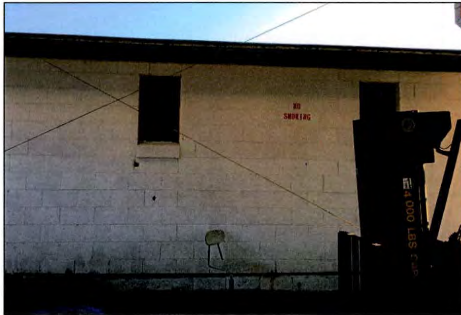
Figure 7.50. Windows along the west elevation of the fire repair building associated with the Butner Armory.
