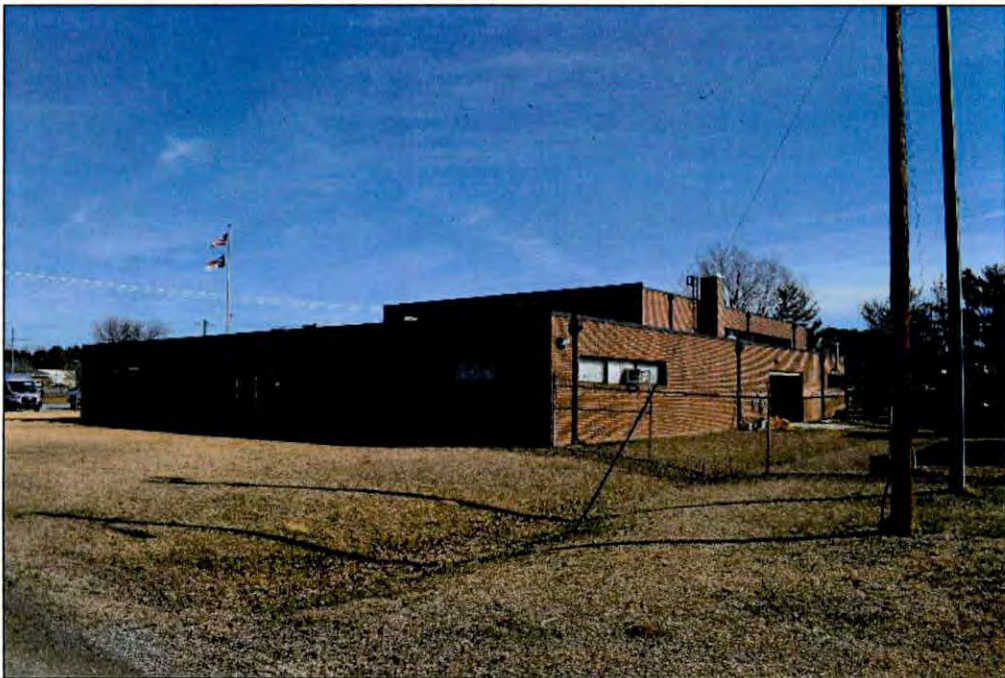
Figure 8.7. West and south elevations of the Dunn Armory.
