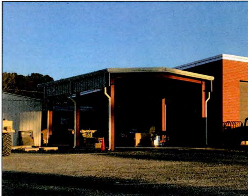
Figure 7.45. West and south elevations of the second shelter associated with the Butner Armory.
