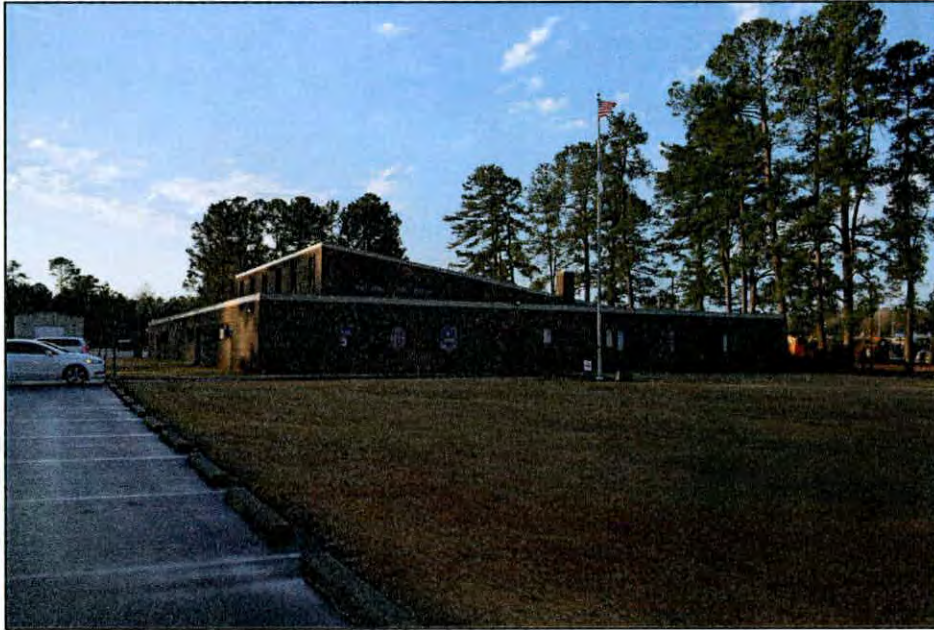
Figure 13.6. North and east elevations of the Whiteville Armory.
