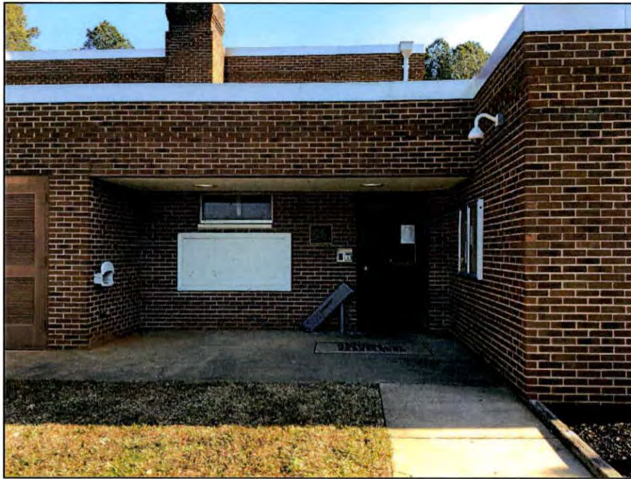
Figure 14.9. Recessed section along the west elevation of the Youngsville Armory.
