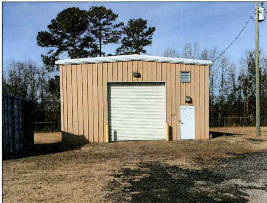
Photo 5.29. East elevation of the large storage building at the Beulaville Armory.
