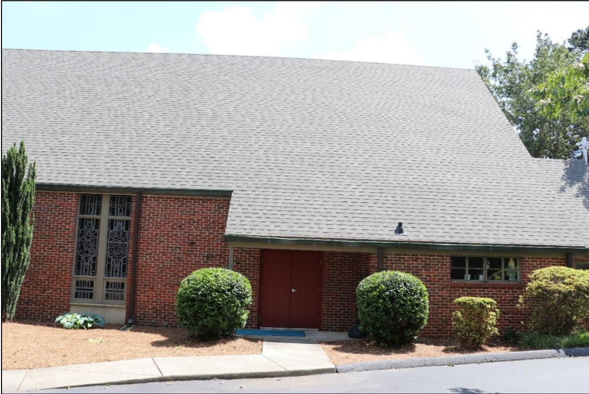
Figure 15: Church, sacristy entrance on the north elevation, looking south, 2024.
