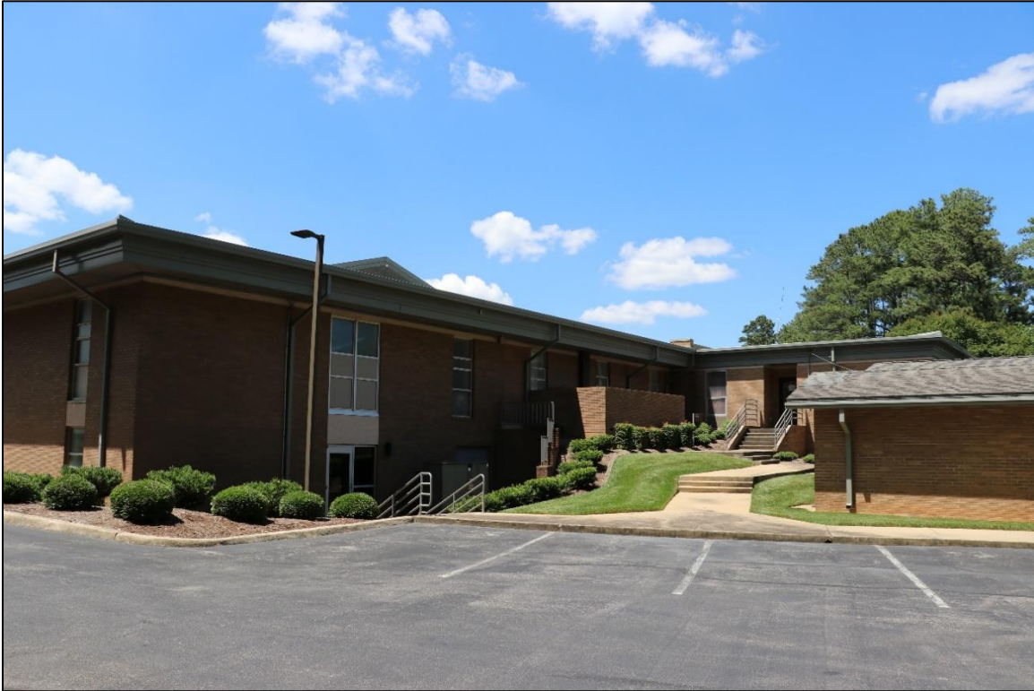
Figure 53: Church, east elevation, looking northwest, 2024 .
