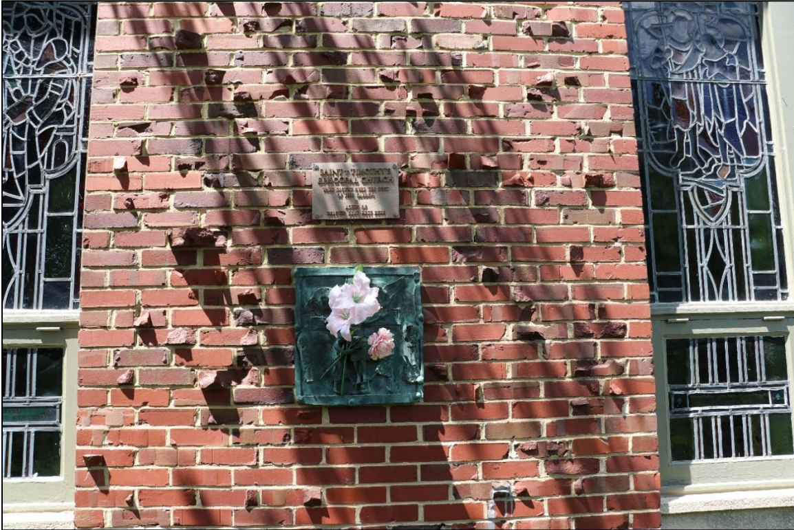
Figure 11: Church, detail view of the clinker brick construction and memorial garden plaque, looking north, 2024.
