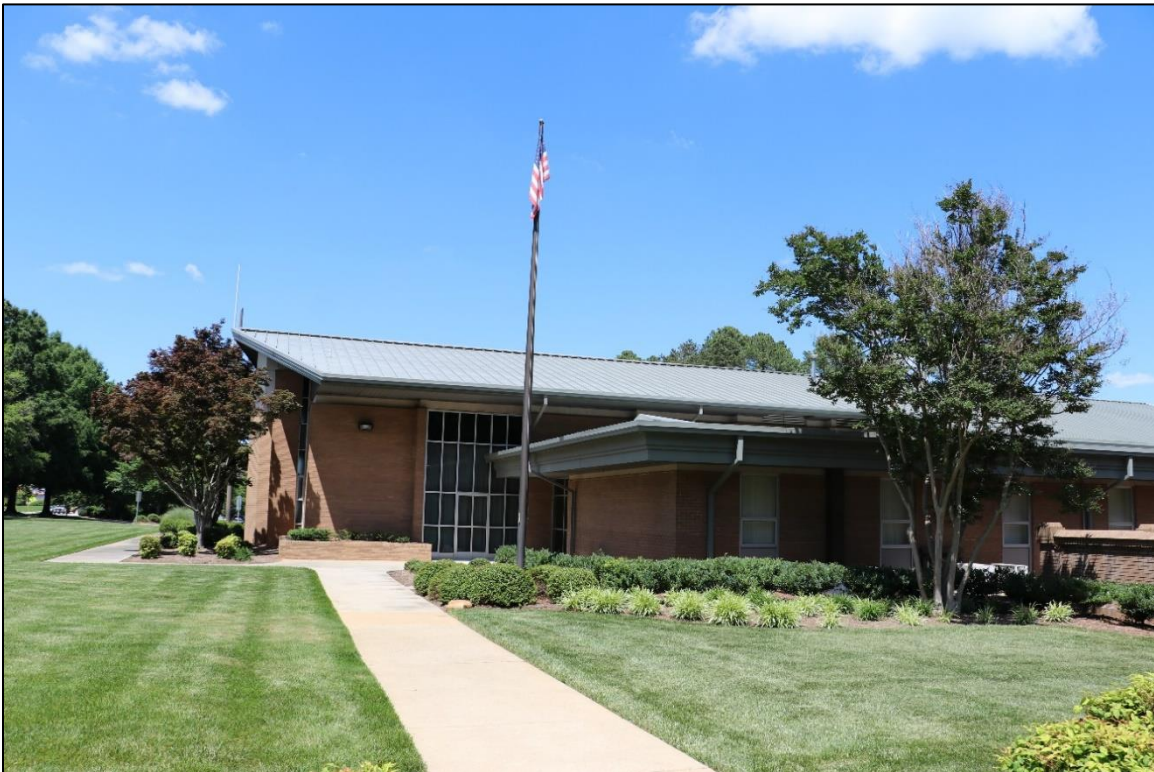
Figure 50: Church, partial south elevation, looking northeast, 2024.
