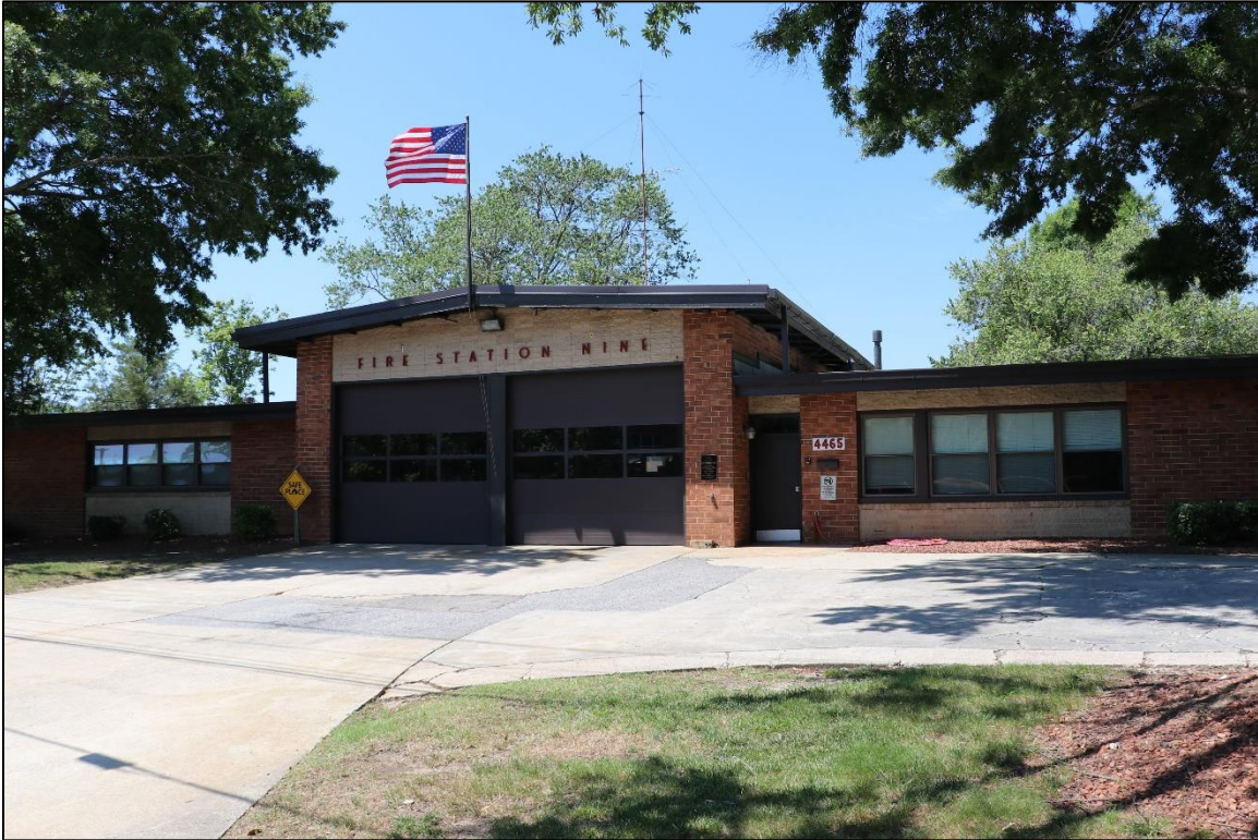
Figure 62: Raleigh Fire Station No. 9 (WA8813), east façade, looking southwest, 2024.
