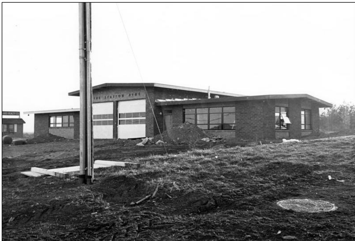
Figure 78: A January 31, 1963, construction photograph of Raleigh Fire Station No. 9. Source: The News and Observer from the Raleigh Fire Museum. Note the three-light windows.
