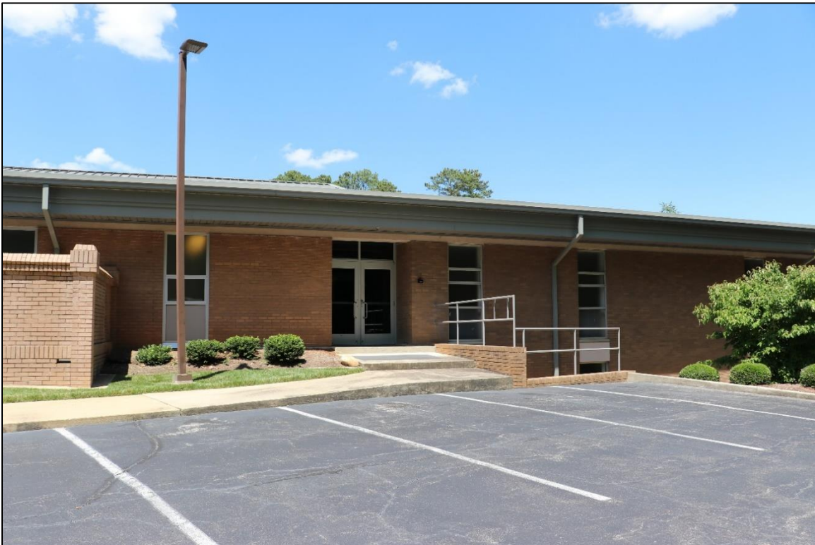
Figure 52: Church, partial south elevation, looking northeast, 2024.
