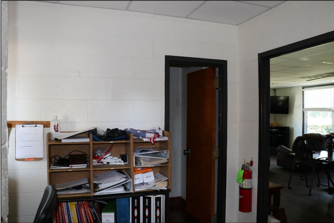
Figure 70: Raleigh Fire Station No. 9, open office space, looking into restroom (left) and lounge area (right), looking west, 2024.
