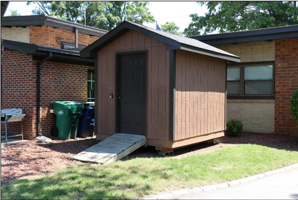
Figure 76: Raleigh Fire Station No. 9, Shed, looking northeast, 2024.
