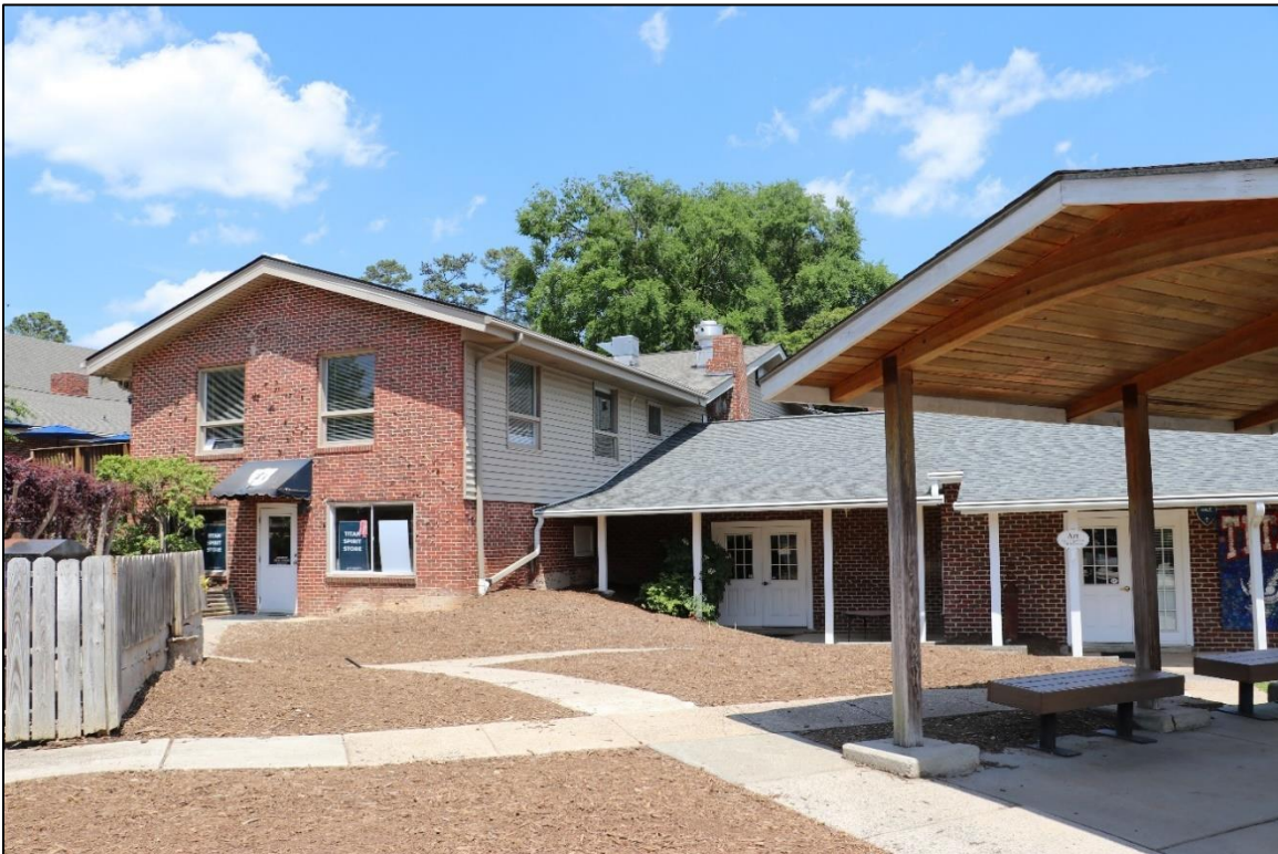
Figure 18: Parish Hall, west and south elevations (left) and Hale Hall, west façade (right), looking northeast, 2024.
