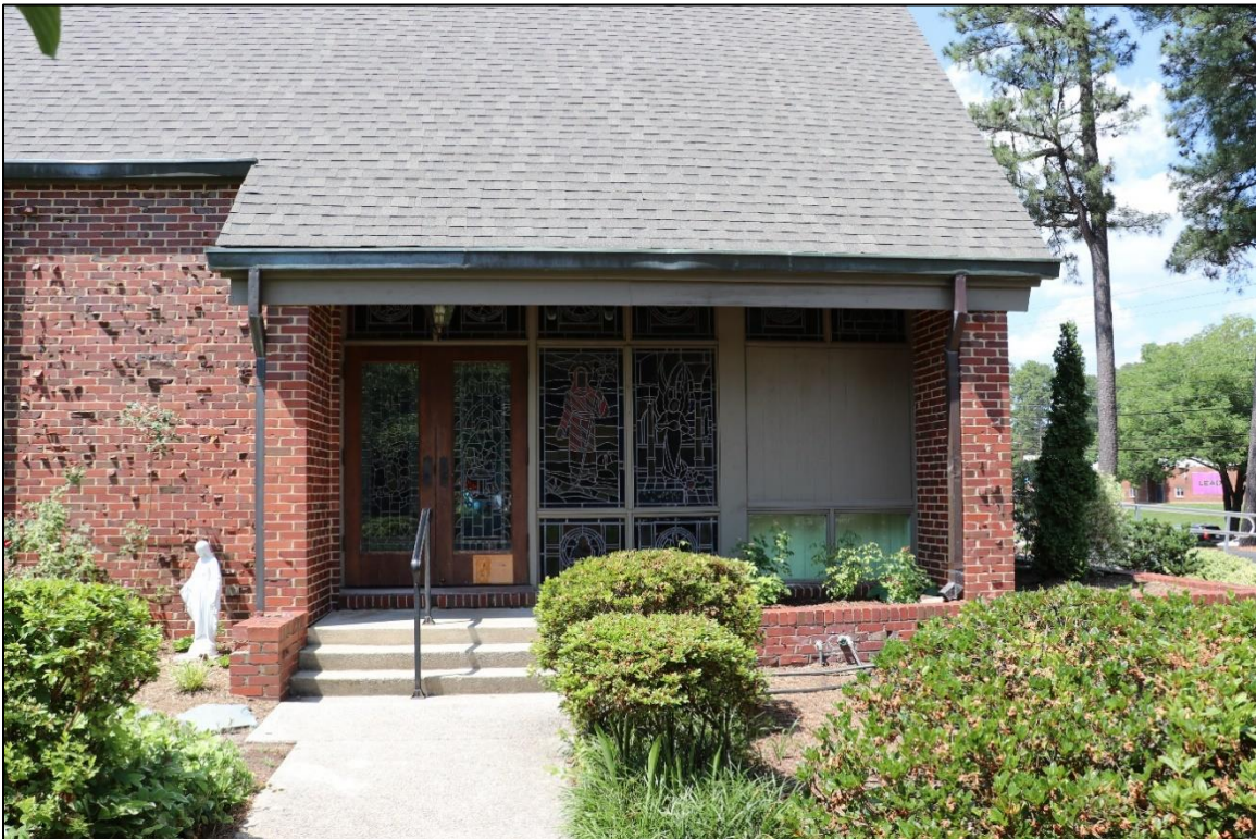
Figure 10: Church, south elevation entry, looking north, 2024.
