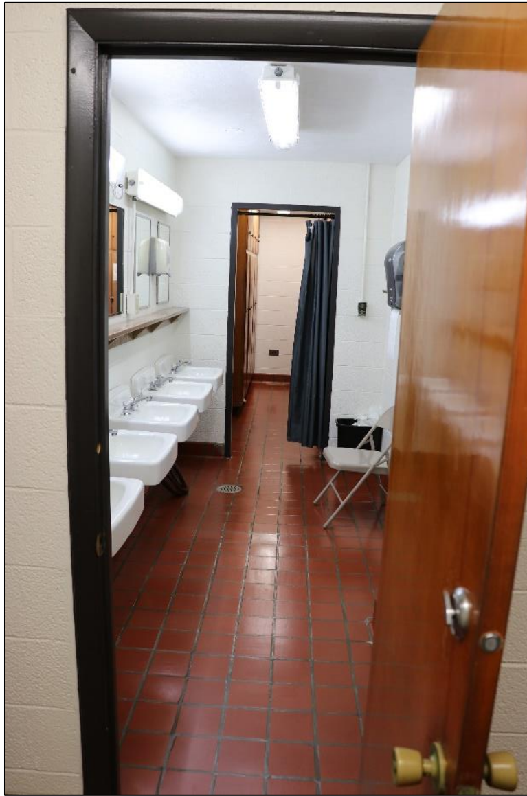
Figure 74: Raleigh Fire Station No. 9, room with showers and sinks, 2024. The locker room is through the door in the background, looking northwest.
