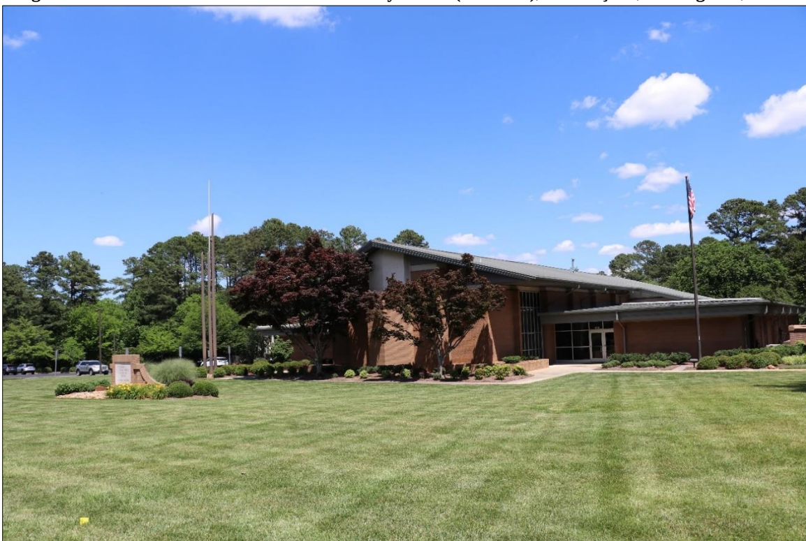
Figure 44: Church, west facade, looking northeast, 2024.
