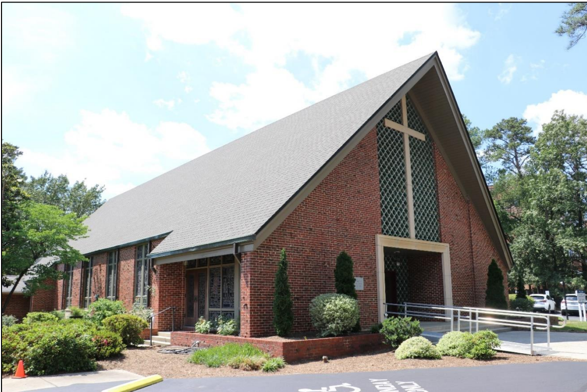
Figure 8: Church, south elevation and east façade, looking northwest, 2024.
