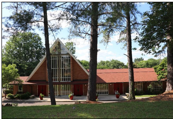
Figure 39: St. Ambrose Episcopal Church (WA8136), 813 Darby Road, Raleigh, North Carolina, 2024.
