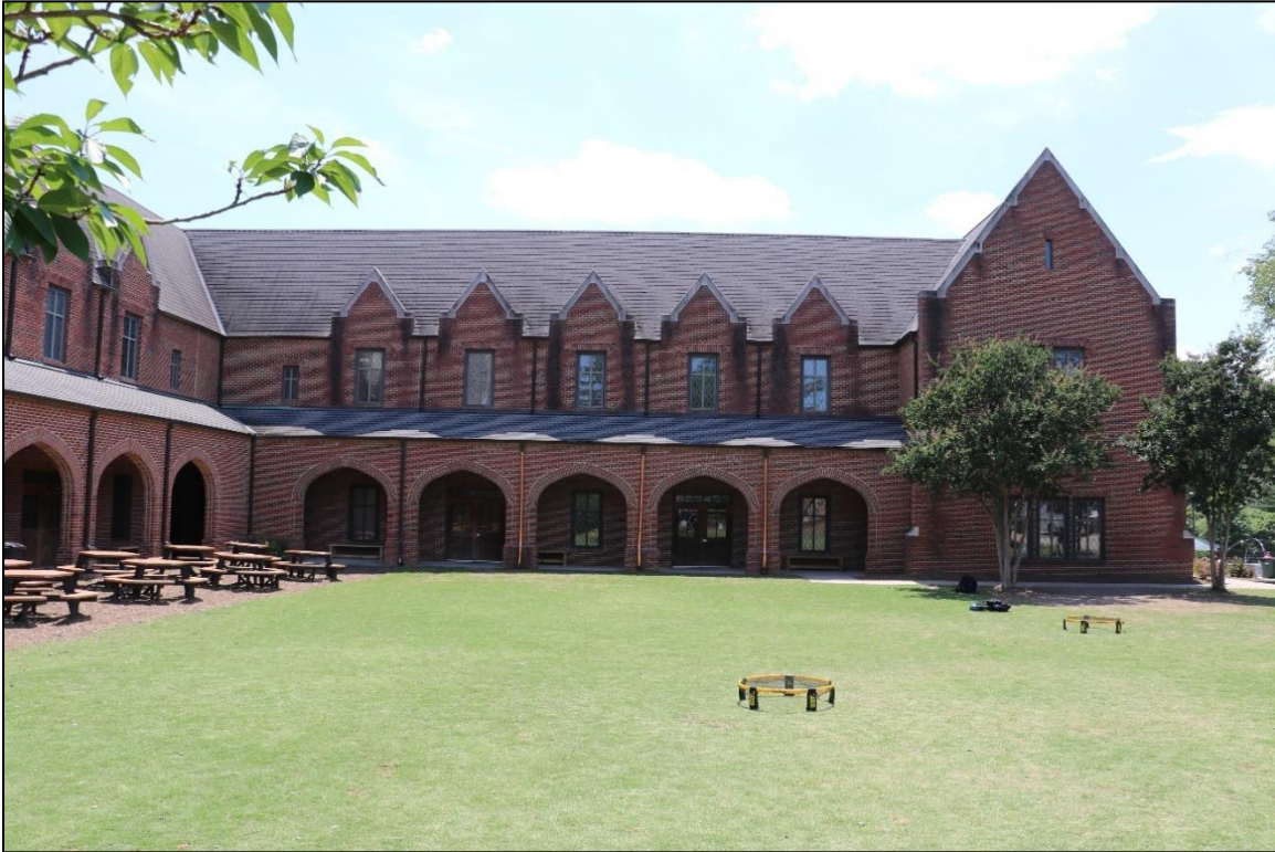
Figure 33: St. Timothy's Episcopal School, northwest (right) and northeast (left) elevations, looking southwest, 2024.
