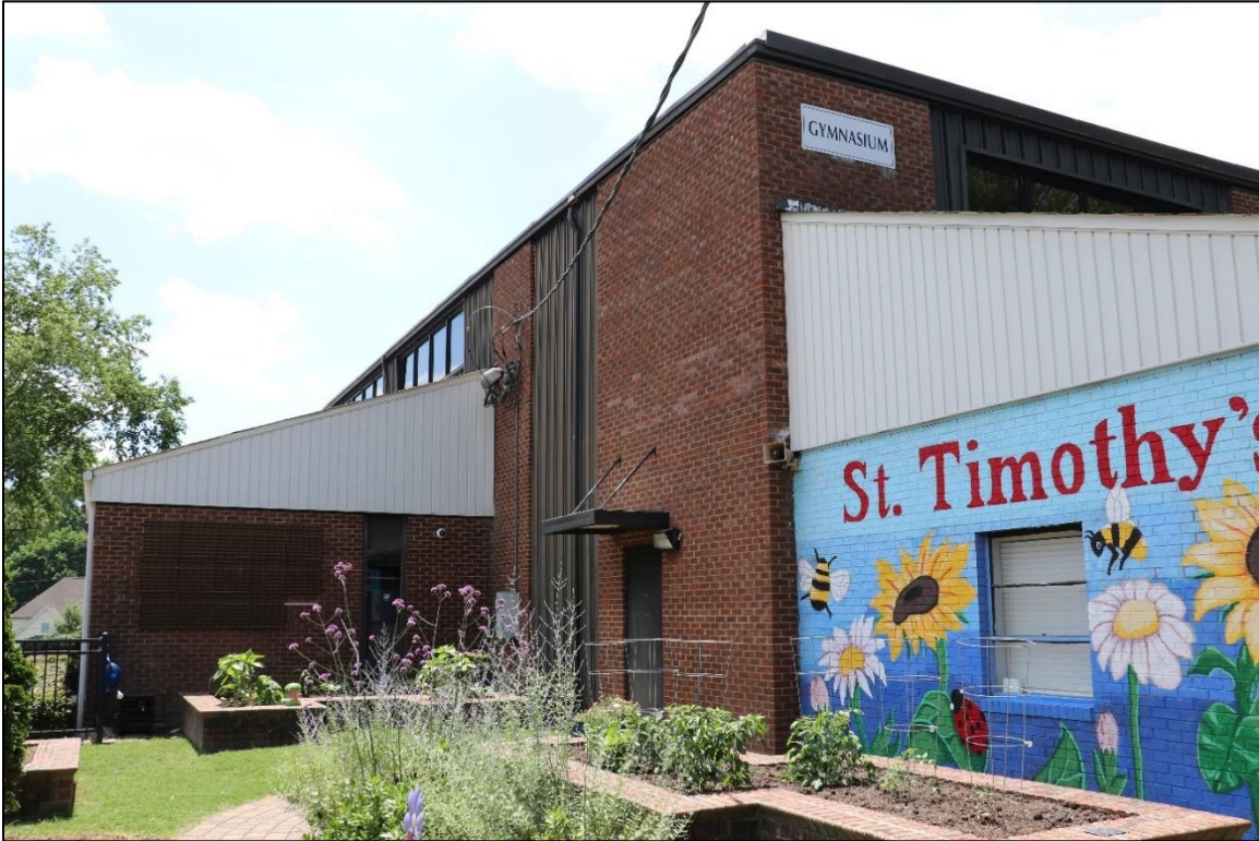
Figure 35: Gymnasium, southeast façade, looking west, 2024.
