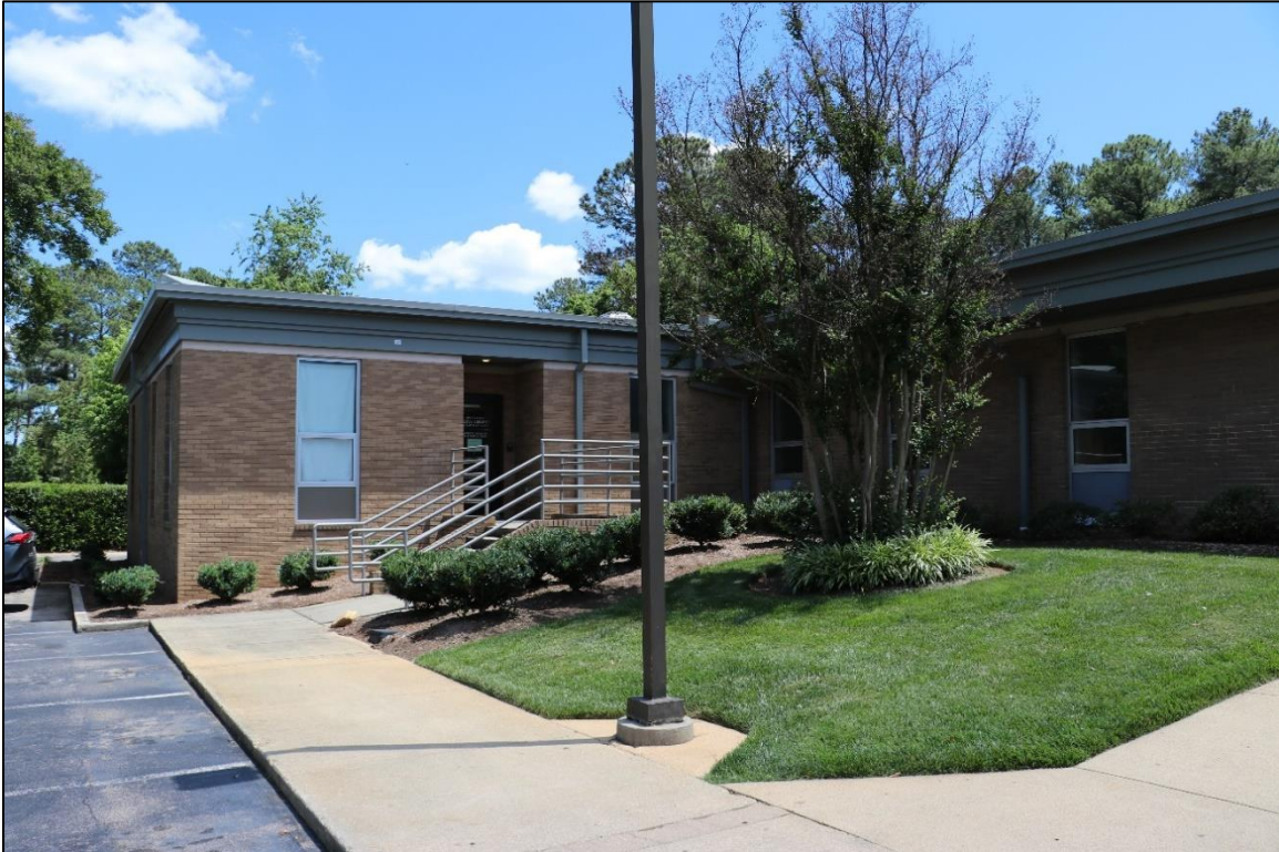
Figure 45: West elevation of Mission Office addition and north elevation of church, looking southeast, 2024.
