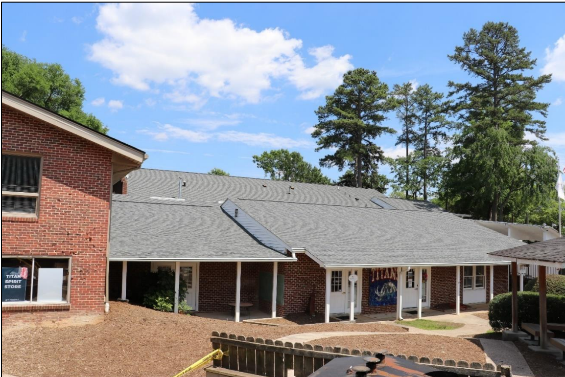
Figure 20: Hale Hall, west façade, looking southeast, 2024.
