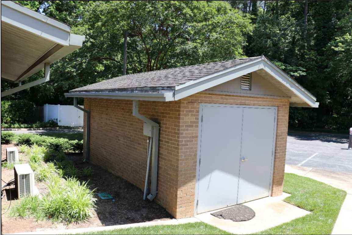
Figure 57: Storage Shed, north elevation and west façade, looking southeast, 2024.
