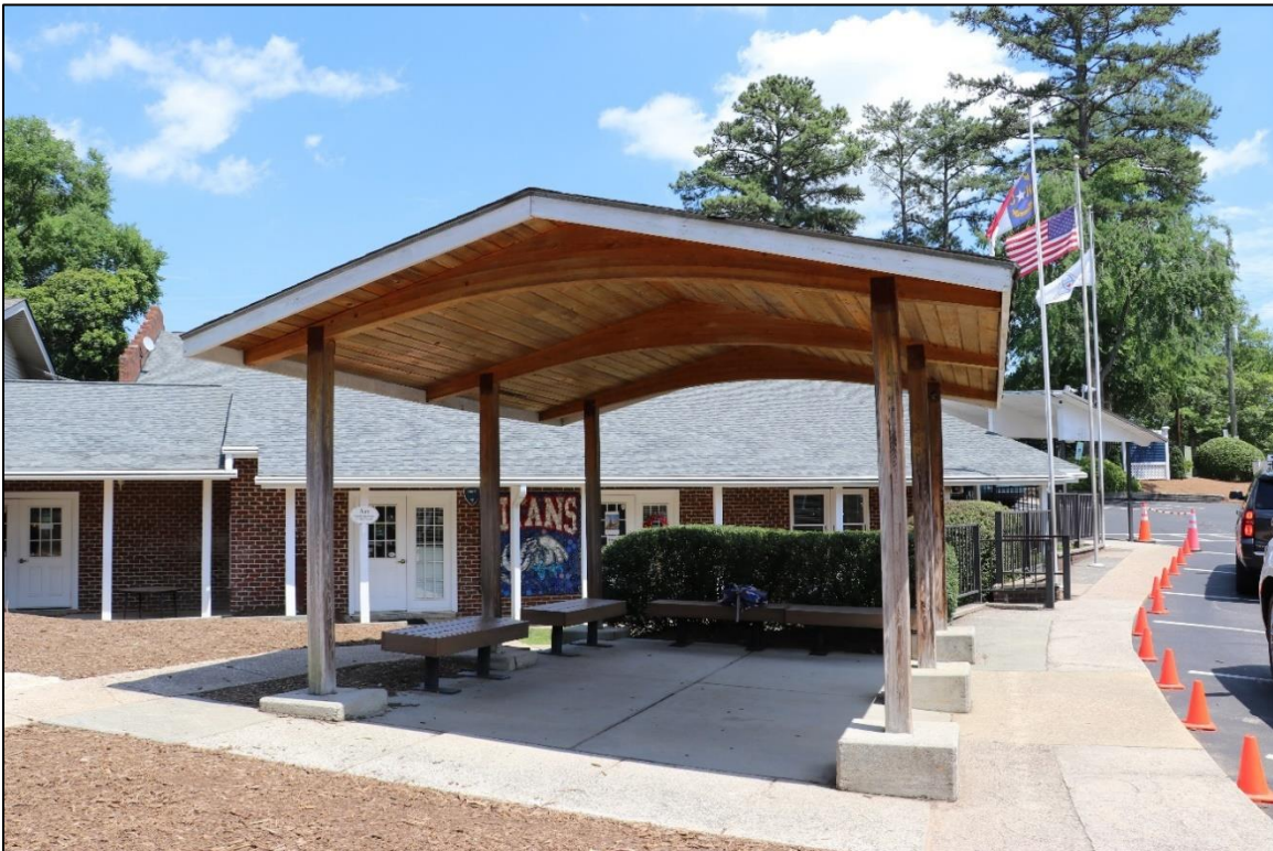
Figure 36: Pavilion west of Hale Hall (background), looking southeast, 2024.
