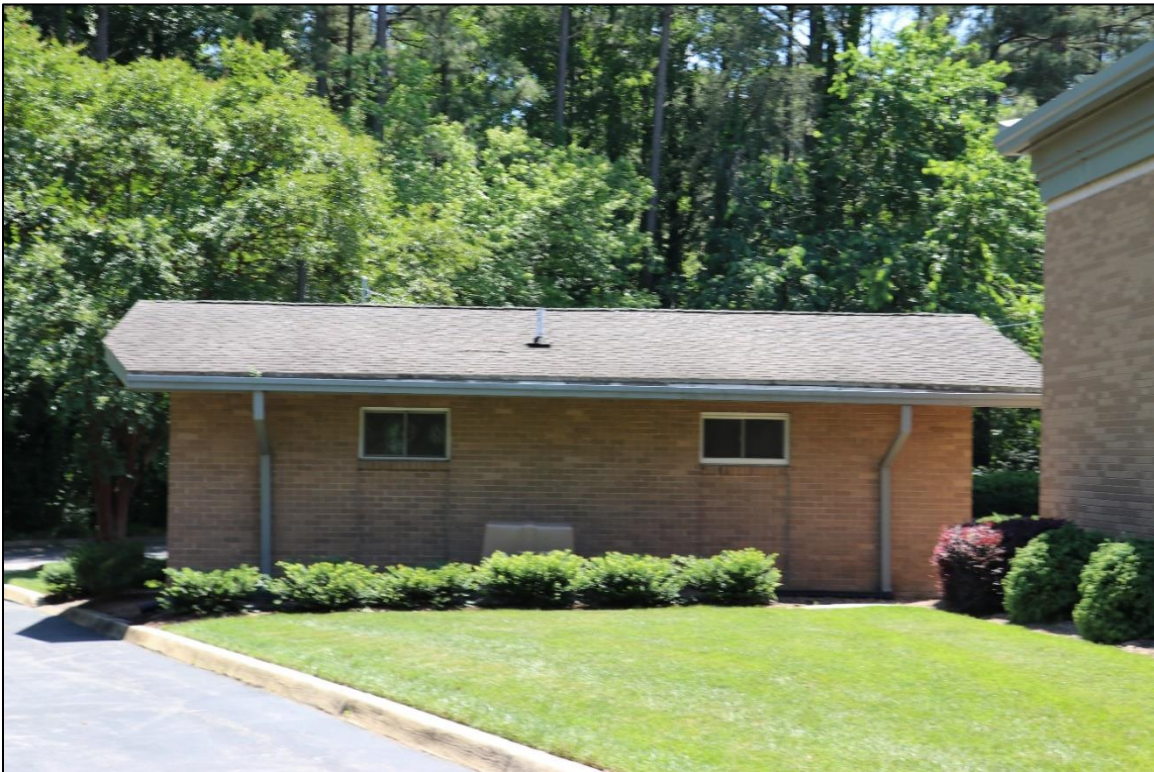
Figure 56: Facilities Management Office, north elevation, looking southwest, 2024.
