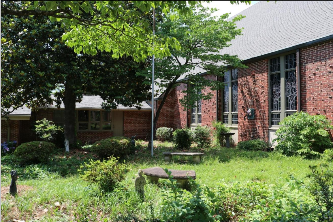
Figure 9: East elevation of the hyphen and south elevation of the church, looking northwest, 2024. The memorial garden is in the foreground.
