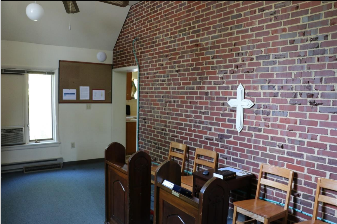
Figure 26: Church, 1990 portion of the sacristy and original west wall of the sanctuary, looking northeast, 2024.
