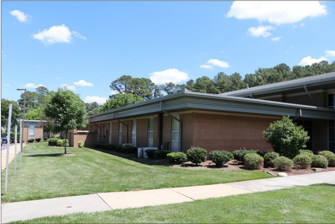
Figure 47: Church, north elevation and west façade, looking southeast, 2024.
