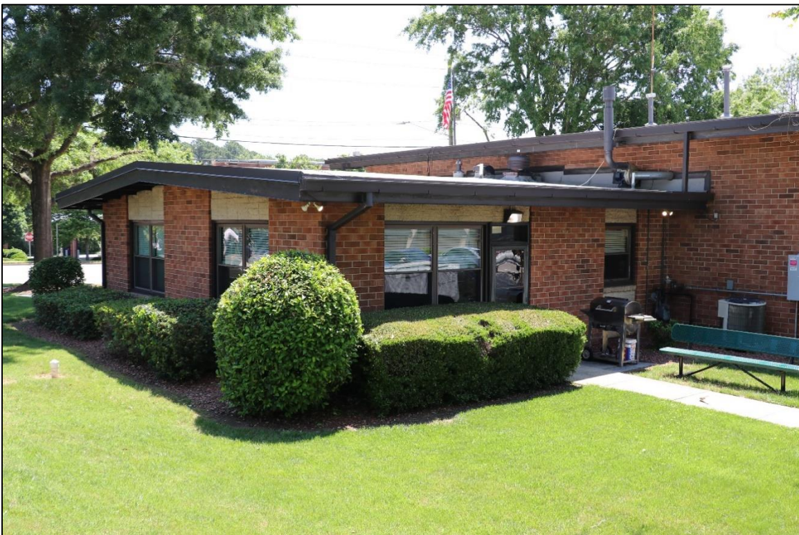
Figure 67: Raleigh Fire Station No. 9, north and west elevations, looking southeast, 2024.
