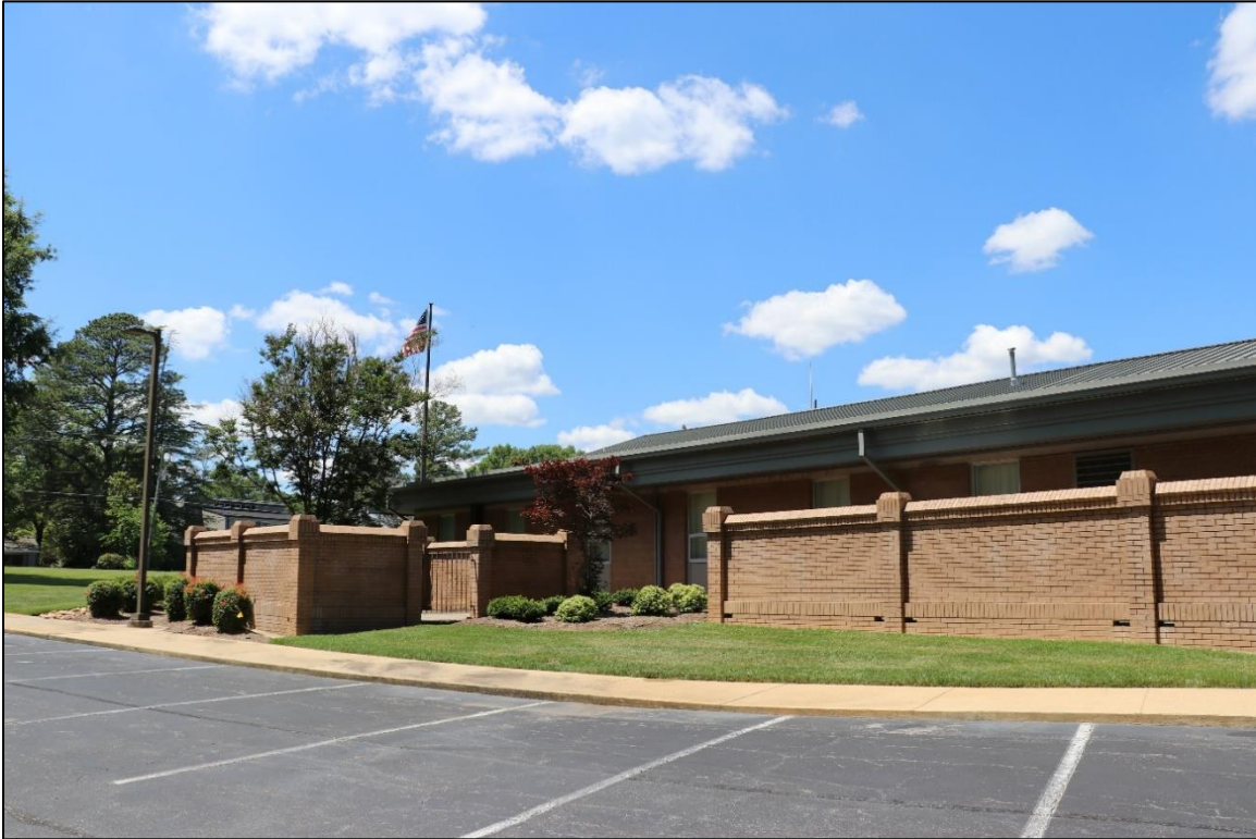
Figure 51: Church, partial south elevation, looking northwest, 2024.
