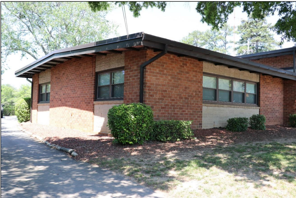
Figure 65: Raleigh Fire Station No. 9, south elevation and east façade, looking northwest, 2024.
