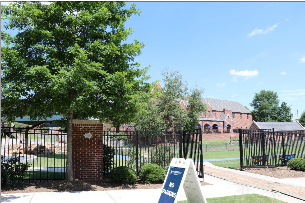
Figure 34: St. Timothy's Episcopal School, southwest elevation, looking northeast across the sports field, 2024.
