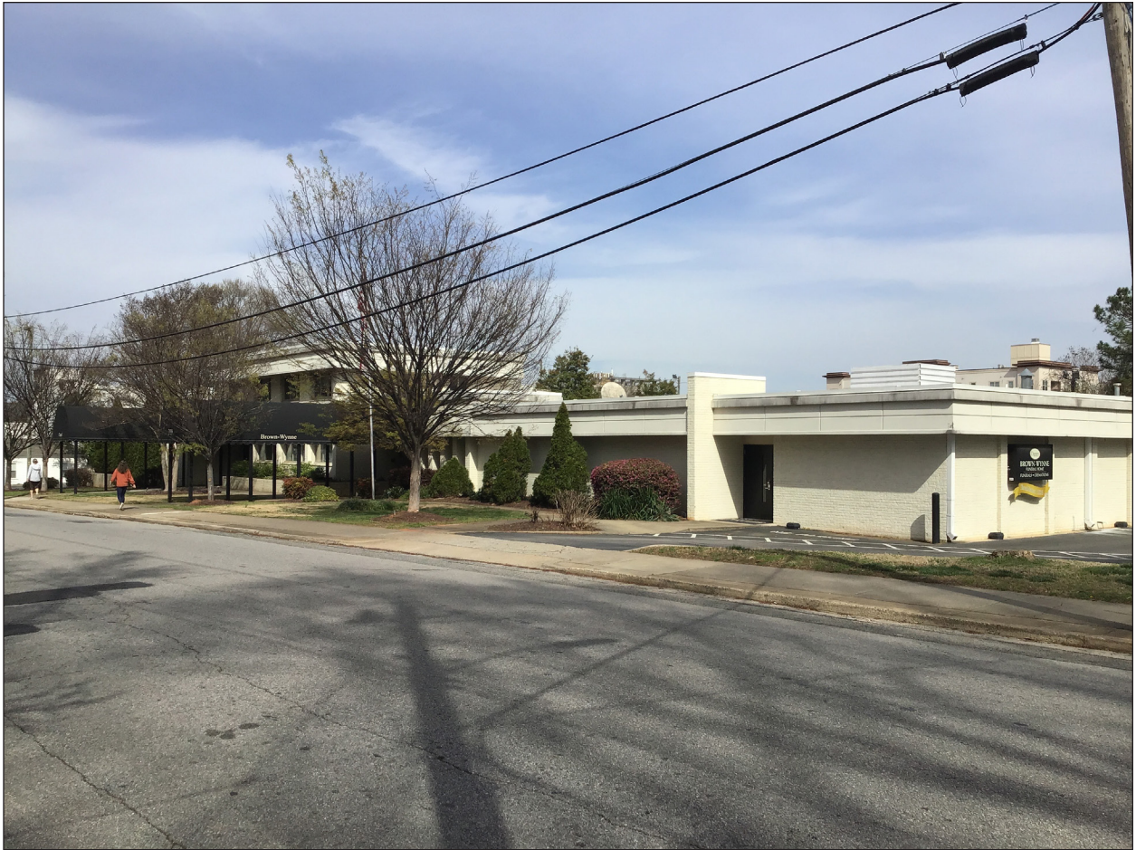
Figure 5.9. Brown-Wynne Funeral Home (WA8034), Facing Northeast
