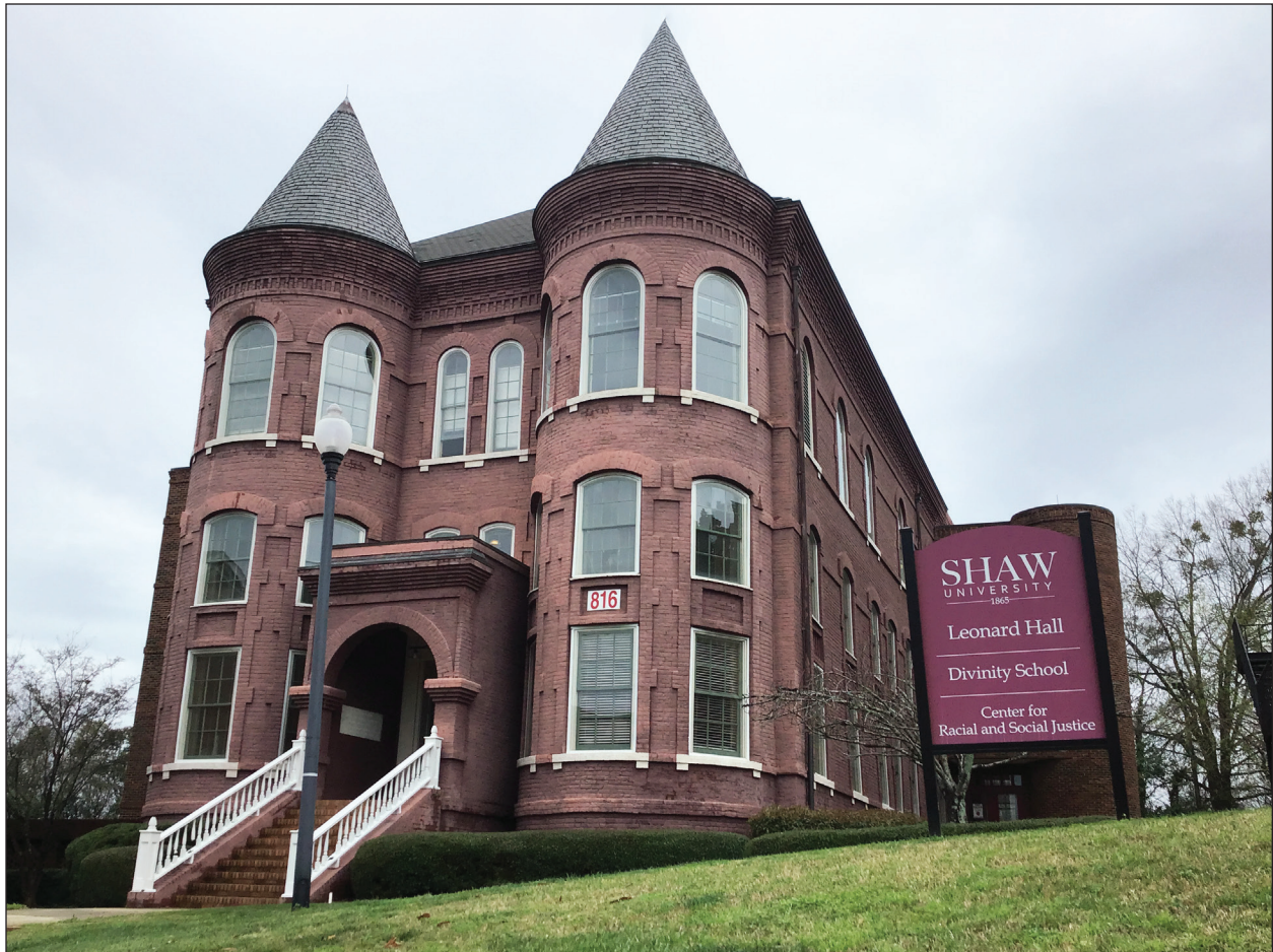
Figure 4.4. Leonard Hall (WA2396), Facing Southwest
