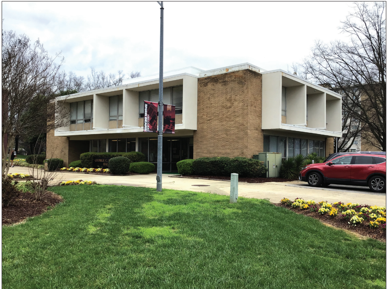
Figure 4.8. Administration Building (WA8073), Facing Northeast
