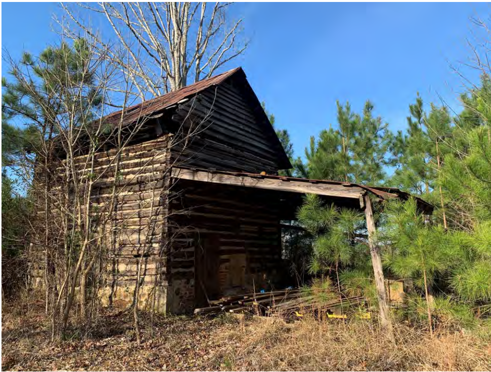
Plate 2.26: Log tobacco barn with stone foundation at the Excel and Elsie Green Farm (WA7194) in Cary near the Durham County border (Heckendorf 2022).
