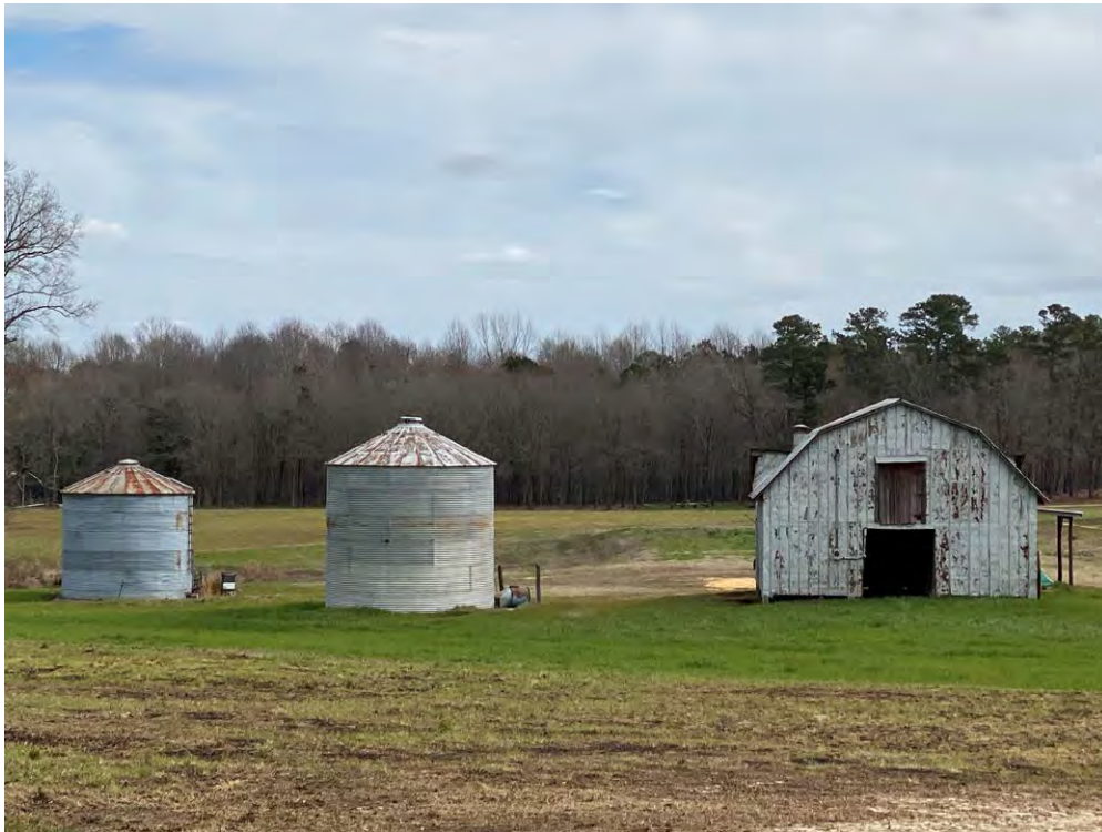
Plate 2.25: Corrugated metal grain bins at the Ogburn-Honeycutt Farm (WA1142) in Fuquay-Varina (Heckendorf 2022).
