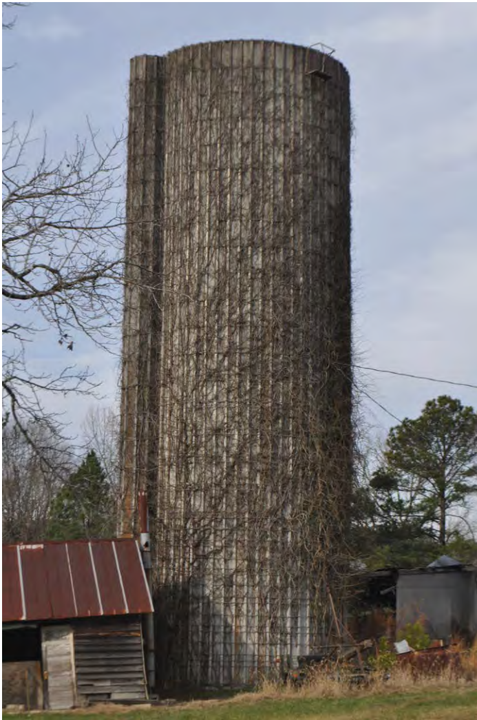
Plate 2.20: This tall, durable concrete stave silo constructed of interlocking masonry units reinforced by metal bands is located on the Harvey Ragan House (WA1070) property (Heckendorf 2022).
