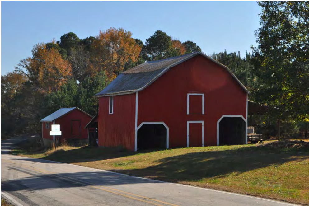
Plate 2.19: The large, gambrel roof barn at the Mills Farm and Store (WA1004) in Green Level has livestock stalls below with plentiful hay storage space above (Heckendorf 2021).
