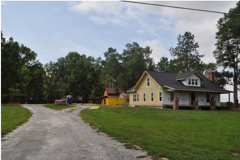
Plate 3.6: The Bowden-Hicks Farm (WA4180) east of Rolesville has been substantially altered through a complete gutting of the farmhouse and the loss of associated outbuildings (Heckendorf 2021).
