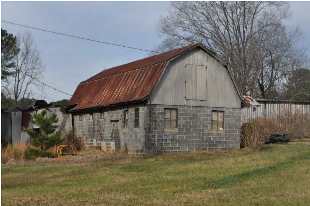
Plate 2.18: The gambrel roof barn at the Harvey Ragan House (WA1070) west of Apex has concrete block walls and industrial metal sash windows which met new standards for sanitation (Heckendorf 2022).
