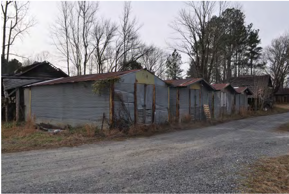
Plate 2.31: Four older bulk curing barns on the James E. Ragan Farm (WA1071) west of Apex (Heckendorf 2022).
