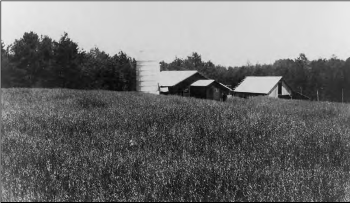
Figure 2.10: Silo and barns at the Sion Williams Farm in Raleigh in 1933 (North Carolina State University 1933).
