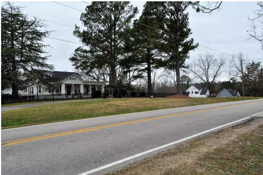
Plate 3.5: The integrity of the B.A. Weathers House and Farm (WA1928) in Knightdale has been compromised by alterations to the house, the demolition of outbuildings, and the construction of new, single-family homes on its former farmland (Heckendorf 2022).
