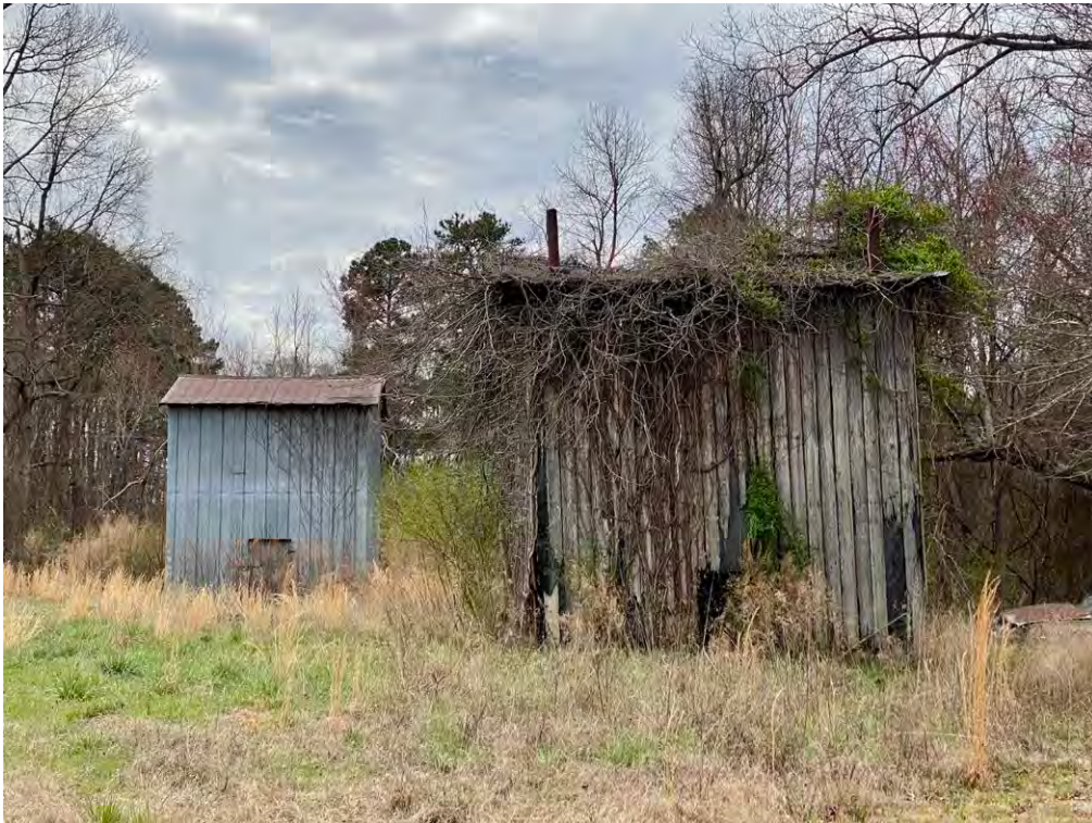
Plate 2.27: Frame tobacco barns like these at the Coley-Howard Farm (WA1124) in Willow Springs were promoted in the mid-twentieth century as an improvement over log construction. They are frequently clad with metal over their original wood plank siding (Heckendorf 2022).
