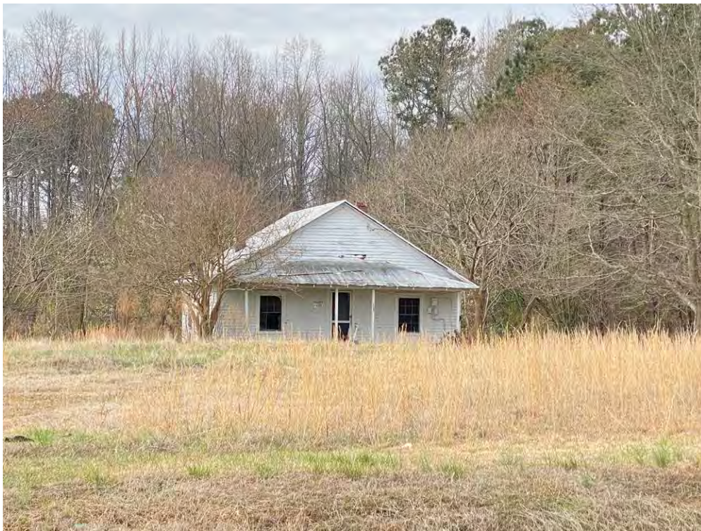
Plate 2.6: Typical tenant house at the J.R. Fowler Farm (WA1840) in the Fowler's Crossroads Community southeast of Rolesville (Heckendorf 2022).
