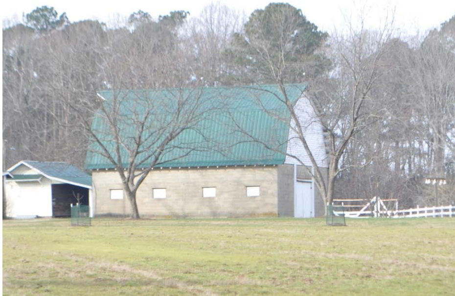
Plate 2.10: Concrete block gambrel-roofed barn at the Allie Lawrence Farm (WA1097) in New Hill (Heckendorf 2022).
