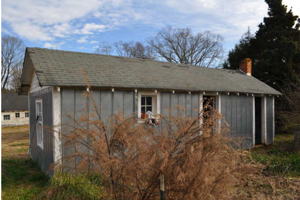
Plate 2.17: The milk house at the Dr. L.J. Faulhaber Farm (WA4811) south of Garner is an example of a specialized outbuilding used by dairy farmers to chill, store, bottle, and ship their products (Heckendorf 2021).
