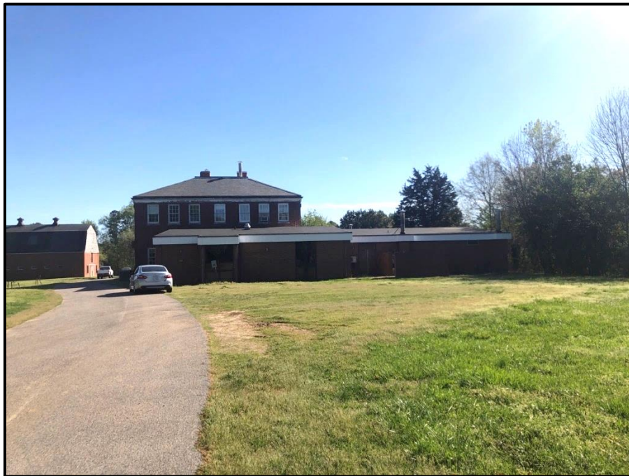
Figure 8 State Laboratory of Hygiene Farm's Main Laboratory Building, Looking South.
