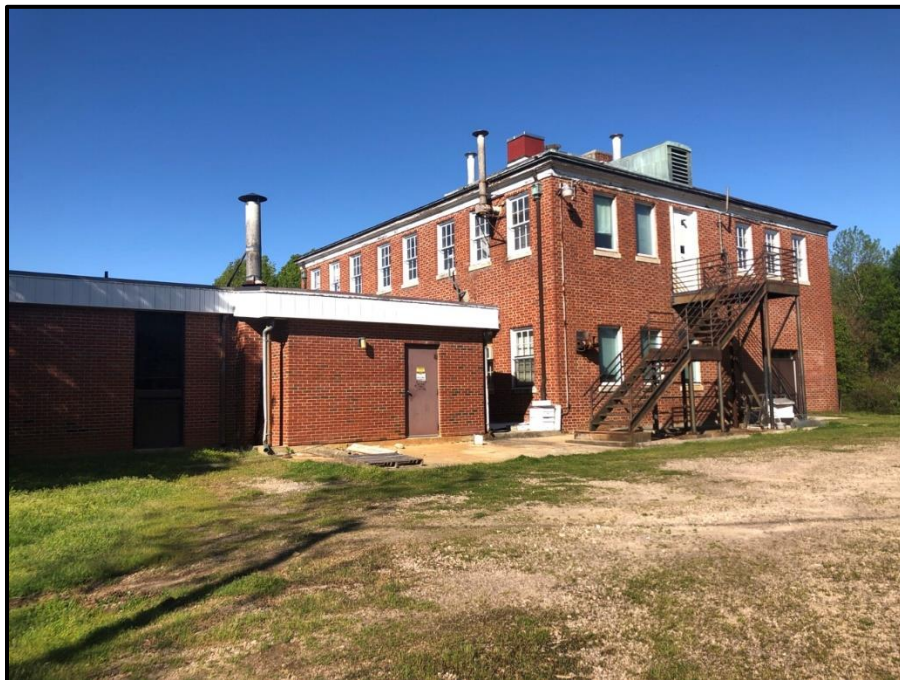
Figure 12 State Laboratory of Hygiene Farm's Main Laboratory Building, Looking Northeast.
