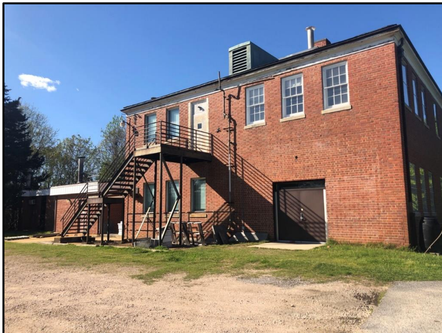
Figure 10 State Laboratory of Hygiene Farm's Main Laboratory Building, Looking Northwest.
