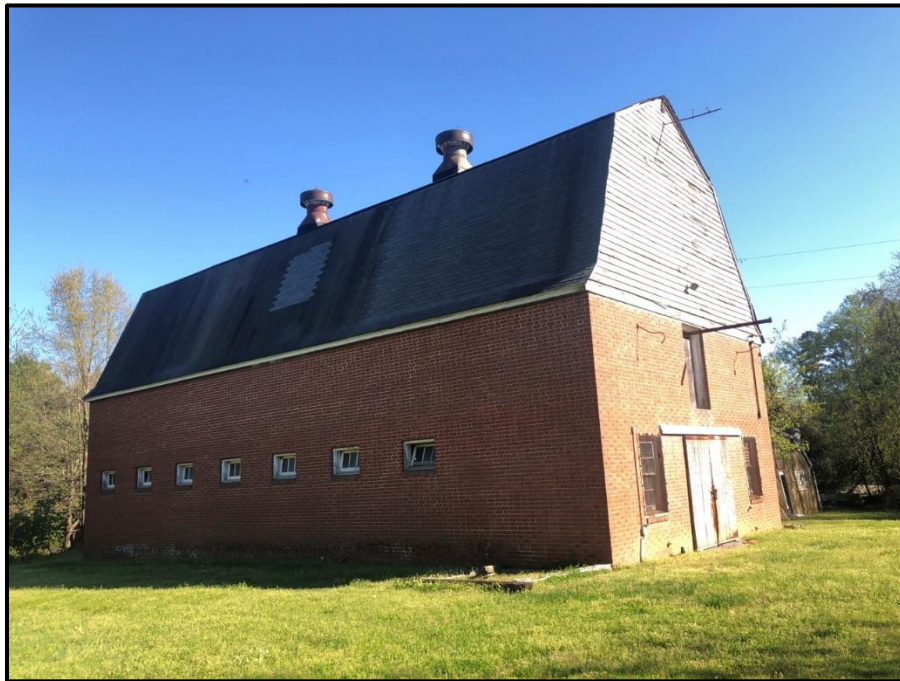
Figure 13. Barn, Looking Southeast.
