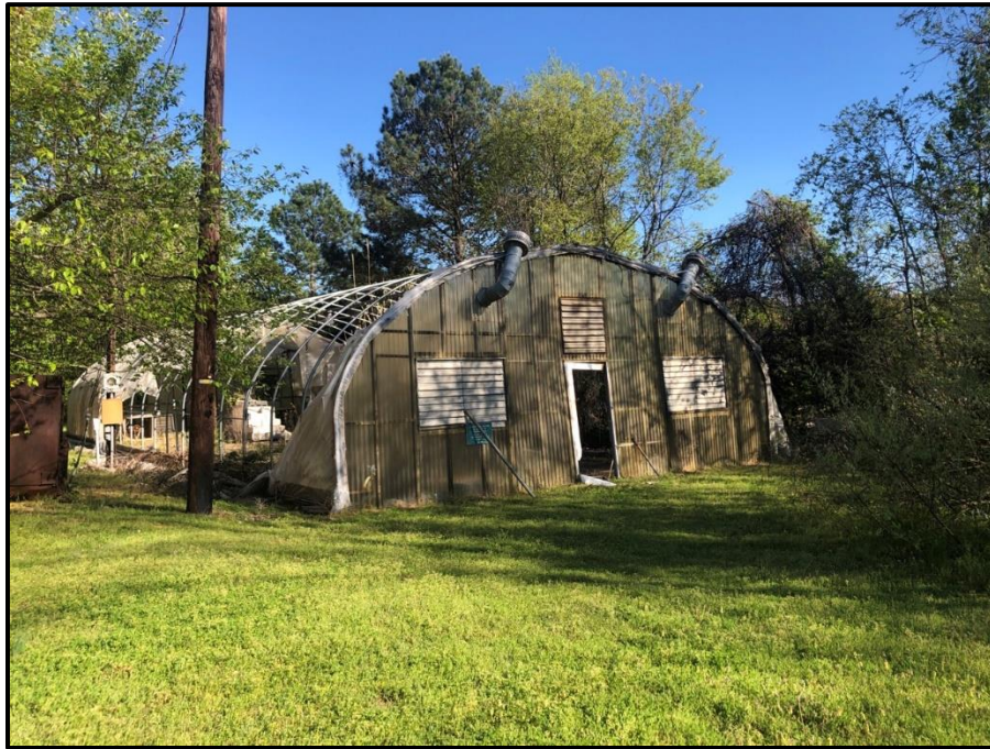
Figure 17 Greenhouse 3, Looking Southeast.
