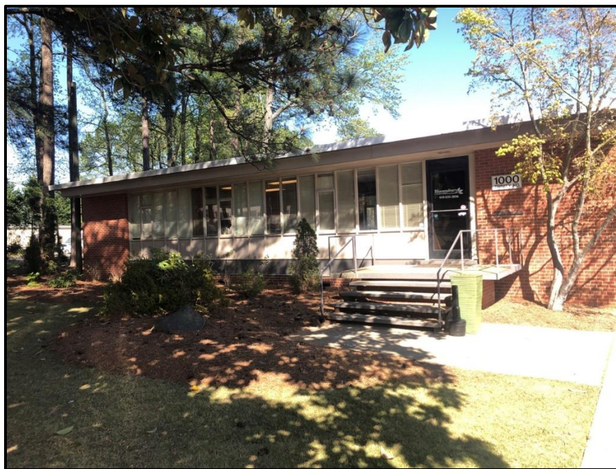
Figure 3 Commercial Building (WA6438), 1000 Trinity Road, Looking Northeast.
