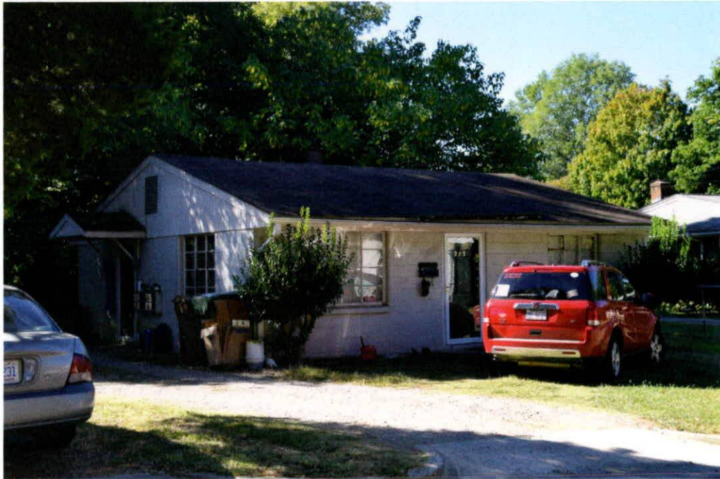
Concrete-block, side-gabled Ranch house with metal casement windows and plywood in gable ends.
