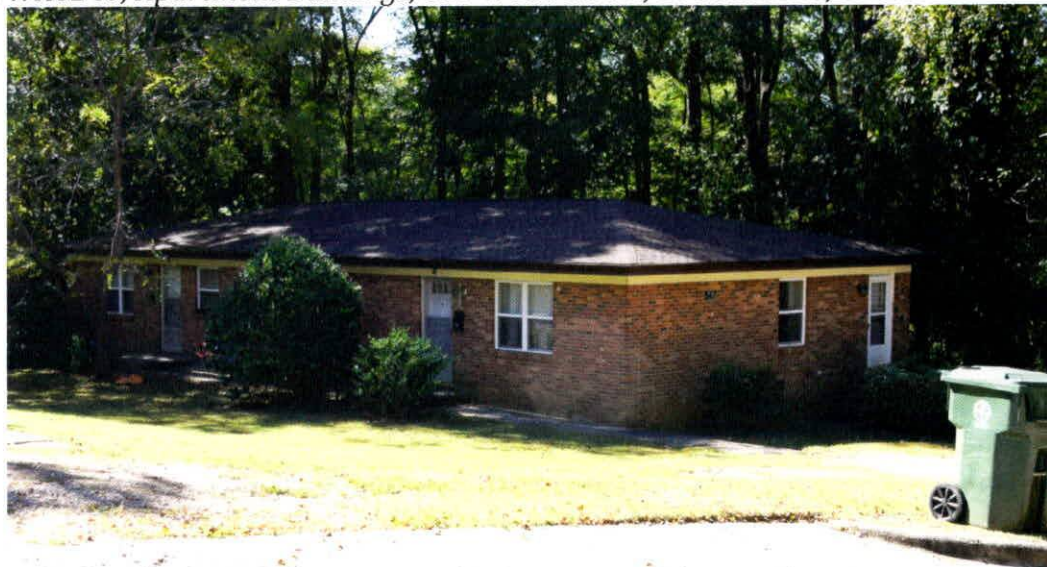
36. WA8240, Apartment Buildings, 539 Wood Street, 0764228161, 1968.
