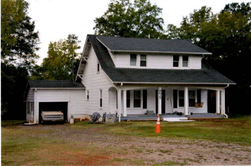
53. WA7321, House, 8635 Chapel Hill Road, 0764332193, 1938.
