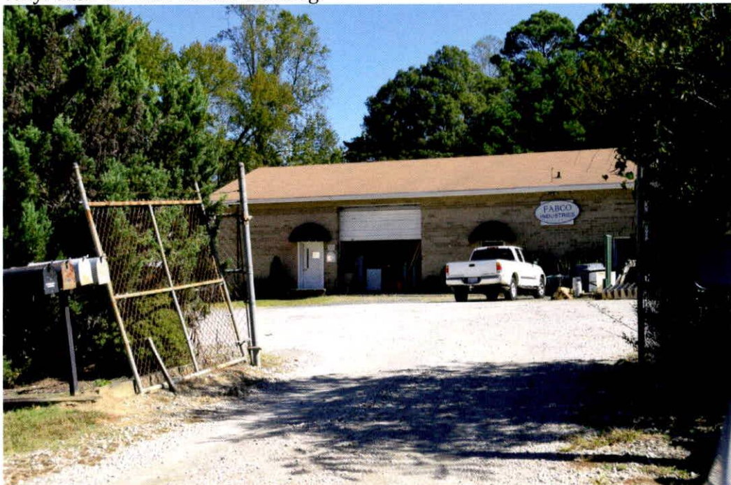
54b. Warehouse 2, 1971. Side-gabled, light-brown brick exterior with single-leaf personnel doors and overhead-lifting garage doors at west-facing façade.
