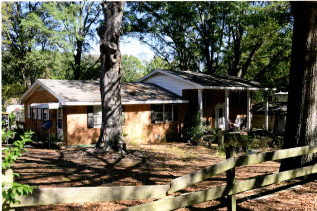
43a. House, 1967. Split-level brick-clad house with Mt. Vernon-style double-height front porch, paired 6/6 sash with faux shutters, broken pediment architrave at front door, and vinyl in gable end of two-story height section.
