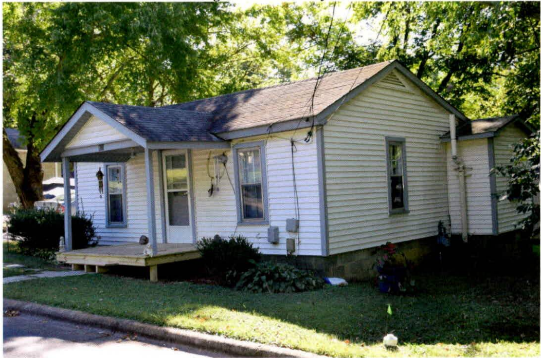
16a. House, 1910: One-story, single-pile, side-gabled vernacular house with 4/4 sash, vinyl siding, front-gabled replacement porch with wood deck and slender square porch posts, partially glazed front door, and brick stack at side elevation. Small, shed-roofed room at rear elevation is inset at east end but extends past west end of house, terminating with a side-gabled roof. Photos at the Wake County GIS website show asbestos shingle siding predated application of vinyl siding; the latter was applied after 2014.
