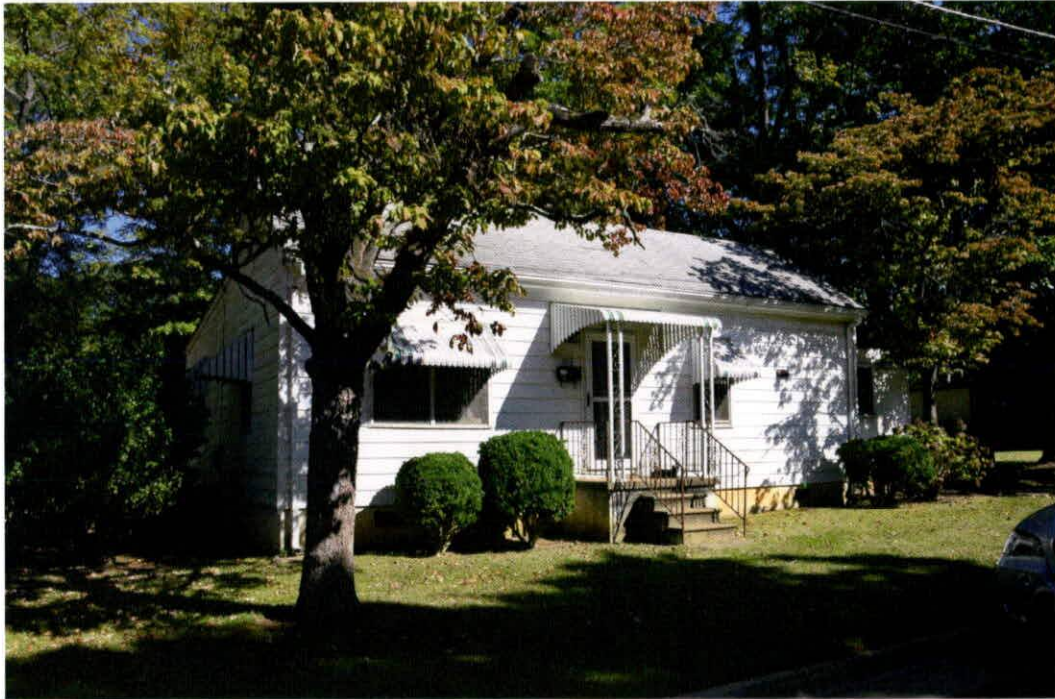
23. WA7160, House, 222 Hillsboro Street, 0764327116, ca. 1955.
