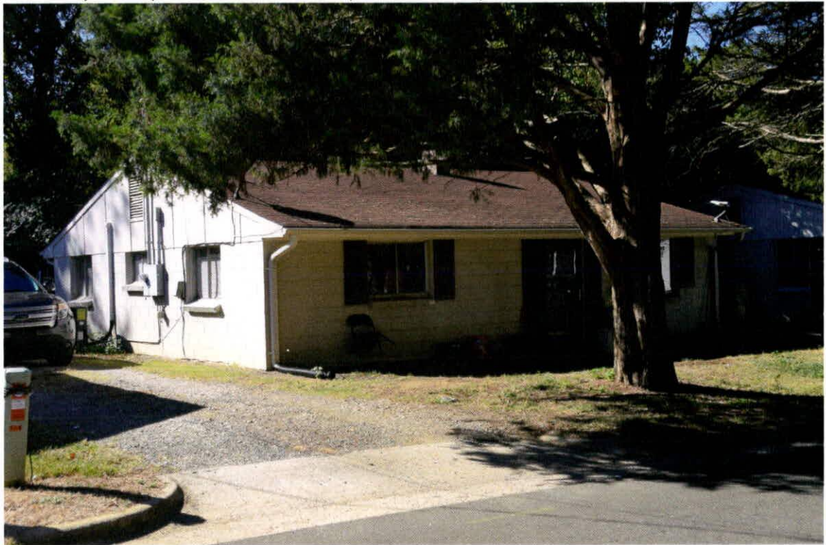
Concrete-block, side-gabled Ranch house with aluminum slider windows, faux shutters, and plywood in gable ends.
