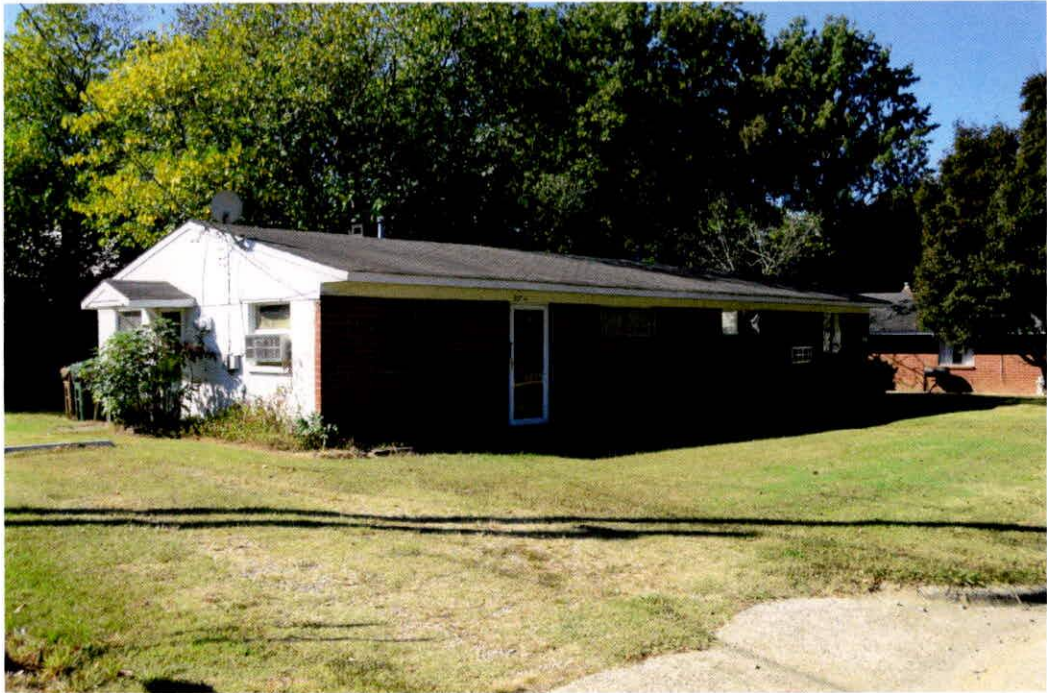
Concrete-block and brick-veneered side-gabled single-story house with plywood and vent in the gable ends and aluminum slider windows.
