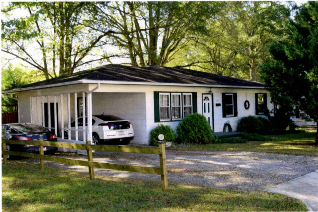
Ranch house with hip roof, replacement door and windows, asbestos-shingle siding, and inset carport.
