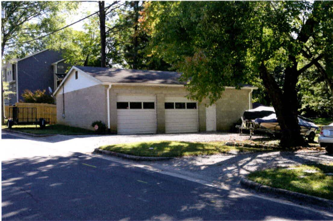
16b. Garage, ca. 1980: Concrete-block, side-gabled, two-car garage with façade perpendicular to the street; stands east of the house. Single-leaf paneled personnel door in south end of façade, next to overhead-lifting garage door. Plywood with centered vent in gabled ends above concrete wall. Asphalt roofing.
