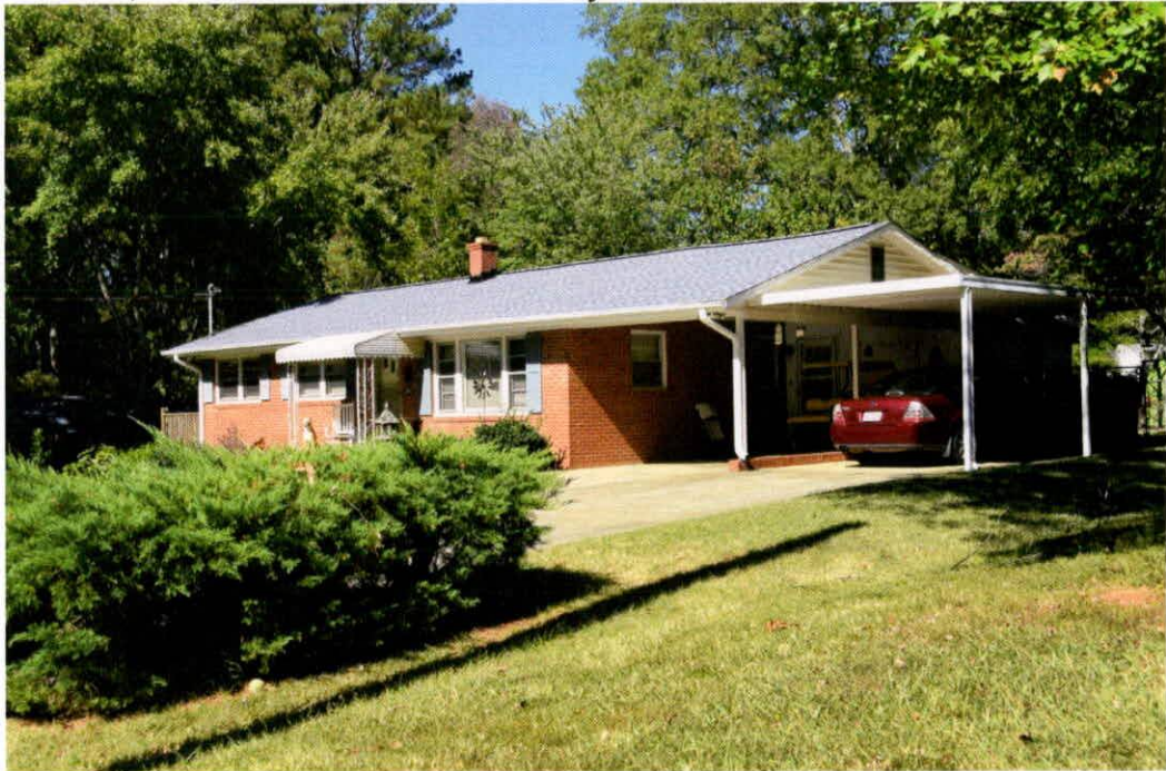
52a. House, 1959. Side-gabled Ranch house with brick exterior, vinyl siding in gable ends, 2/2 horizontal sash, and integrated carport.
