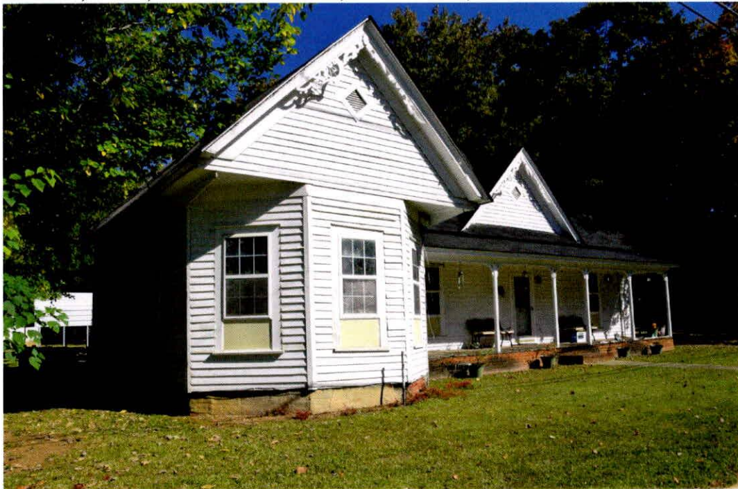
24. WA7159, House, 226 Hillsboro Street, 0764326146, ca. 1900.
