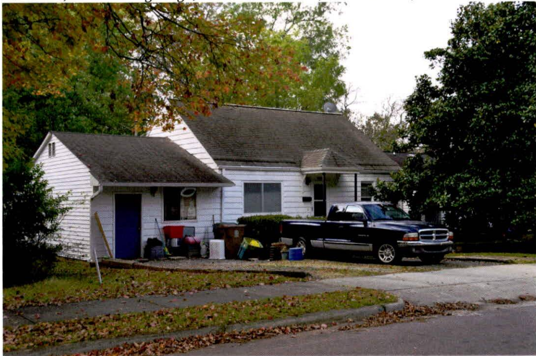
63a. House, 1949. Side-gabled Cape Cod dwelling with replaced windows, hipped porch on metal posts, aluminum siding, and added side wing or enclosed garage.
