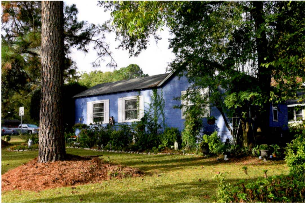
69. WA8265, House, 102 Adams Street, 0764428825, 1950
