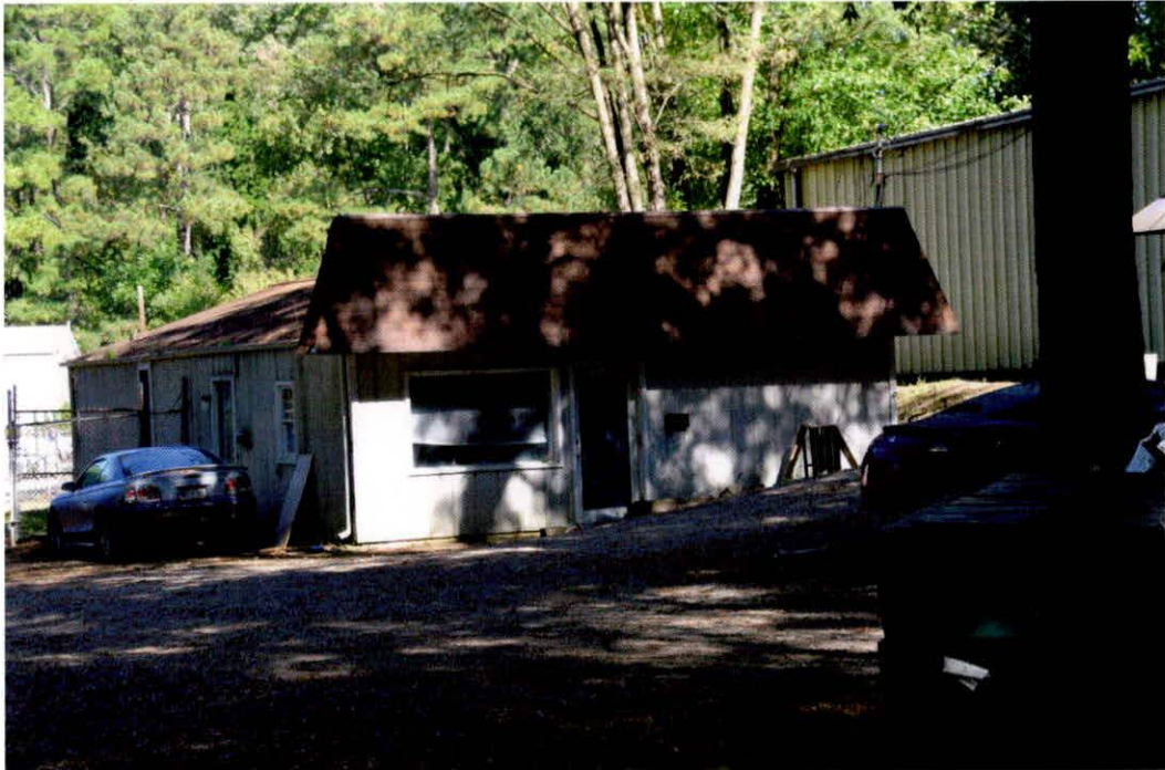
Gable-roofed warehouse with shingled parapet, picture window at façade, 1/1 sash at side elevations, personnel doors at façade and side elevation.
