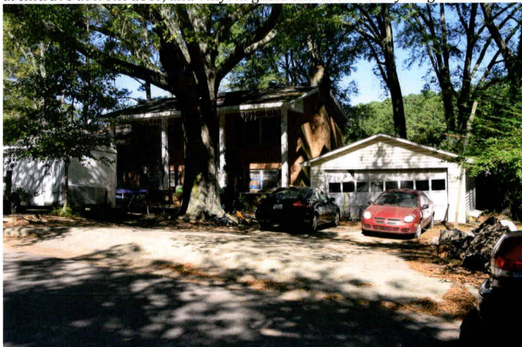
43b. Garage, 1967. Frame, front-gabled garage with vinyl siding and overhead lifting garage door with windows in upper portion of door.
