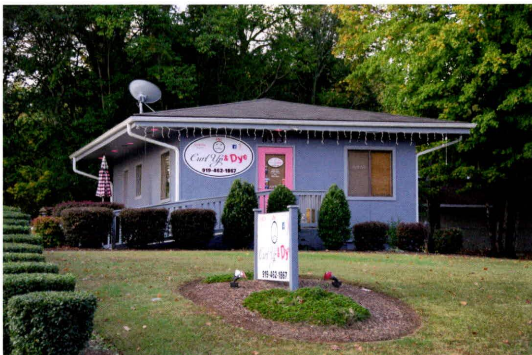
82c. Retail Building, 1982. Single-story hip-roofed building with replacement slider sash, single-light glazed wood door, ramp with wood rail and balustrade to front door, stucco exterior, deep boxed eaves.
