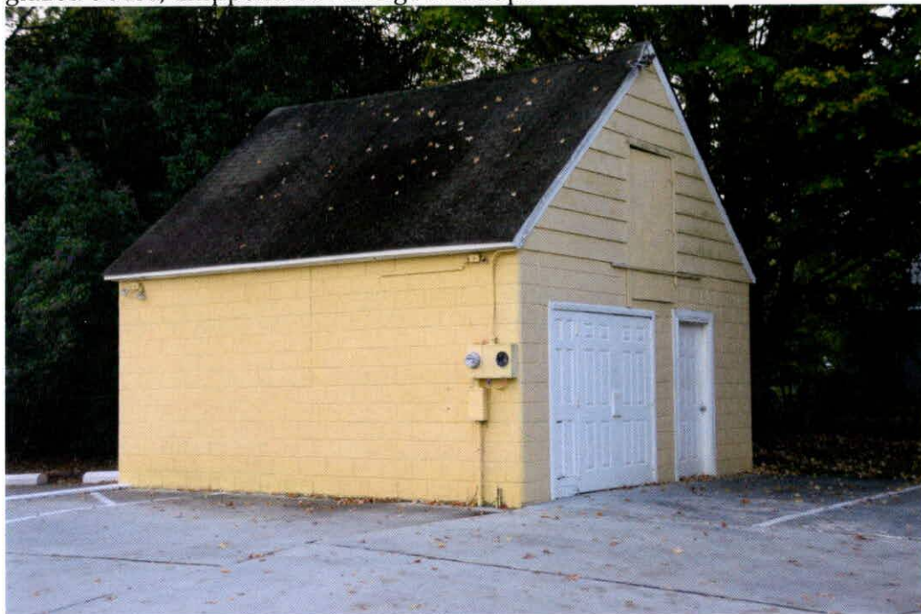
82b. Garage, 1960. Concrete-block front-gabled garage with fiber-cement siding in gable end, overhead lifting door and personnel door at façade, which faces west.
