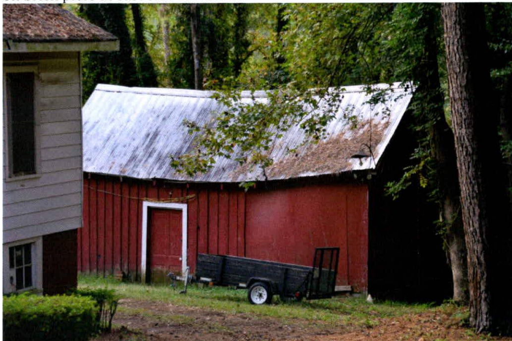
91b. Barn, ca. 1930. Large gabled barn with board-and-batten and plywood siding; standing-seam metal roofing; and single-leaf personnel door along north eave wall, board-and-batten doors on east gable end, and shed room along south eave wall. This building stands southwest of the dwelling.
