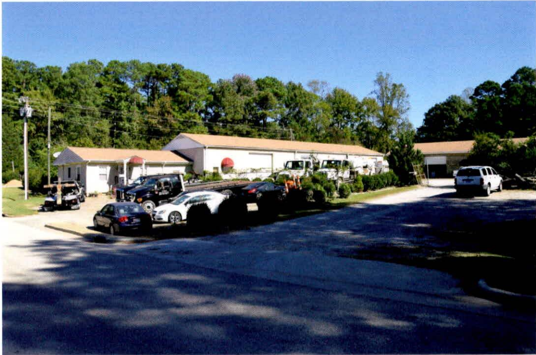
54a. Warehouse 1, 1972. Side-gabled, concrete-block warehouse with garage entrances in main block along south-facing elevation and personnel door under gabled portico in smaller gabled office block with vinyl siding and 6/6 vinyl sash at west end of building.
