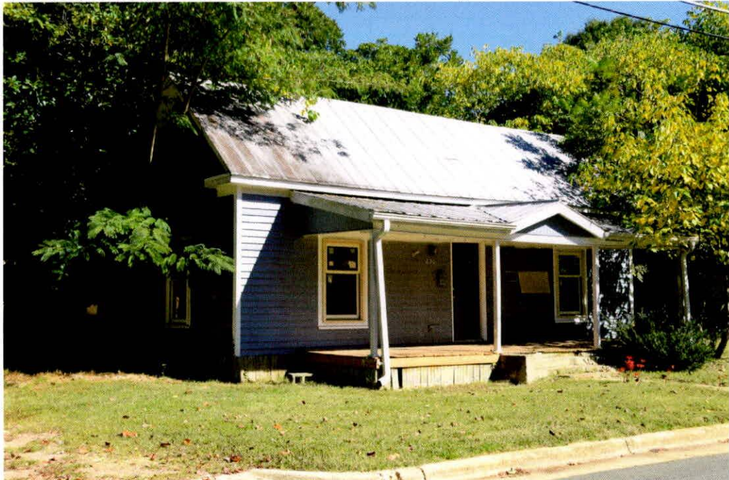
25. WA7158, House, 230 Hillsboro Street, 0764325157, ca. 1910.
