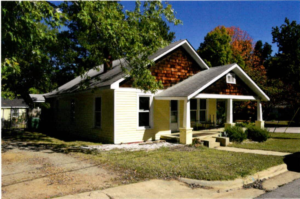
37a. House. One-story, front-gabled bungalow with a offset front-gabled front porch on tapered posts on brick piers that wraps around the east side. Small shed-roofed addition at rear. Windows and lap siding and shingles in gable ends are all replaced, but a 3/1 sash window remains in shed addition.
