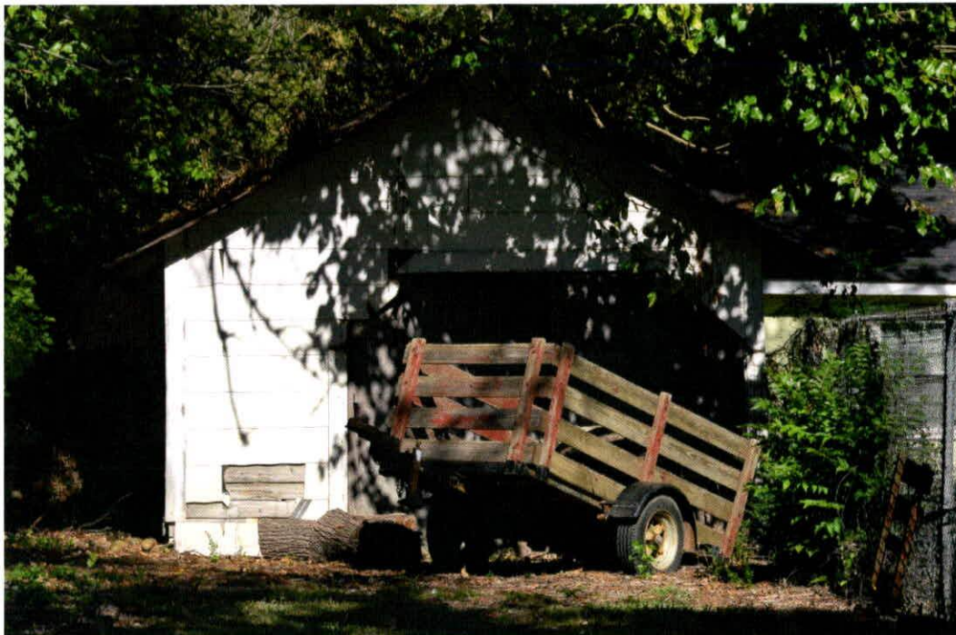
37b. Garage. Front-gabled, one-car garage with asbestos shingles over lap siding.
