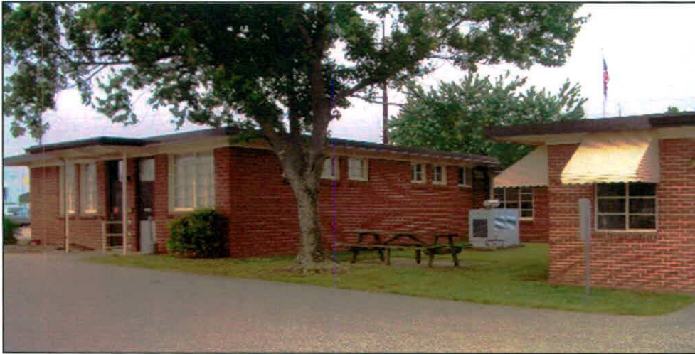
1: State Highway Patrol Logistics and Communications Headquarters, ca. 1955. East elevations pictured above, south and west elevations below.
