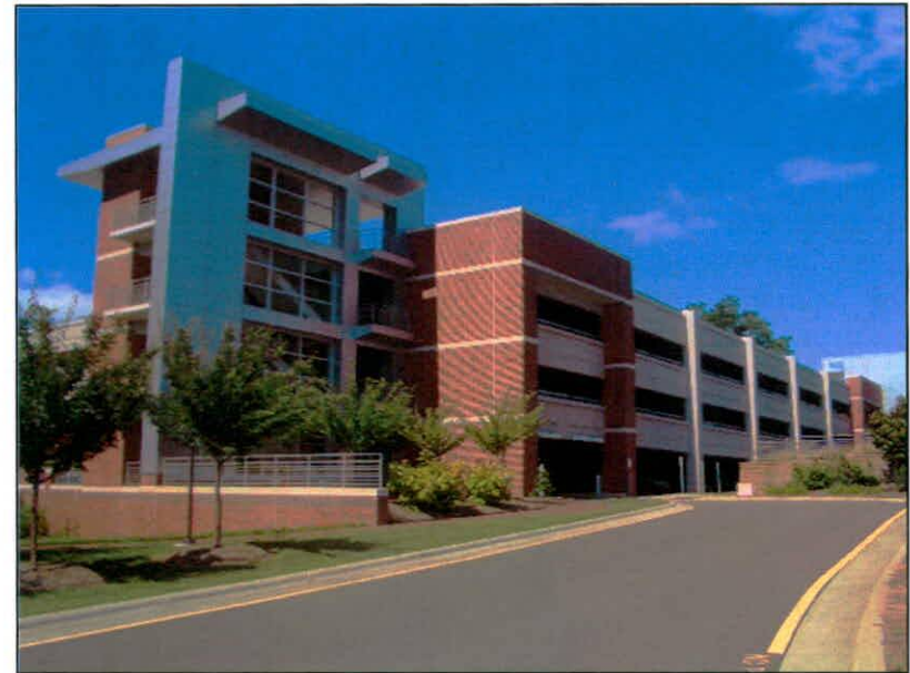
2: CVM Parking Deck, 2009, north elevation.
