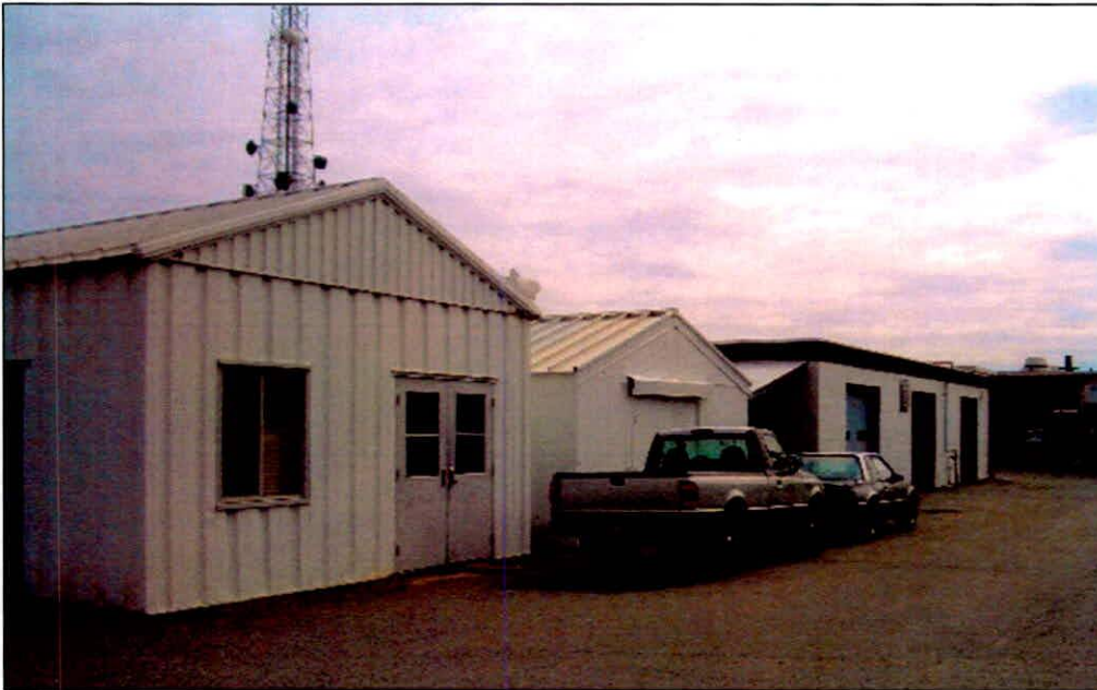
6: storage buildings and Body Shop, date unknown. Metal modular and concrete block buildings, with gabled and flat roofs. South elevations.
