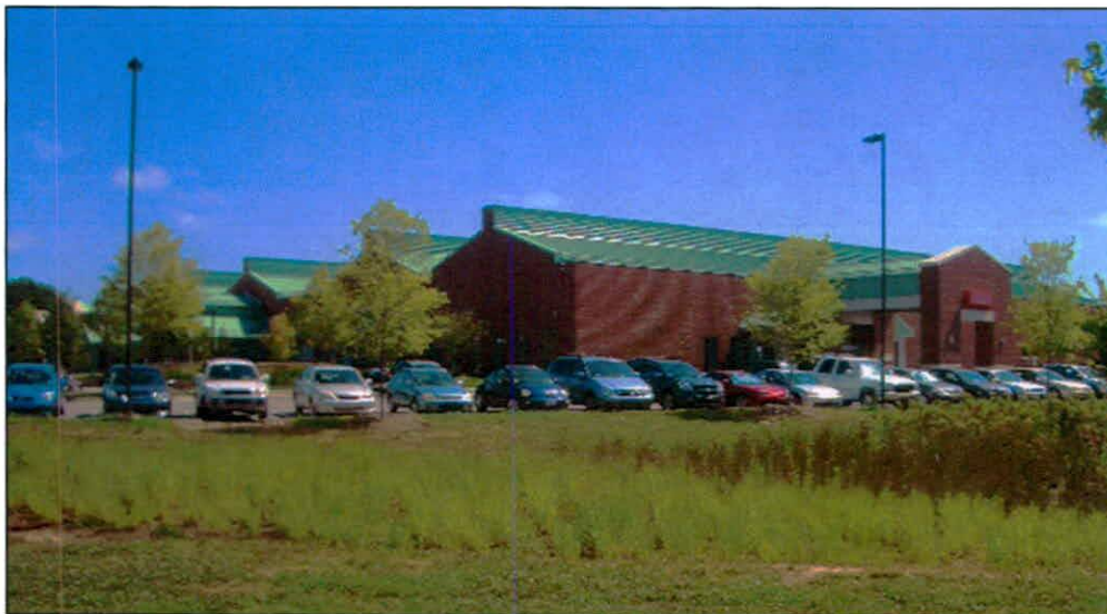
3: Terry Companion Animal Medical Center, 2008-2011, south and east elevations.
