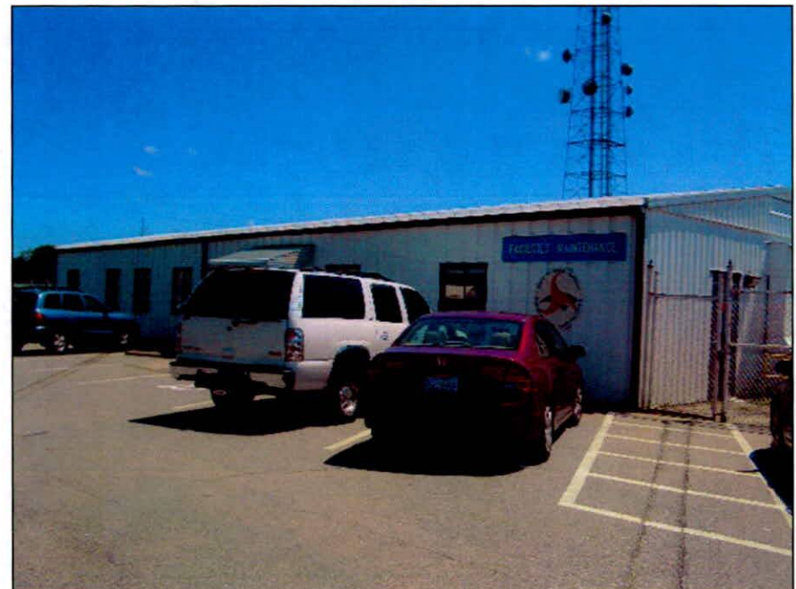
7: NCDOT Facilities Maintenance, ca. 1995. Metal modular buildings, with gabled roof pierce by garage and window bays. West elevation.
