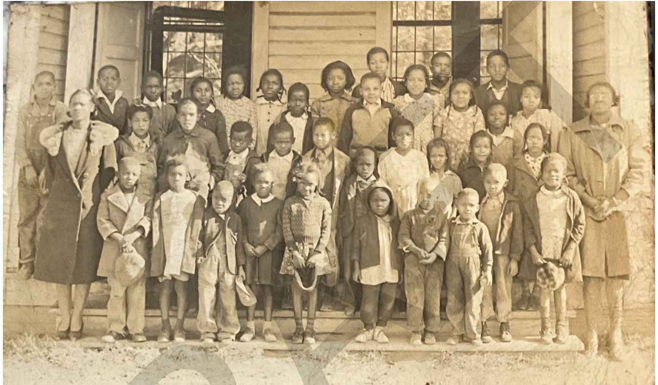
Exhibit A. Sunshine School, west elevation, undated photograph from the collection of former student Minnie Miller
