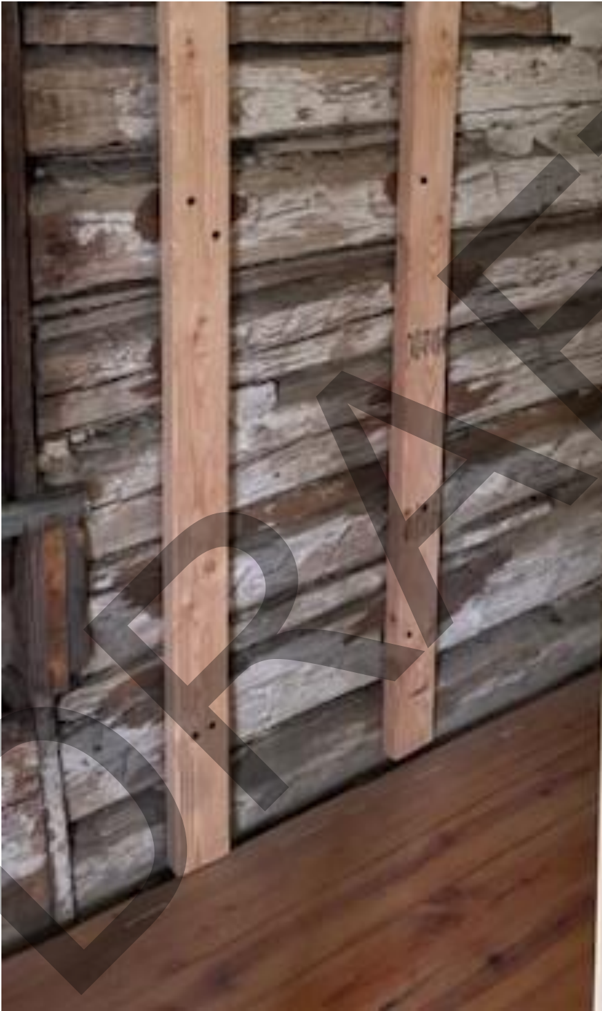
Figure 2. Log construction exposed, 2025.
