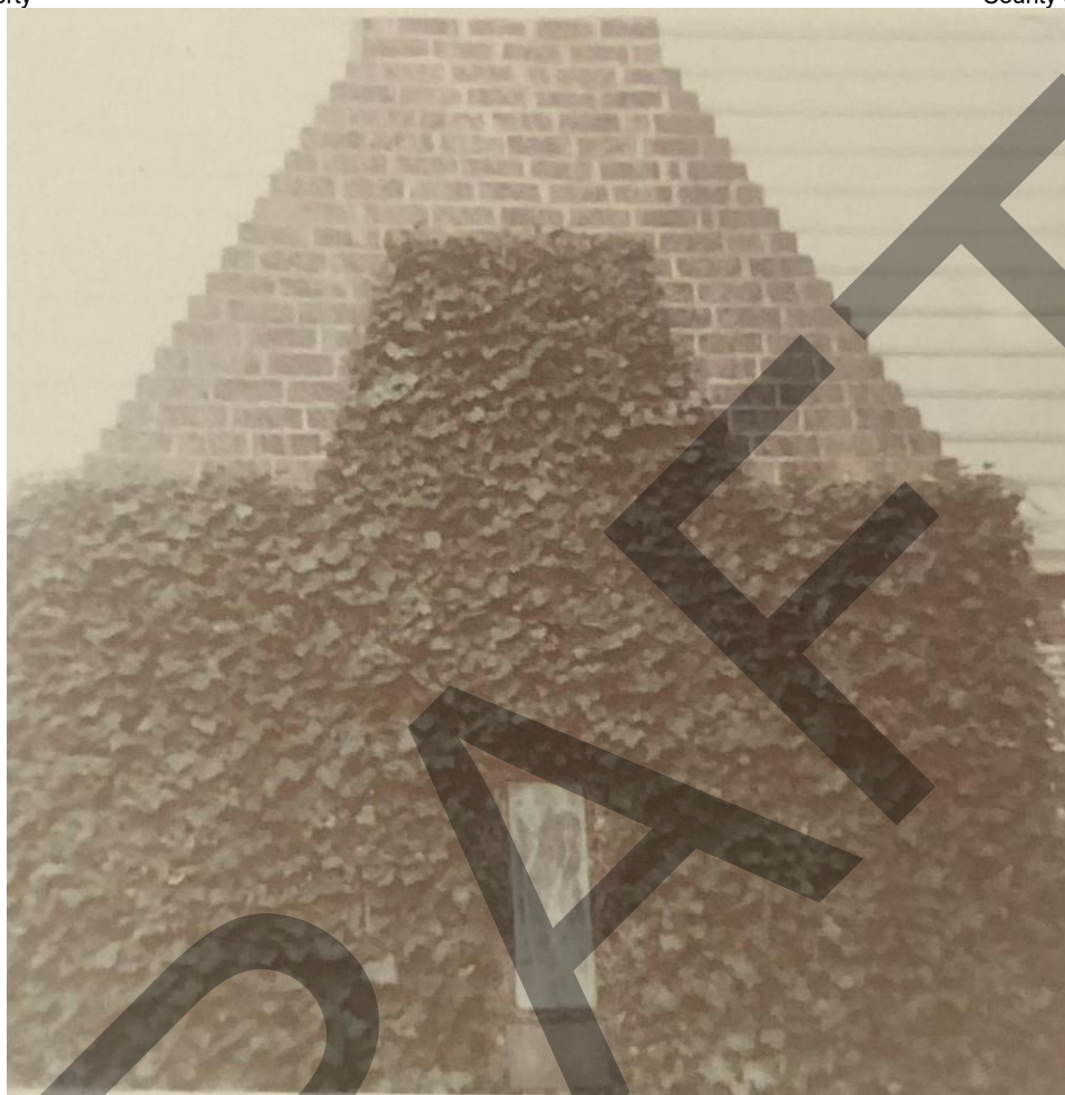
Figure 5: West end chimney at Moorefields, showing English ivy atop a layer of parge, 1968. Mary Claire Engstrom Photographic Collection, University of North Carolina at Chapel Hill, Wilson Library, North Carolina Collection: P0050, Print Box 3, folder 152.
