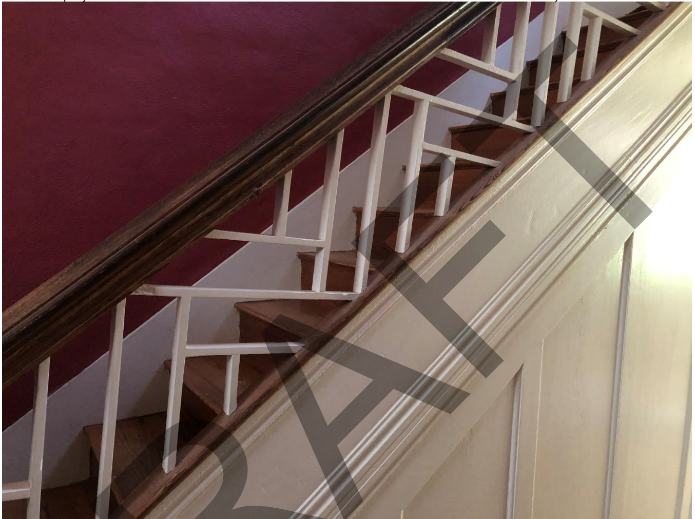
4 of 21. NC_OrangeCounty_MoorefieldsAD_0004. Interior, Moorefields house, side passage of main block, detail Chinese lattice stair rail, looking west.
