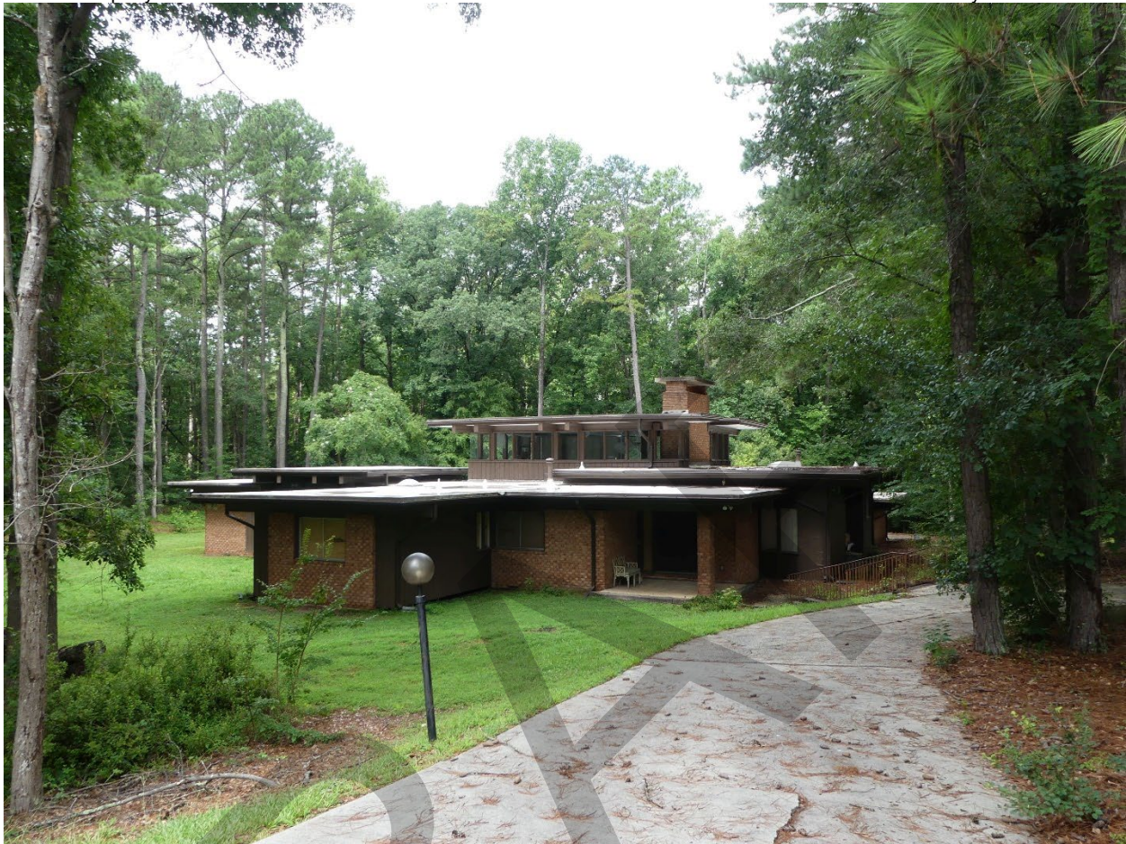
Photograph 32. (NC_Durham_Emorywood Estates_0032) Barbara and Dr. Donald Moore House at 920 Chowan Avenue. View looking southwest.
