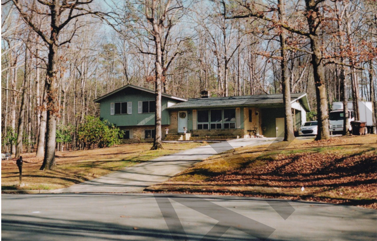
Photograph 31. (NC_Durham_Emorywood Estates_0030) 1112 Scranton Place, Ruth Pool House, looking northeast.
