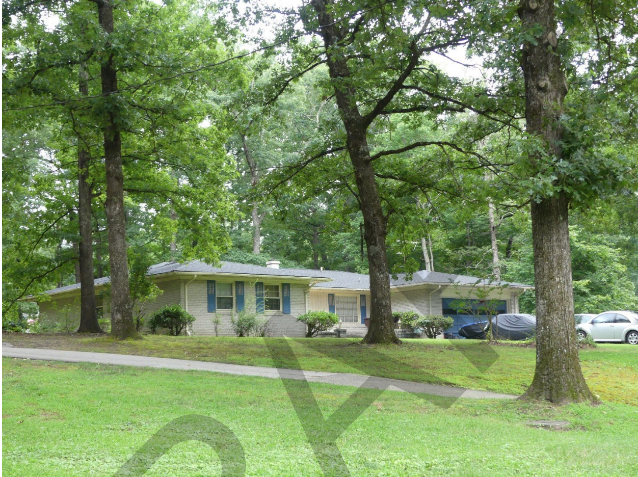
Photograph 25. (NC_Durham_Emorywood Estates_0025) 1108 Scranton Place, looking northeast.
