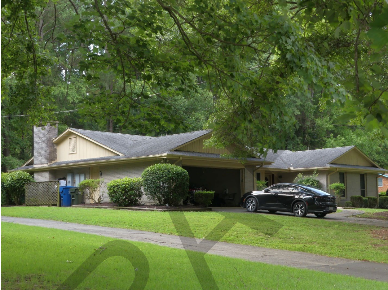
Photograph 26. (NC_Durham_Emorywood Estates_0026) 1006 Jerome Road, looking south.
