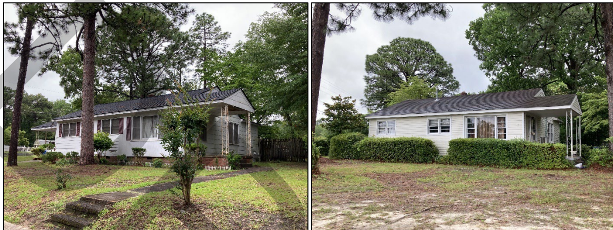
Figure 1. 1561 Seabrook Road at left and 1710 Seabrook Road at right.
