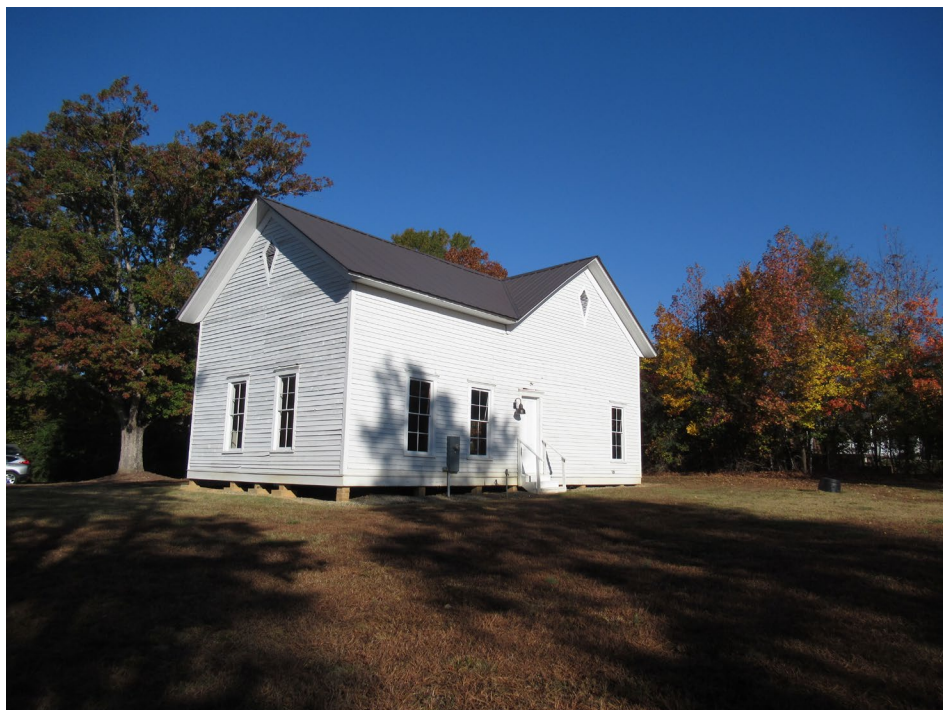
Exterior View to NNW
