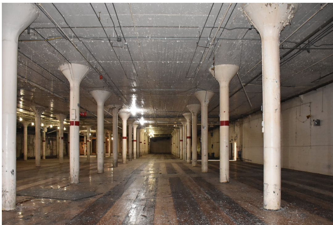
1923 First floor, looking east
