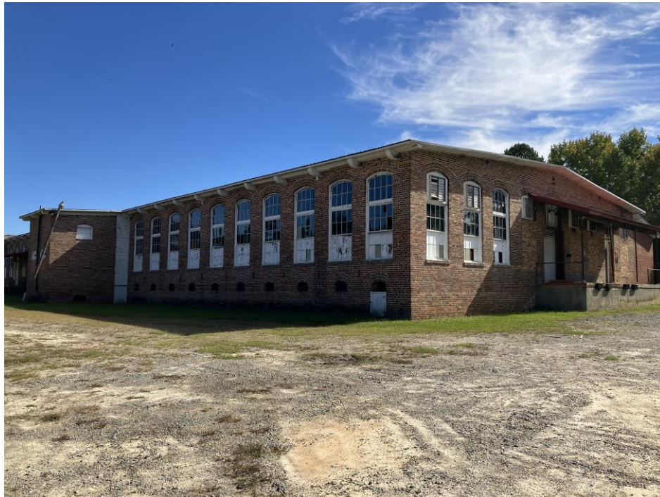
Mill, west corner, view to northeast
