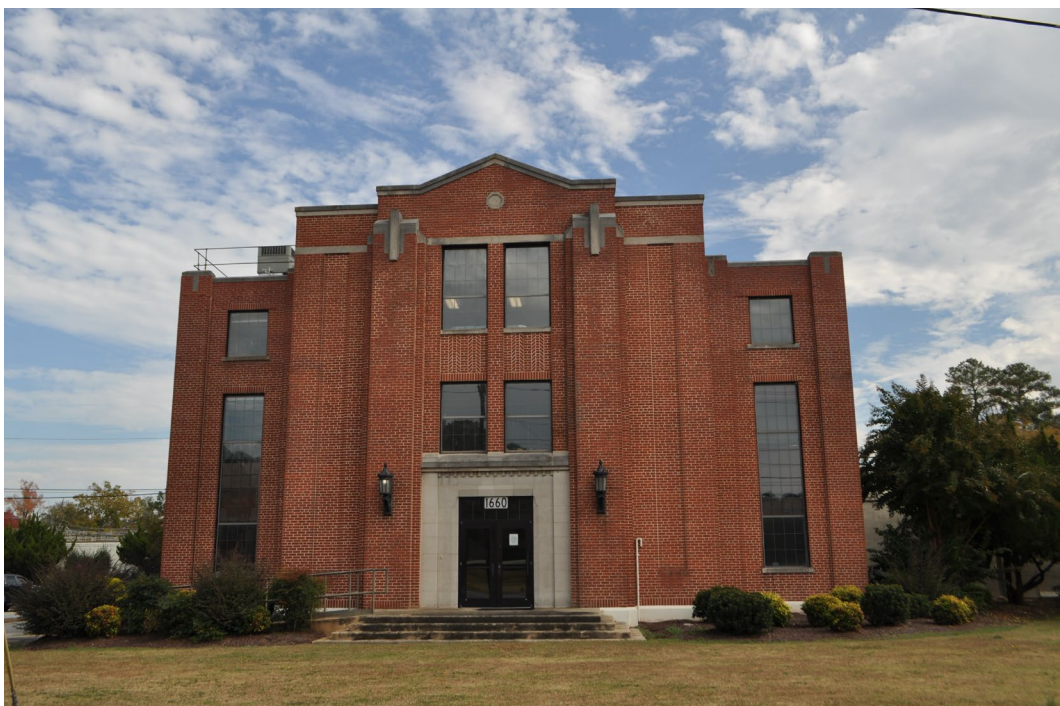
Sunset Avenue Water Treatment Plant, façade (west) elevation, east direction
