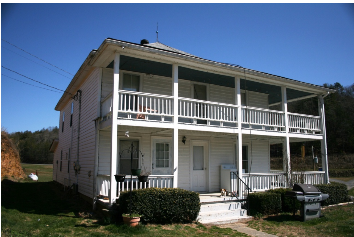
Hickey House, oblique rear view to northeast. New siding on rear elevation and original weatherboards under the porch
