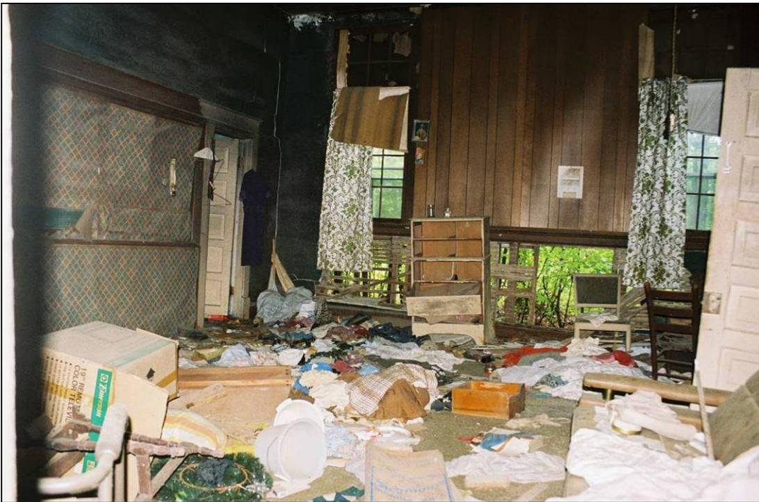
Plate 75. Chestnut School: central classroom; note original cross-panel doors, covered partition and window bank, and loss of plaster, lathe, and weatherboards beneath chair rail
