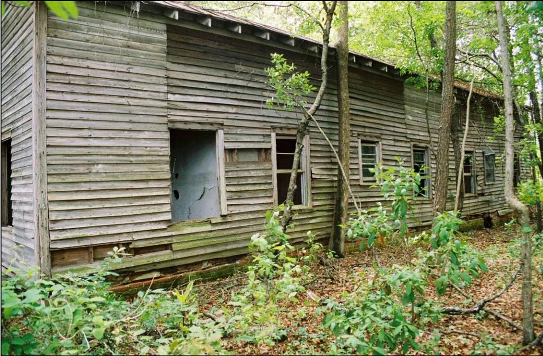
Plate 34. Keech School: east rear elevation with south classroom at left and north classroom at right; note heavy alteration of bays
