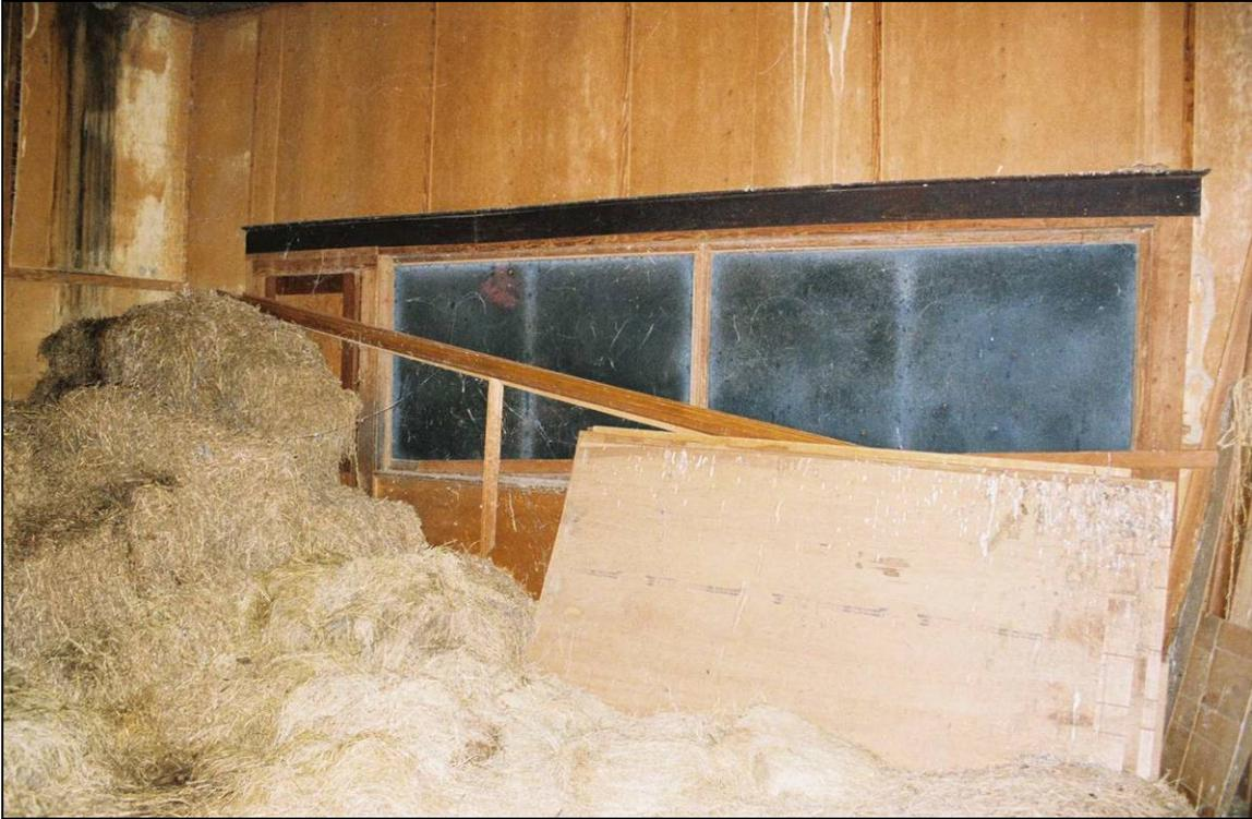
Plate 98. Springfield School: partition wall with sliding blackboard intact in north classroom
