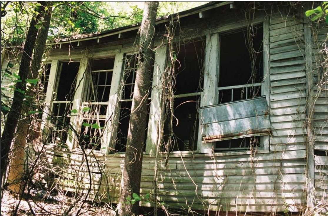
Plate 148. Bailey School: center classroom bank of windows at east rear elevation; cornerboard at far right marks original end of school
