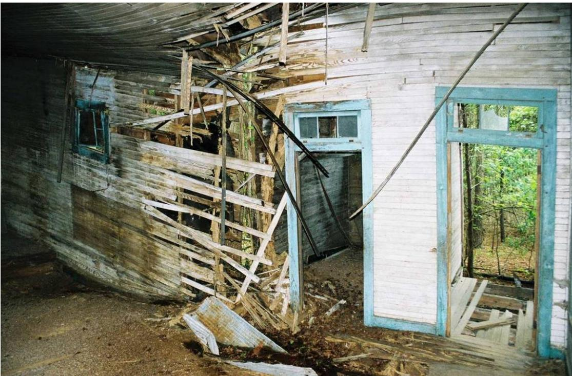
Plate 31. Coakley School: south classroom, exit at right and entrance to narrow cloakroom at center; note collapsing ceiling and wall of cloakroom at left
