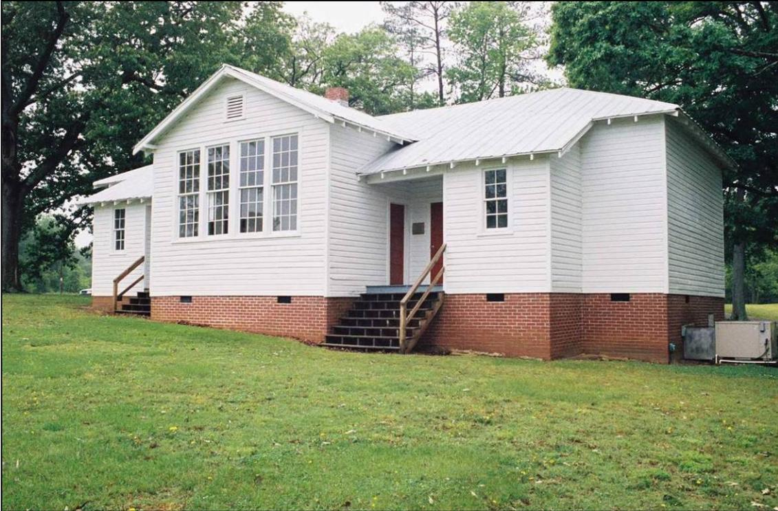
Plate 61. Allen Grove School: east front and north side elevations; note tall brick foundation fitted to current site
