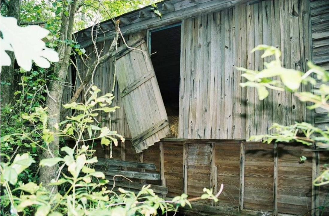
Plate 28. Coakley School: west rear elevation; note boarded-up windows of north classroom with weatherboards fallen beneath
