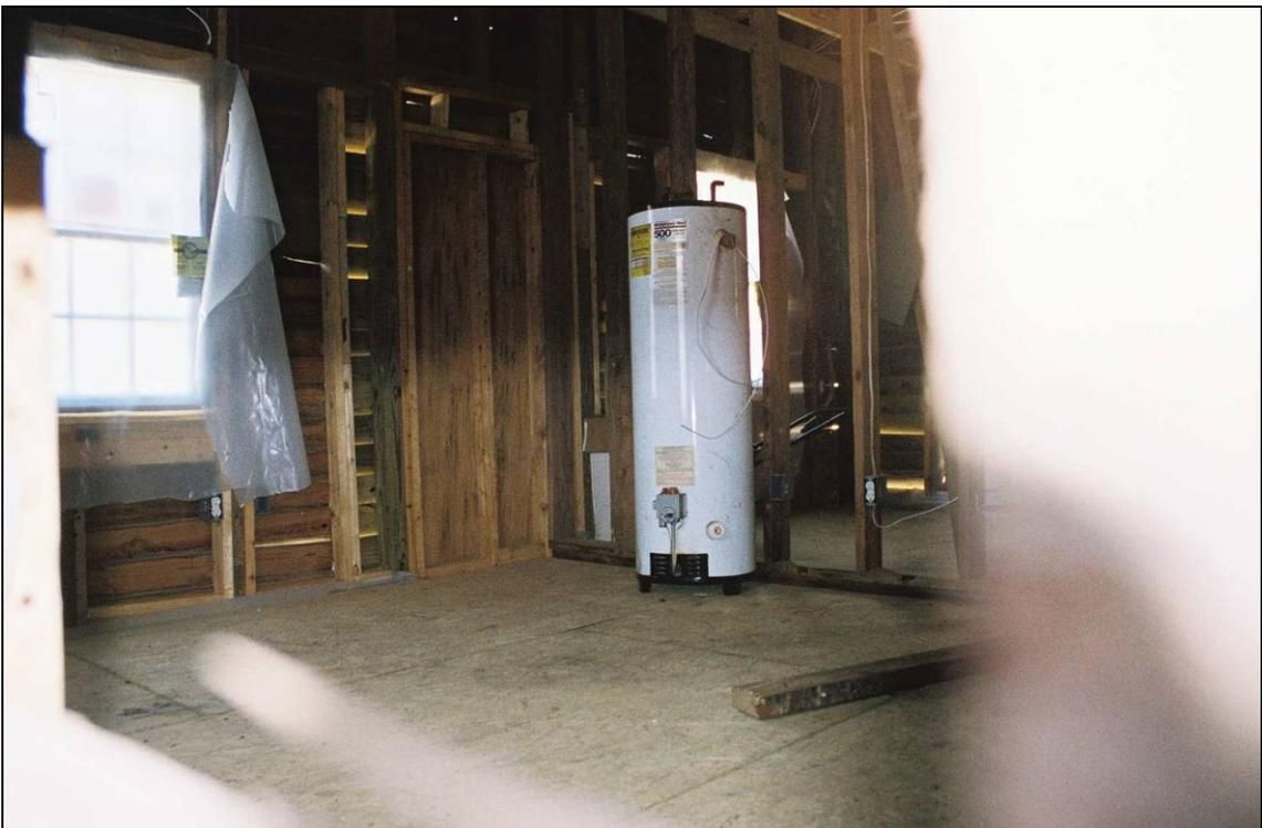
Plate 171. Evans School: interior stripped to studs; boarded-over front entry to left of water heater
