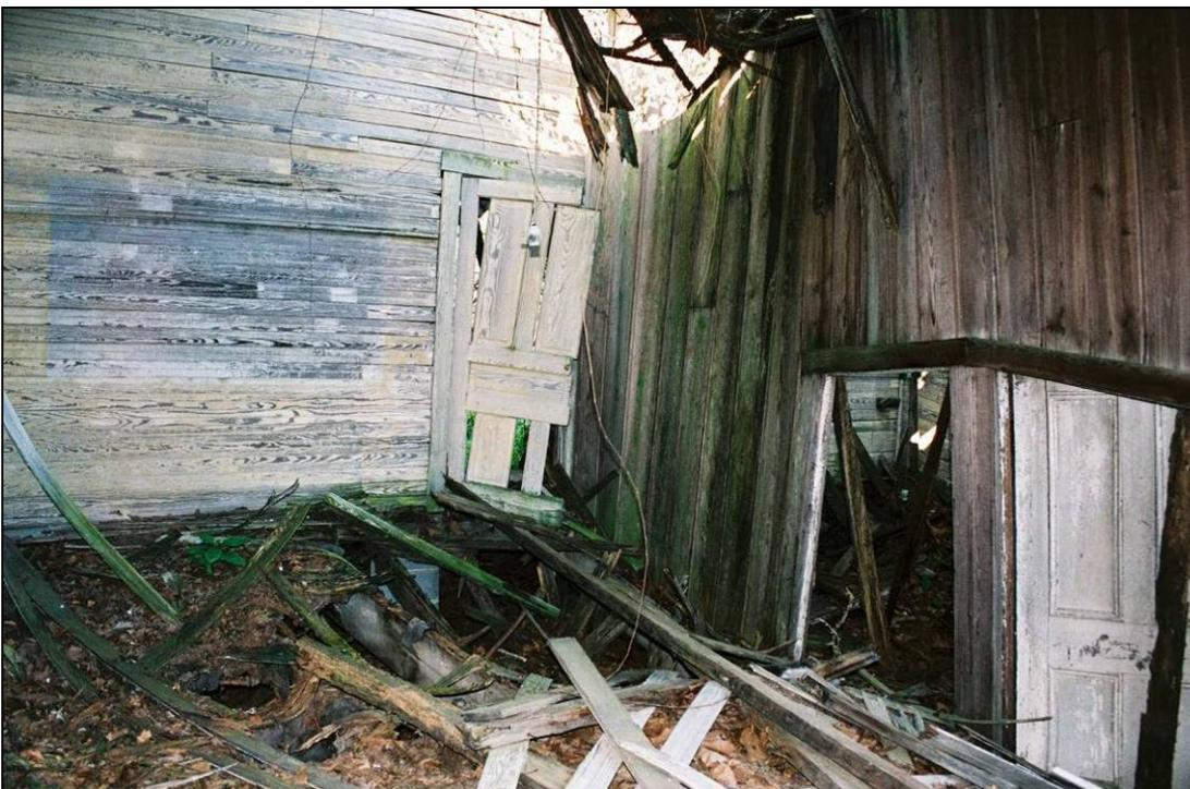
Plate 235. Bunn School: looking from partition wall into west classroom; note added partition walls dividing classroom into three rooms and ruinous condition of walls, roof, and floor
