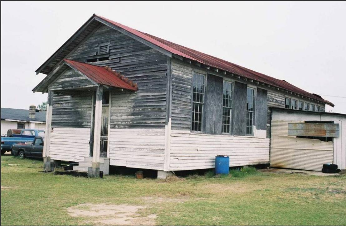
Plate 241. Dudley School: south front and east side elevations; note partial infill of window bank at front classroom
