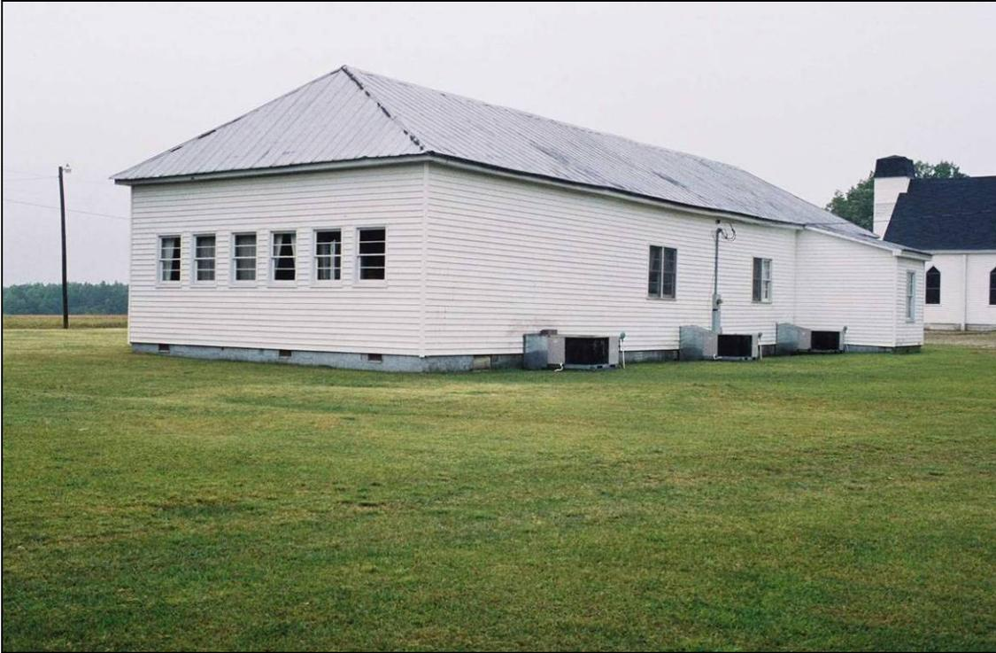
Plate 85. Marys Chapel School: east side and north rear elevations; note alteration of bays, including addition of six windows to side elevation and removal of three banks of windows from rear elevation
