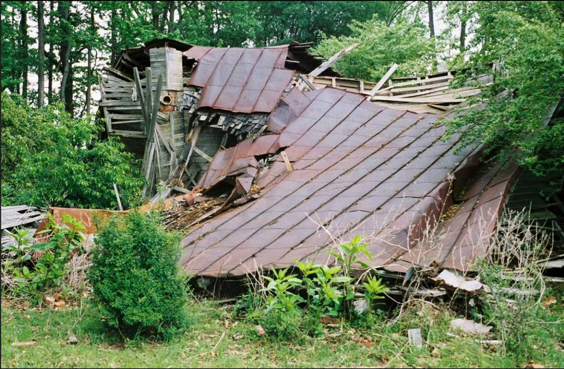
Plate 46. Wimberly School: seam-metal roof upon collapsed frame and ground
