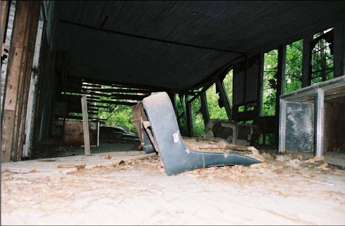
Plate 254. Sims School: looking from fallen west side wall into west classroom and, at rear, east classroom; note absence of partition wall and damage to exterior walls
