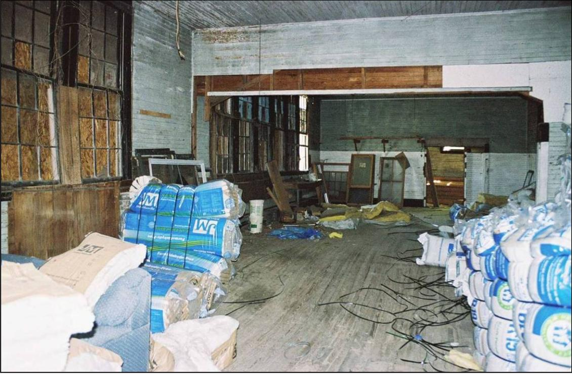
Plate 180. Jeffrey School: looking from northeast front classroom through missing partition to southeast front classroom; note banks of windows, floors, and beaded boards in place
