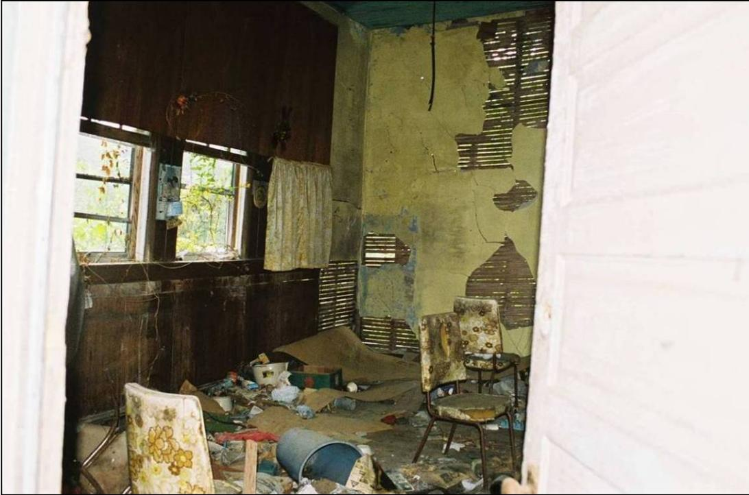
Plate 74. Chestnut School: industrial room; note collapsing plaster walls and altered and partially boarded-over bank of windows
