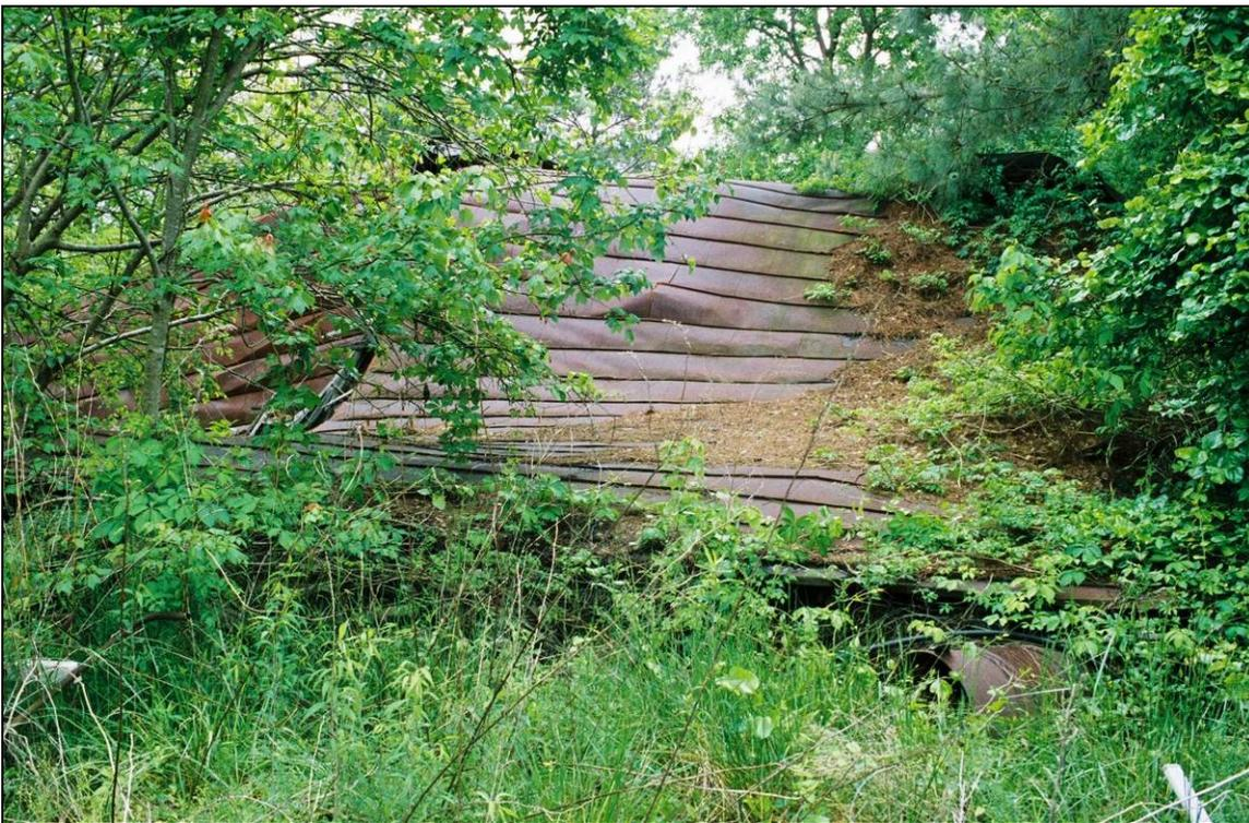
Plate 38. Lawrence School: seam-metal roof settled upon collapsed frame
