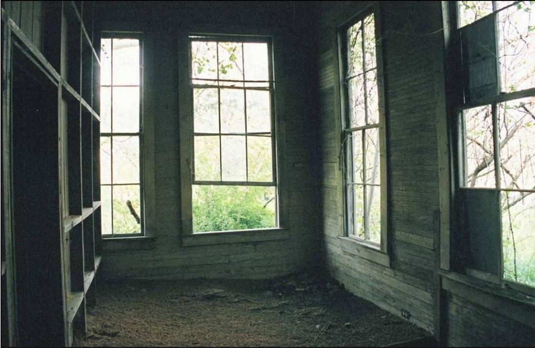
Plate 230. Bunn School: eastern half of industrial room with later-added partition wall at left; windows at right are likely later insertions
