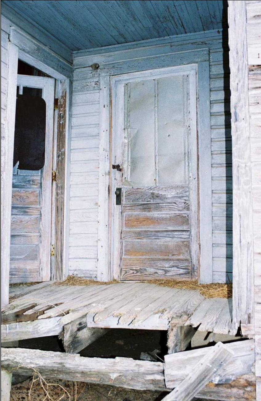
Plate 100. Springfield School: cross-panel doors to north classroom at center and industrial room on right; glass panes completely hidden by sheet metal at classroom door
