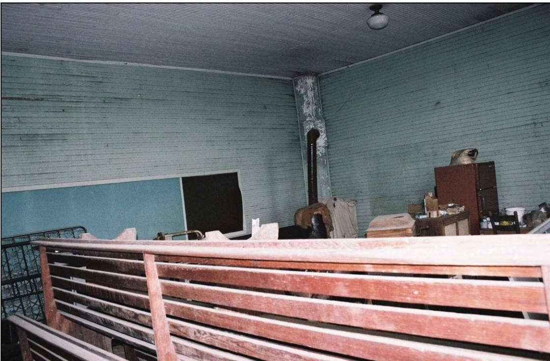
Plate 244. Dudley School: front classroom with long blind wall at left and partition wall between classrooms at right; note unbroken application of beaded boards at walls, ceiling, and partition
