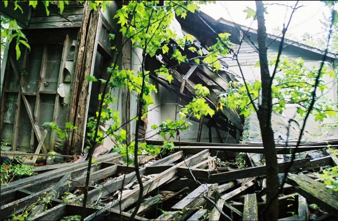
Plate 70. Chestnut School: largely collapsed east side elevation and classroom; note weatherboards at gable of original east end of building
