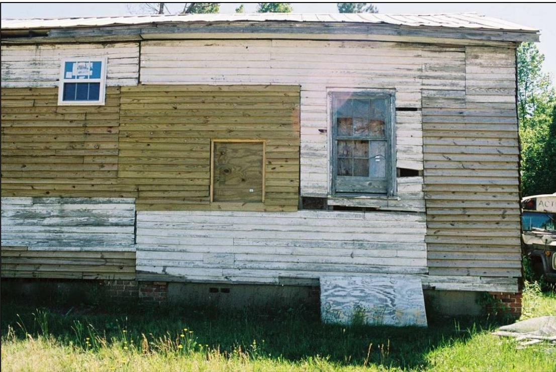
Plate 169. Evans School: east side elevations with infilled bays, later sash and, at right, last remaining original window sash
