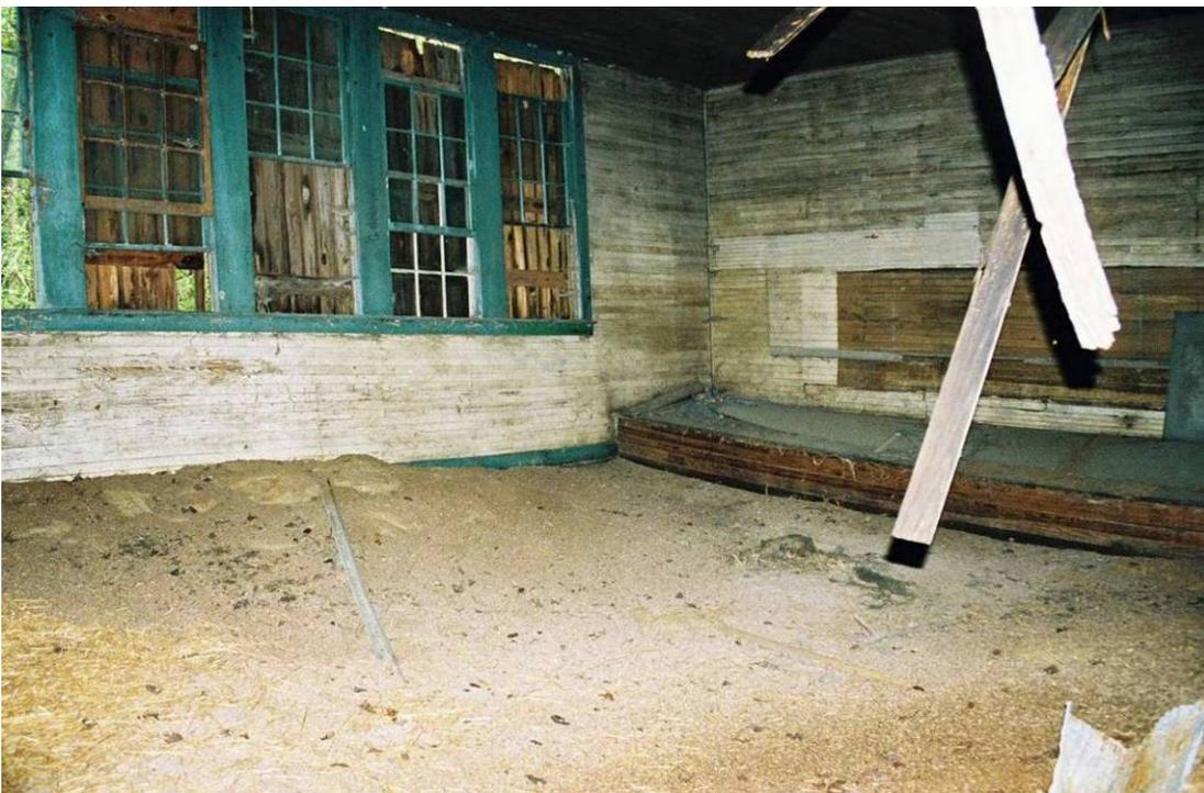
Plate 29. Coakley School: south classroom with bank of 9/9 sash at left and stage and ghost of blackboard at right
