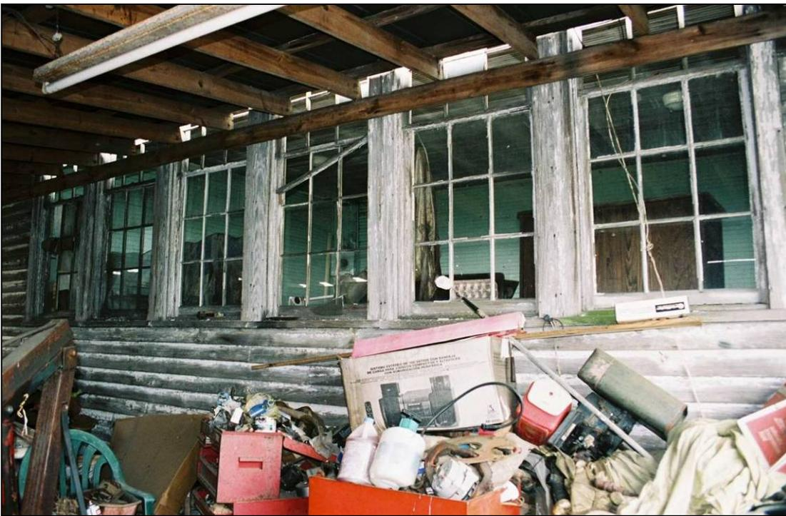
Plate 242. Dudley School: rear classroom with beaded-board walls, partition, and ceiling visible through bank of windows
