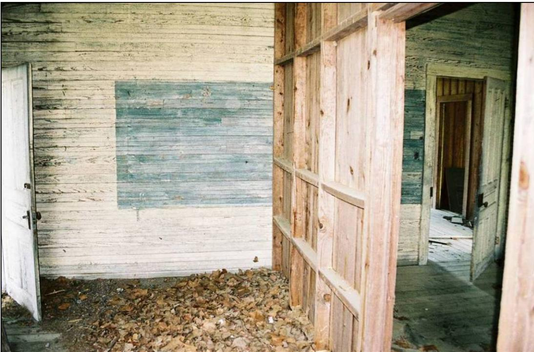
Plate 231. Bunn School: eastern half of industrial room with later-added partition wall at right; note ghost of blackboard extending to either side of partition
