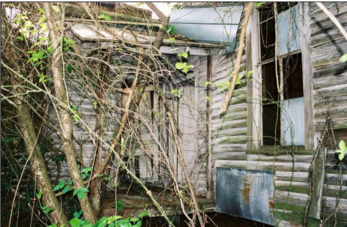
Plate 225. Bunn School: entries to west classroom and industrial room off of porch, at center and later-added 4/4 window at side of industrial room, at right
