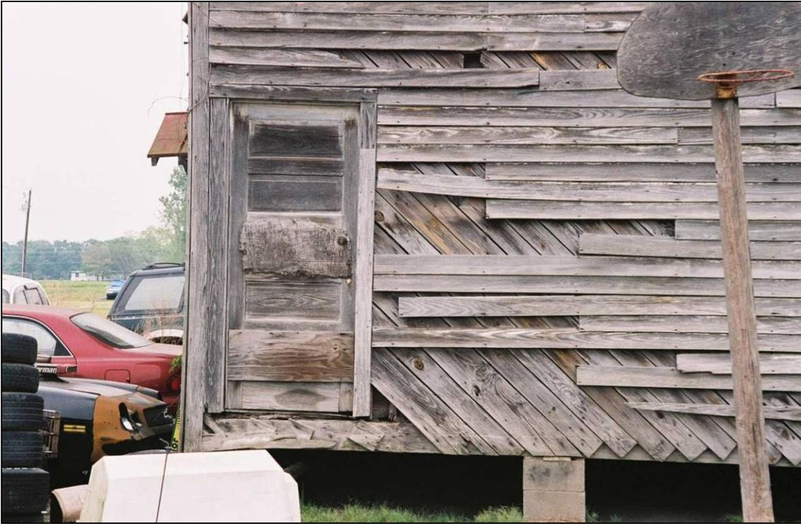
Plate 238. Dudley School: rear of west side elevation; note placement of door hard against corner and exposed vertical sheathing beneath weatherboards
