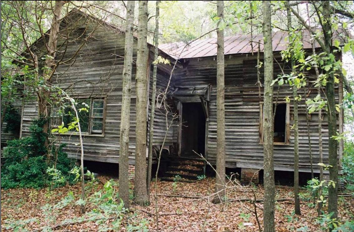
Plate 32. Keech School: west front elevation with south classroom/cloakroom at right, industrial room projecting at center, and north classroom/cloakroom partially visible at far left; note industrial room's later bay window
