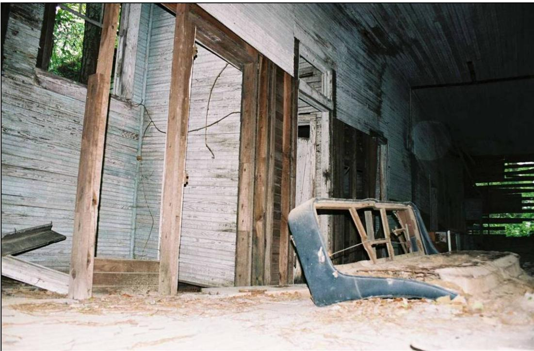
Plate 255. Sims School: looking from fallen west side wall into west classroom; note loss of wall at west cloakroom and loss of beaded-board siding beyond
