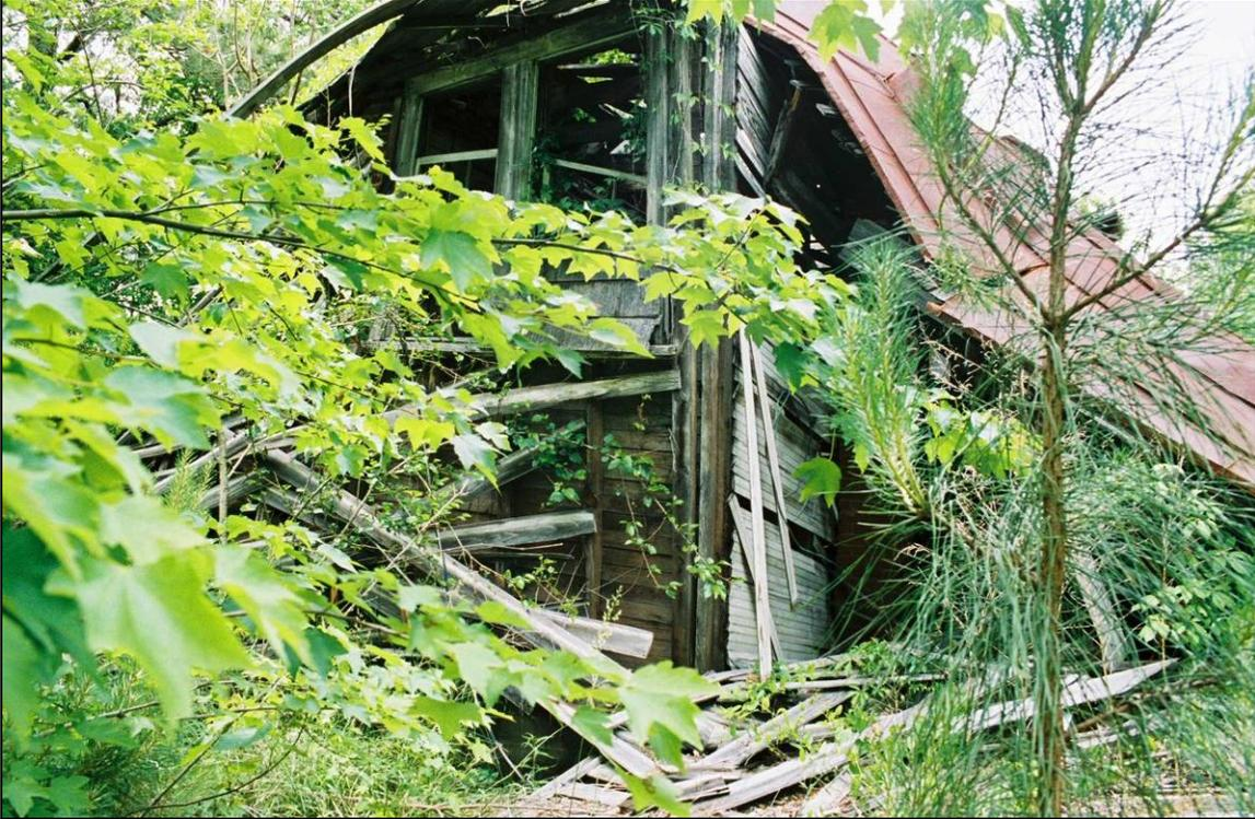
Plate 39. Lawrence School: collapsed frame; note apparently later-added paired windows in gable peak
