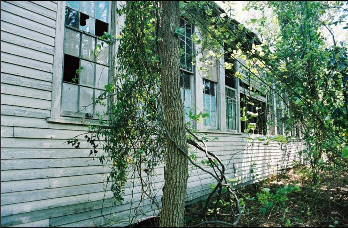
Plate 178. Jeffrey School: west rear elevation of main block; note loss of some weatherboards between the two banks of classroom windows
