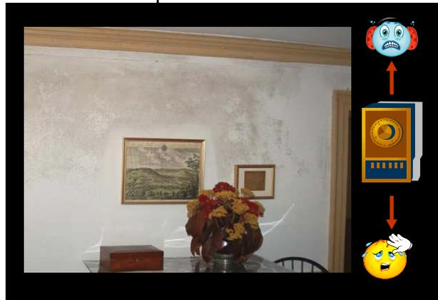
Uncontrolled roof rainwater runoff is a leading and often overlooked cause of indoor humidity problems in buildings. If you have ever installed a rain barrel to a gutter system on your home you may be surprised just how quickly the rain barrel fills-up. One inch of rain on 1,000 square feet of roofing will produce 600 gallons of water. Where does all of this water go?
