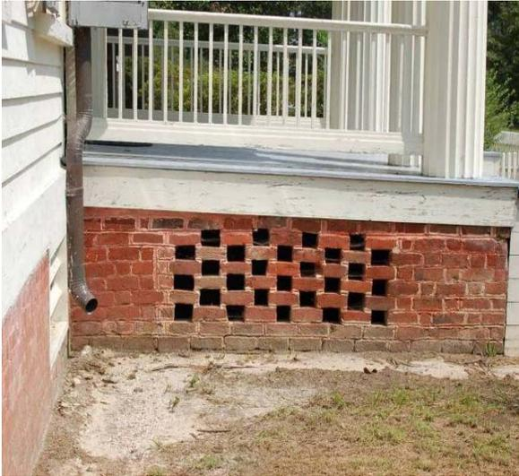
With poor site drainage rainwater runoff can wick-up into older masonry walls and seep under the building into the crawlspace or basement. Even if your home has gutters, downspouts that discharge water around a foundation may be causing moisture problems.
