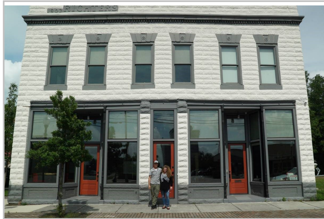
Richter Building Wilmington, New Hanover County
